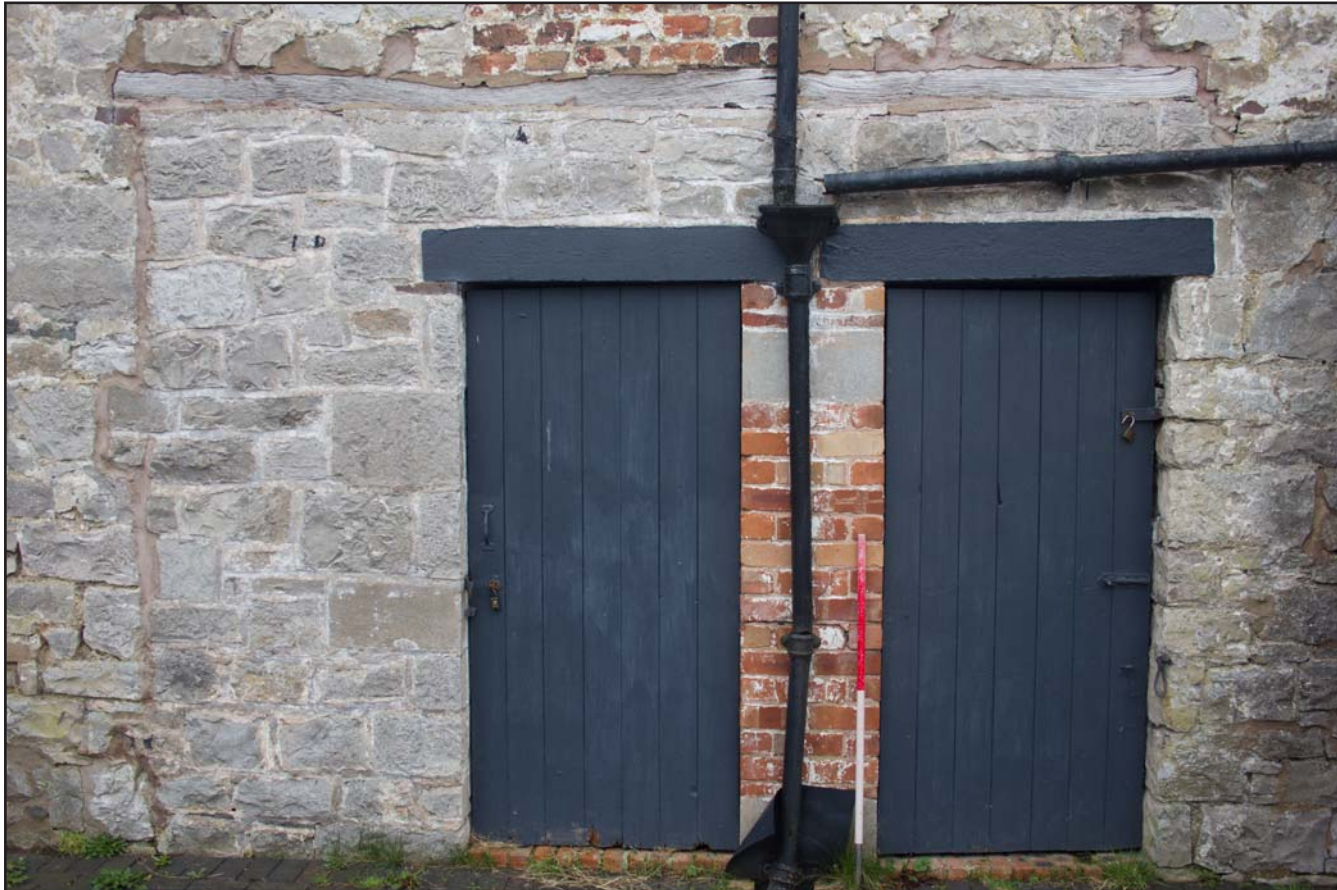
Plate 14: Stone infill of former cart doorway on southern elevation, of Coach House at Hafod Ynys, Rhewl, Denbighshire - from the south - 1.00m scale
