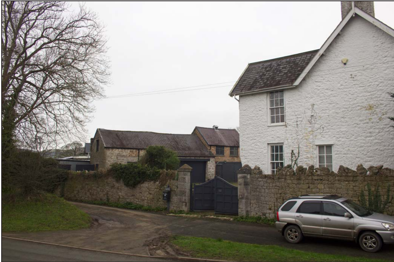
Plate 01: Context Shot of Coach House at Hafod Ynys, Rhewl, Denbighshire - from the southwest - no scale
