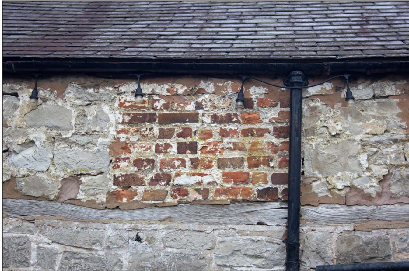
Plate 15: Brick infill of window above former cart doorway on southern elevation, of Coach House at Hafod Ynys, Rhewl, Denbighshire - from the south - 1.00m scale
