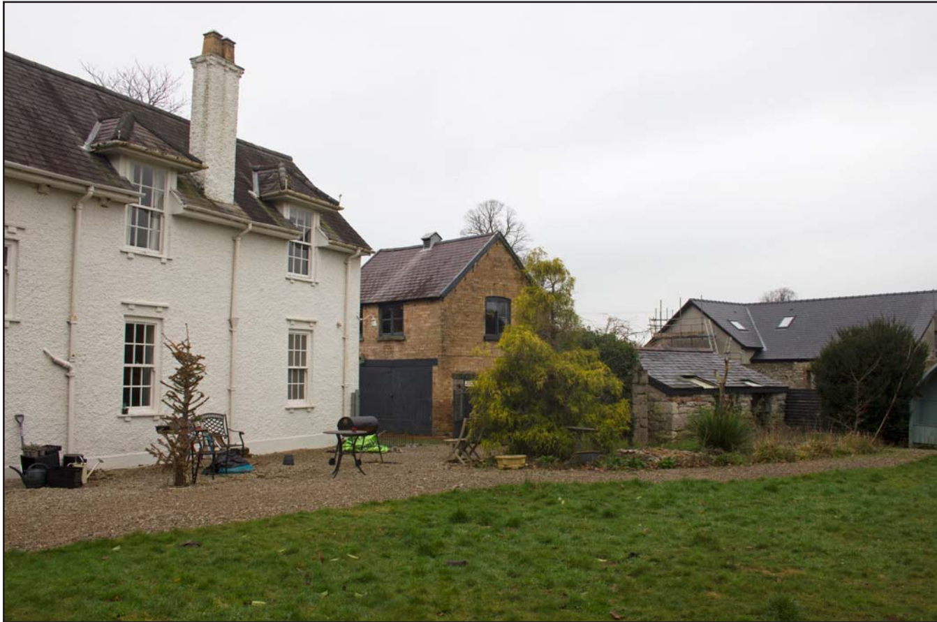
Plate 04: Context Shot of Coach House at Hafod Ynys, Rhewl, Denbighshire - from the southeast - no scale
