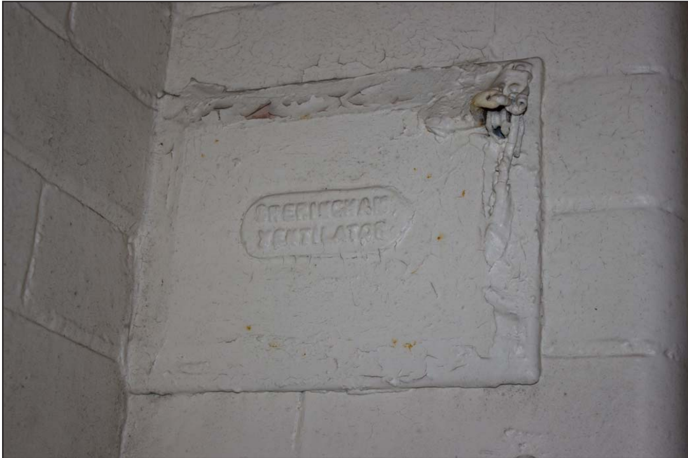
Plate 91: Cast iron ventilation hatch within Operations Room, Miner's Rescue Center, 3-5 Maesgwyn Road, Wrexham - from the north - no scale
