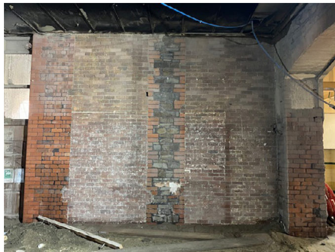
The scarring of the two infilled doors on the north side of the Market Hall.
