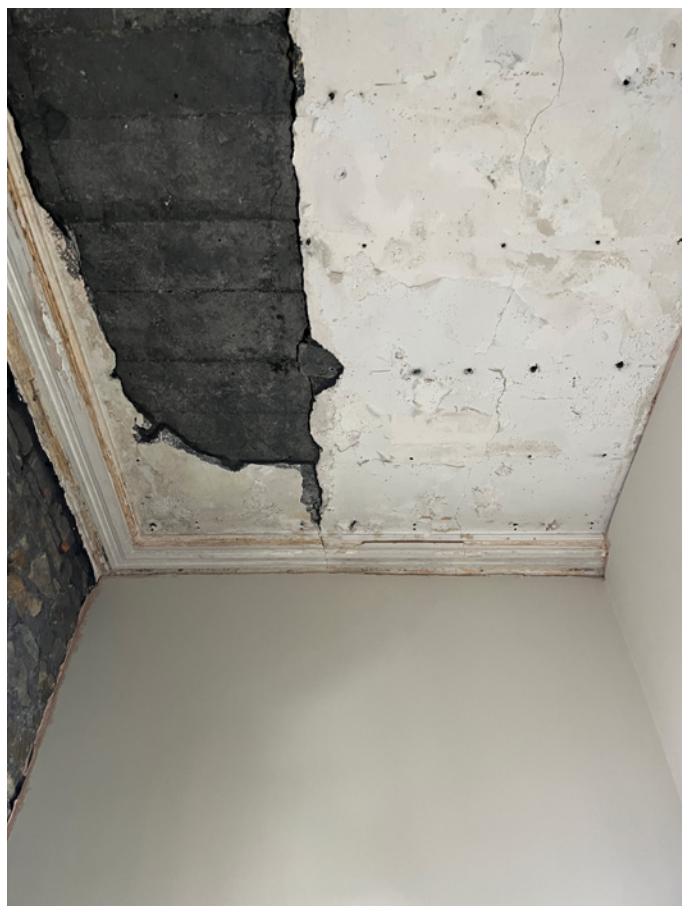
The damaged cornice and plaster ceiling to the staff office which was repaired to a matching decorative scheme.
