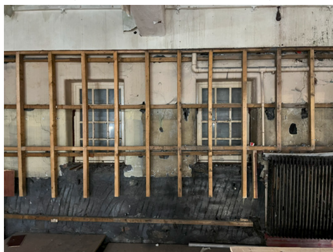
The four 19th-century windows uncovered behind modern wall linings in the Main Hall beneath the balcony.
