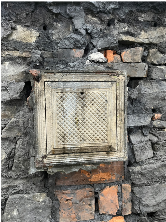
The wall vents revealed from behind the 1970s panelling in the Main Hall.
