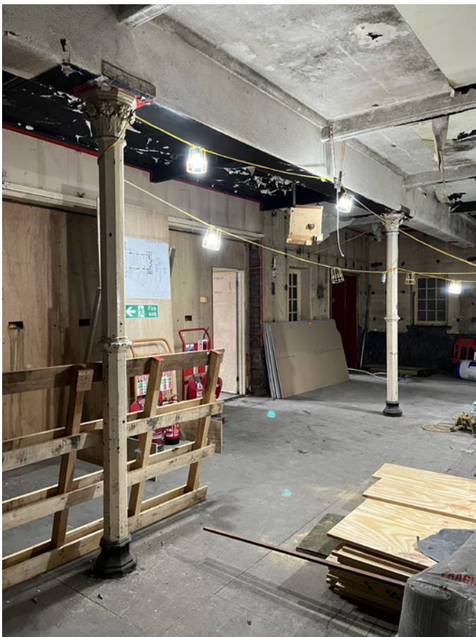
The cast iron columns in the Main Hall.
