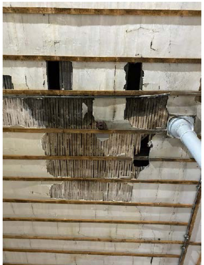
The historic lath and plaster supported by timber battens.
