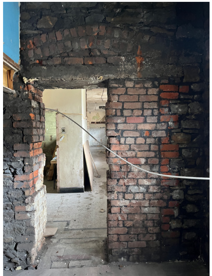
The adapted opening partially infilled with brick, with a segmented brick arch above, previously obscured behind modern wall coverings.
