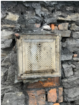
005 - Cast Iron Wall Vents within C19 Wainsc...
