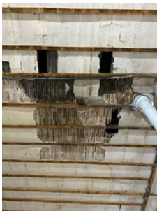
021 - Former Plain Lath and Plaster Ceiling to ...
