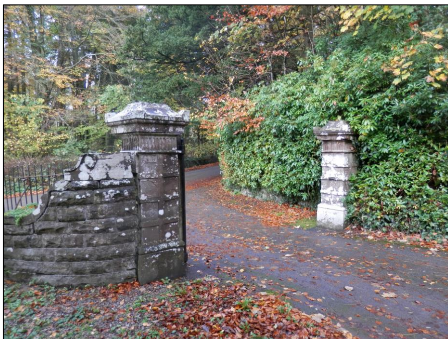
Plate 33: View looking NE towards the gatepiers
