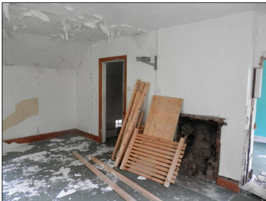
Plate 28: View looking SW across the larger bedroom
