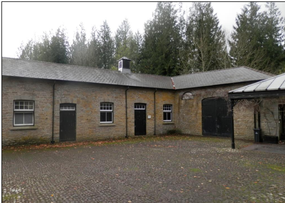
Plate 8: View looking SW at the Stable Block at Ffrwdgrech
