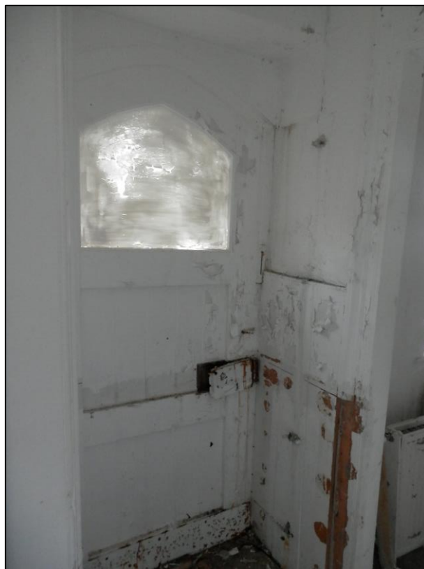
Plate 20: View looking N across the entrance hall
