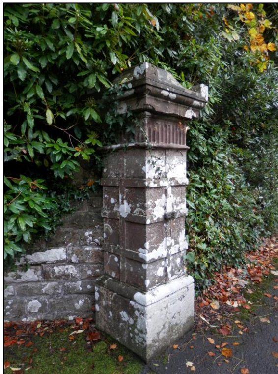
Plate 31: View looking SE at the E gatepier
