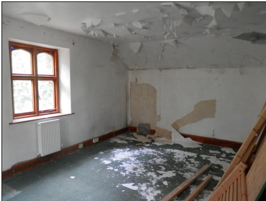
Plate 27: View looking SE across the larger bedroom
