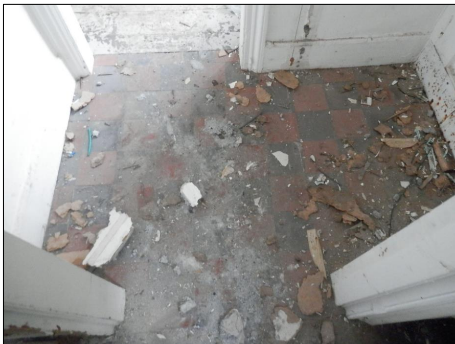
Plate 21: View looking at the tiled floor of the entrance hall
