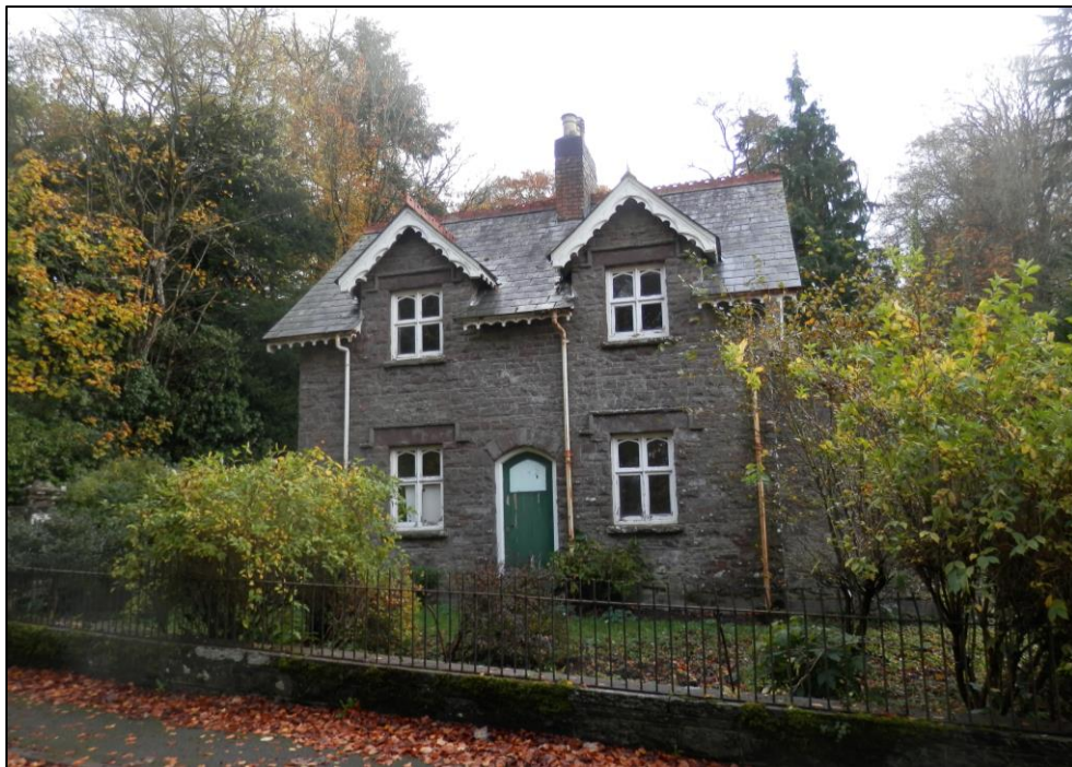
Plate 1: View looking SE towards the front of Brecon Lodge
