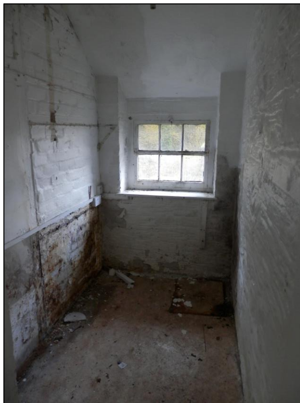
Plate 24: View looking SW across the interior of the kitchen
