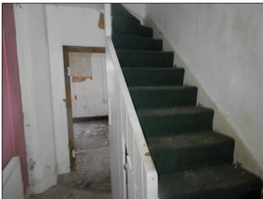
Plate 25: View looking NE towards the stairs to the first floor
