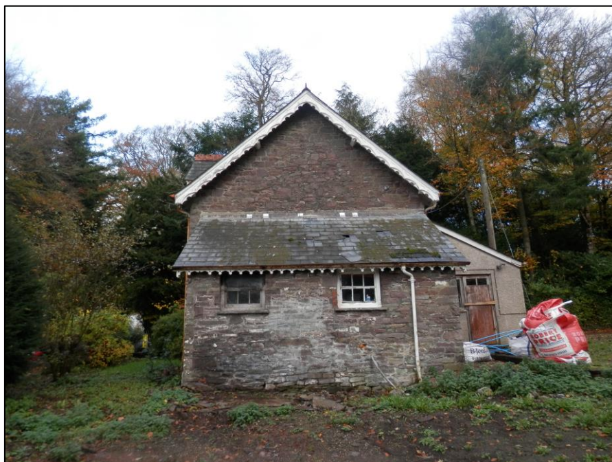
Plate 14: View looking E towards the W gable end of Brecon Lodge
