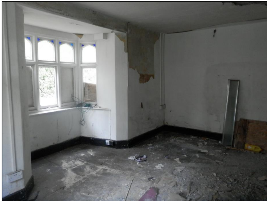
Plate 18: View looking SE across the interior of the living room
