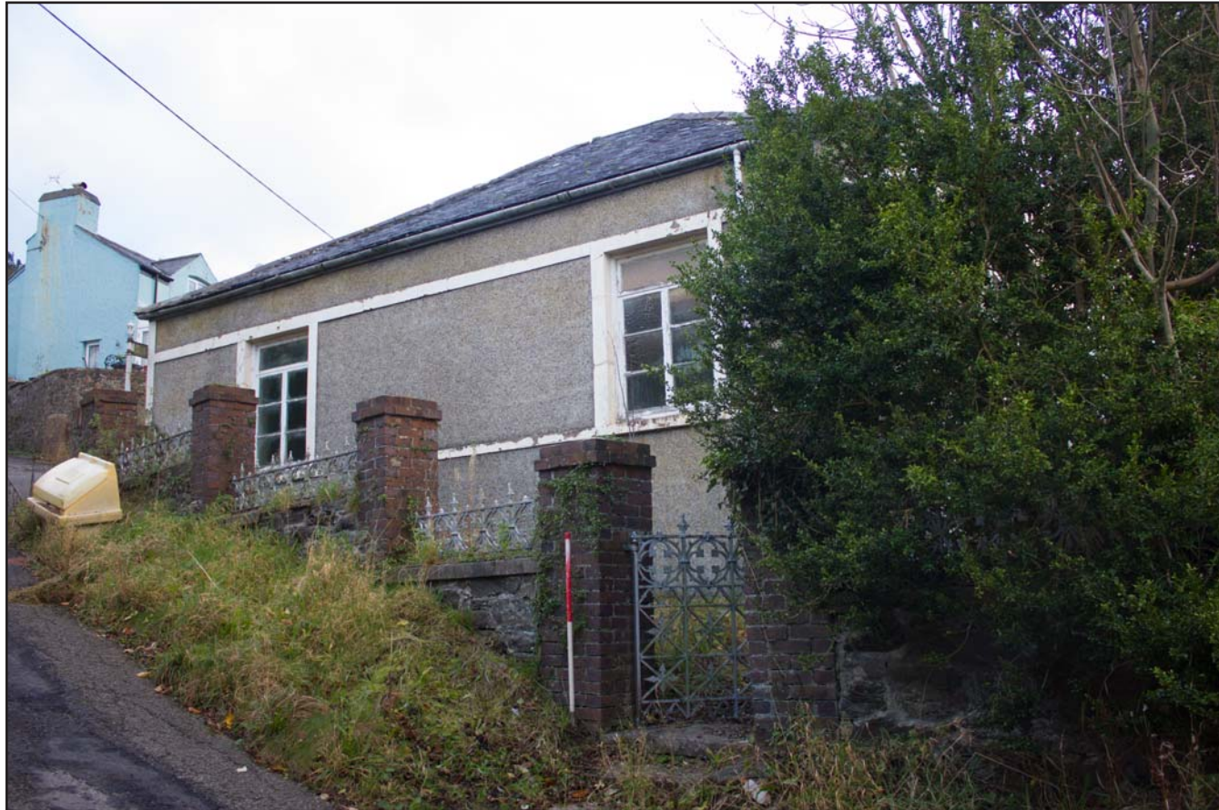
Plate 11: External oblique shot of north eastern elevation, Tŷ Capel, Denbigh Road, Llanfairtalhaiarn, Conwy - from the north - 1.00m scale
