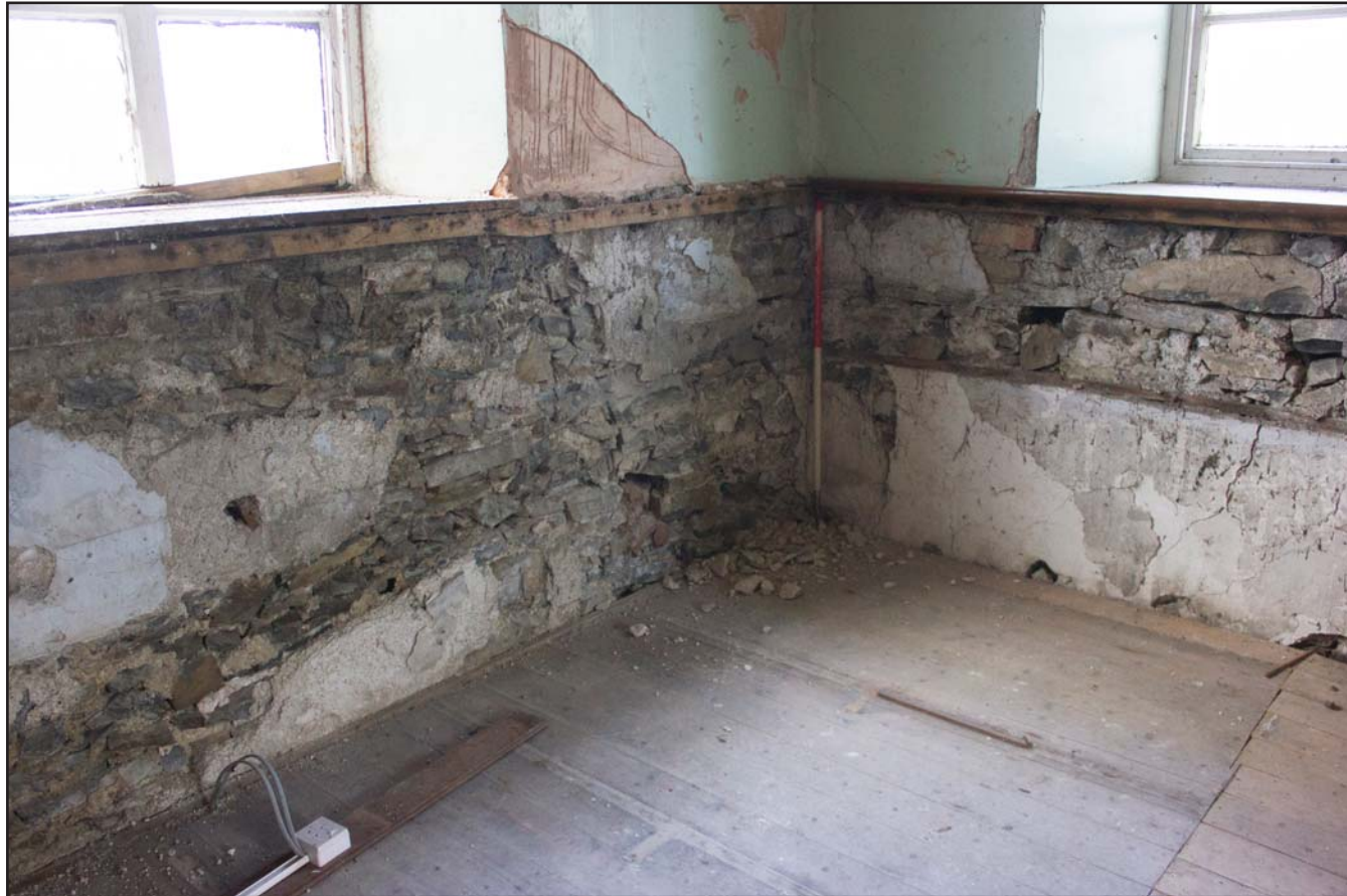
Plate 29: Internal shot, plaster line on south western elevation showing where tiered seating was previously located, Tŷ Capel, Denbigh Road, Llanfairtalhaiarn, Conwy - from the east - 1.00m scale
