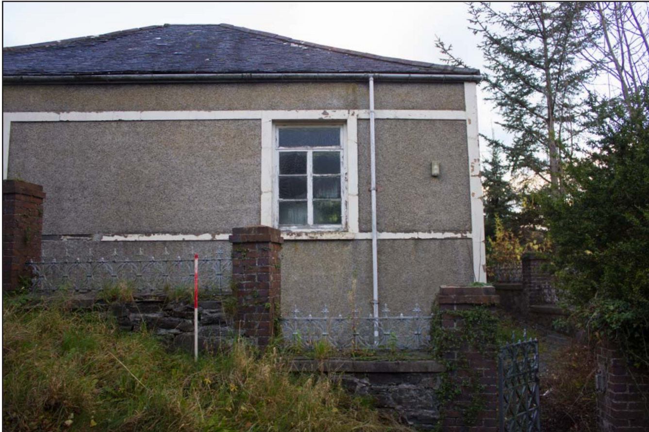
Plate 12: External shot of north eastern elevation (right), Tŷ Capel, Denbigh Road, Llanfairtalhaiarn, Conwy - from the northeast - 1.00m scale
