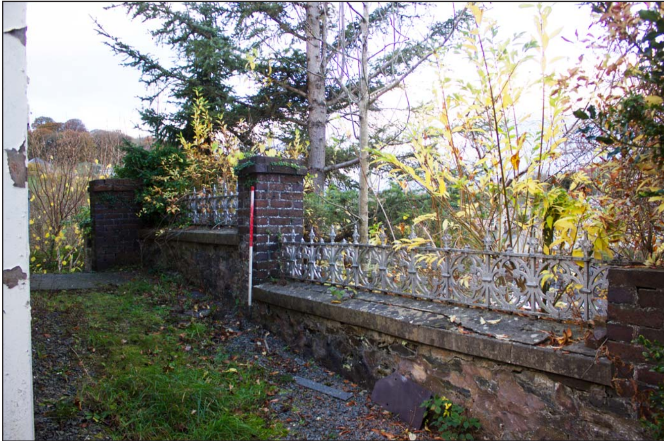
Plate 09: Cast iron railings to northwest of the Primary elevation, Tŷ Capel, Denbigh Road, Llanfairtalhaiarn, Conwy - from the east - 1.00m scale
