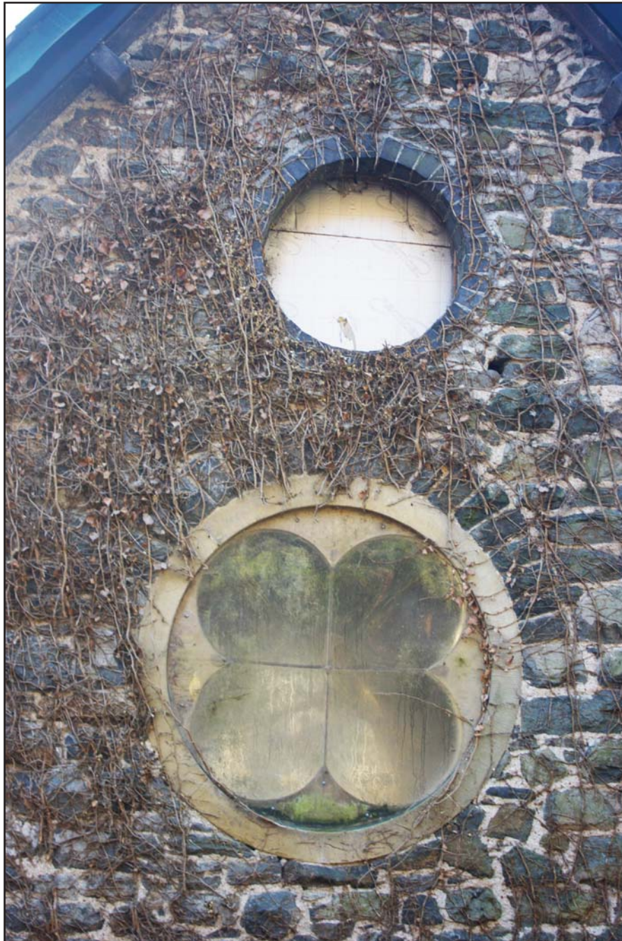
Plate 22: Rose/occulus (lower quatrefoil) windows on northeast facing elevation of Bethesda Chapel, Back Chapel Street, Llanrhaeadr ym Mochnant - from the northeast - no scale
