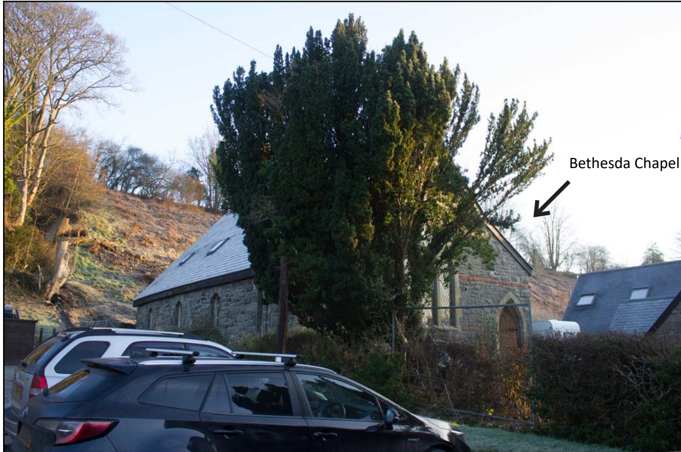
Plate 05: Oblique shot of southwest and northwest facing elevations of Bethesda Chapel, Back Chapel Street, Llanrhaeadr ym Mochnant - from the southwest - no scale
