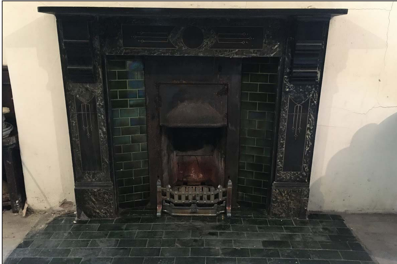
Plate H: Former fireplace within the Vestry - from the northwest.
