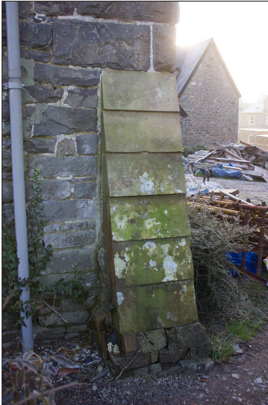
Plate 20: Decorative buttress on southwest corner of Bethesda Chapel, Back Chapel Street, Llanrhaeadr ym Mochnant - from the northwest - no scale
