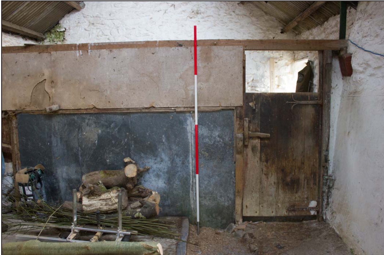
Plate 27: Slate divider in Room 1 within outbuilding at Penrhyn Garn, Rhydlydan, Pentrefeolas, Conwy - from the south - 2.00m scale
