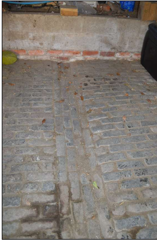
Fig. 12 Flooring in the northern end of the west range Photo CPAT 5031_020
