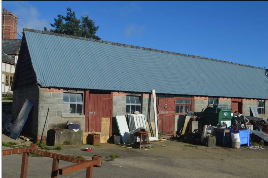
Fig. 7 View from the south of the north range Photo CPAT 5031_036
