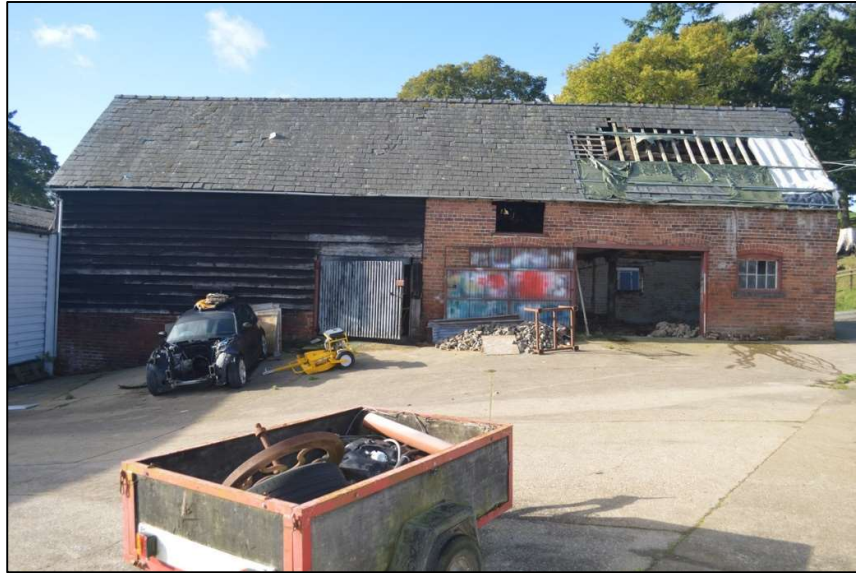
Fig.11 The west range viewed from the east Photo CPAT 5031_074
