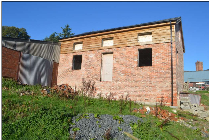
Fig. 6 The new building viewed from the south-east in November 2022 Photo CPAT 5031_005
