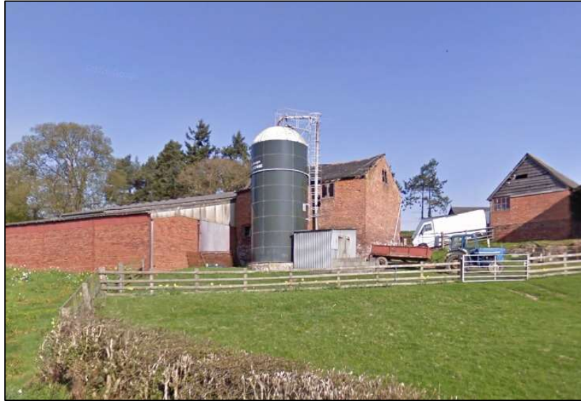
Fig. 5 The south range viewed from the south-east in April 2010 (Reproduced courtesy of Google Maps)
