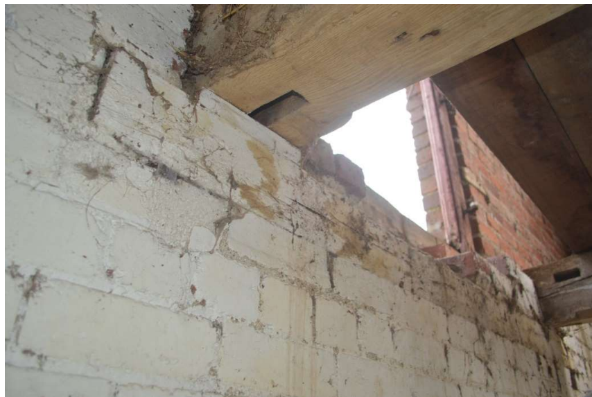
Fig. 16 Slots in the horizontal beams in the northern end of the western range possibly for wall timbers Photo CPAT 5031_101
