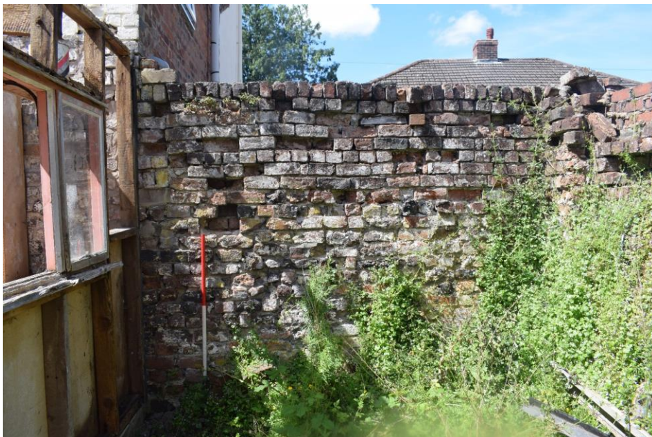
Fig. 8 East-facing yard wall. CPAT Photograph 4998_19
