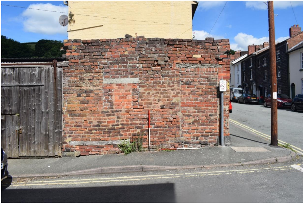
Fig. 4 Eastern elevation of Union Street frontage CPAT Photograph 4998_01
