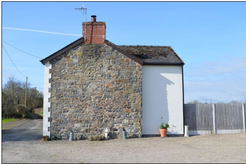
Fig. 7: The north-east end of Hafod, showing the stone end wall, the later brick extension seen on the 1902 map is to the right. CPAT 4983-0001
