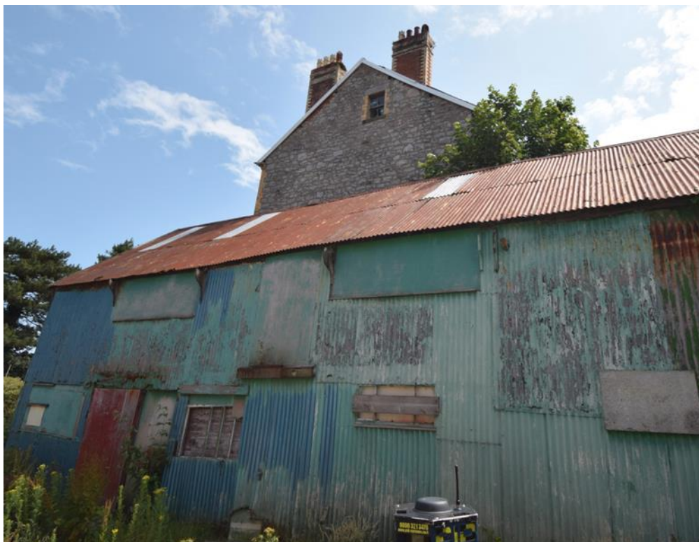
Fig 8 Workshop adjacent to 7 Bay View Road, looking south and east 5077_086 & 087
