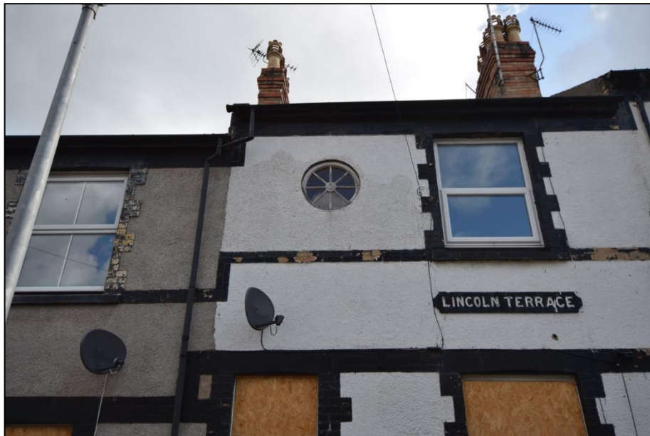
Fig. 4 Ox eye window and sign on the frontage of No. 2 Photo CPAT 5077_004
