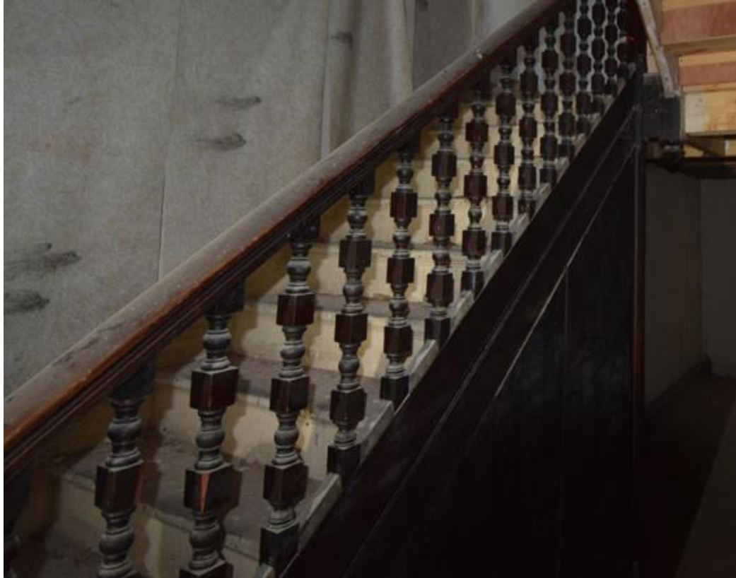
Fig. 13 Main staircase to first floor level CPAT 5077_120
