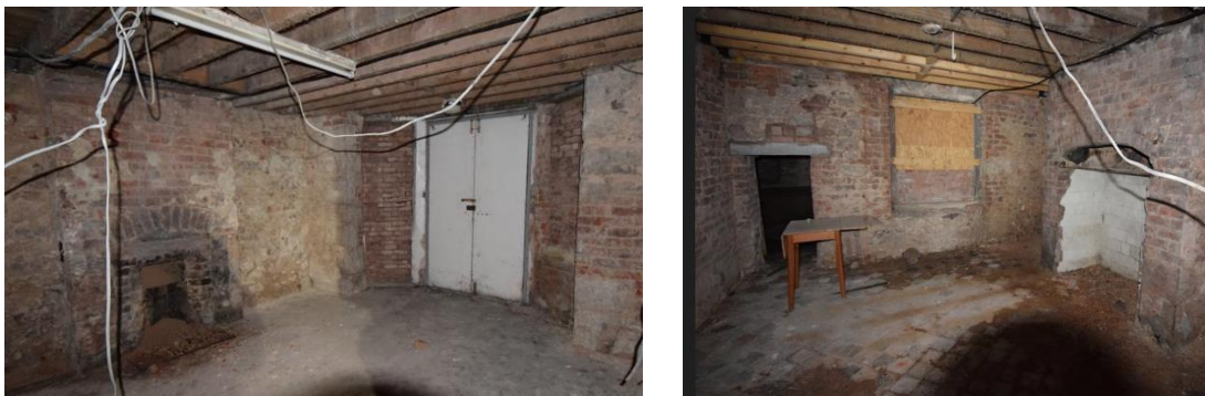
Fig 10 Basement showing replacement door, fireplaces and tiled floor CPAT 5077_121 & 122
