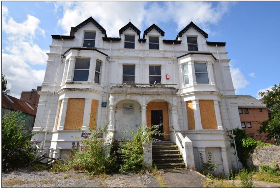
Fig. 6 North facing (principal) elevation of No 3-4 Photo CPAT 5077_031
