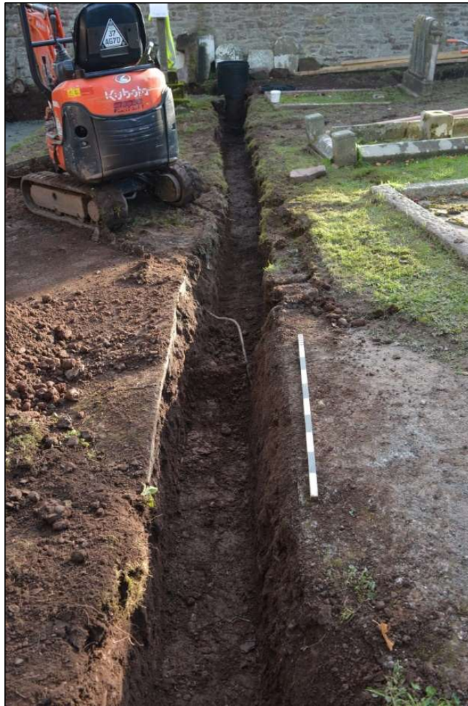
Fig. 7: The trench running south from the tower, from the north. CPAT 4725-0036
