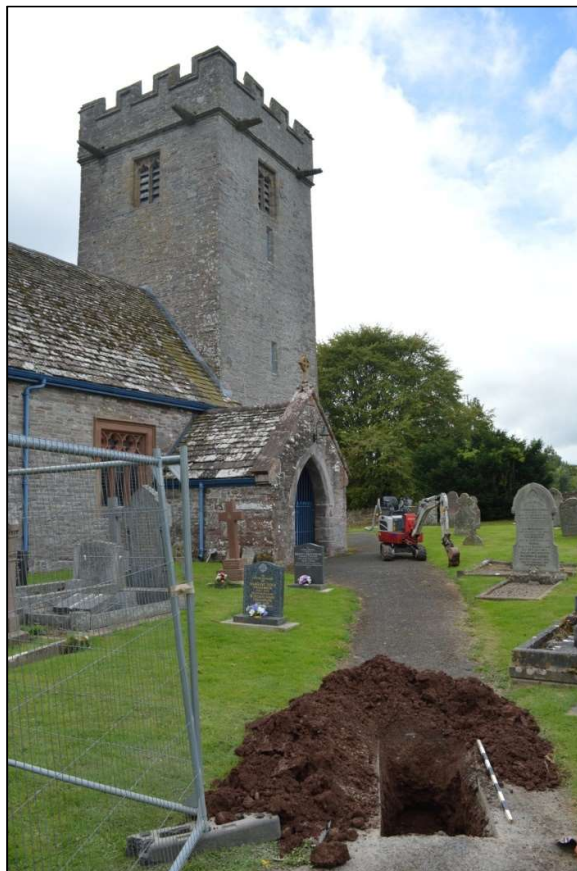
Fig. 2: One of the trenches in the churchyard path. CPAT 4725-0010
