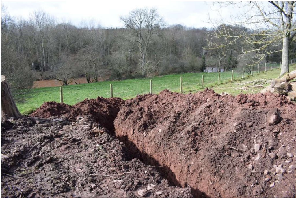
Fig. 9: The trench excavation for the soakaway, from the north-east. CPAT 4725-0053
