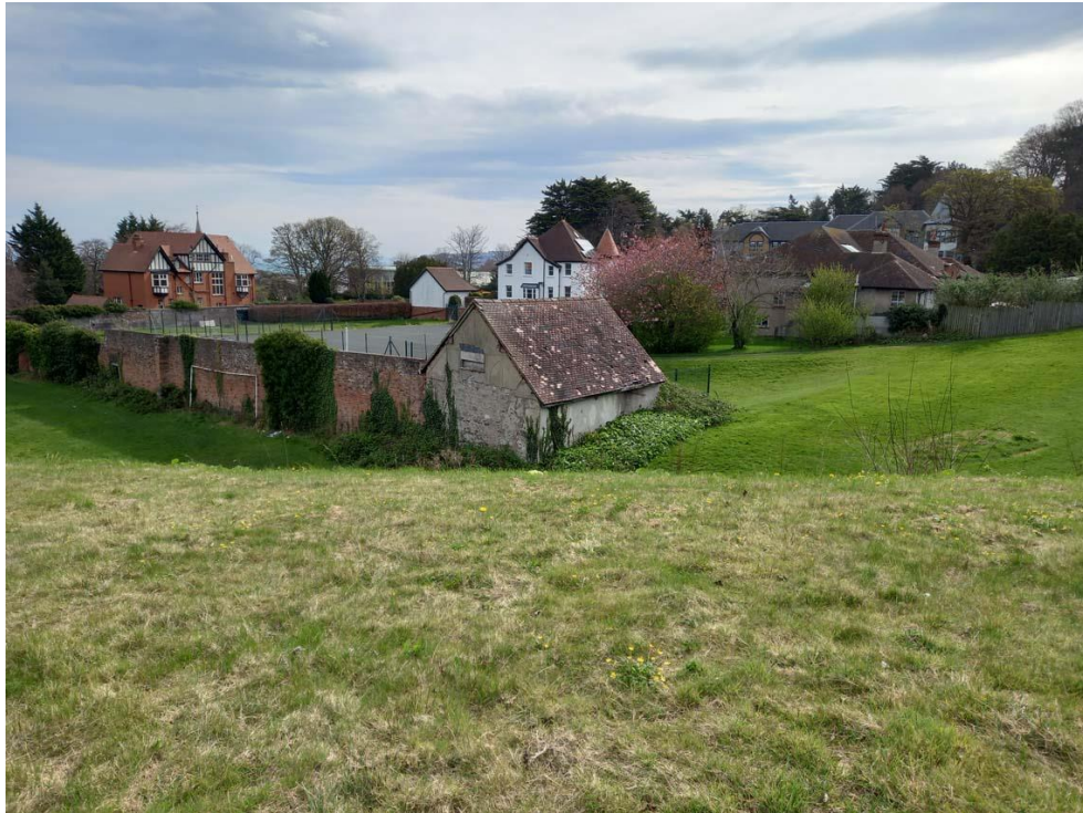
Fig. 10 Pumphouse adjoining walled garden. CPAT Photo 4985-012
