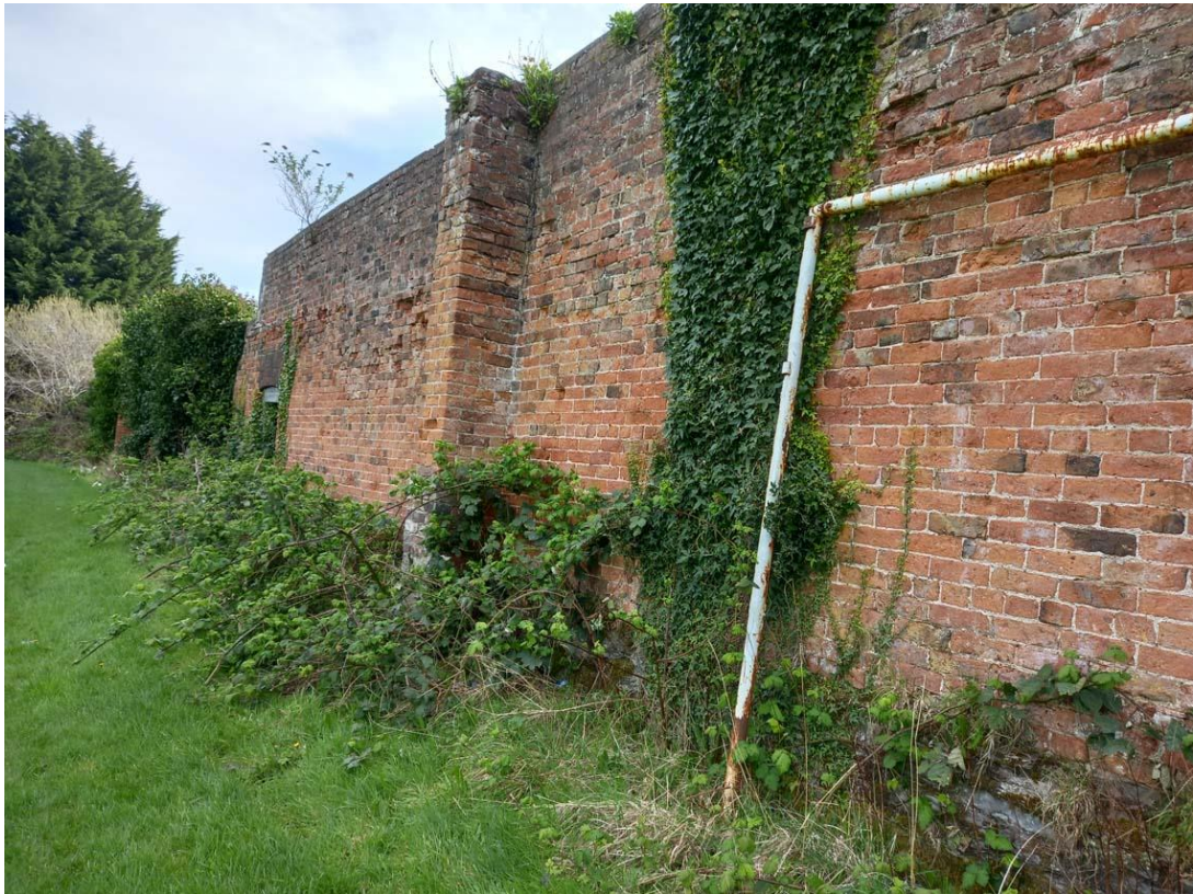
Fig. 9 Northwest facing elevation of walled garden. CPAT Photo 4985-005
