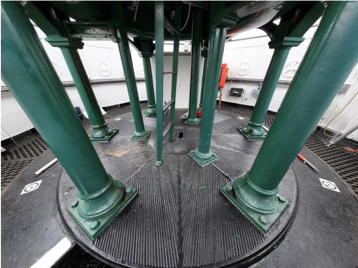
Figure 4.5: View of inner and outer-pillars of the lens pedestal (© Crown Copyright: RCAHMW).
