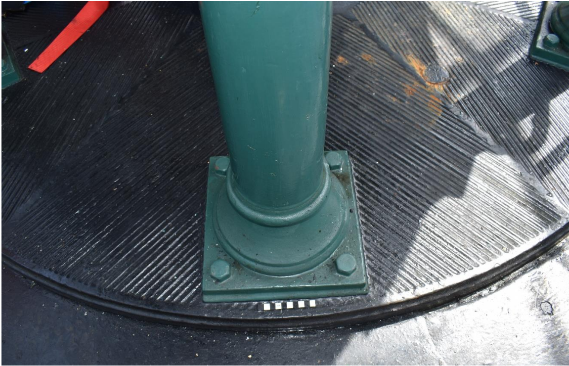
Figure 4.3: Detail of pedestal outer-pillar base and lower moulding, scale is 10cm (© Crown Copyright: RCAHMW).
