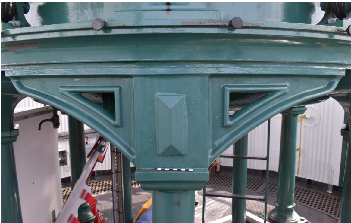
Figure 4.4: Detail of pedestal outer-pillar top, capital and brackets, scale is 10cm (© Crown Copyright: RCAHMW).
