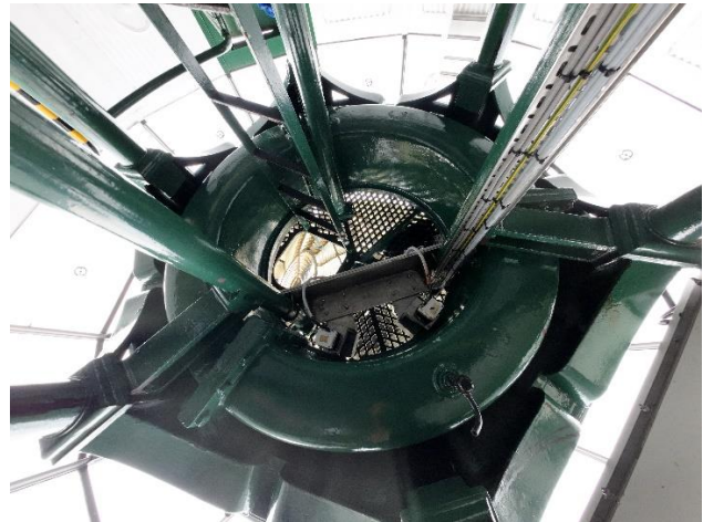
Figure 4.9: Left: Modern electrical circuit board on one side of the pedestal. Right: Wiring loom running up an inner-pillar within the pedestal (© Crown Copyright: RCAHMW).
