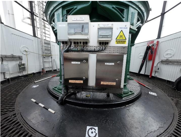
Figure 4.9: Left: Modern electrical circuit board on one side of the pedestal. Right: Wiring loom running up an inner-pillar within the pedestal (© Crown Copyright: RCAHMW).
