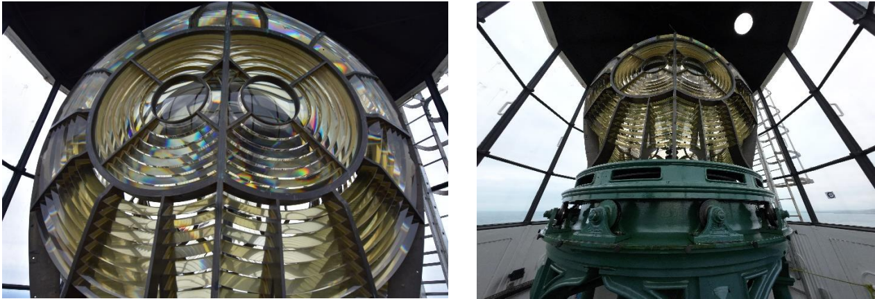
Figure 2.1: Two images of the same view of the Skerries Fresnel Lens. Left: Conventional wide-angle lens at maximum field of view. Right: 155° field of view afforded by a DJI Action2 camera (© Crown Copyright: RCAHMW).
