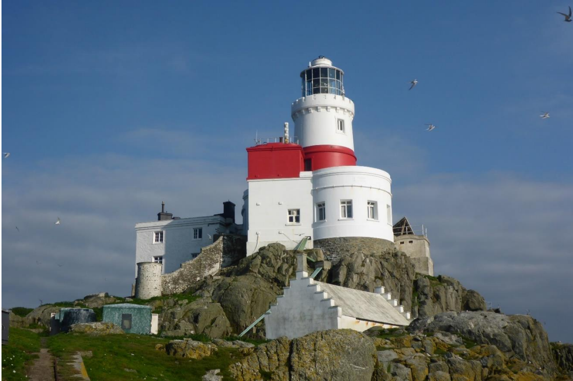
Figure 1.2: General view of the Skerries Lighthouse on the 16 th July 2024 (© Crown Copyright: RCAHMW).
