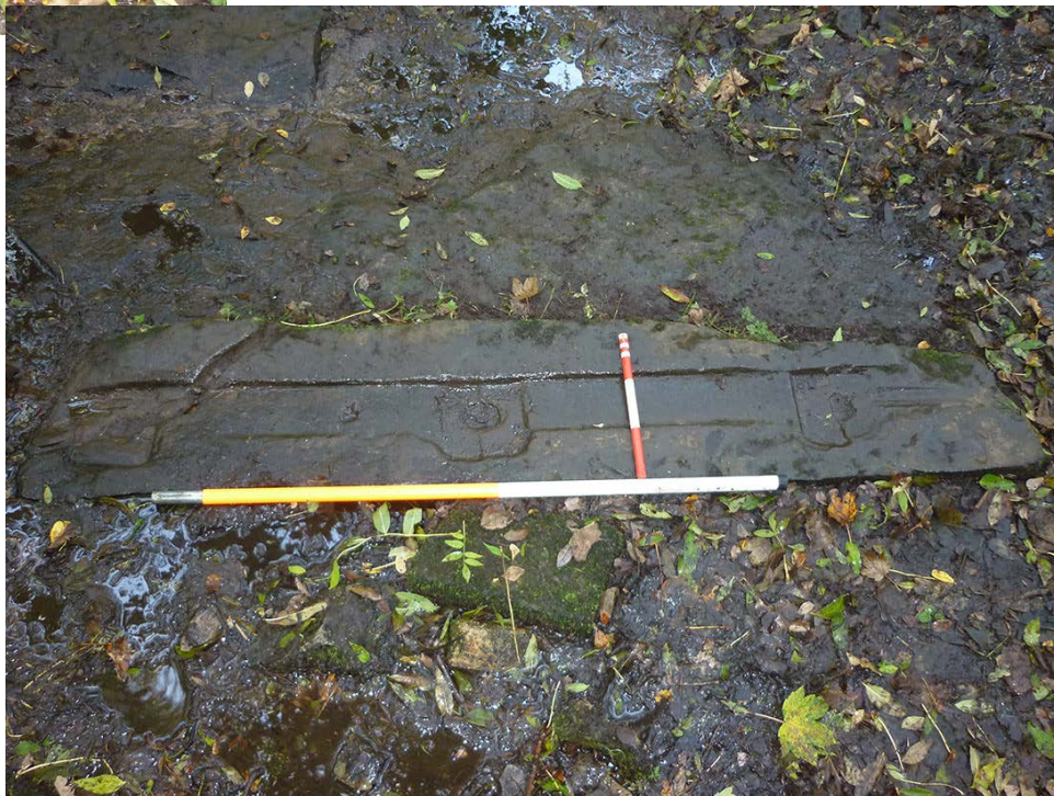
Fig. 5 Wear marks from Outram style plates on sleeper stones at Chain 80
