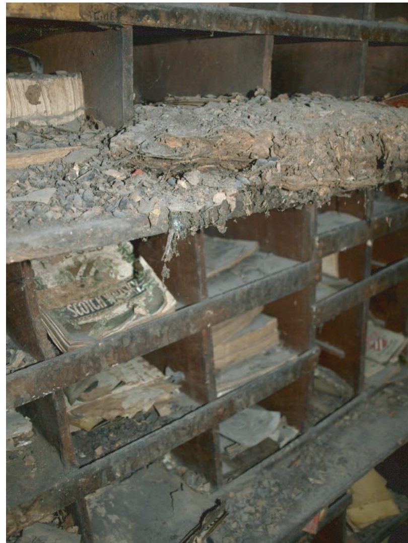
Plate 168. Llanelly House - Sir Thomas Stepney's Study (Room G2) - Detail shot showing remains of former 19th century wine and spirit bottle label cupboard hidden behind wooden panelling in west facing elevation beside fireplace.
