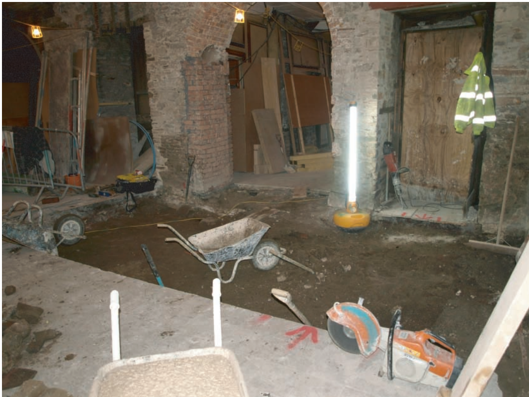
Plate 129. Llanelly House - The Great Hall (Room G1). Working shot during removal of modern concrete floor and ground reduction. Looking southeast.
