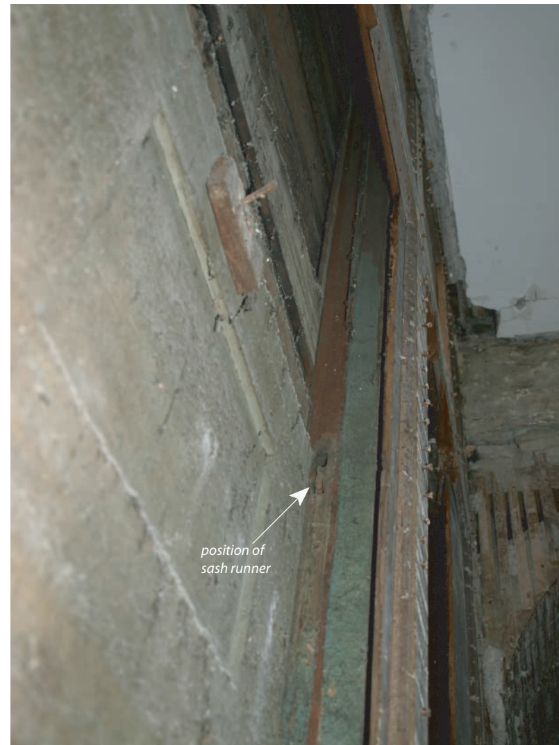
Plate 164. Llanelly House - Sir Thomas Stepney's Study (Room G2) - View of sash runners hidden within wooden partition that encloses the small storage space in Room G2. Likely associated with a former sliding door that screened the hidden storage space beneath the floor of Sir Thomas Stepney's study
