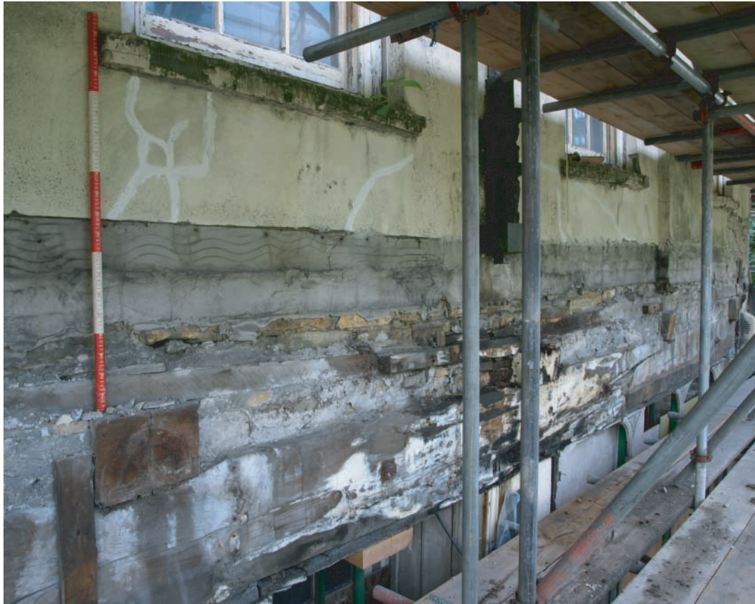
Plate 35. Llanelly House - Oblique view looking westward toward position of victorian shopfront at west end of front facade, 1st level of scaffolding. Note oak bessemer beam. Looking southwest.
