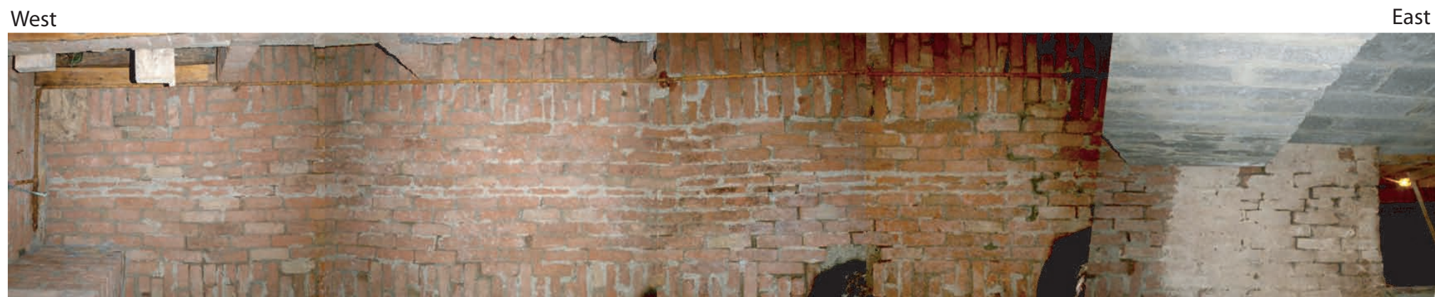
Plate 262. Spliced photo of central spine of vaulted ceiling interior in Victorian red brick cellar. Looking upwards from interior of cellar.
