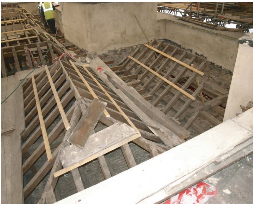
Plate 95. Llanelly House - Roof area in process of repair following removal of slates and irreparable timbers. Looking north from southeastern corner of roof.
