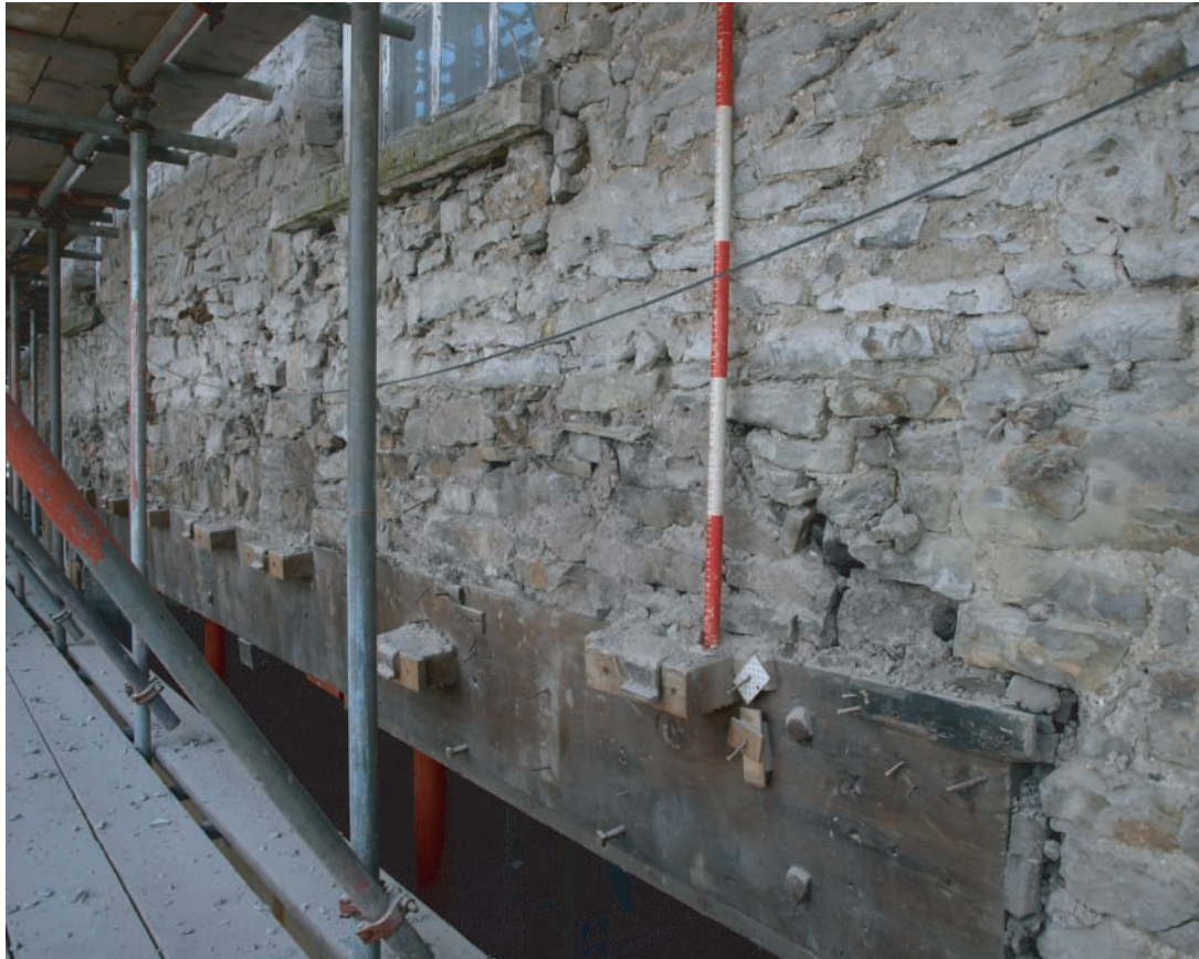
Plate 63. Llanelly House - View of oak bessemer beam exposed behind modern shopfront at far southern end of west facing elevation. Looking northwards.
