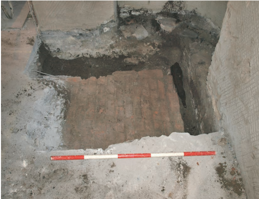
Plate 214. Removal of modern concrete floor in area of proposed lift shaft exposes the ceiling of victorian red brick cellar (Bay No.6). Looking south.
