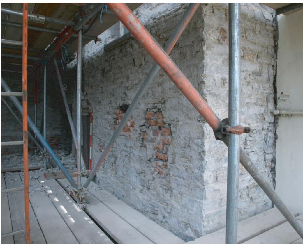
Plate 74. Llanelly House - View of south facing elevation in area above rear entrance, following removal of external render. Looking northwest.
