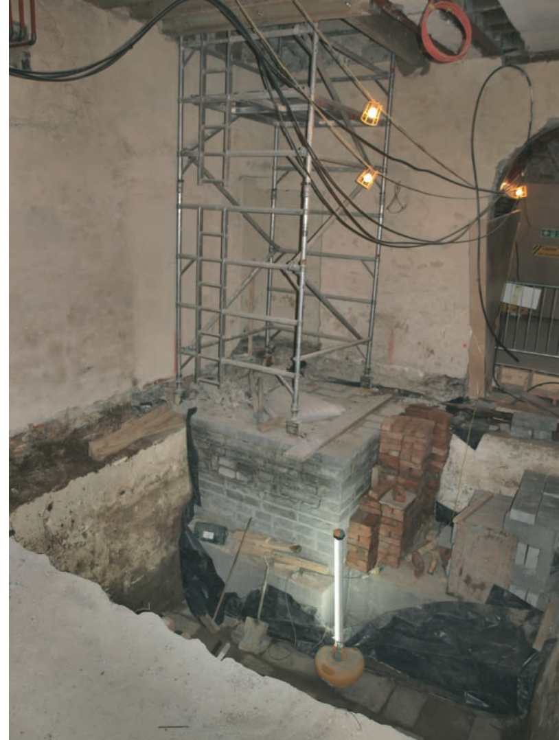
Plate 245. Working shot during Victorian red brick cellar dismantling. View of lift shaft area during construction of base. Looking west.
