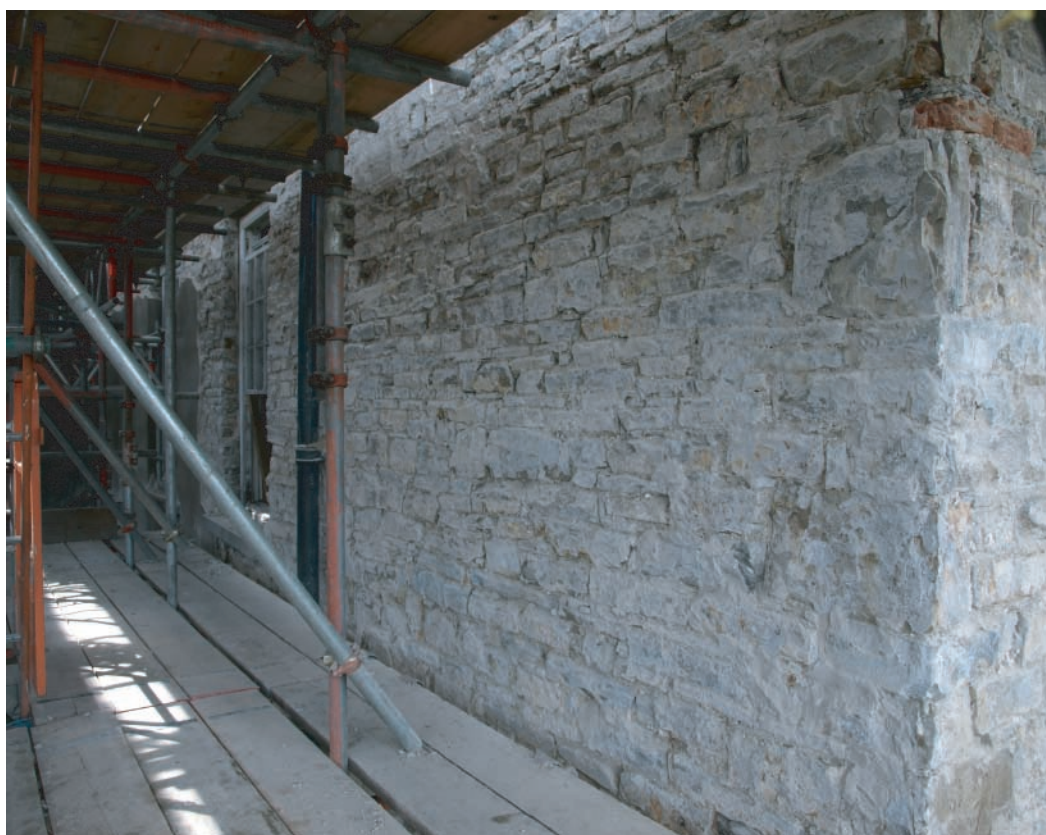
Plate 78. Llanelly House - Oblique view of south facing elevation at second floor level following removal of external render. Looking northwest.
