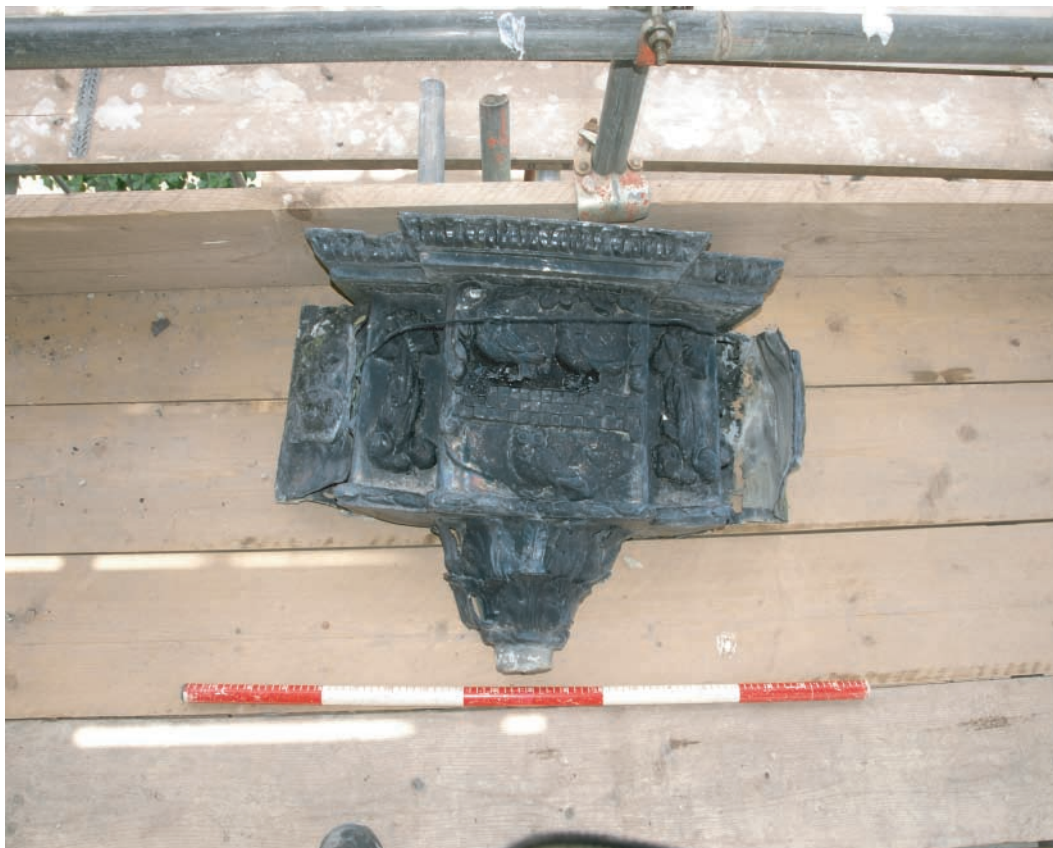
Plate 45. Llanelly House - View of lead drain hopper from west facing elevation. Note Stepney coat of arms - three owl design on a fess chequy (archaic) or 'chequered band'.
