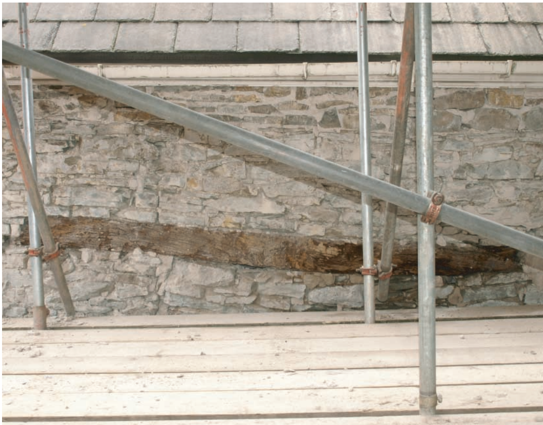
Plate 92. Llanelly House - View of east facing elevation at uppermost level above former courtyard alongside western range. Shows the remains of an oak timber lintel, likely a former 18th century window opening, also visible as being blocked in. Looking west.
