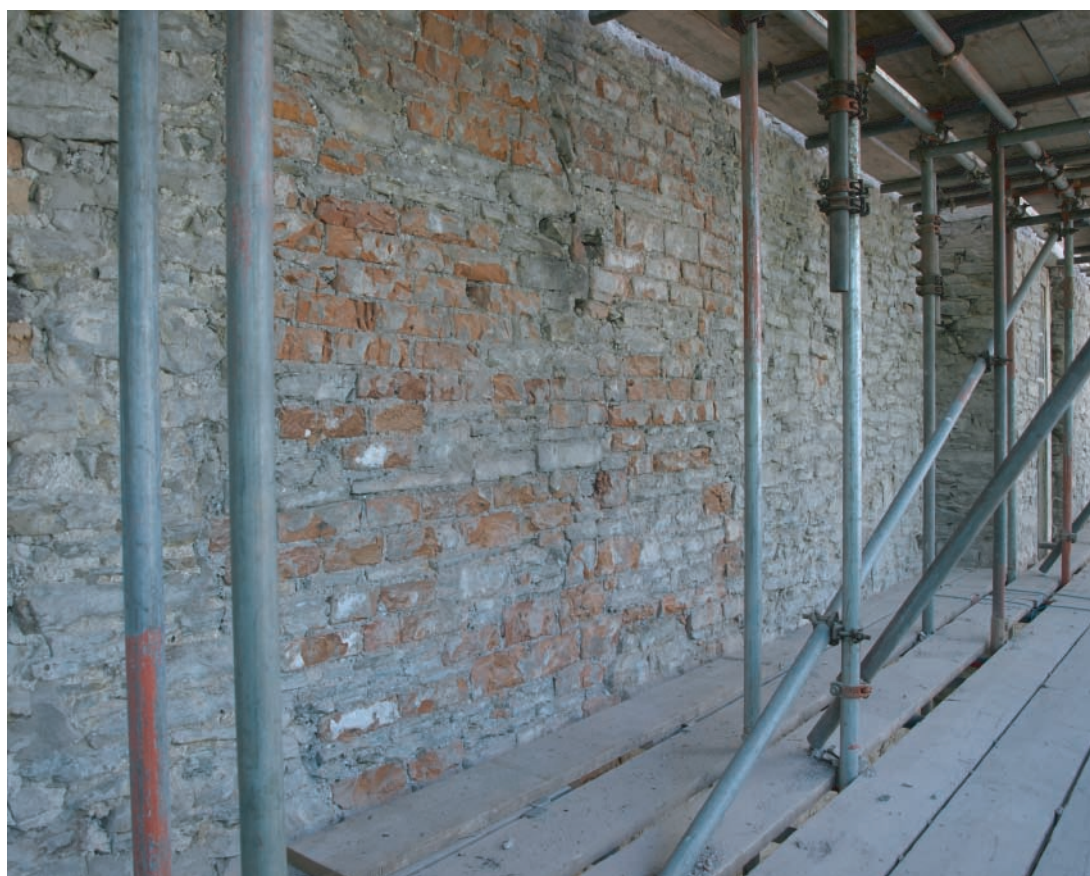
Plate 66. Llanelly House - View of first floor level above former Victorian shop front in west facing elevation following removal of external render. Looking southwards. Note red brick repair in position of former projected chimney.
