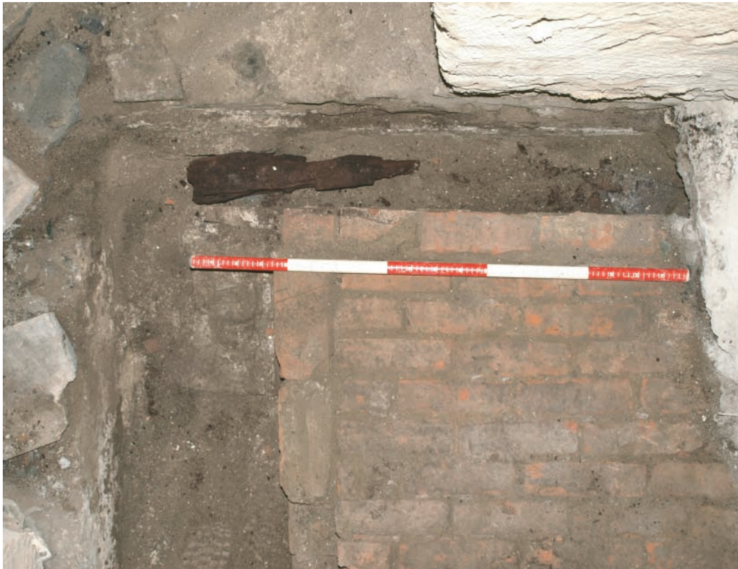
Plate 216. Detail shot showing remains of oak timber floor joist alongside victorian red brick cellar ceiling in area of proposed lift shaft (Bay No. 6)
