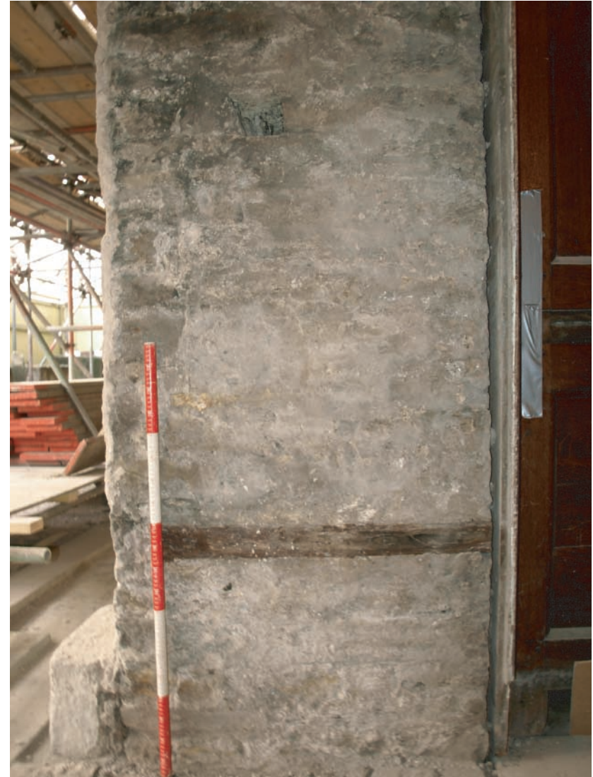
Plate 156. Llanelly House - The Great Hall (Room G1) - West facing former 18th century central doorway elevation revealed following removal of victorian rebuild.
