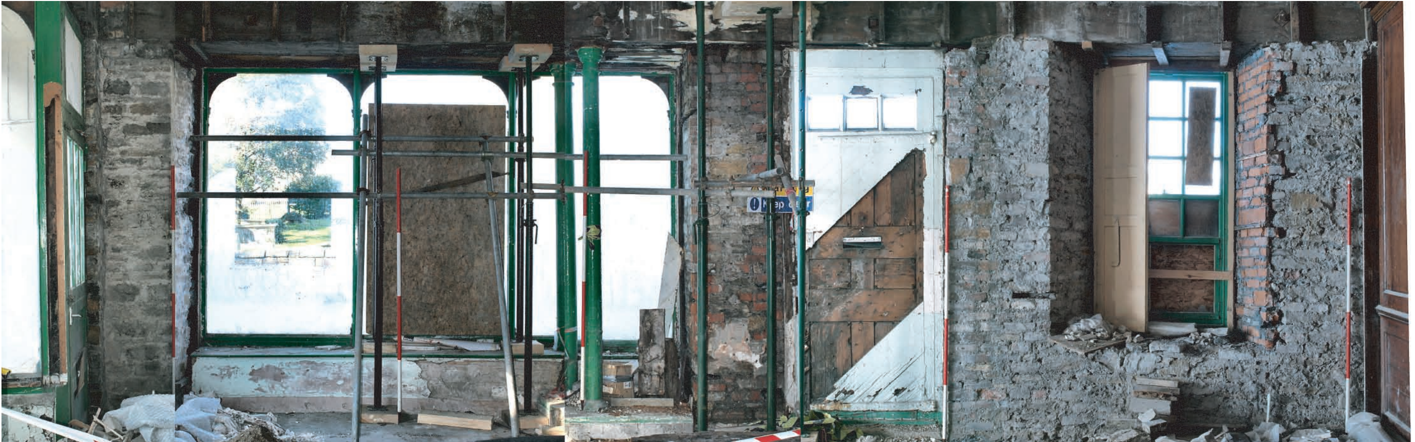
Plate 105. Composite photograph of south facing elevation of supposed former 'Great Hall' (Room G1), following removal of wall plaster from former contract work in 2003/03. Note victorian shopfront and original 18th century front door having been reused and reinserted in a new position from its original central position at the right of the photo, in the position of the new window opening. All of the visible standing fabric is 19th century in date in this elevation.
