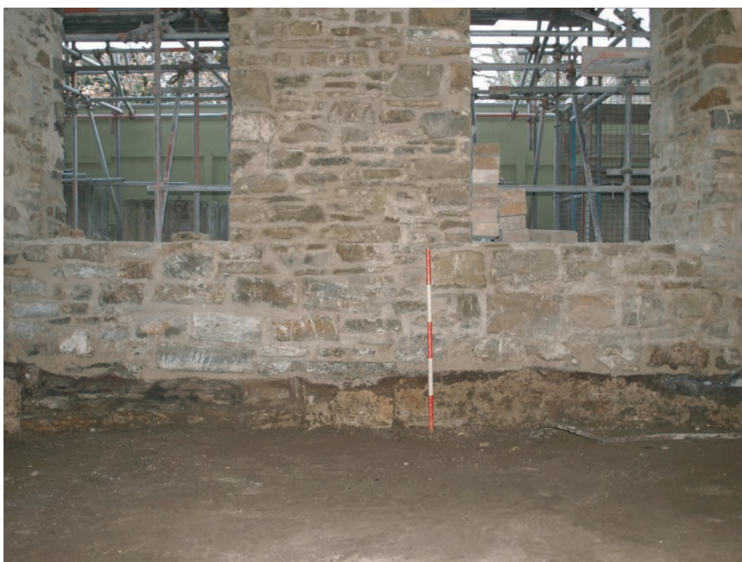
Plate 150. Llanelly House - The Great Hall (Room G1). South facing elevation following complete removal of modern concrete floor and 18th - 19th century overburden. Note remains of former 17th century wall plaster and position of former blocked in 17th century window opening at left of photo.
