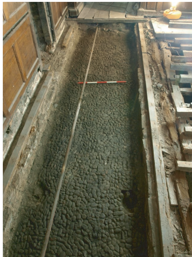
Plate 117. Llanelly House - The Great Hall (Room G1) - View of exposed 16th - 17th century cobbled floor, following removal of overburden (demolition material). Note framed pictorial cobble work at far end. Looking south.
