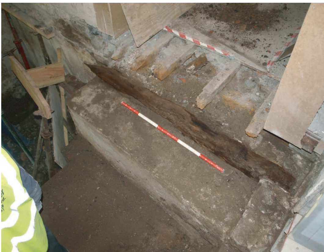
Plate 231. View of 'projecting wall' with overburden and victorian red brick vaulting removed.
