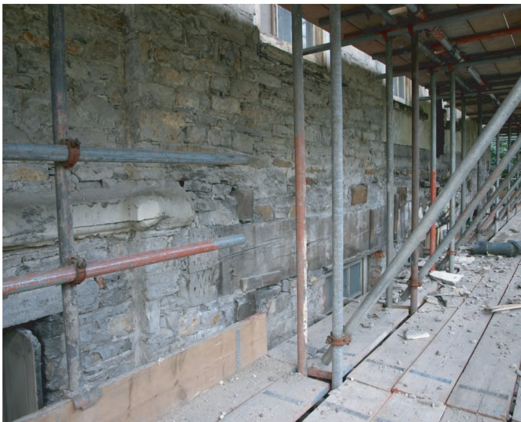
Plate 34. Llanelly House - Oblique view looking westward toward position of victorian shopfront at west end, 1st level of scaffolding. Note oak bessemer beam. Looking southwest.
