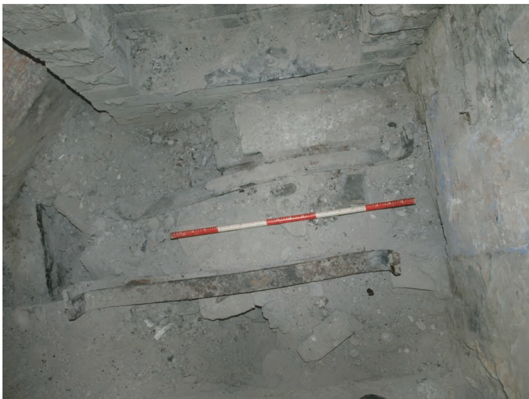
Plate 267. Overhead view of remains of pair of wrought iron support bars found at base of stone block in at far north east corner of Room G3. Iron bars lie directly above mortared yellow firebricks, suggesting a possible arched opening directly beneath, possibly a 'warming oven' on the west credit union side?
