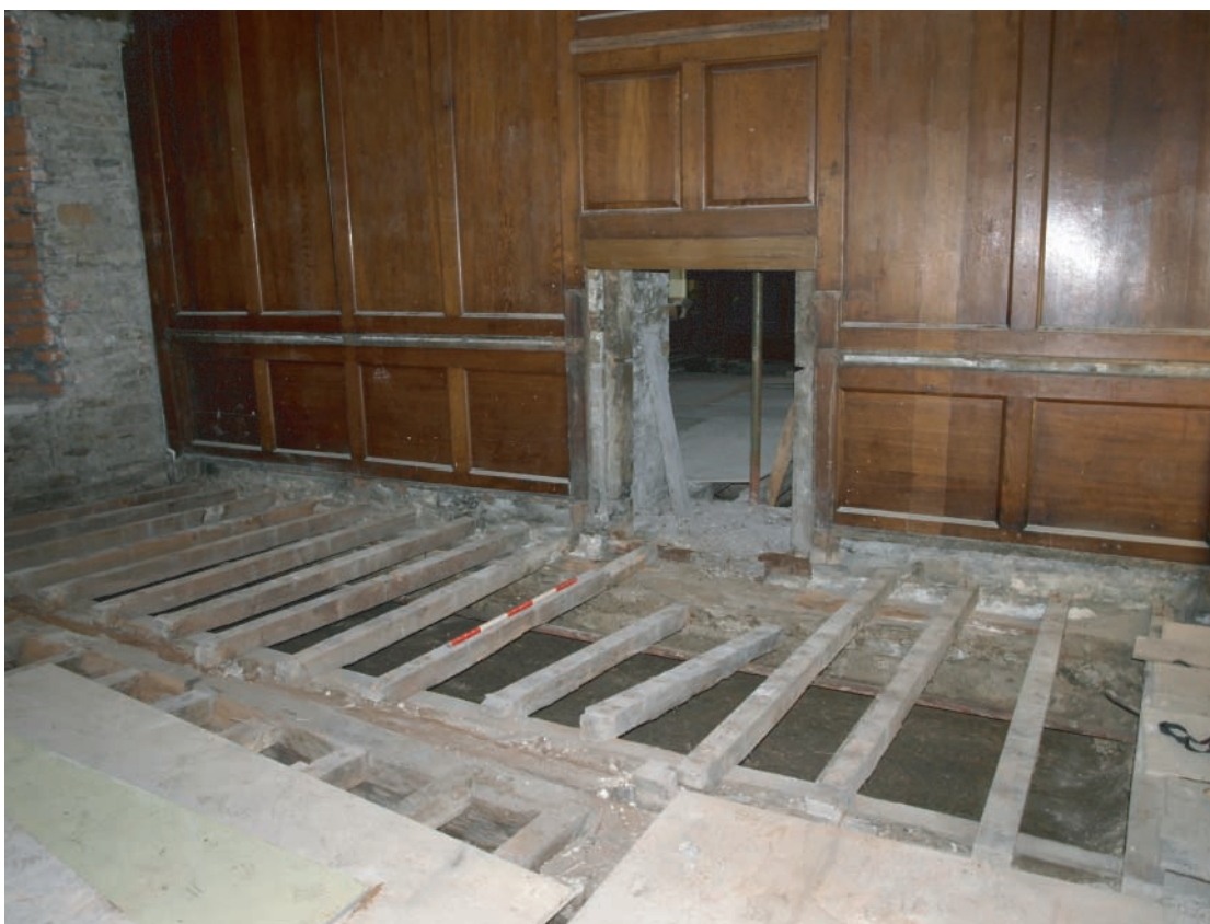
Plate 122. Llanelly House - The Great Hall (Room G1). Oblique view of area of exposed cobble floor with original floor joists put back in place. Looking eastwards. Also note 19th century fireplace and block in removed from former 18th century doorway.
