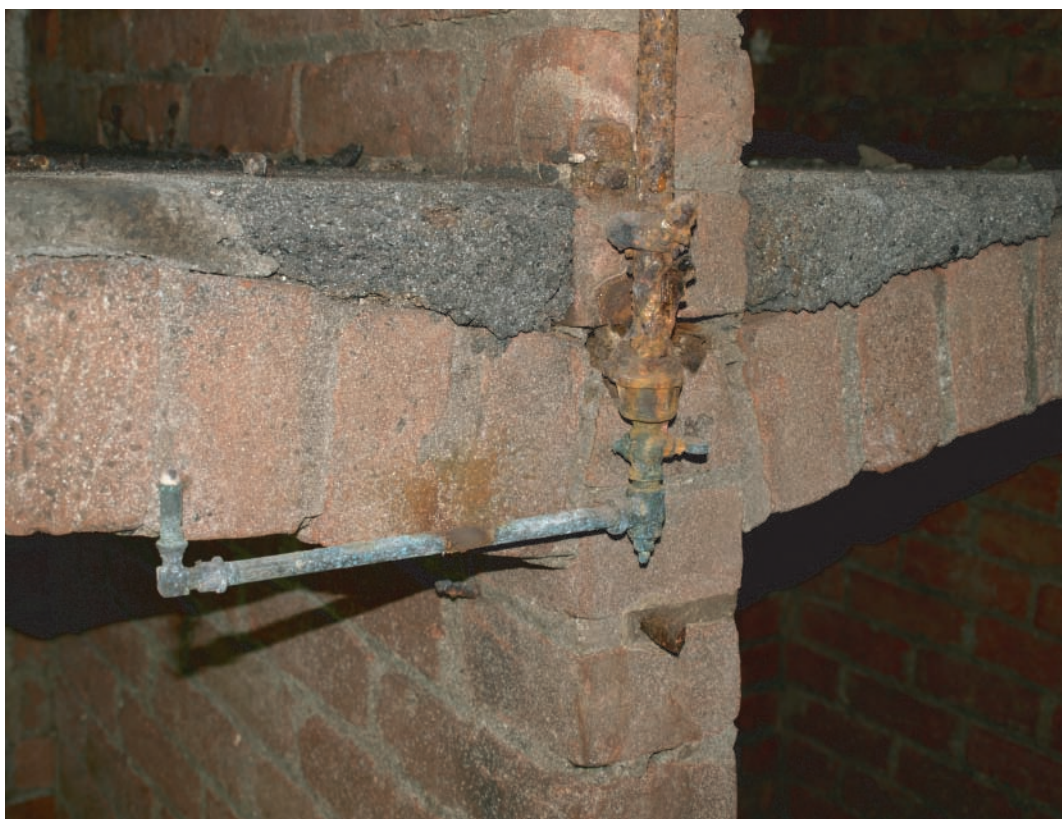
Plate 208. Detail of victorian gas-light fitting. Looking southwest alongside Bay No. 8.
