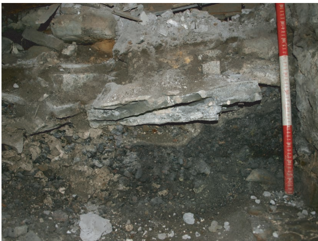
Plate 184. Llanelly House - Sir Thomas Stepney's Study (Room G2). Depth and character of overburden deposits blocking former access opening into low basement room in Room G2. Looking west from low basement at position of access opening.
