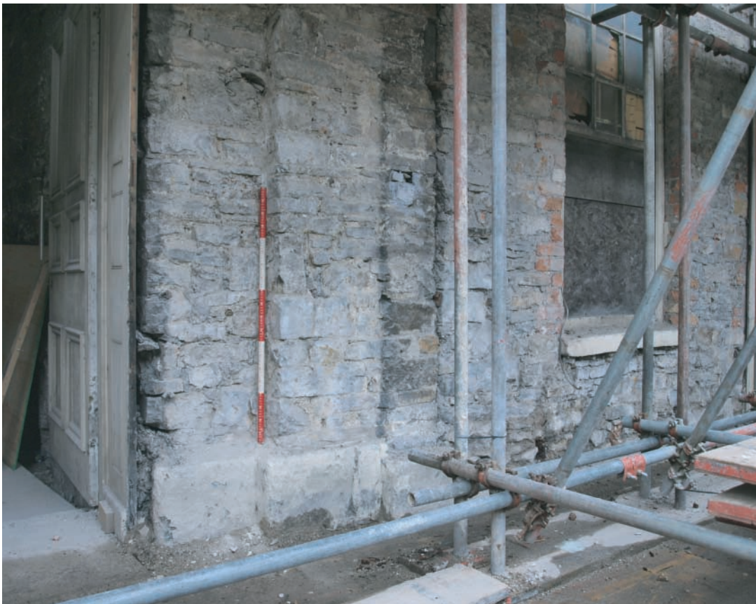
Plate 30. Llanelly House - Ground floor eastern end of north facing elevation, in area of former Margrave Brothers Spirit & Wine Merchants. Following removal of external render. Looking southwest toward position of former 18th century entrance.
