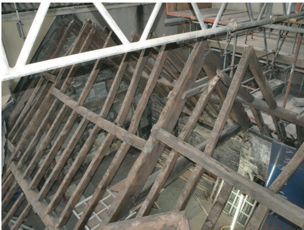
Plate 98. Llanelly House - Roof of eastern range following removal of slates, floor and floor joists. Looking southwest.
