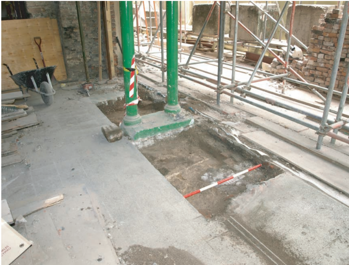
Plate 123. Llanelly House - The Great Hall (Room G1). Shot showing small evaluation trench at base of former victorian shopfront in west wall. Trench inserted in order to ascertain existence, character and extent of former 18th century fireplace. Looking southwest.
