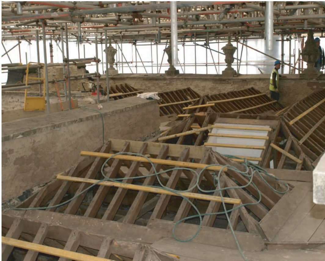
Plate 94. Llanelly House - Roof area in process of repair following removal of slates and irreparable timbers. Looking northwest from southeastern corner of roof.
