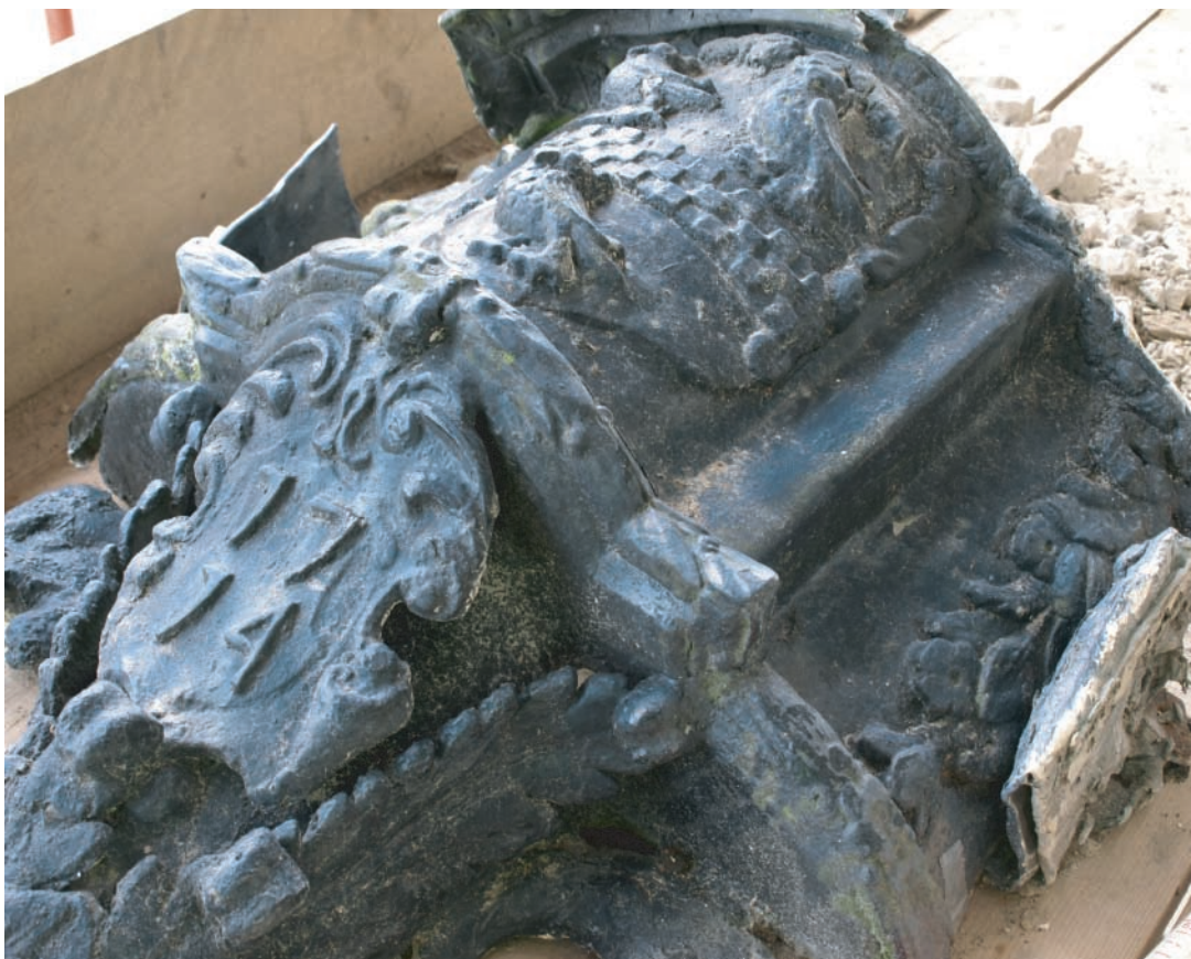
Plate 52. Llanelly House - Oblique view of central lead rain hopper.
