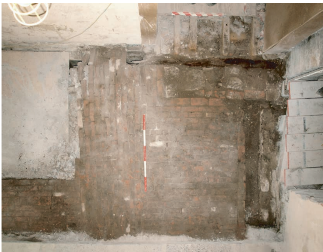
Plate 228. Overhead view of western end of exposed victorian red brick cellar vaulted ceiling, following removal of section of modern concrete floor.
