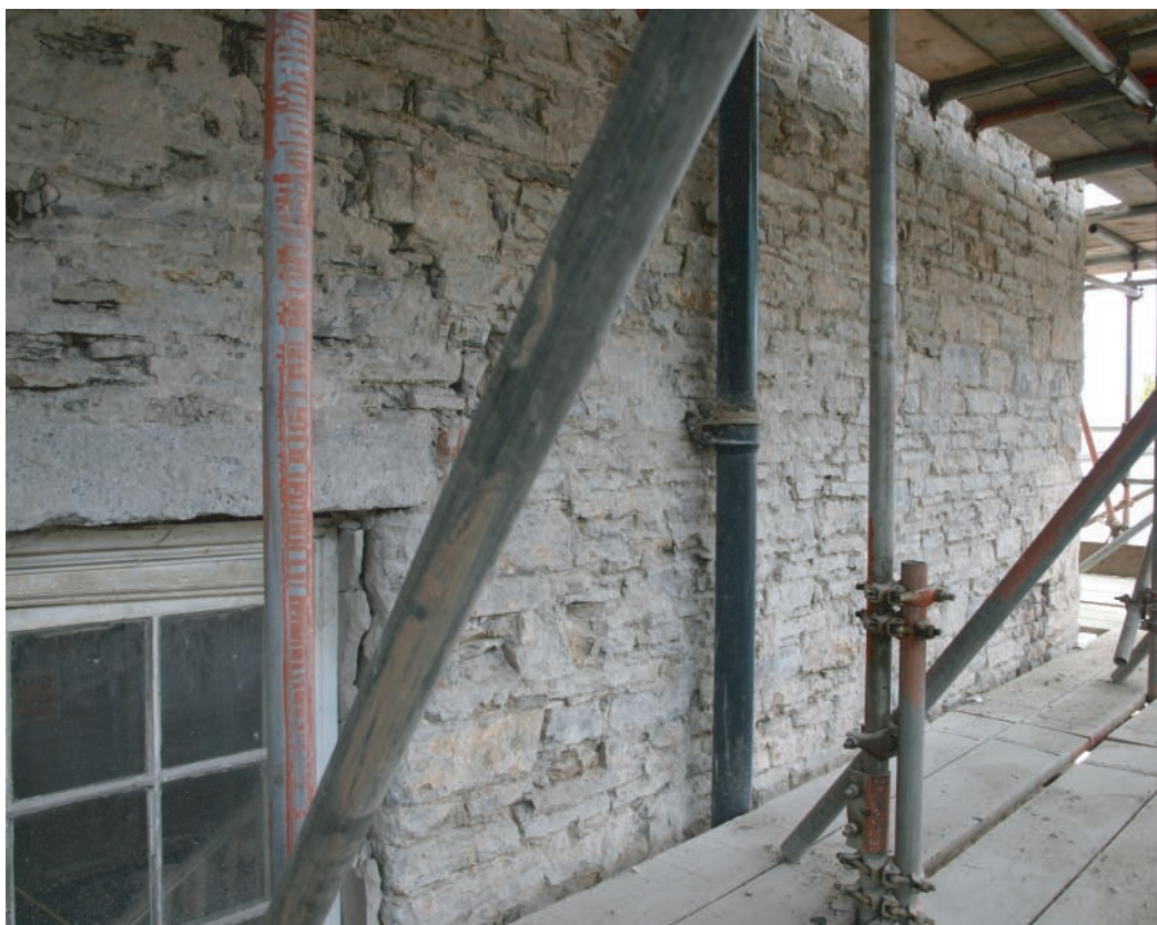
Plate 77. Llanelly House - Oblique view of south facing elevation at second floor level following removal of external render. Looking northeast.
