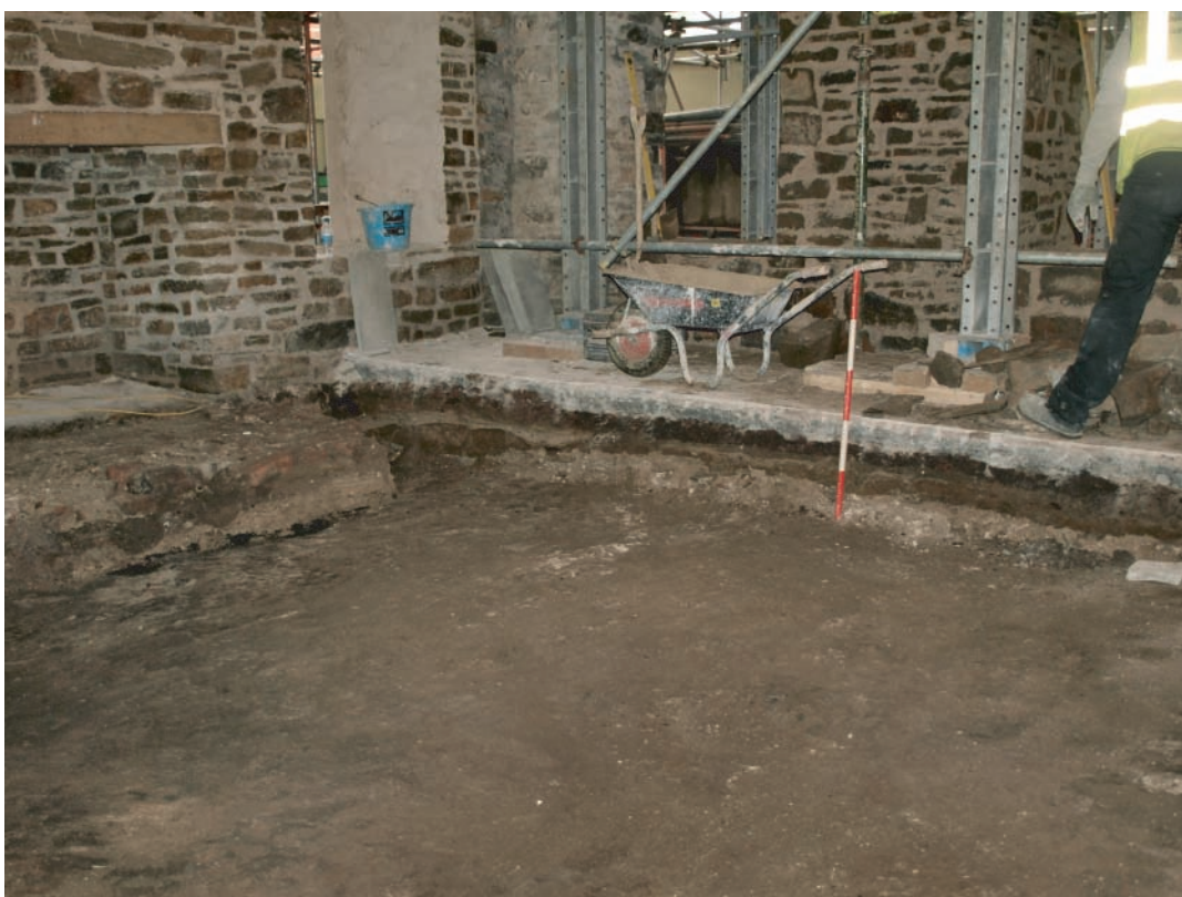
Plate 136. Llanelly House - The Great Hall (Room G1). Shot showing depth of overburden. Overburden cleared down to former compacted earth 17th century floor level. Looking northwest.
