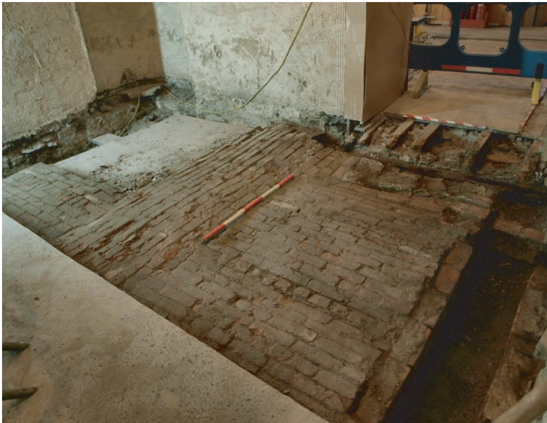
Plate 226. Further removal of modern concrete floor revealing victorian red brick cellar vaulted ceiling. Looking southwest.
