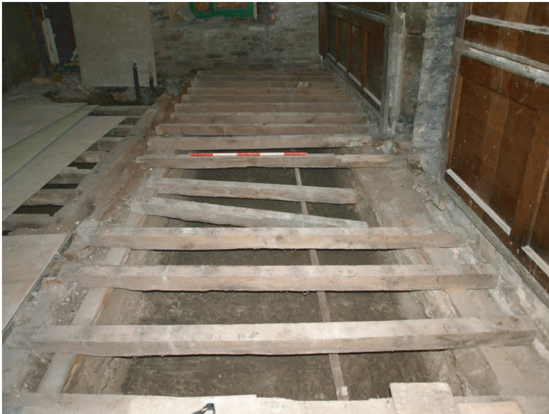
Plate 121. Llanelly House - The Great Hall (Room G1). View of area of exposed cobbled floor with original floor joists put back in place. Looking north.
