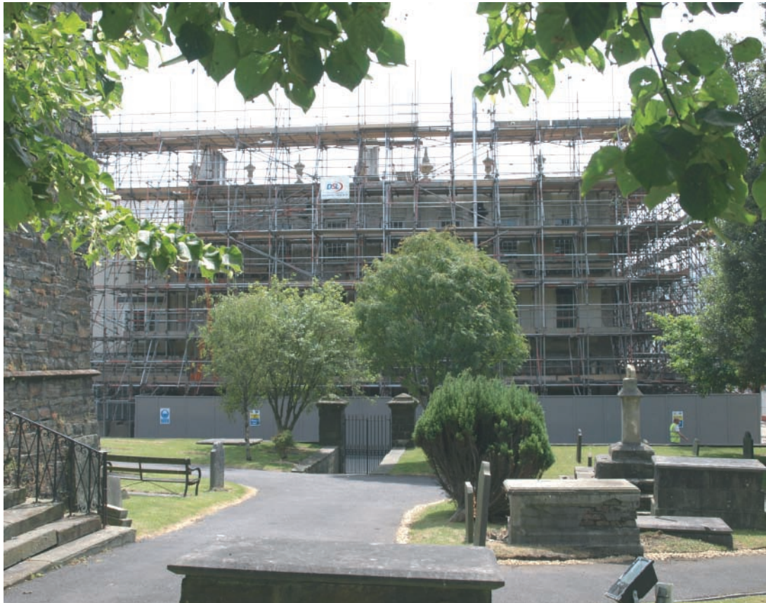
Plate 25. Llanelly House - North facing elevation during erection of scaffolding and partial removal of external render. Looking south.
