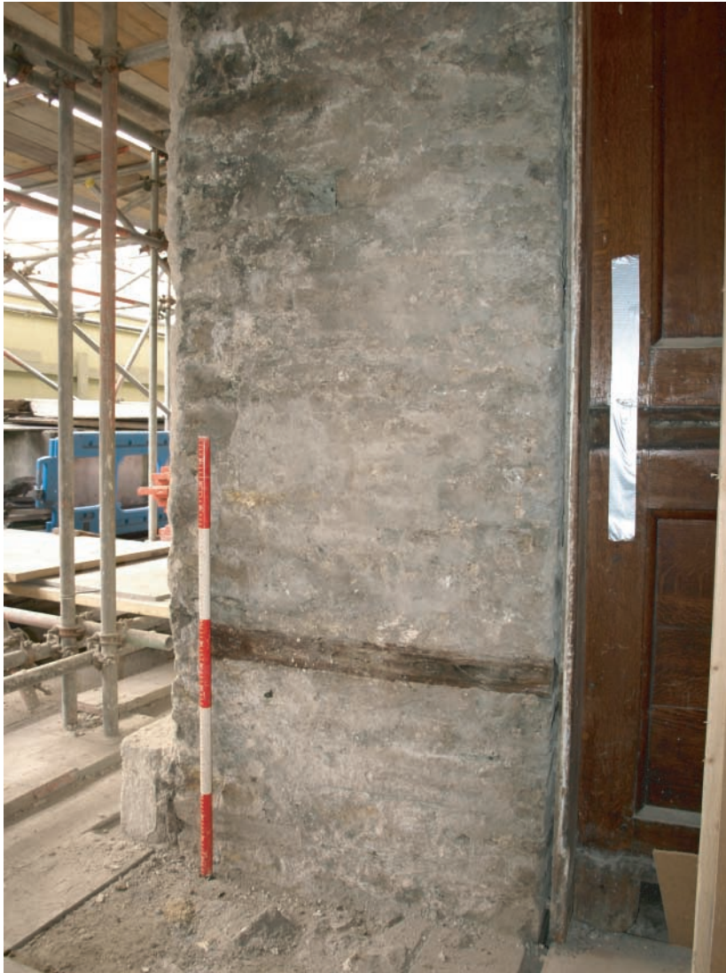
Plate 155. Llanelly House - The Great Hall (Room G1) - West facing former 18th century central doorway elevation revealed following removal of victorian rebuild.
