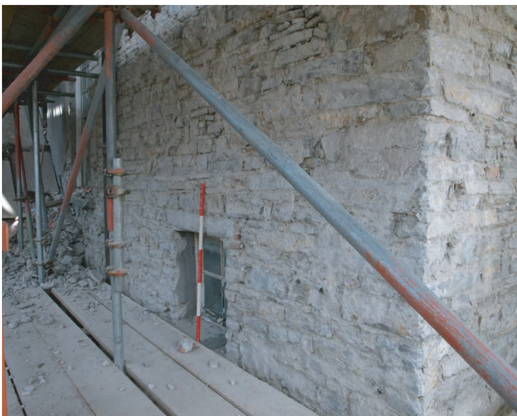
Plate 76. Llanelly House - Oblique view of south facing elevation at first floor level following removal of external render. Looking northwest.
