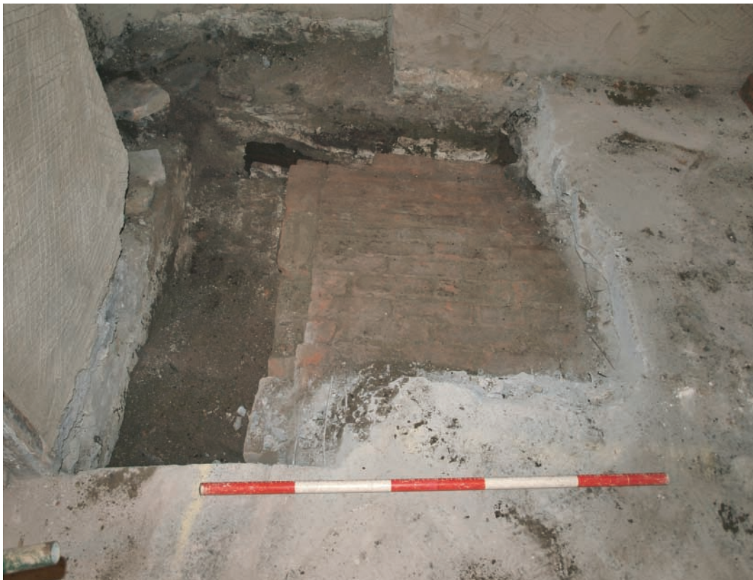
Plate 215. Removal of modern concrete floor in area of proposed lift shaft exposes the ceiling of victorian red brick cellar (Bay No.6). Looking west. Note remains of early oak timber floor joist.
