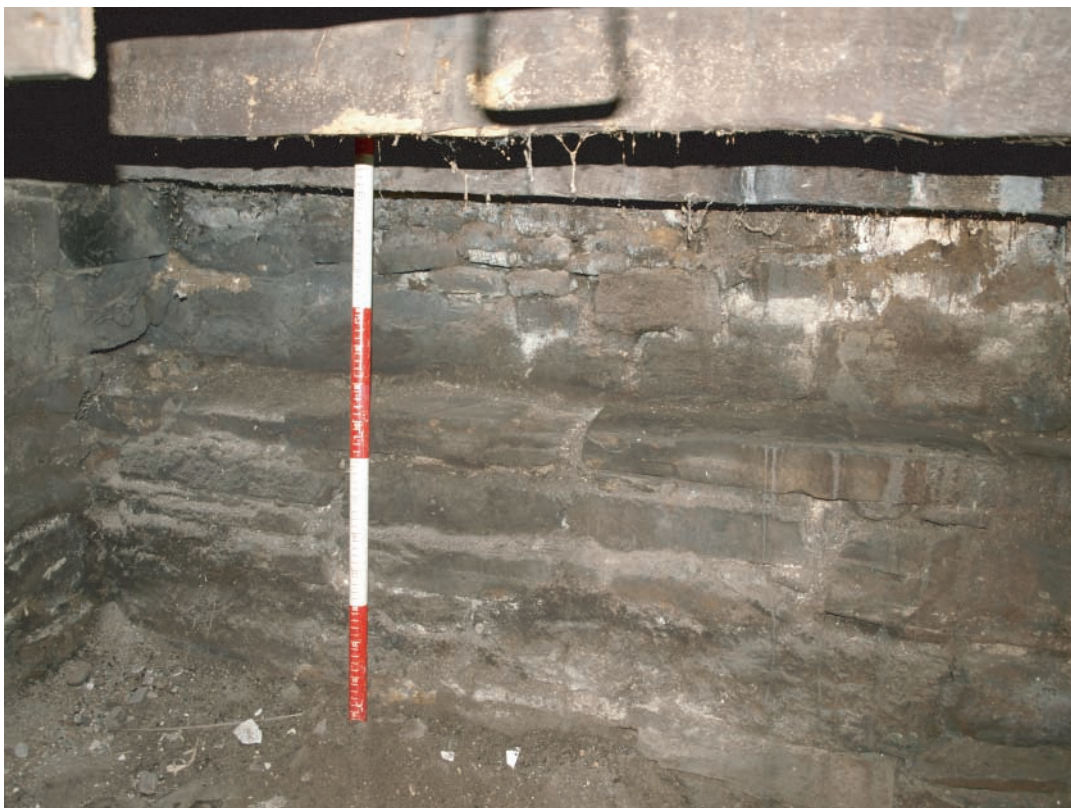
Plate 180. Llanelly House - Sir Thomas Stepney's Study (Room G2). View of base of north facing elevation in hidden basement room, showing position of former 17th century floor joist supporting ledge. Looking southeast.
