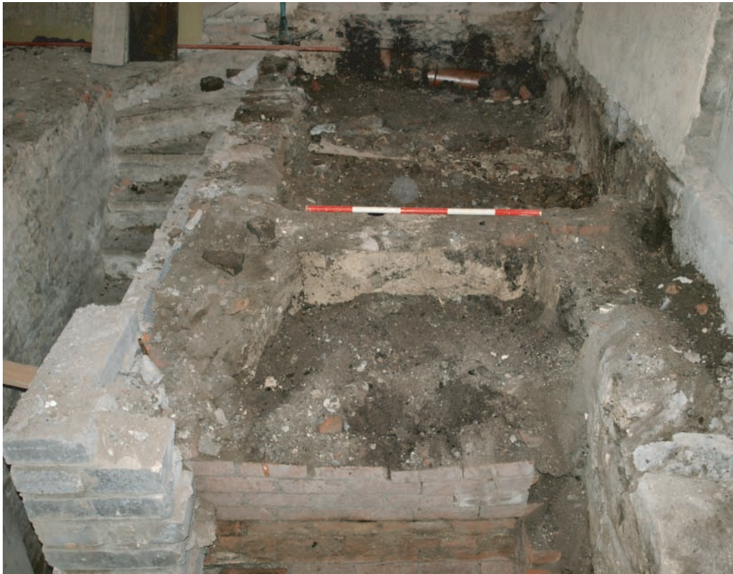
Plate 256. View of top of cross retaining wall at far southeast end of cellar following removal of concrete floor. Looking east.
