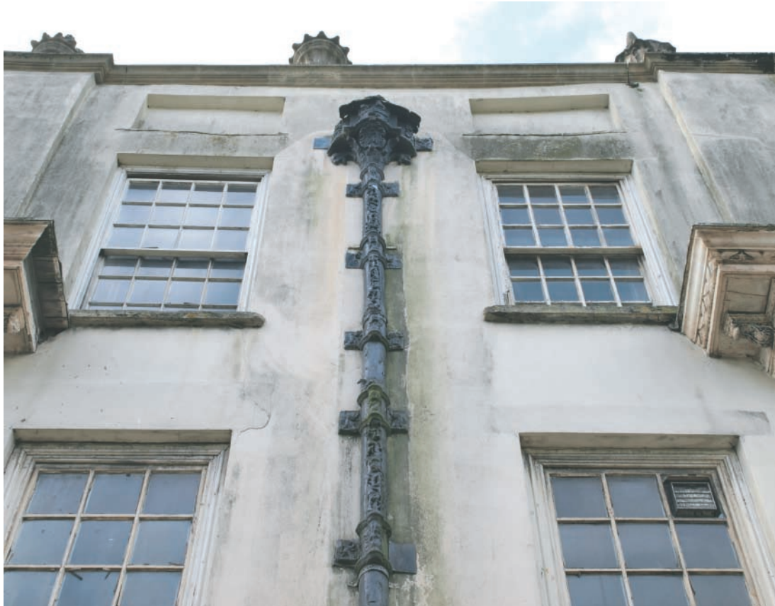
Plate 15. Llanelly House - Detail of cast iron and lead rain drainage pipe and hopper. on north facing elevation. Looking south.
