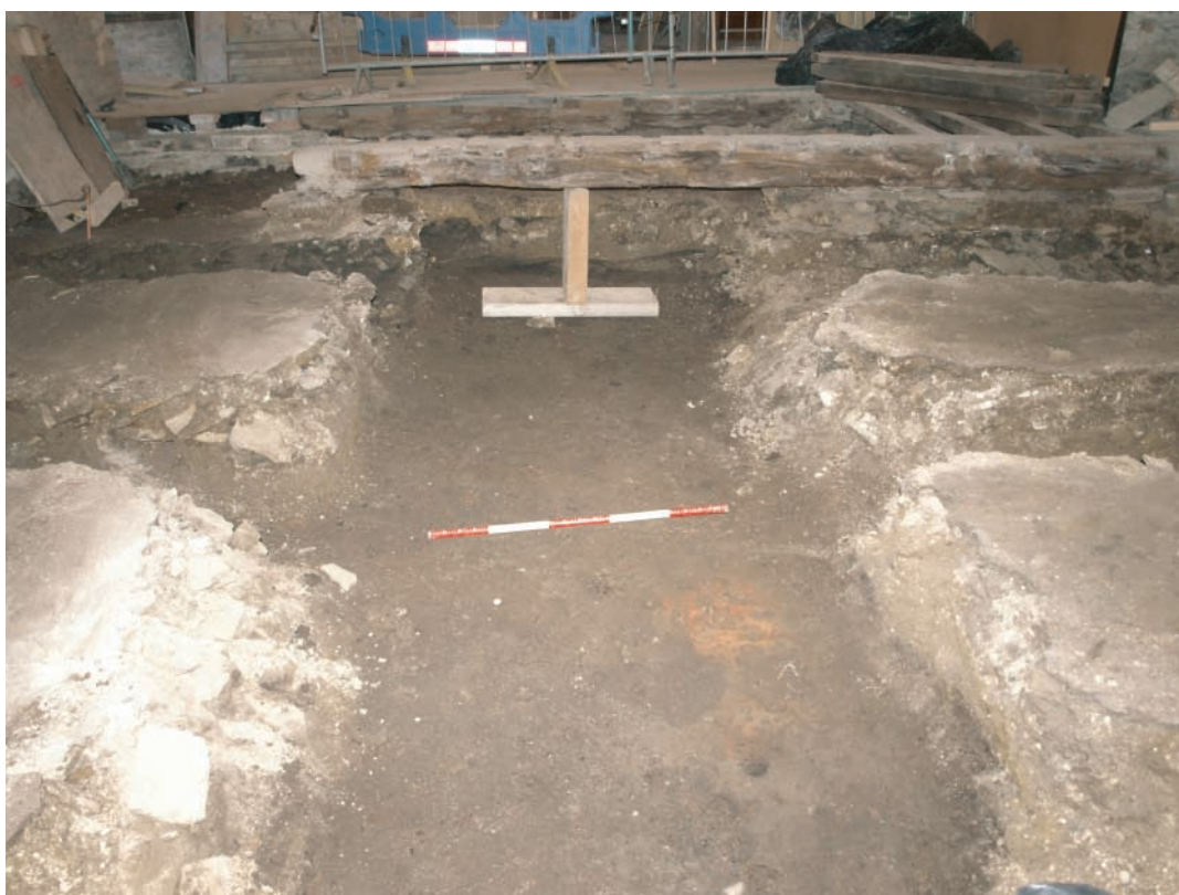
Plate 152. Llanelly House - The Great Hall (Room G1). View of excavated proposed concrete base trench and other new floor support trenches. Looking east.
