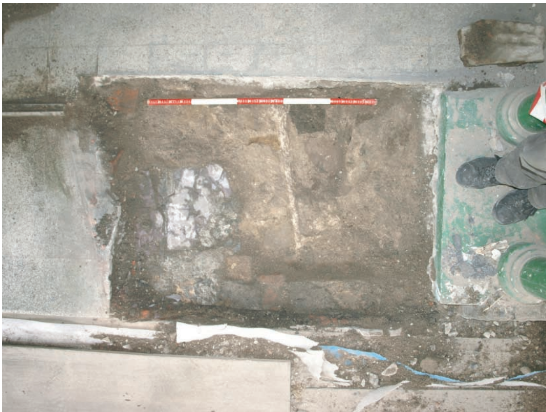
Plate 125. Llanelly House - The Great Hall (Room G1). Overhead view of evaluation trench at base of west wall following removal of victorian shopfront and concrete floor. Note remains of 18th century plaster outline marking extent of former fireplace opening. Photo taken from the northern side of the 19th century cast iron timber beam supports.
