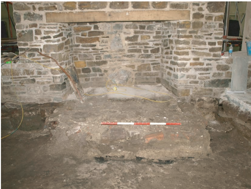
Plate 135. Llanelly House - The Great Hall (Room G1). View of remains of 18th century hearth foundation in front of newly constructed fireplace opening, built on the footprint of the 18th century fireplace opening. Looking west.
