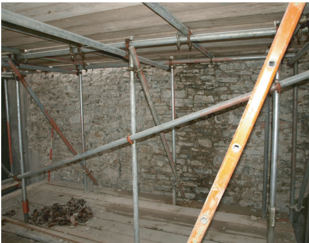
Plate 90. Llanelly House - Oblique view of east facing elevation at central upper level above former courtyard of western range. Note blocked in opening in centre of photo, suggestive of a former window opening, likely 18th century. Looking southwest.
