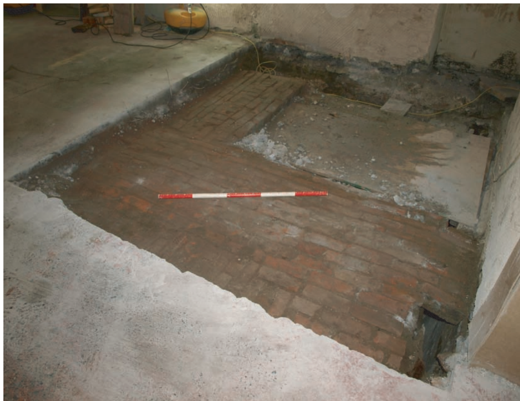
Plate 225. Further removal of modern concrete floor to accommodate lift shaft through victorian red brick cellar and Bay No. 6. Looking south.
