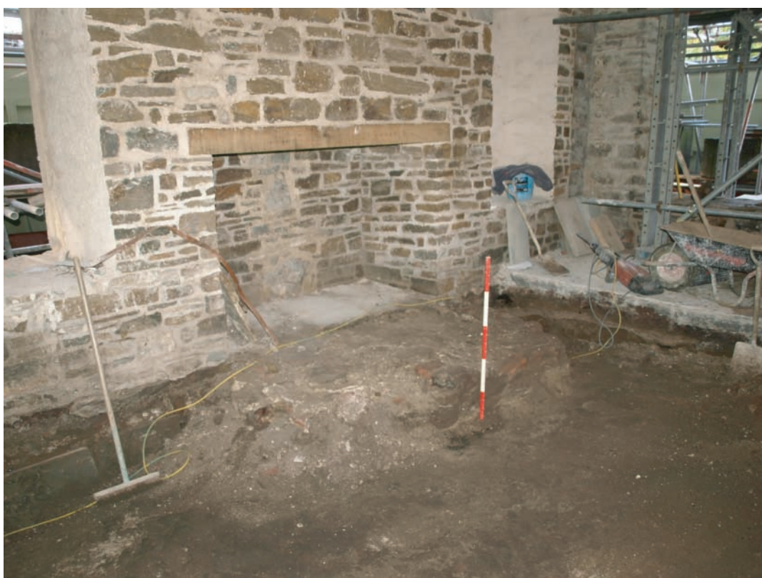
Plate 134. Llanelly House - The Great Hall (Room G1). View of remains of 18th century hearth foundation in front of newly constructed fireplace opening, built on the footprint of the 18th century fireplace remains. Looking northwest.
