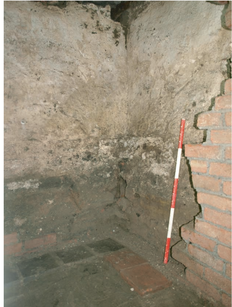
Plate 219. Section of victorian red brick cellar removed for proposed lift shaft, exposing earlier cellar wall. Looking south.
