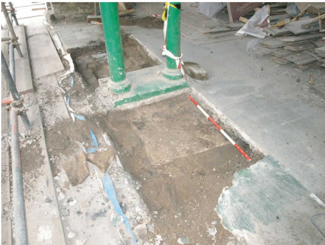
Plate 124 Llanelly House - The Great Hall (Room G1). Shot showing small evaluation trench at base of former victorian shopfront in west wall. Trench inserted in order to ascertain existence, character and extent of former 18th century fireplace. Looking northwards..
