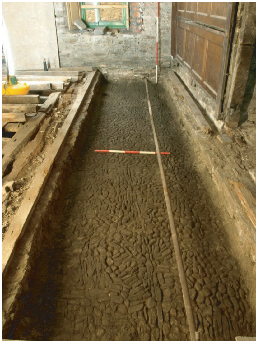
Plate 116. Llanelly House - The Great Hall (Room G1) - View of exposed 16th - 17th century cobbled floor, following removal of overburden (demolition material). Note framed pictorial cobble work in foreground. Looking north.
