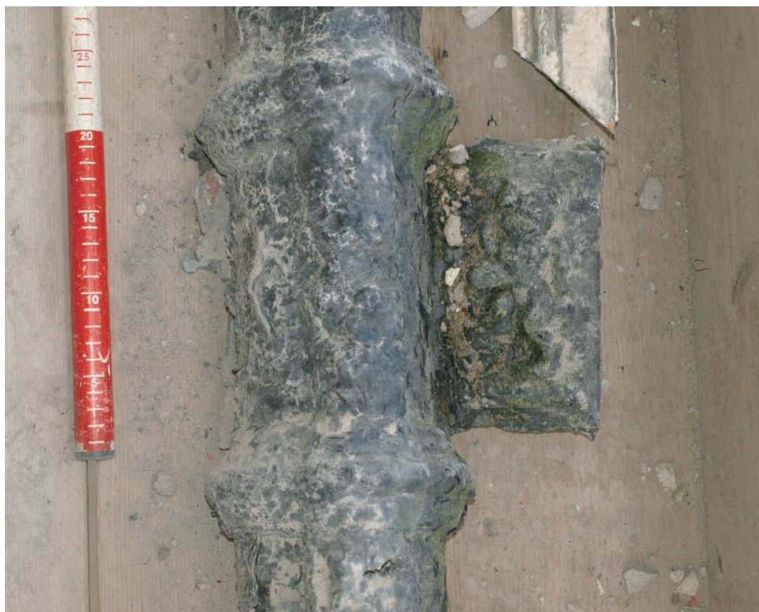
Plate 54. Llanelly House - Detail of lead drain pipe from west facing elevation. Shows lion motif and wild boar, the latter hard to discern from this photo.
