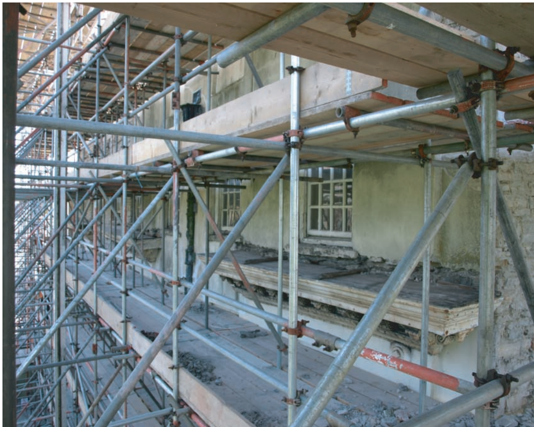
Plate 28. Llanelly House - North facing elevation during erection of scaffolding and partial removal of external render. Third floor level. Looking southeast.
