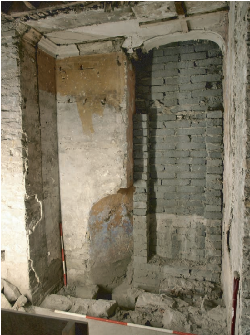
Plate 265. Remains of former 17th - 18th century opening exposed following removal of stone blocking in at far northeastern corner of Service Hall. Opening once linked Llanelly House with what is now the West Credit Union building. Looking northwards.
