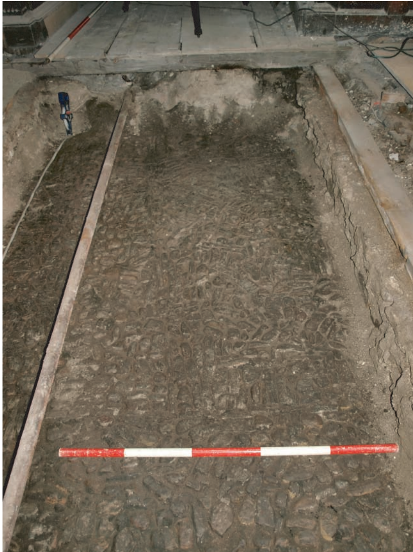
Plate 118. Llanelly House - The Great Hall (Room G1) - View of exposed 16th - 17th century cobbled floor, following removal of overburden (demolition material). Detailed shot of area of framed pictorial cobbled area. Looking south.
