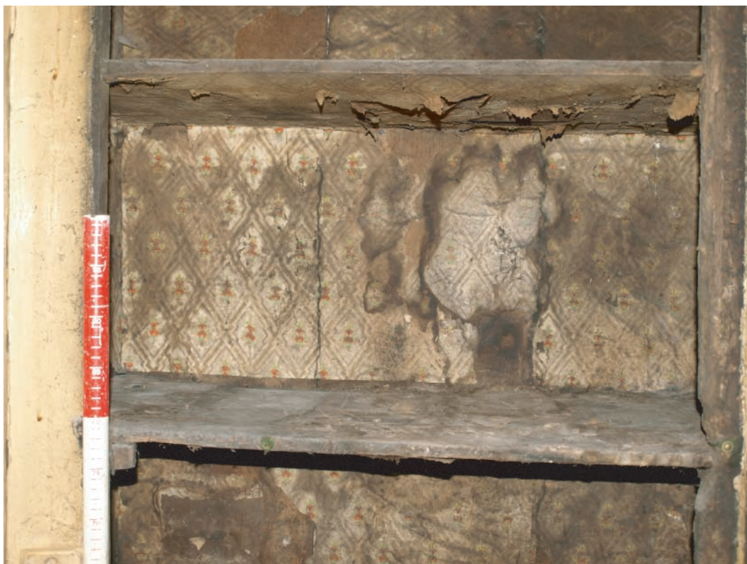
Plate 171. Llanelly House - Sir Thomas Stepney's Study (Room G2). Detail shot of handpainted wallpaper at back of cupboard following cleaning and recording work.
