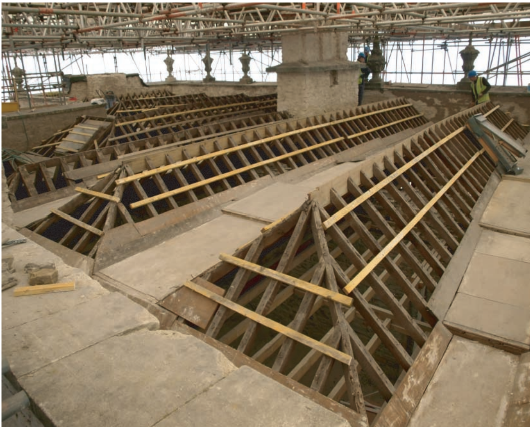
Plate 93. Llanelly House - Roof area in process of repair following removal of slates and irreparable timbers. Looking northwest from southeastern corner of roof.
