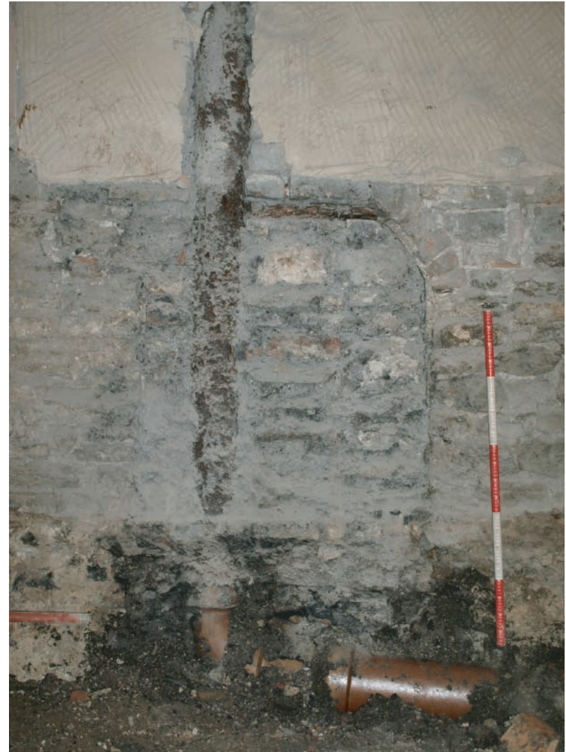
Plate 261. Enlarged view of blocked opening in area of secondary stairs in east wall. Opening cut by early 20th century foul drainage pipe. Looking east.
