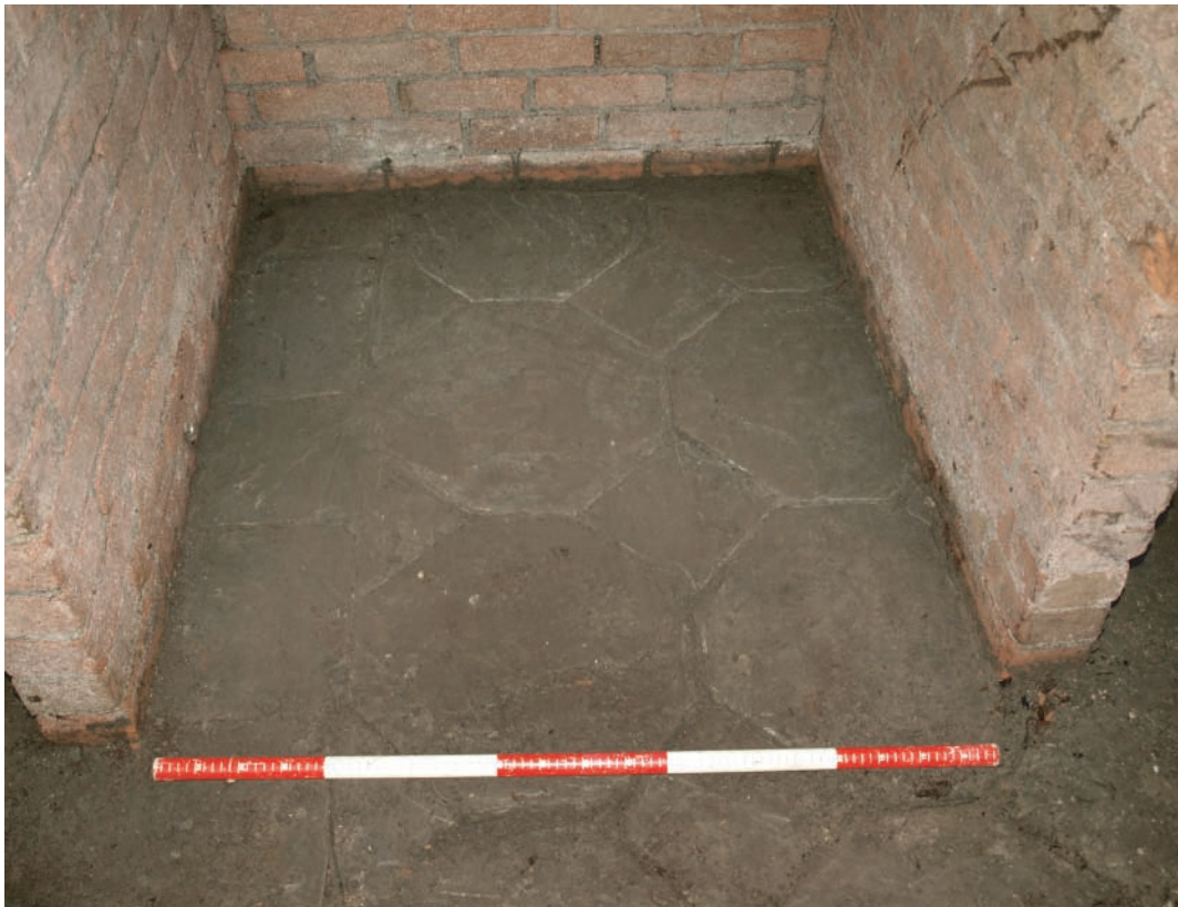
Plate 212. Detail of octagonal cut flagstones at east end of cellar floor.
