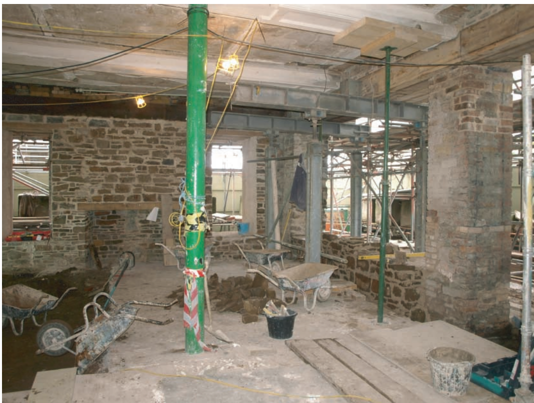
Plate 127. Llanelly House - The Great Hall (Room G1). Working shot during construction of new north and west facing walls following removal of victorian shopfronts and consolidation of timber bessemer beams. Looking northwest.
