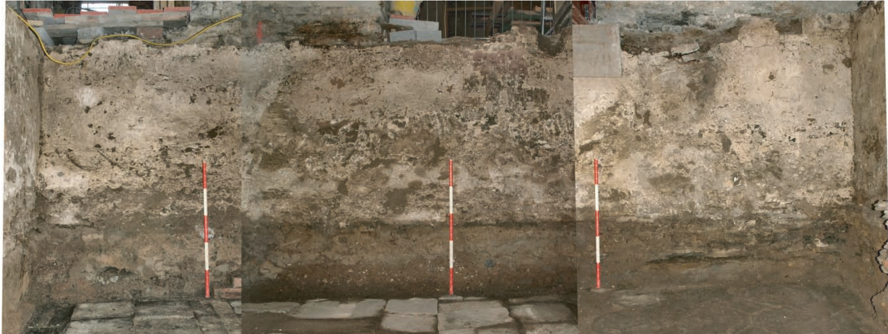
Plate 263. Composite photograph of south facing elevation of former 18th and early 19th century cellar following removal of Late 19th century red brick cellar. Looking north.
