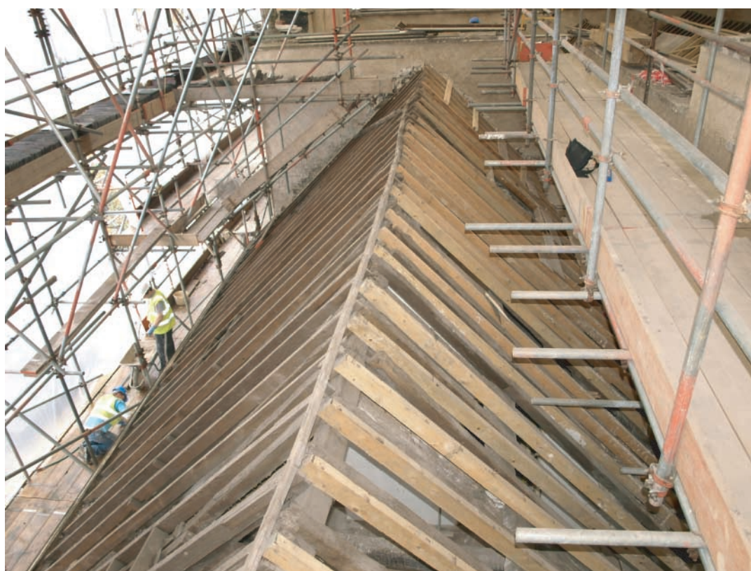
Plate 99. Llanelly House - Roof of western range following removal of slates. Looking northwards.
