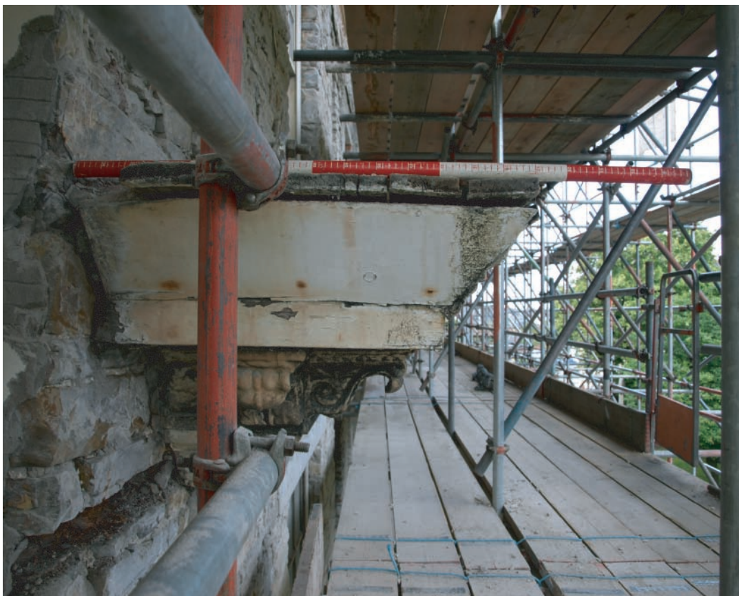
Plate 41. Llanelly House - West looking view detailing the profile of one of the ornate entablatures in the north facing elevation.
