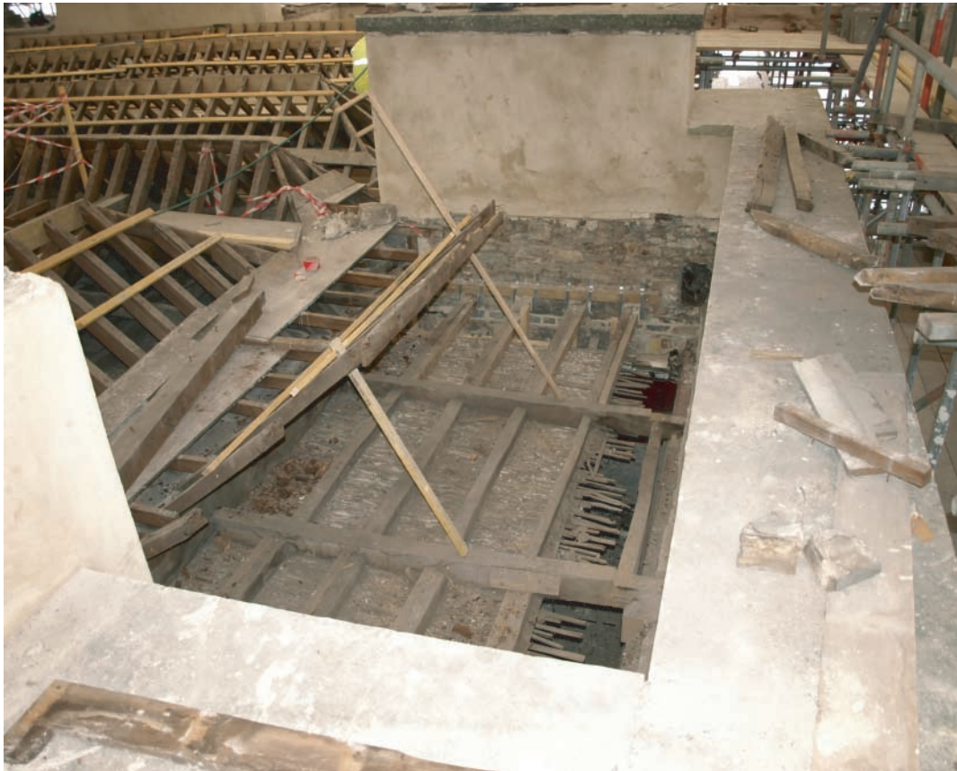
Plate 96. Llanelly House - Roof area in process of repair following removal of slates and rotten timbers. Looking west.
