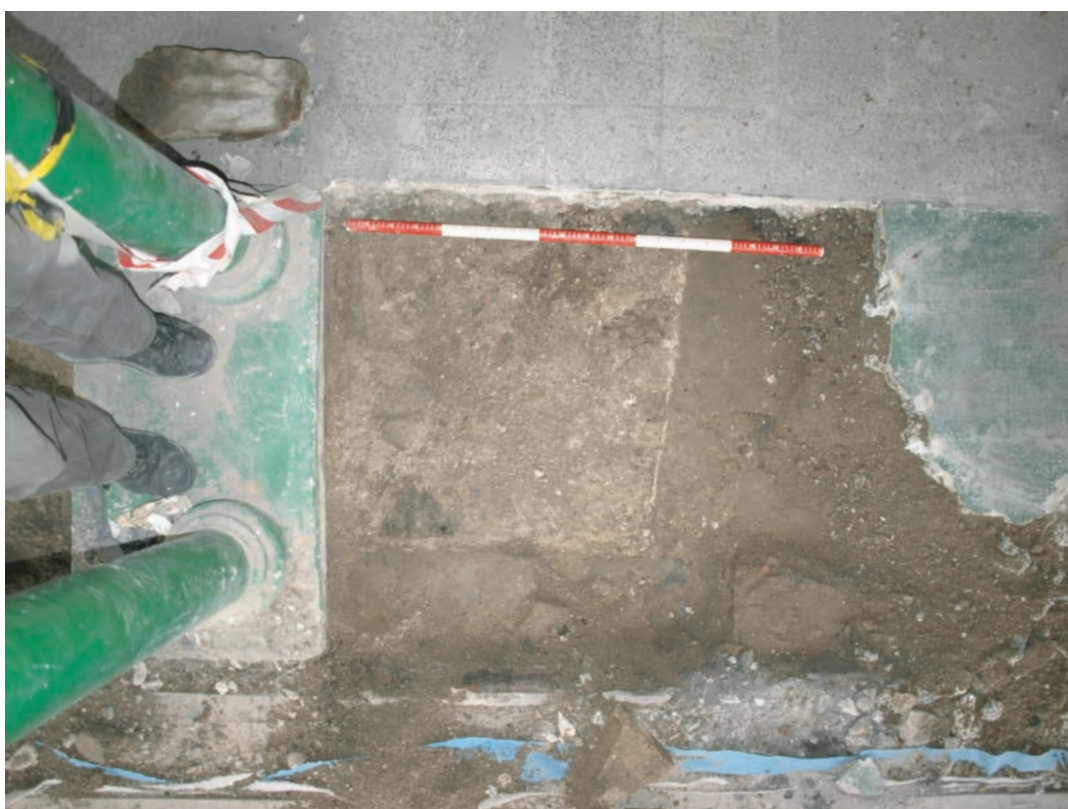
Plate 126 Llanelly House - The Great Hall (Room G1). Overhead view of evaluation trench at base of west wall following removal of victorian shopfront and concrete floor. Note remains of 18th century plaster outline marking extent of former fireplace opening. Photo taken from the southern side of the 19th century cast iron timber beam supports.
