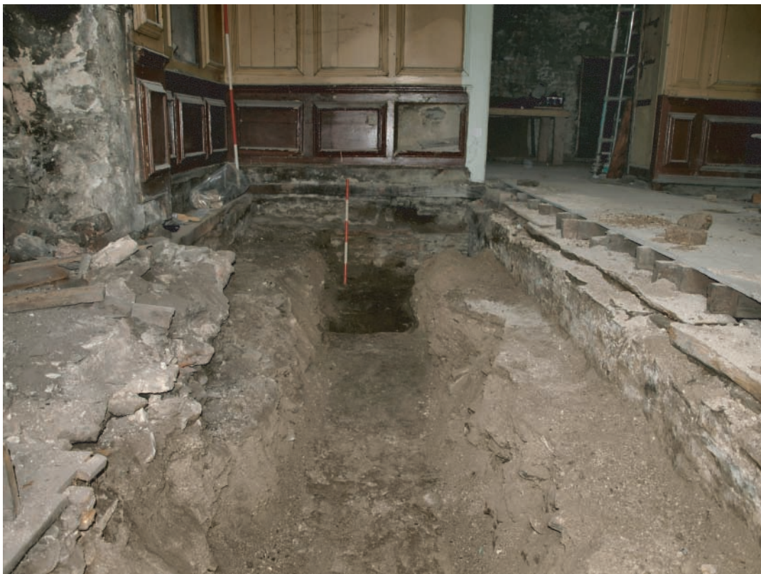
Plate 188. Llanelly House - Sir Thomas Stepney's Study (Room G2). View along floor support trench at east side of room. Trench cut through 18th century overburden onto natural clay floor. Looking south.
