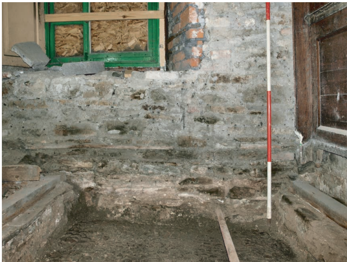
Plate 115. Llanelly House - The Great Hall (Room G1). View of lower section of eastern end of north facing elevation following removal of floorboards and demolition material. Note 16th - 17th century cobbles in foreground and mark in fabric, where the former 18th century front door would have been positioned. Unfortunately very little of this early feature is clearly visible due to its destruction in the 19th century following the creation of the Victorian shopfront. Looking north.
