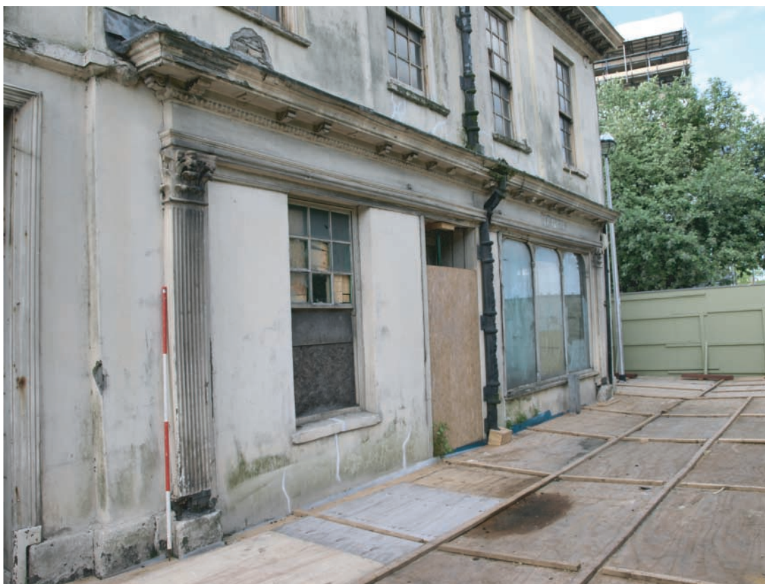
Plate 6. Llanelly House - Victorian shopfront in north facing elevation at west end. prior to restoration work. Looking southwest. Note original 18th century pilaster at left of photo alongside scale. Marks original central entrance.
