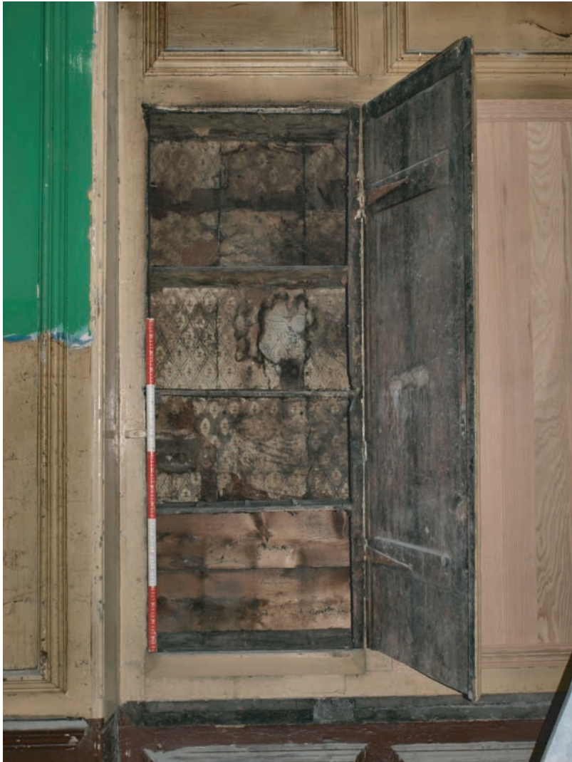
Plate 169. Llanelly House - Sir Thomas Stepney's Study (Room G2) - Spirit & Wine bottle label cupboard cleaned out of 19th century material following investigation and recording, revealing 18th century wallpapered cupboard. Looking east.
