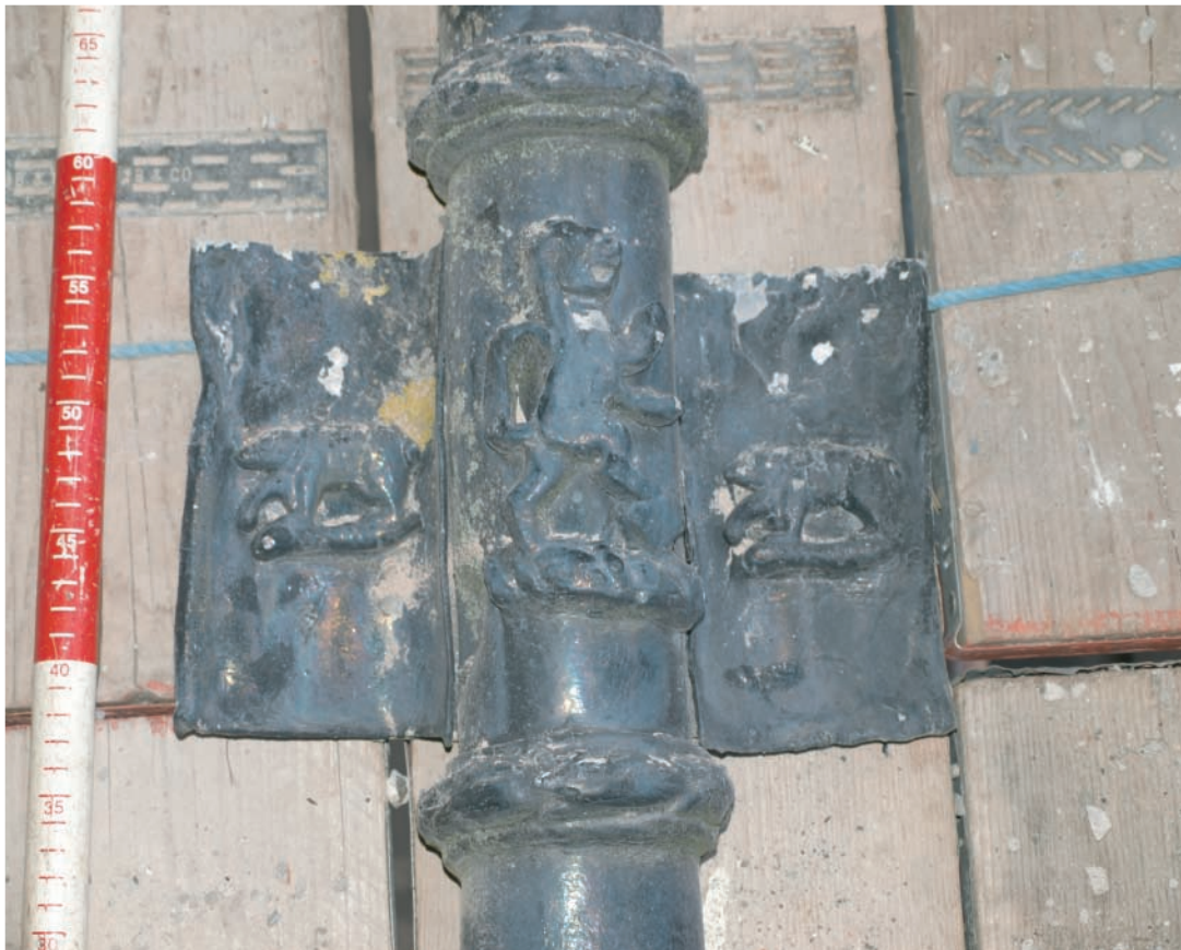
Plate 56. Llanelly House - Detail of lead drain pipe from west facing elevation. Shows prancing lion motif and wild boar or bear motif either side at mounting areas.
