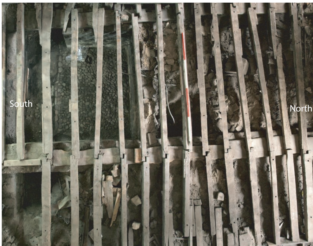
Plate 173. Llanelly House - Sir Thomas Stepney's Study (Room G2). Overhead view of timber floor joists following removal of floorboards and part clearance of overburden in hidden low basement store room.
