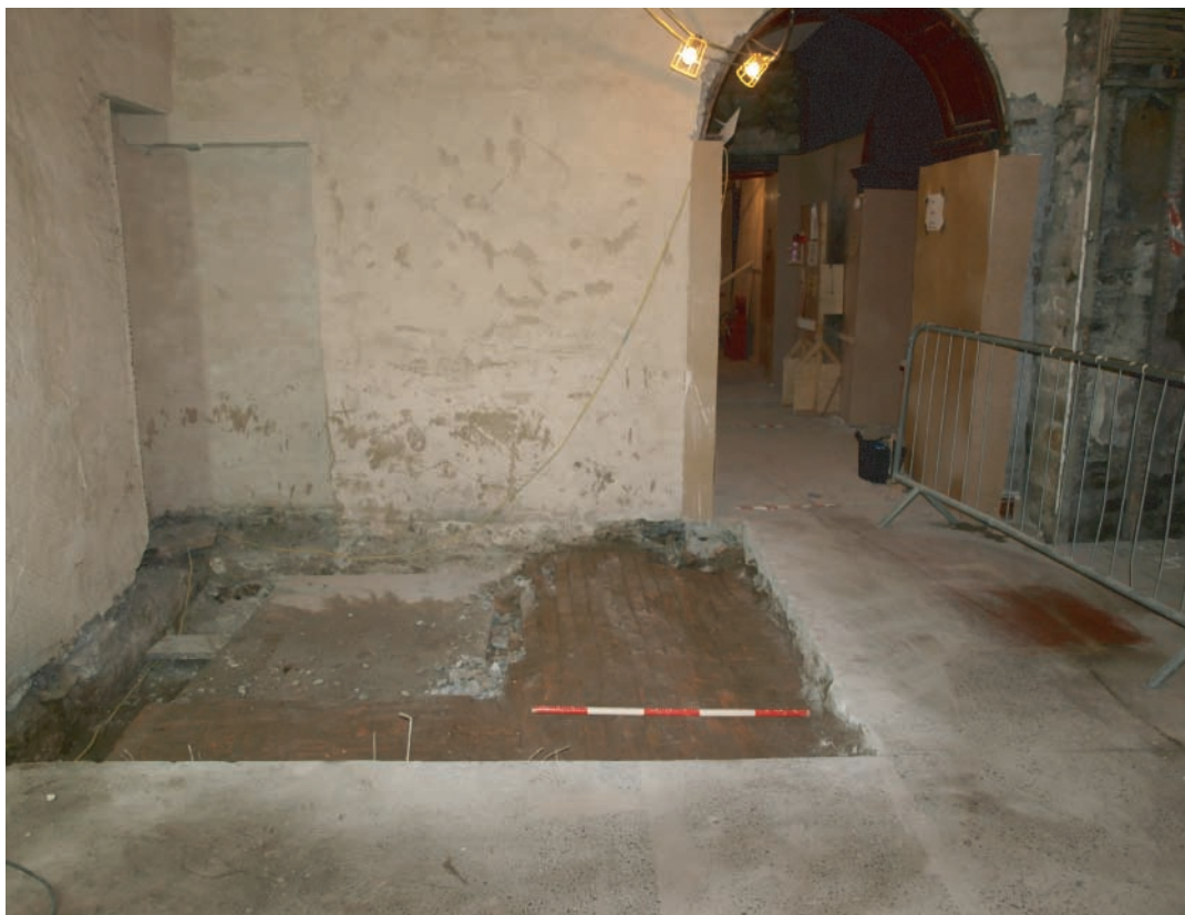
Plate 224. Further removal of modern concrete floor to accommodate lift shaft through victorian red brick cellar and Bay No. 6. Looking west.
