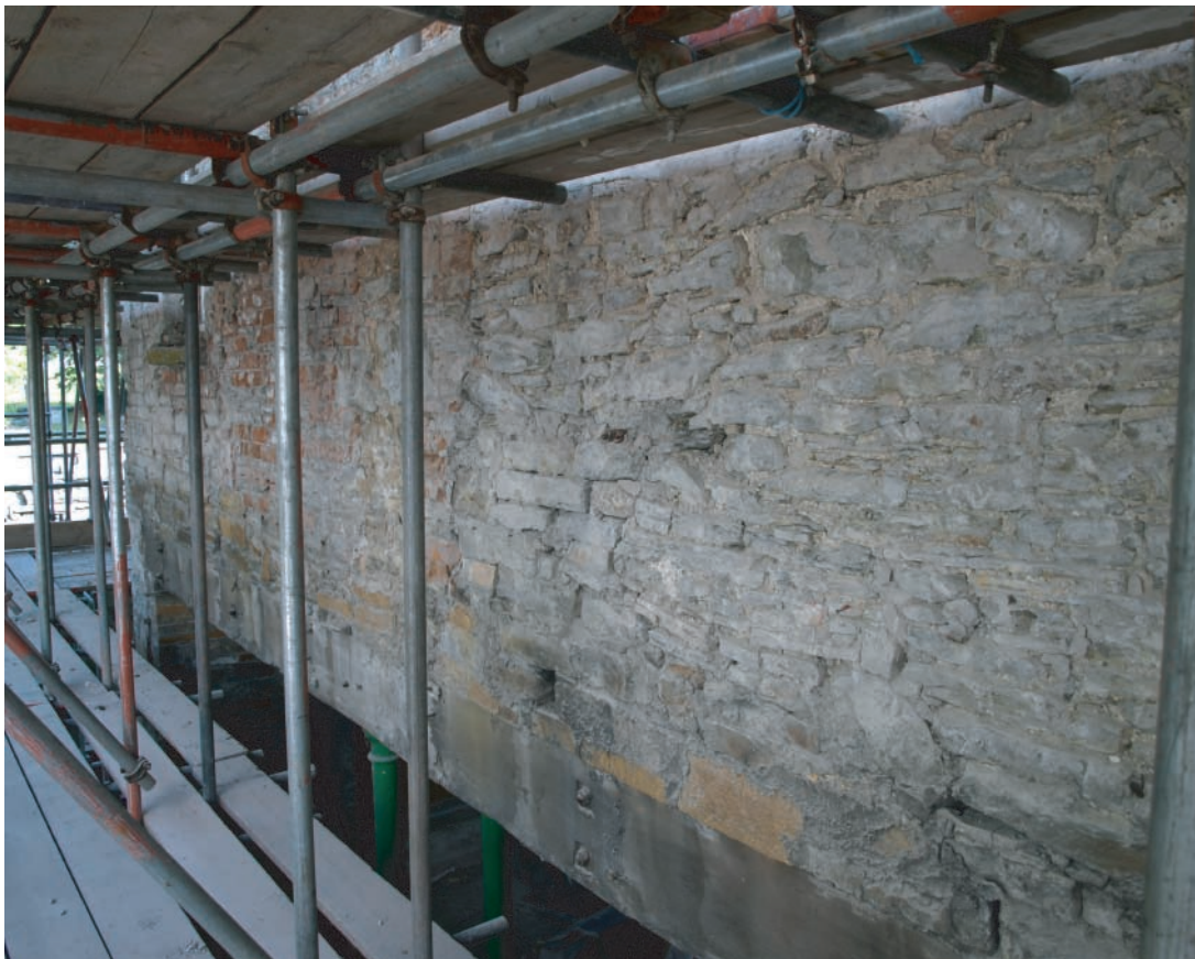
Plate 64. Llanelly House - View of oak bessemer beam exposed following removal of victorian shop front and external render in west facing elevation. Looking northwards.
