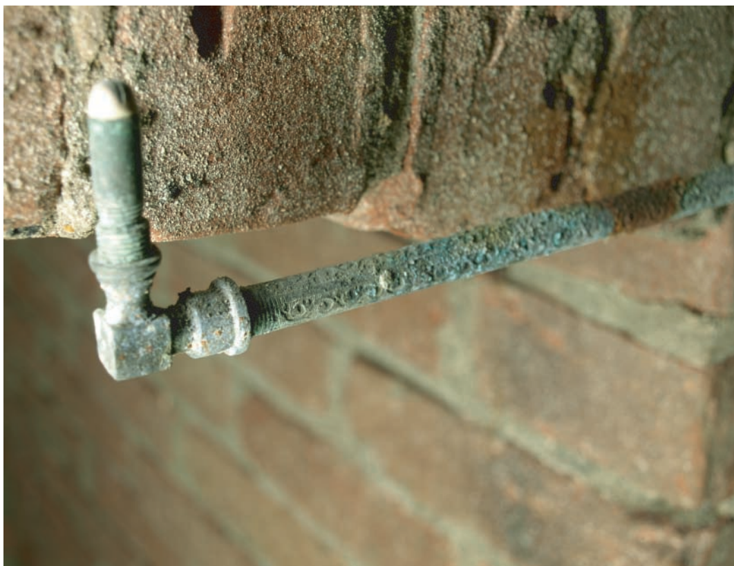
Plate 209. Closer view of gas-fitting showing scrolling detail on pipework.
