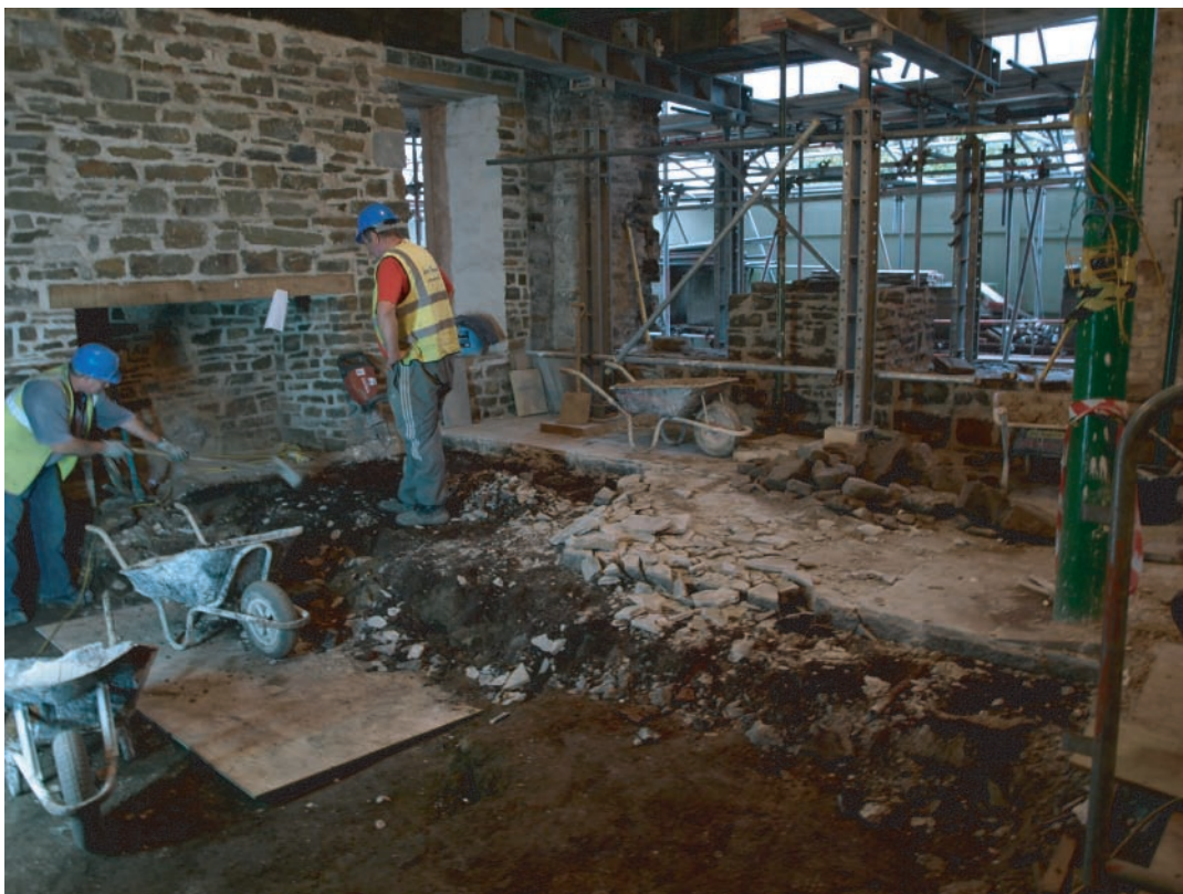
Plate 128. Llanelly House - The Great Hall (Room G1). Working shot during removal of modern concrete floor and ground reduction. Looking southeast.
