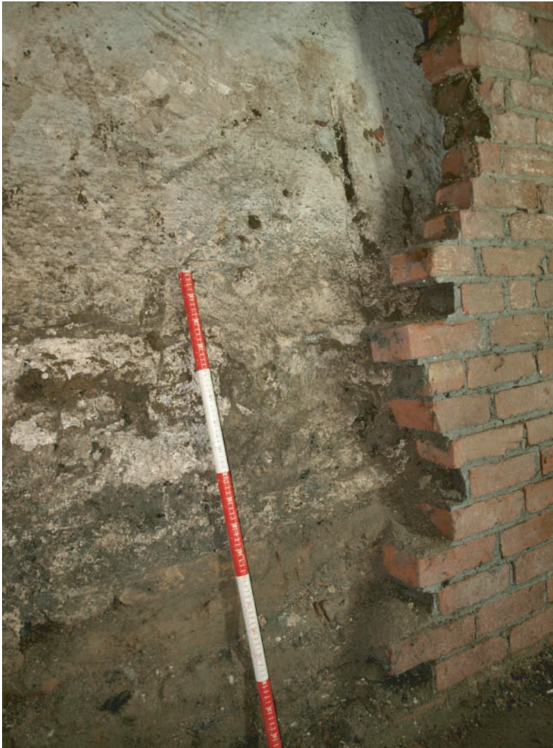
Plate 220. Exposed section of east facing elevation following removal of section of victorian red brick cellar for lift shaft insertion. Looking northwest.
