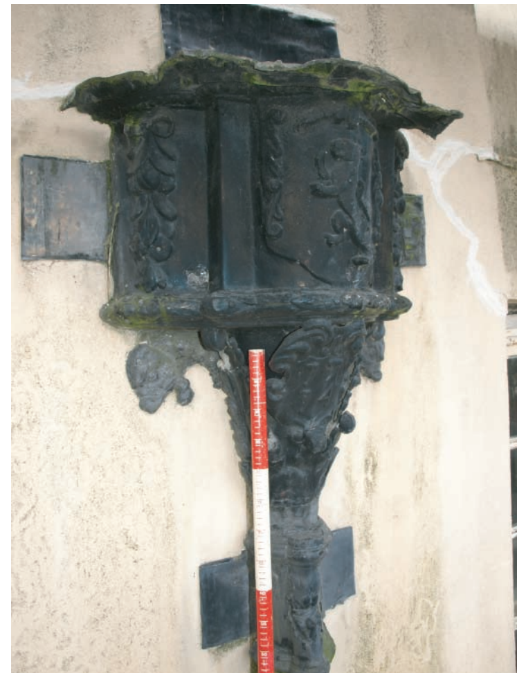
Plate 48. Llanelly House - View of lead hopper on north facing elevation. Note lion symbol and 1714 date on front of hopper neck. Looking east
