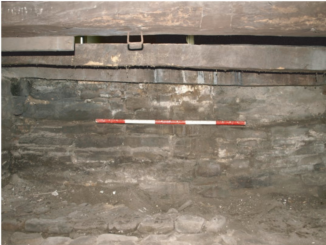
Plate 181. Llanelly House - Sir Thomas Stepney's Study (Room G2). View of base of north facing elevation in hidden basement room, showing position of former 17th century floor joist supporting ledge. Looking south.
