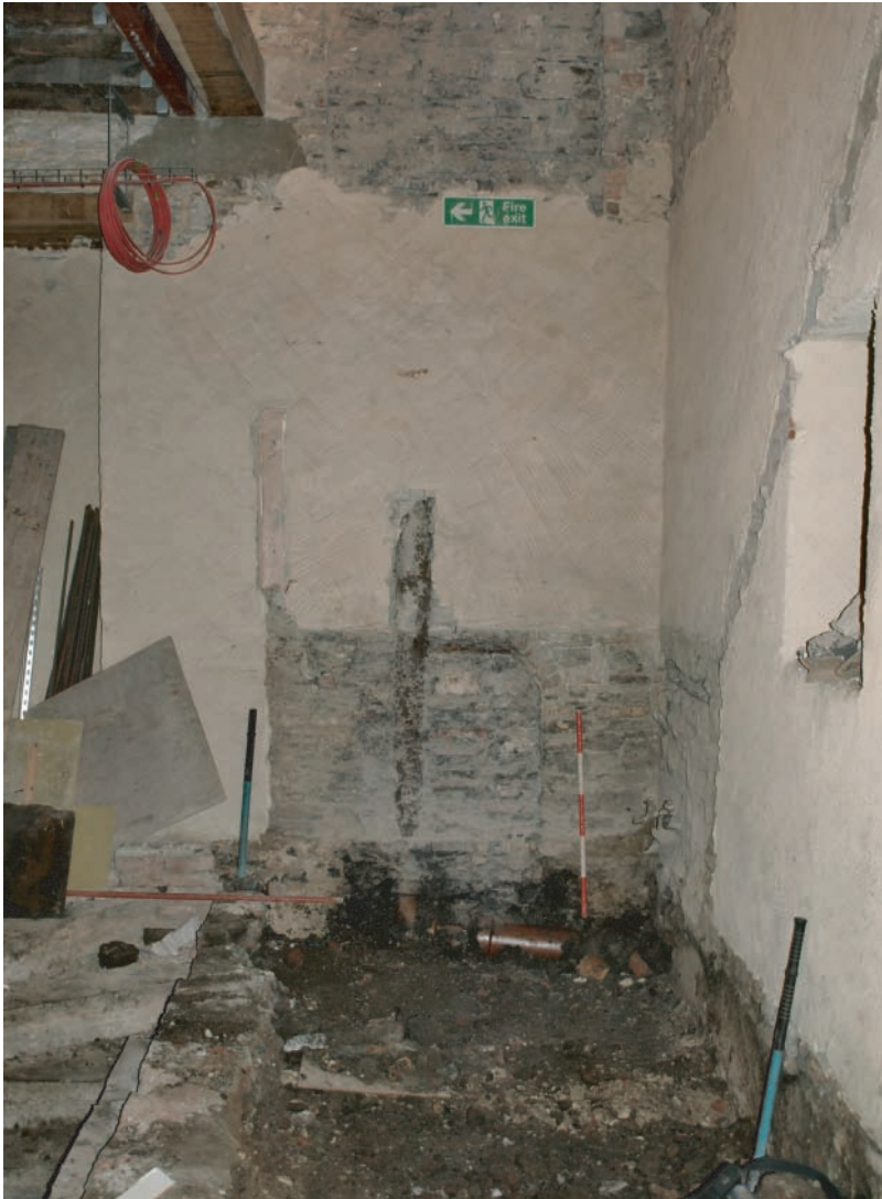
Plate 260. West facing elevation of Room G3, showing blocked in opening newly exposed following removal of secondary stairs and concrete floor. Looking east.
