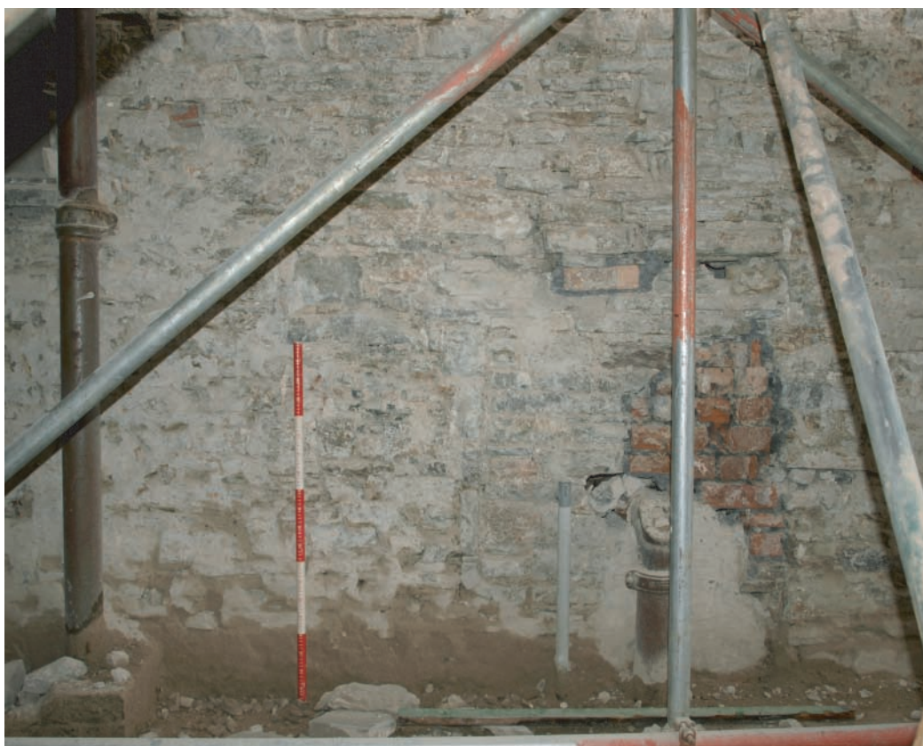
Plate 72. Llanelly House - Detail view of blocked in window feature at ground level in south facing elevation in rear courtyard area. Feature at right of photo, partly blocked in with red brick. Looking north.
