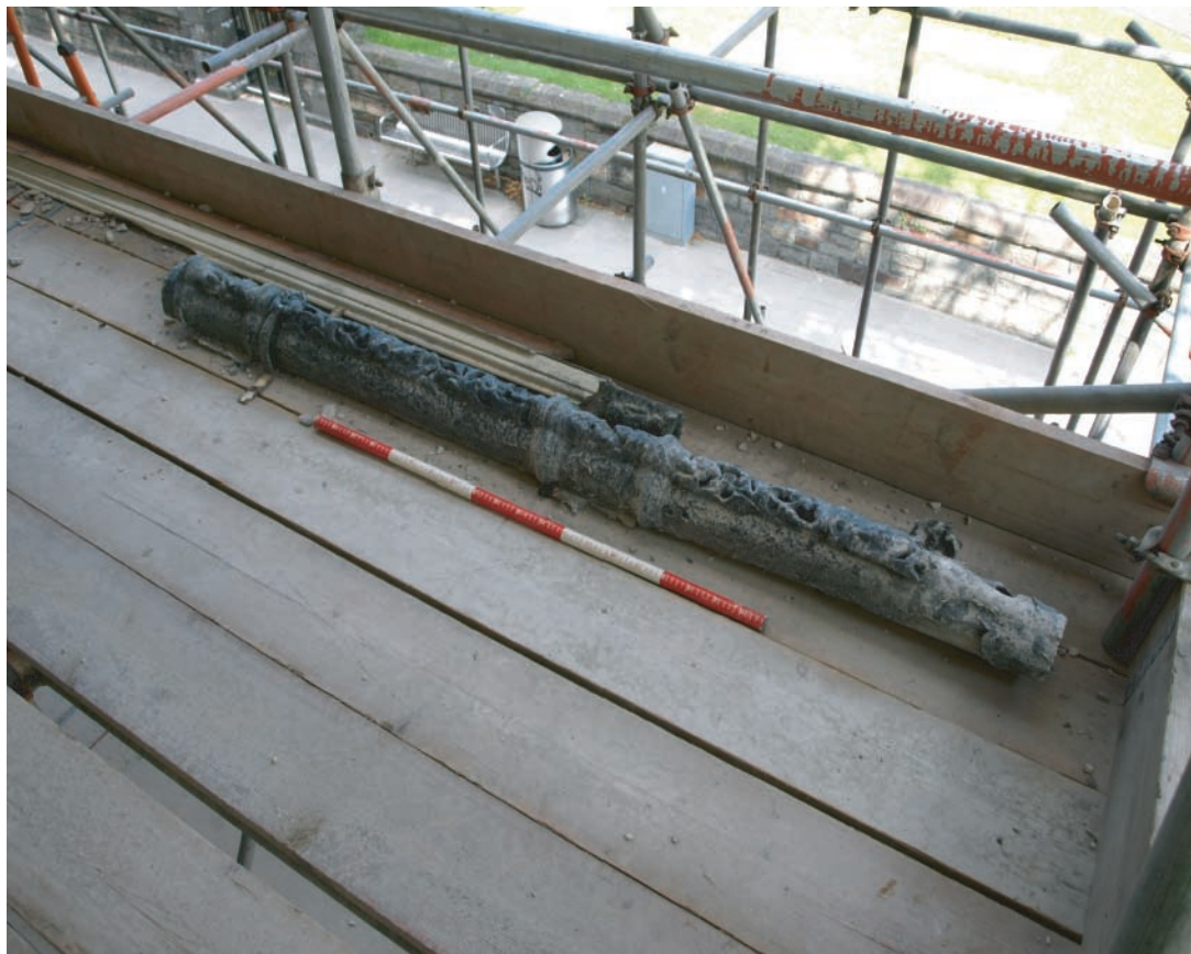
Plate 53. Llanelly House - View of length of lead rainweater drain pipe with leaded motifs. From west facing elevation.
