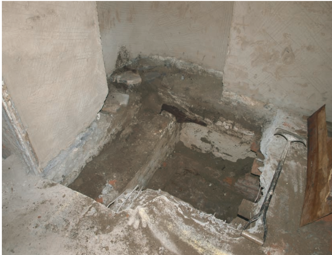
Plate 217. Concrete floor and section of red brick cellar ceiling now removed. Looking southwest.
