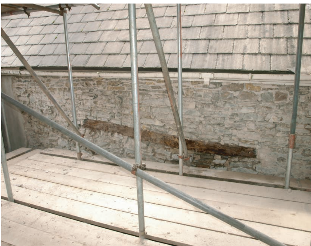
Plate 91. Llanelly House - Oblique view of east facing elevation at uppermost level above former courtyard of western range. Shows remains of former 18th century timber window lintel. Looking southwest.
