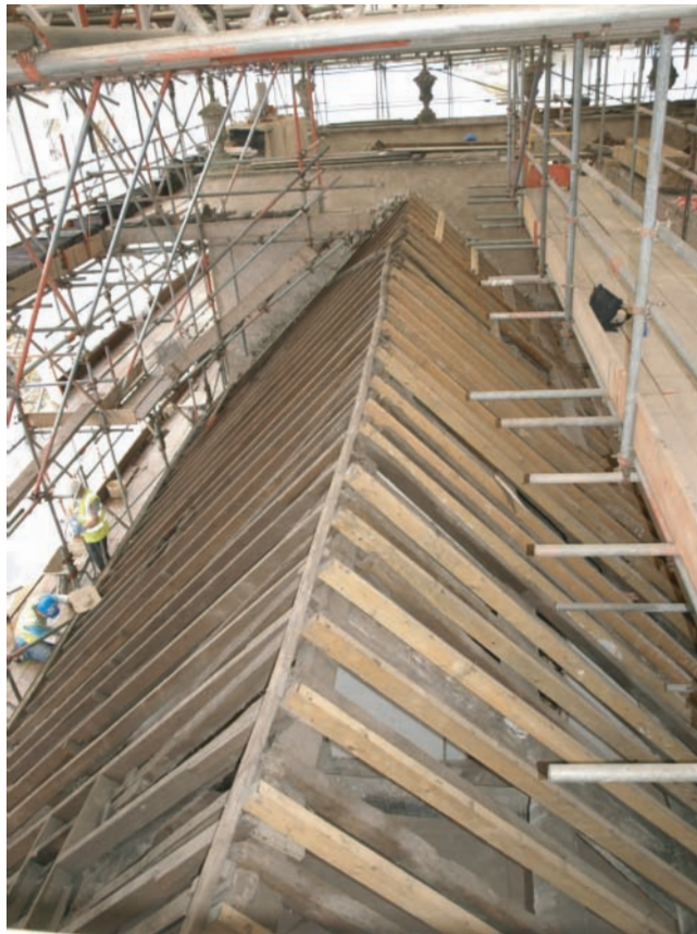
Plate 101. Llanelly House - Roof of western range following removal of slates. Looking northwards.
