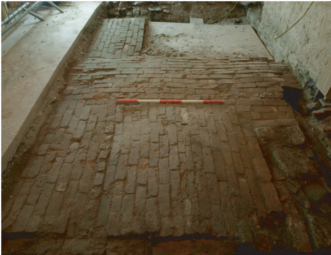
Plate 227. Further removal of modern concrete floor revealing victorian red brick cellar vaulted ceiling. Looking south.
