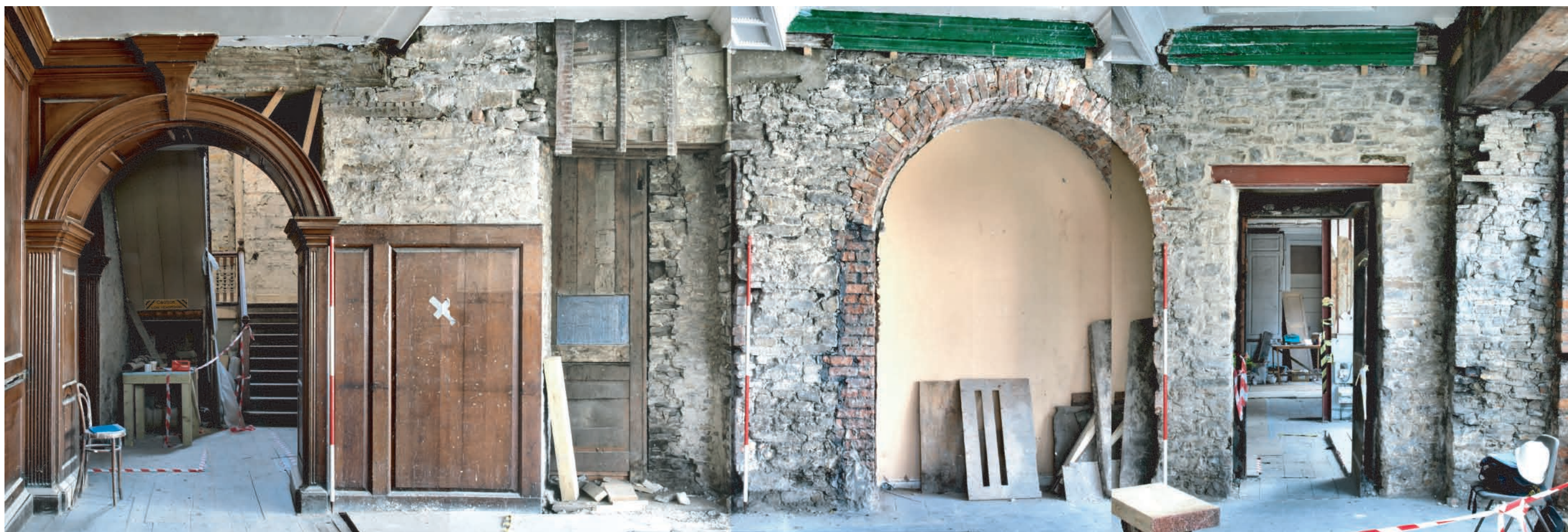
Plate 104. Composite photograph of north facing elevation of supposed Great Hall (Room G1), following removal of wall plaster from former contract work in 2003/03.
