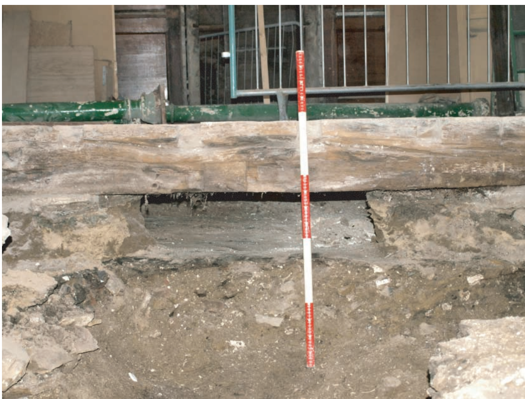
Plate 146. Llanelly House - The Great Hall (Room G1). West facing section of concrete base trench showing character and depth of deposits between the 18th century floor level (timber floor joist), the 17th century floor level and the late medieval floor level. Looking east.
