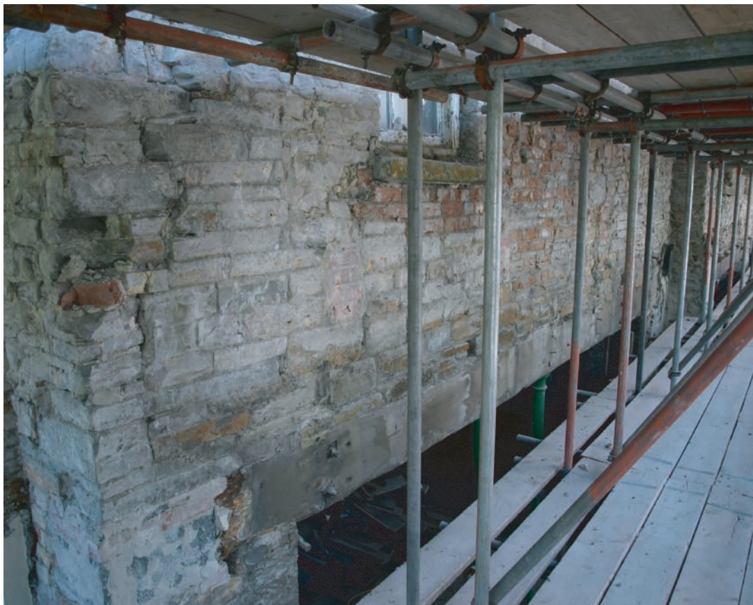
Plate 61. Llanelly House - View of oak bessemer beam exposed behind former victorian shop front in west facing elevation.
