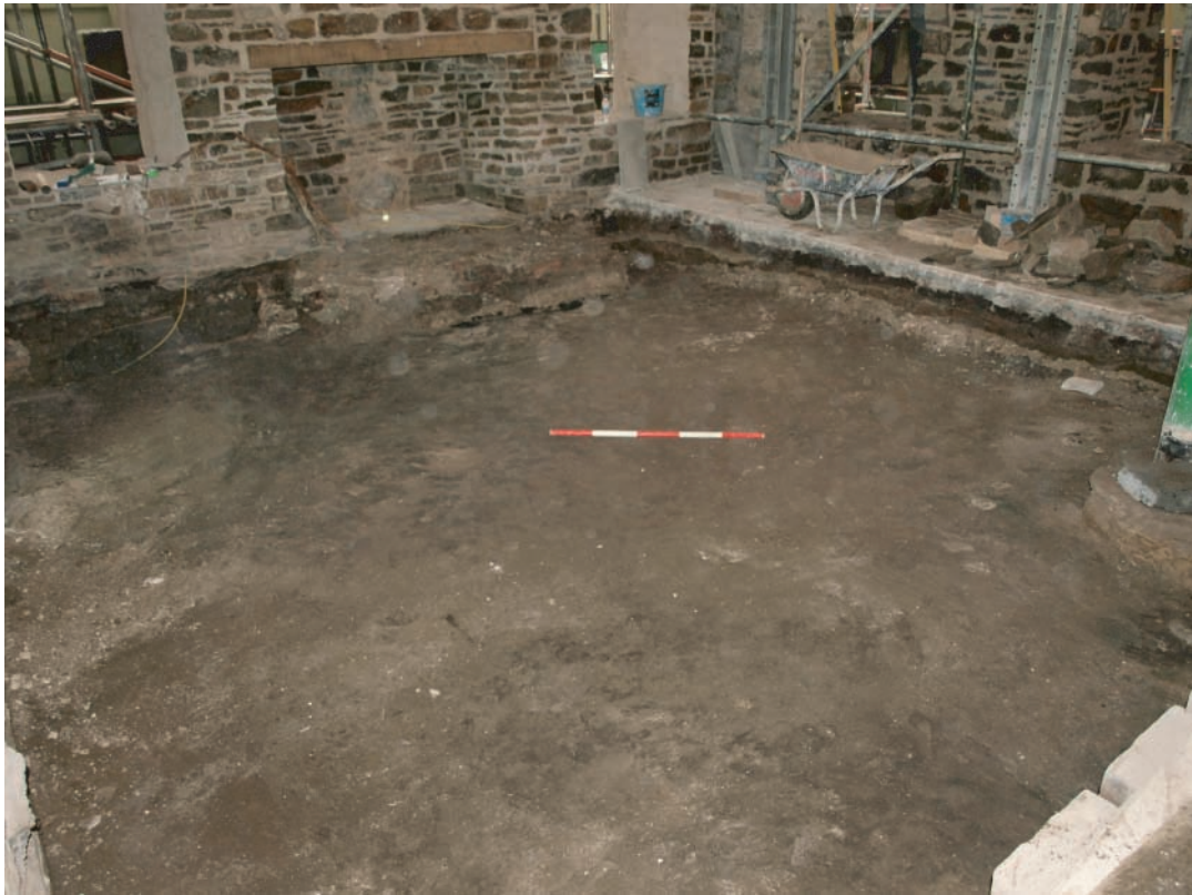
Plate 137. Llanelly House - The Great Hall (Room G1). View of former 17th century compacted earth floor ,following partial removal of overburden Looking north west.
