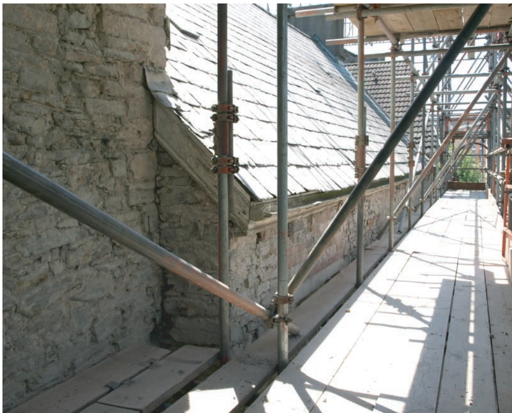
Plate 69. Llanelly House - View of first floor level in west facing elevation following removal of external render. Shows butt joint between west range and west facing elevation, but only at this upper level, suggesting that the roof line has been raised at some time. Looking southwards.
