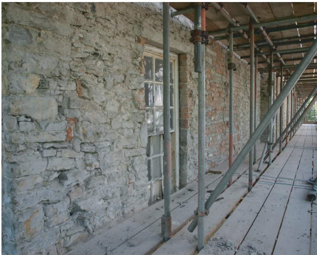
Plate 65. Llanelly House - View of first floor level in west facing elevation following removal of external render. Looking southwards.
