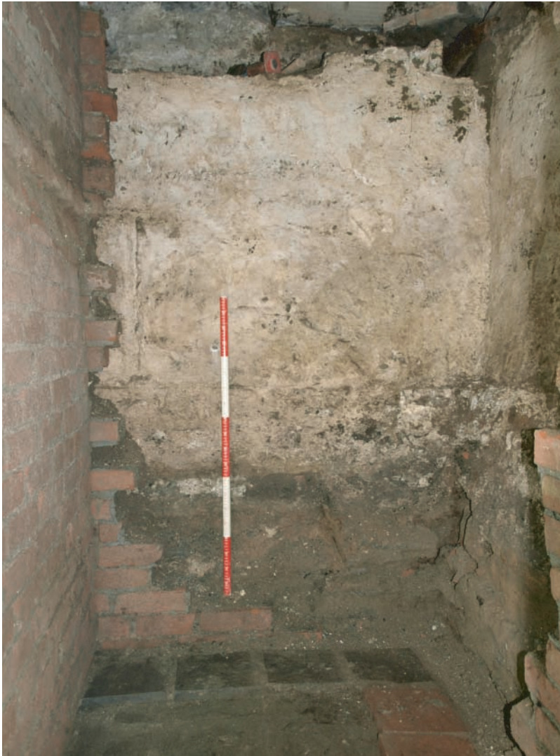
Plate 218. Section of victorian red brick cellar removed for proposed lift shaft, exposing earlier cellar wall. Looking south.
