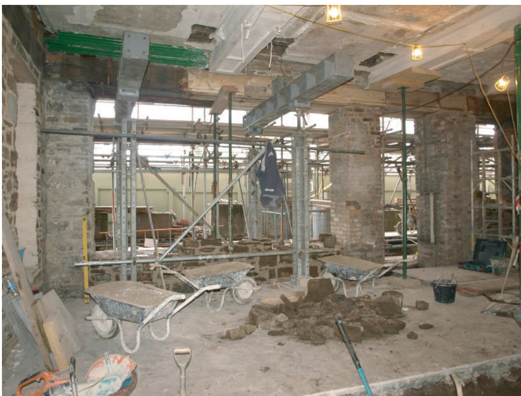
Plate 128. Llanelly House - The Great Hall (Room G1). Working shot during construction of new north and west facing walls following removal of victorian shopfronts and consolidation of timber bessemer beams. Looking north.
