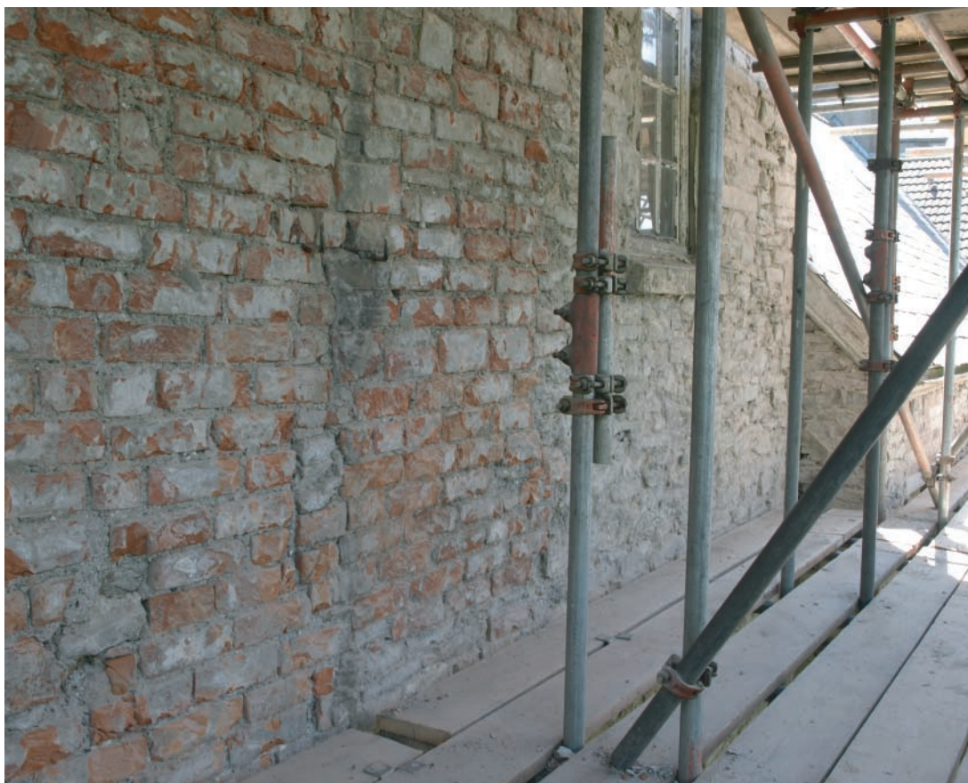
Plate 68. Llanelly House - View of first floor level above former victorian shop front in west facing elevation following removal of external render. Looking southwards. Note red brick repair in position of former projected chimney.
