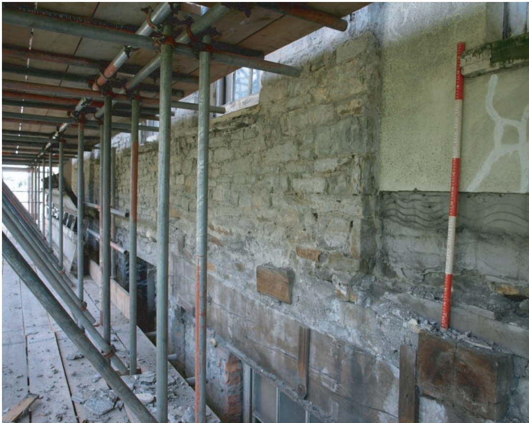
Plate 36. Llanelly House - Oblique view looking eastward toward position of victorian shopfront at west end of front facade, 1st level of scaffolding. Note oak bessemer beam. Looking southeast
