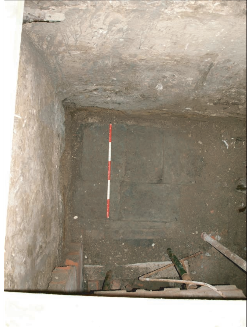
Plate 223. Section of flagstone cellar floor following removal of section of victorian red brick cellar for lift insertion at far southwestern corner.
