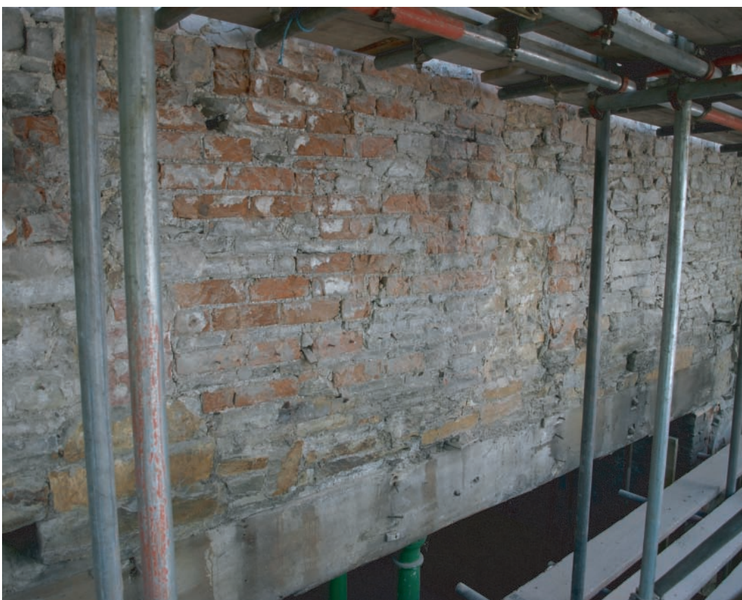
Plate 62. Llanelly House - View of red brick repair and oak bessemer beam exposed behind former victorian shop front in west facing elevation. Red brickwork was used to repair/replace the former projecting chimney that was present in the west facing elevation in the 18th century.
