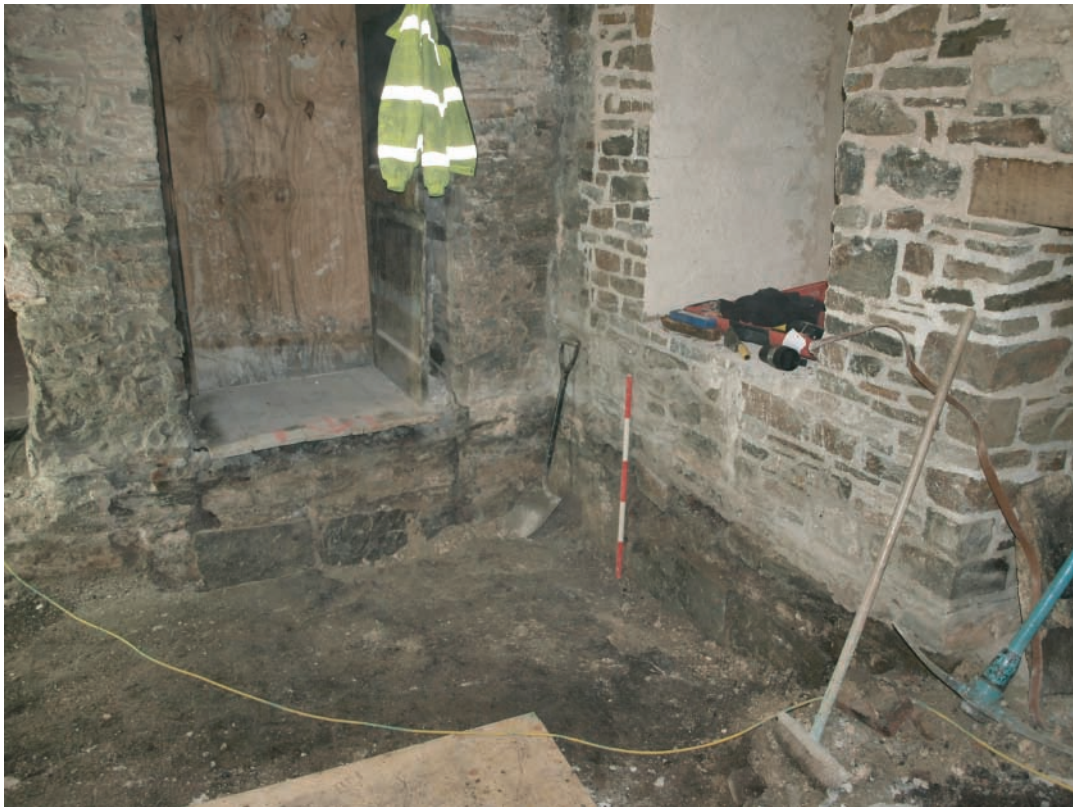
Plate 131. Llanelly House - The Great Hall (Room G1). View showing position of former lower doorway openings in south wall at west end and in west wall at southern end. Delineated by slate shutters? Looking southwest.
