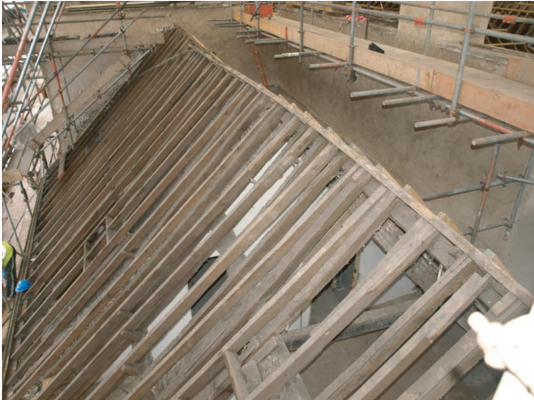
Plate 100. Llanelly House - Roof of western range following removal of slates. Looking northwards.
