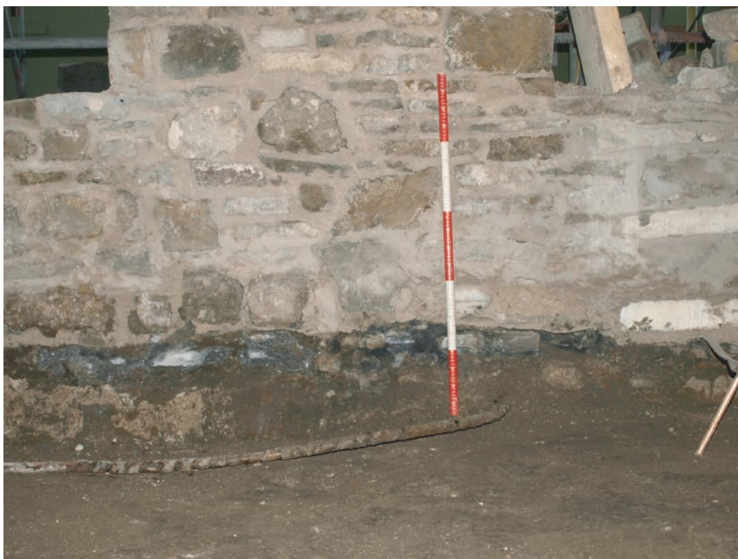
Plate 151. Llanelly House - The Great Hall (Room G1). South facing elevation following complete removal of modern concrete floor and 18th - 19th century overburden. Note remains of former 17th century wall plaster and position of former blocked in 17th century opening at base of newly constructed wall.
