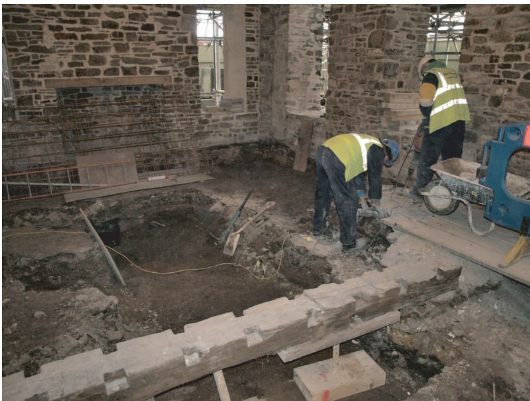
Plate 149. Llanelly House - The Great Hall (Room G1). Working shot during removal of remaining concrete floor against north wall. Looking northwest.
