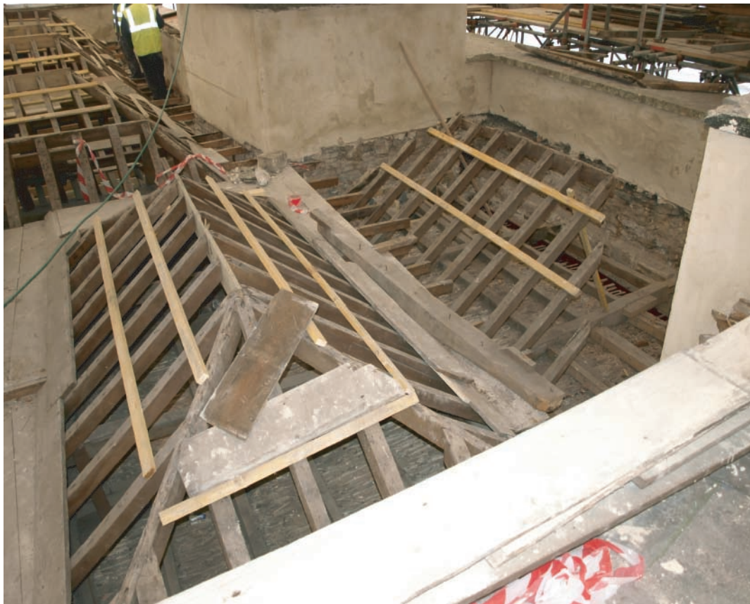
Plate 97. Llanelly House - Roof area in process of repair following removal of slates and rotten timbers. Looking north.
