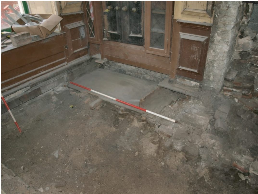
Plate 187. Llanelly House - Sir Thomas Stepney's Study (Room G2). View of timber constructed 'coin trap' positioned beneath safe at northeastern corner of room. Looking northeast.
