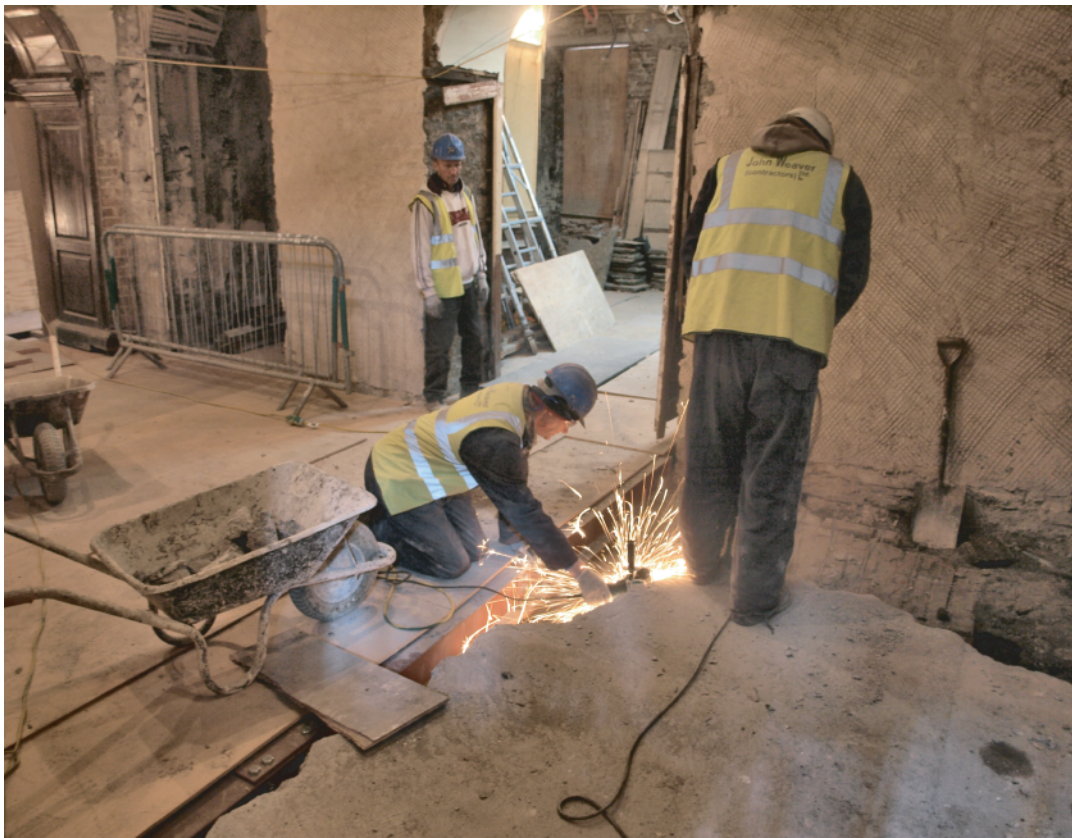
Plate 250. Working shot during concrete floor removal and red brick cellar dismantling. Looking northwards.
