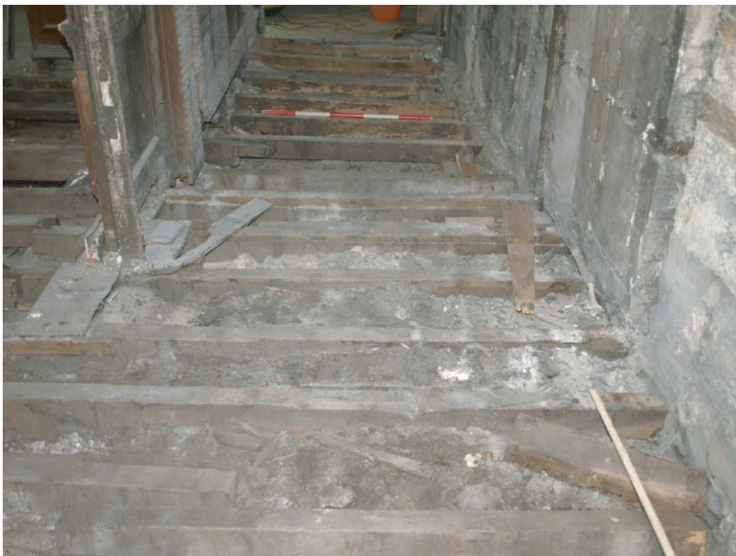
Plate 183. Llanelly House - Sir Thomas Stepney's Study (Room G2). View of exposed timber floor joists along passage at west end of Room G2 that allows access to Service Hall. Looking south
