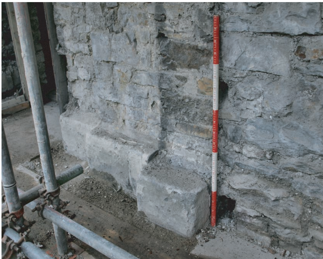
Plate 32. Llanelly House - Detail shot showing position of former central doorway in ground floor north facing elevation. and remains of former pilaster plinth. Looking southeast.
