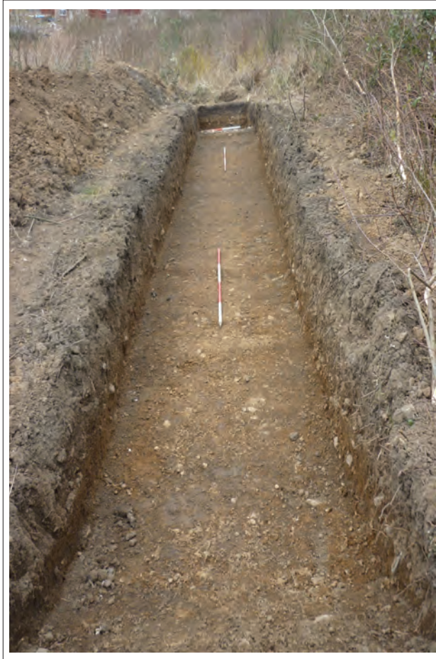
Plate 1: View north along trench 1 Scales 2x2m & 1x1m
