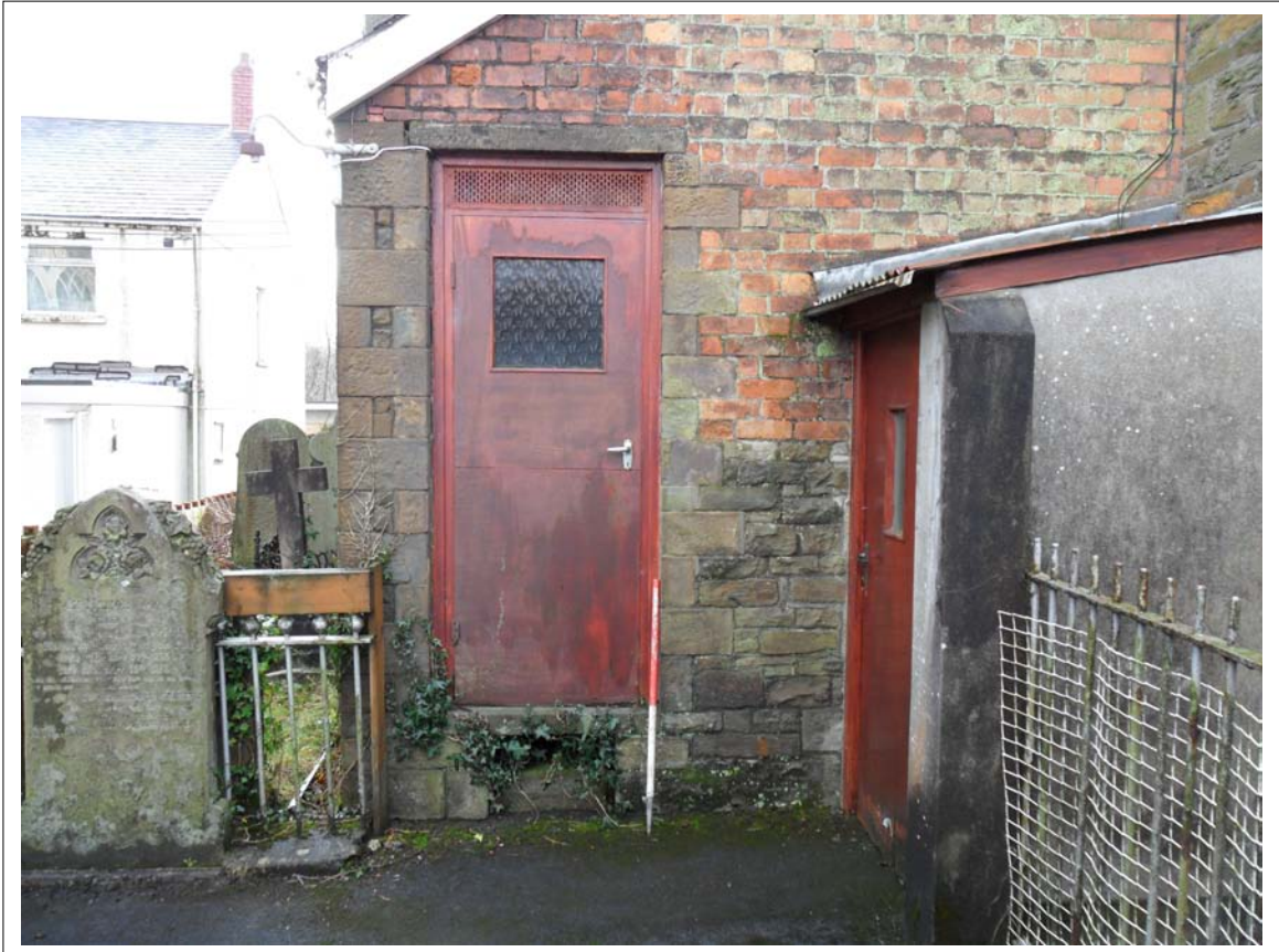
Plate 41:View of door leading from outside to upper level Organ Pit
