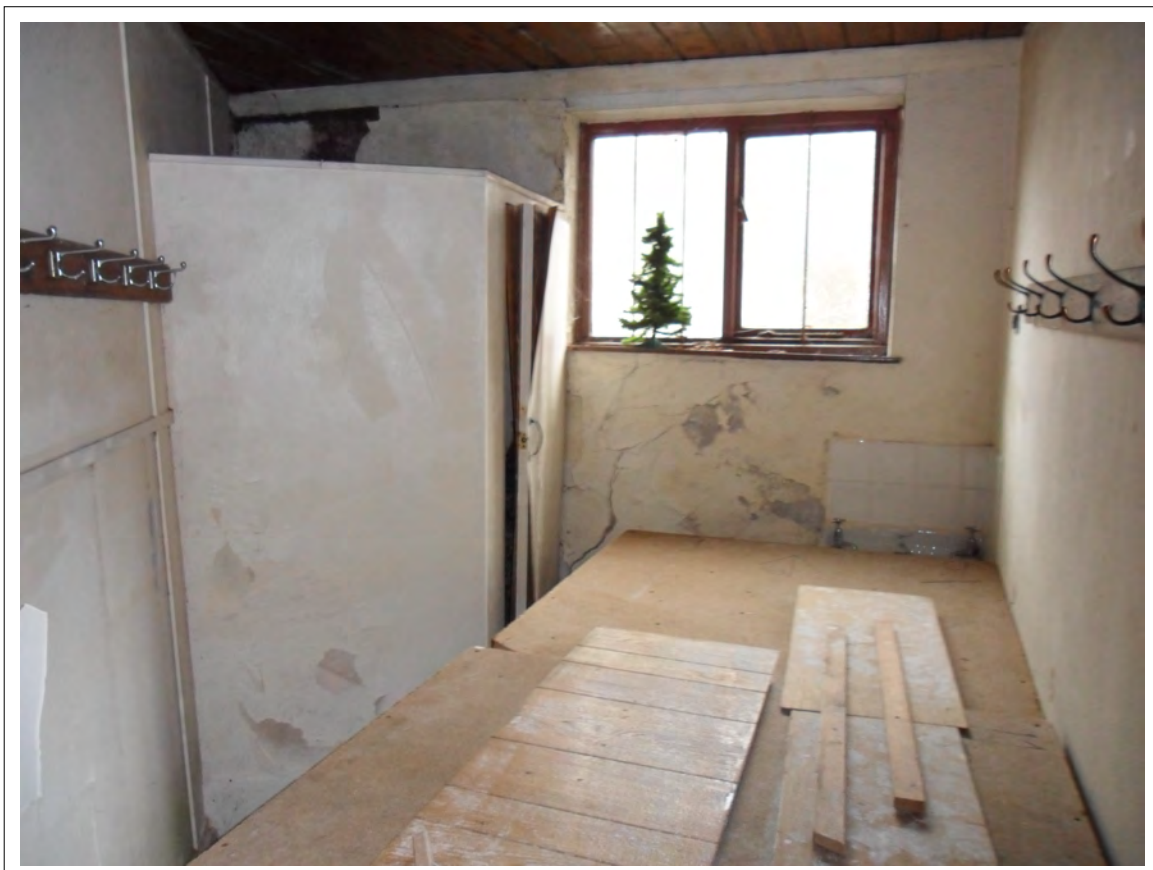
Plate 22:View of Bathroom at far NW end of Chapel
