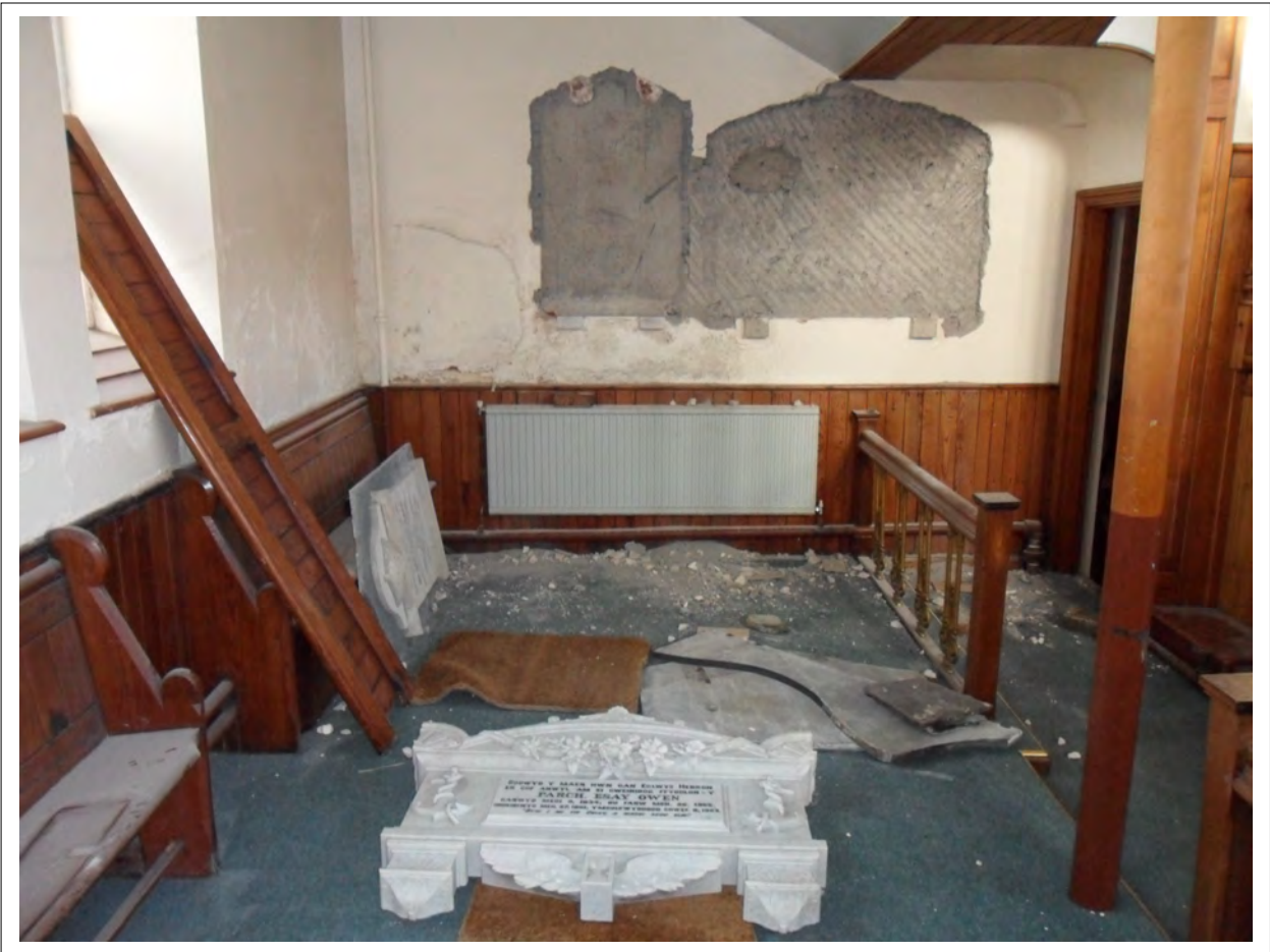
Plate 6:View of small enclosure within Chapel during memorial removal
