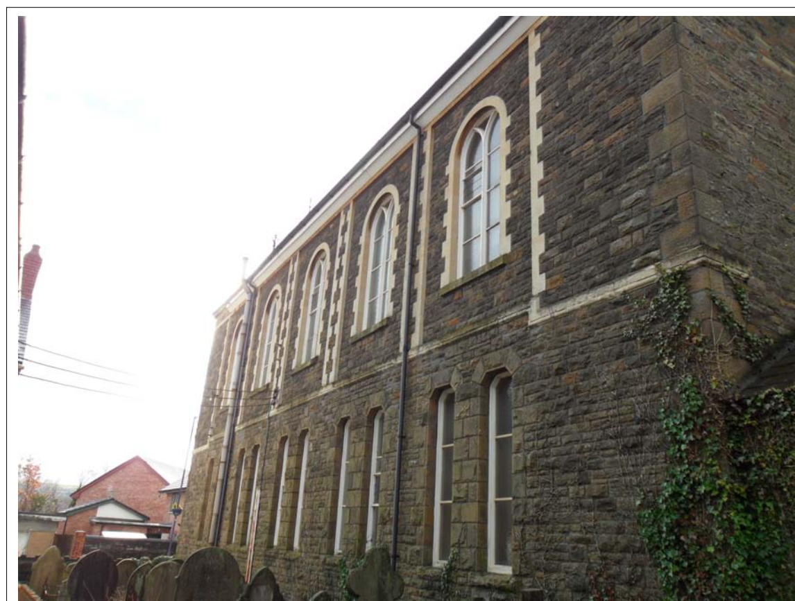
Plate 48: View of eastern elevation of Chapel
