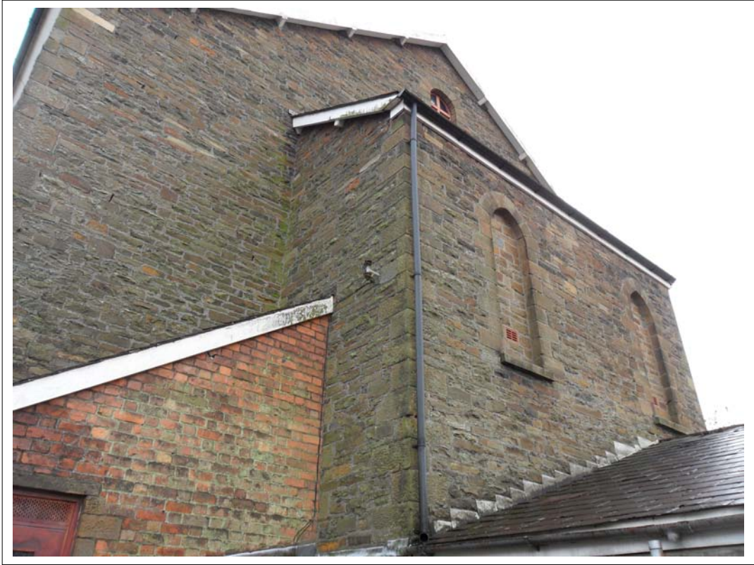
Plate 43:View of rear of Chapel
