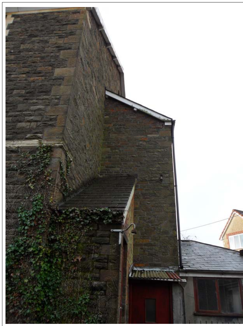
Plate 46: View of building additions at NW end
