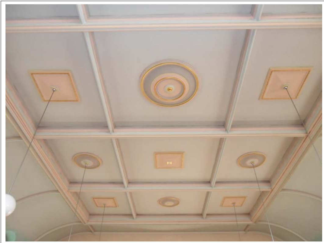
Plate 56: View of Ceiling detail
