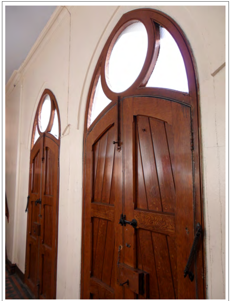
Plate 30: View of rear of main entrance doors
