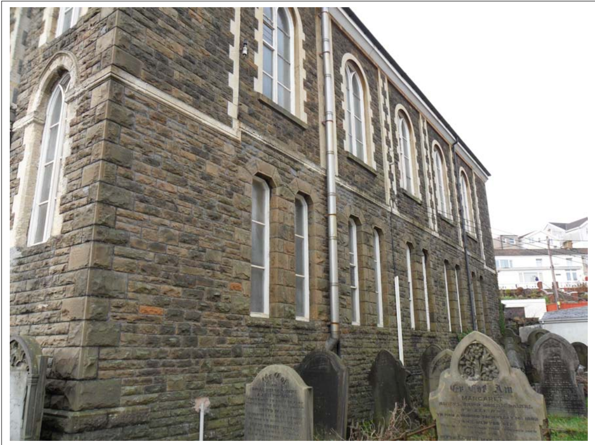
Plate 49: View of eastern elevation of Chapel
