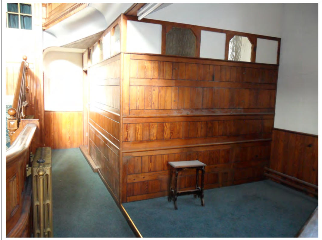
Plate 15: View of small office enclosure in north east corner
