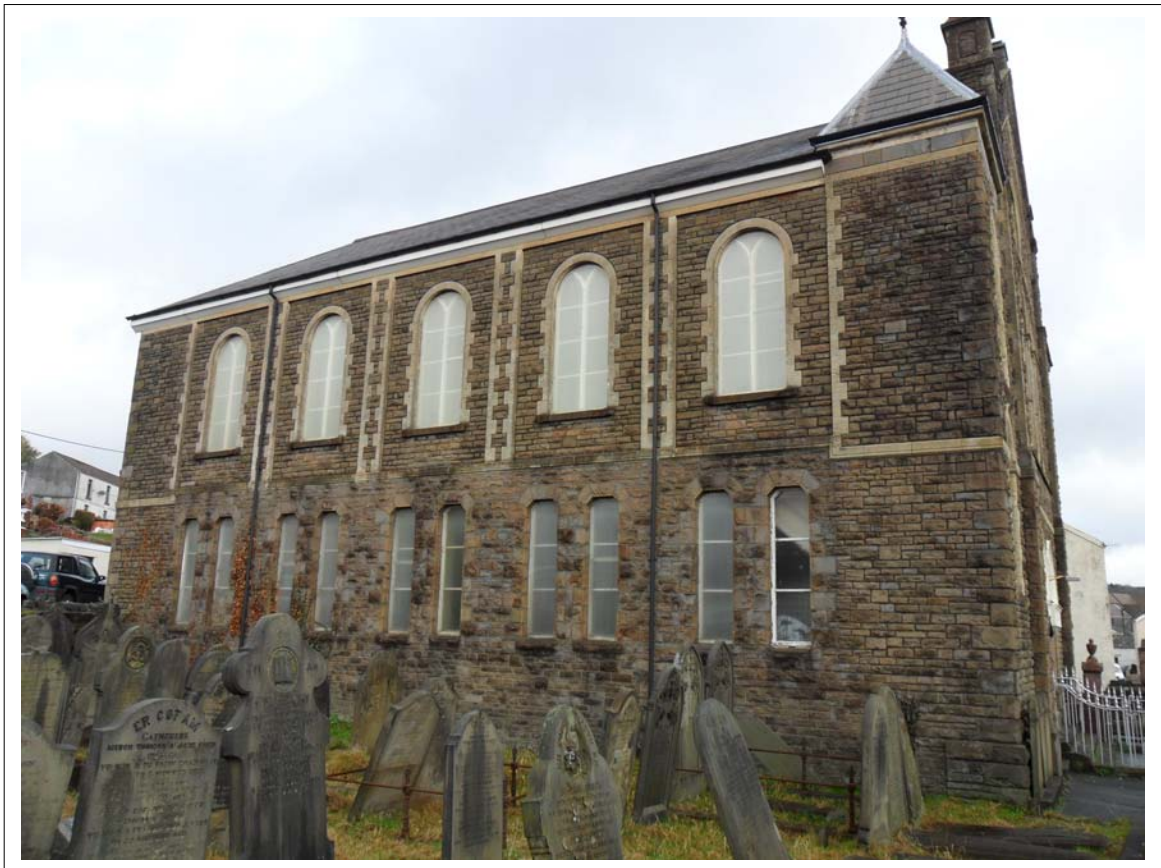
Plate 51: Western elevation of Chapel
