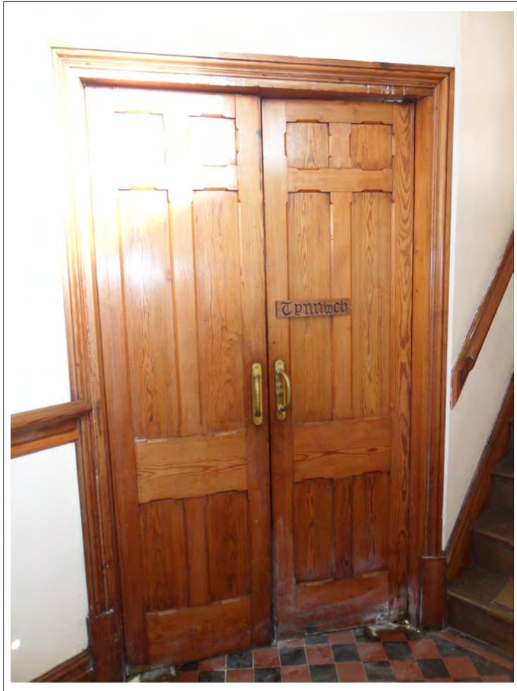
Plate 29: View of internal doorway from reception to rear of Chapel
