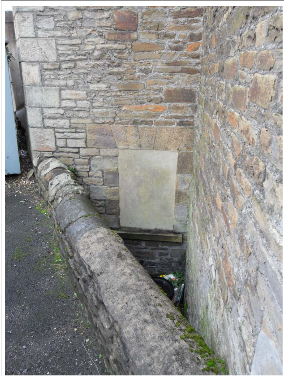
Plate 53: View of small blocked window in rear of Chapel
