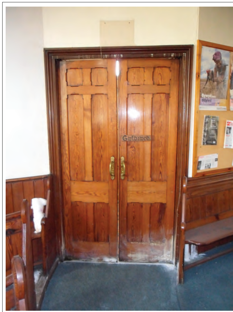
Plate 2: View of inner face of internal door
