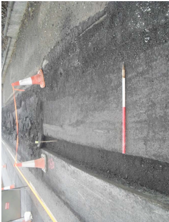
Photo 23. Section 6. Detail of pecked road surface, in advance of laying of new path surface. 1m scale. Facing North East.
