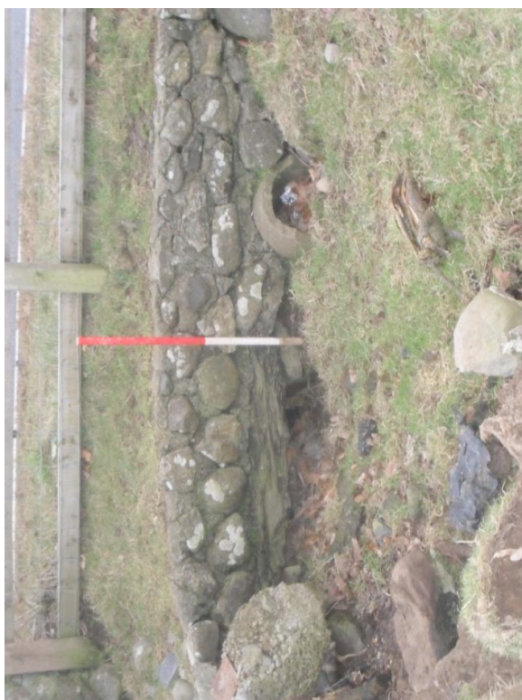
Photo 27. Section 7/8. 19 th century culvert carrying stream under present modern road. 1m scale, Facing North West.
