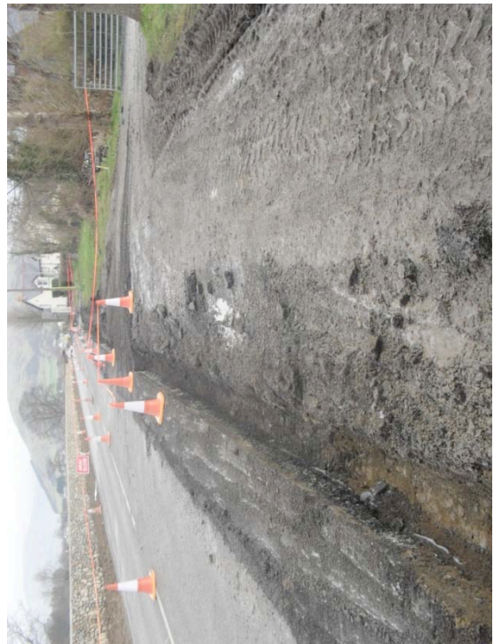
Photo 20. Section 5. Post excavation shot showing underlying and pre-existing hardcore. Facing North East.
