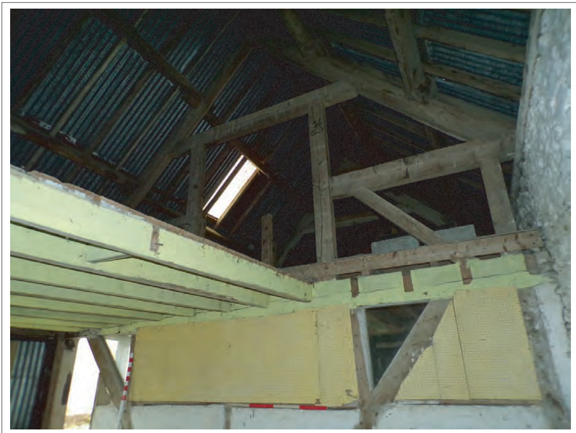
Plate 75: View south east of upper timbers of westernmost partition within 1870s extension, Scale 2x1m
