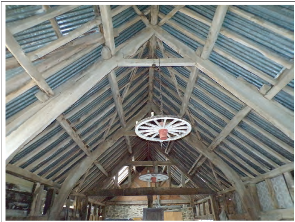
Plate 42: View of roofing detail, looking west
