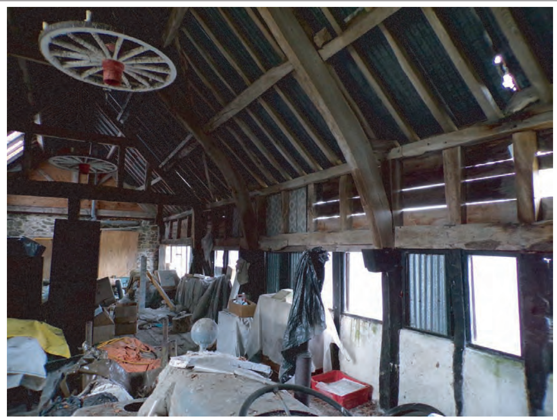
Plate 44: Oblique view looking north east along internal face of northern elevation
