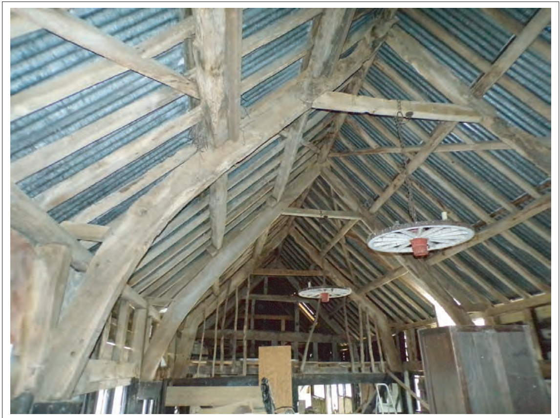
Plate 40: View of upper crucks on northern half of structure. Note deeply elbowed cruck in background above partition. Looking west
