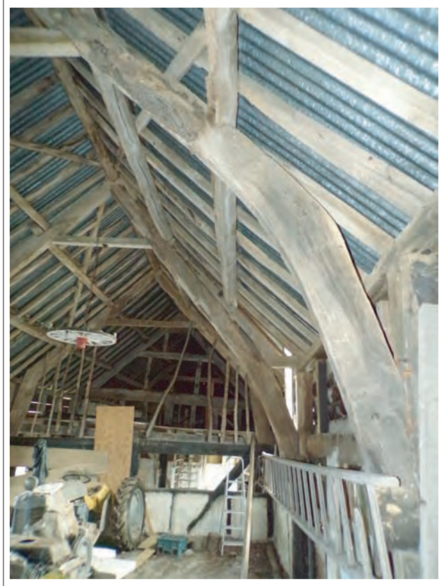
Plate 41: View east of crucks on southern half of structure
