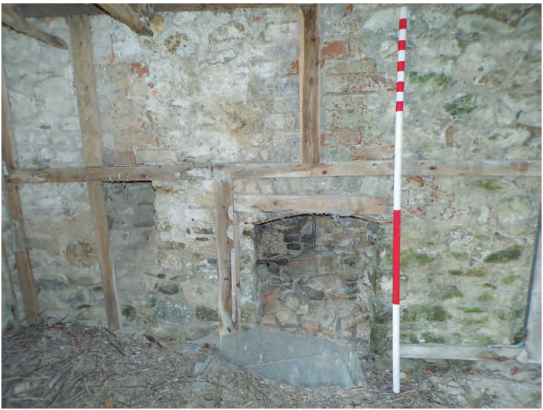
Plate 68: View of later inserted fireplace within eastern end wall, Scale 1x2m
