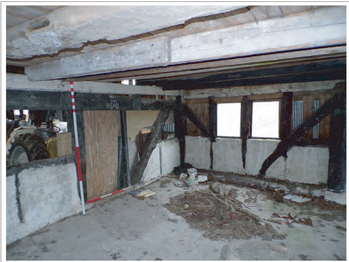
Plate 52: Oblique view north west of surviving 1772 partition forming easternmost of four bays. Scales 1x1m & 1x2m
