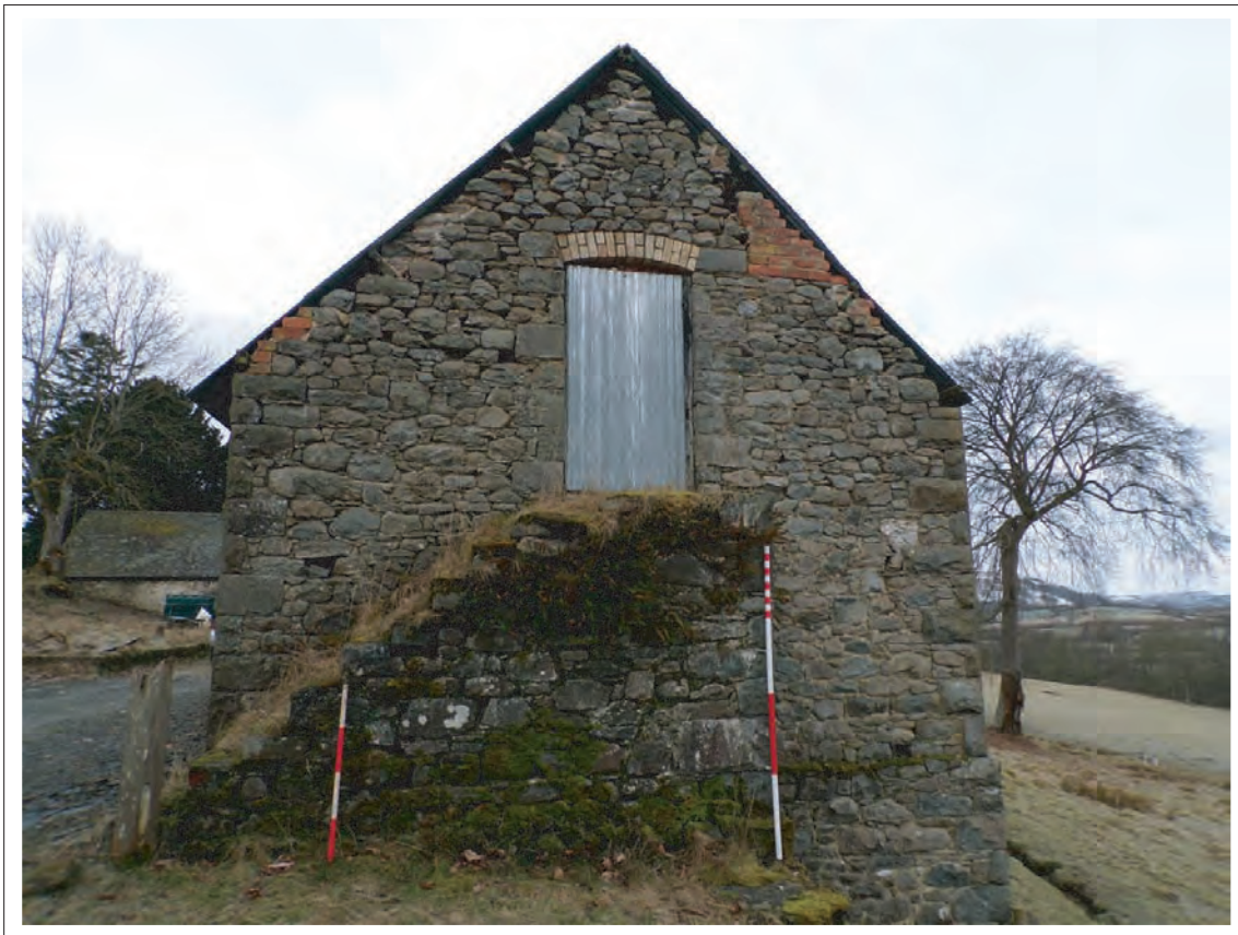
Plate 1: View of eastern elevation of structure, looking west Scales 1x1m & 1x2m
