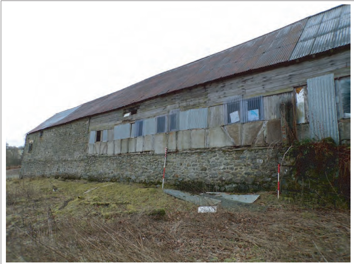
Plate 17: View south east showing 1772 structure to right butted by 1870s extension on left of shot. Scales 1x1m & 1x2m
