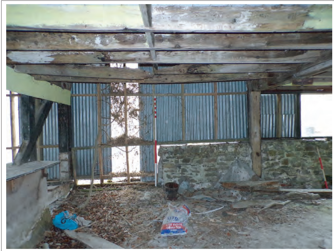
Plate 65: View of modern corrugated sheeting covering former open area within southern elevation of 1870s extension. Looking south, Scales 1x1m & 1x2m
