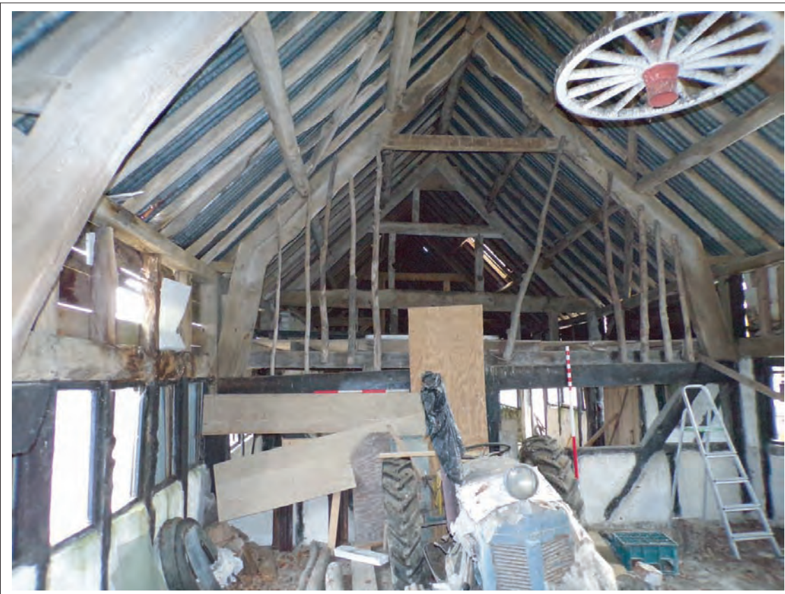
Plate 48: View of deeply elbowed cruck above only surviving 18th century partition at eastern end of 1772 structure. Looking east, Scales 1x1m & 1x2m
