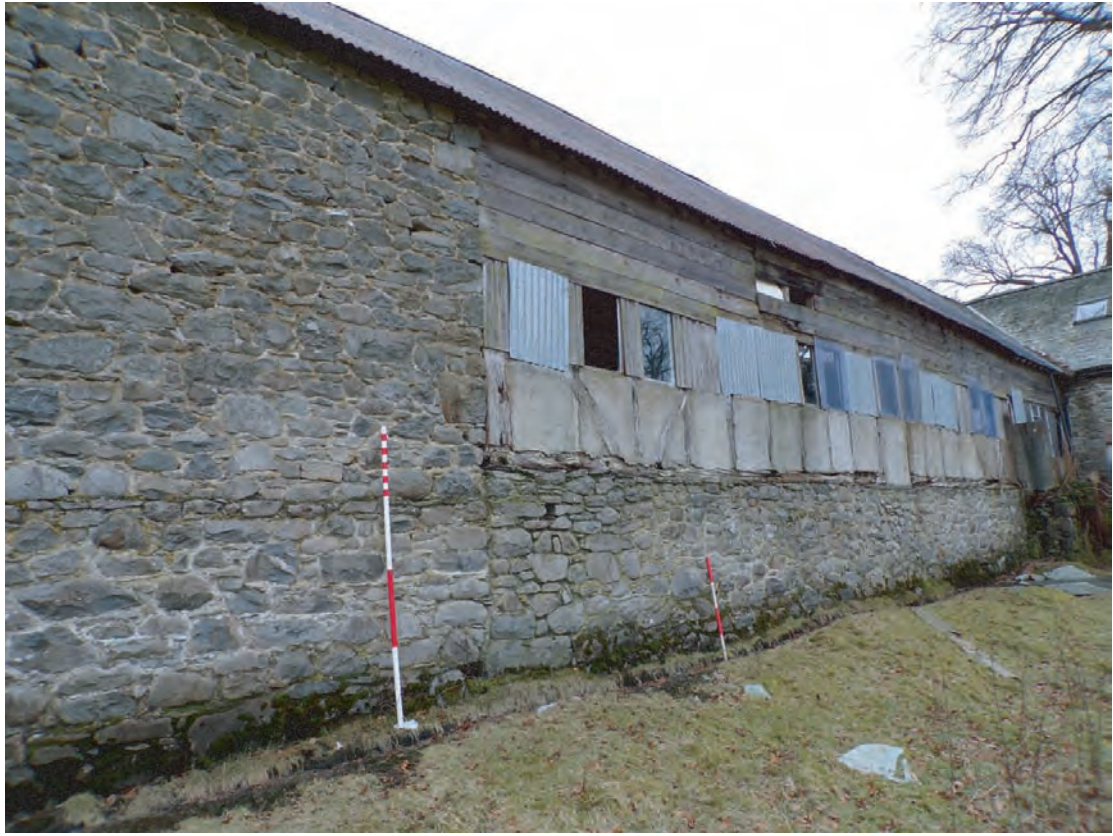
Plate 23: View of butt joint in southern elevation Looking south west, Scales 1x1m & 1x2m
