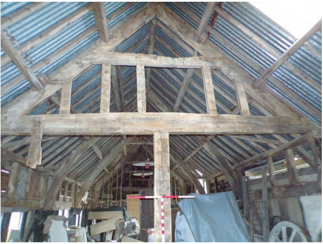
Plate 35: View of upper box frame gable end at western end of 1772 cowhouse Scales 2x1m
