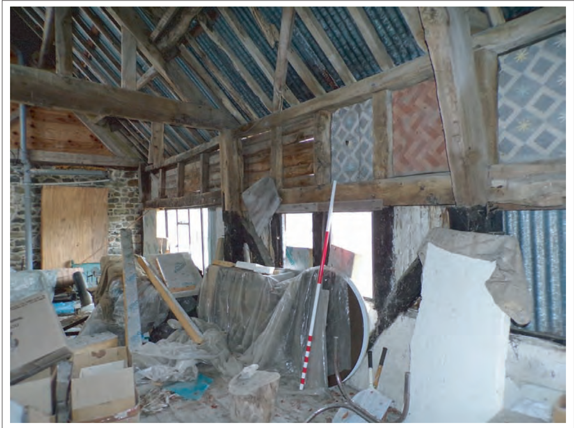
Plate 39: View west along internal face of northern elevation Scale 1x2m
