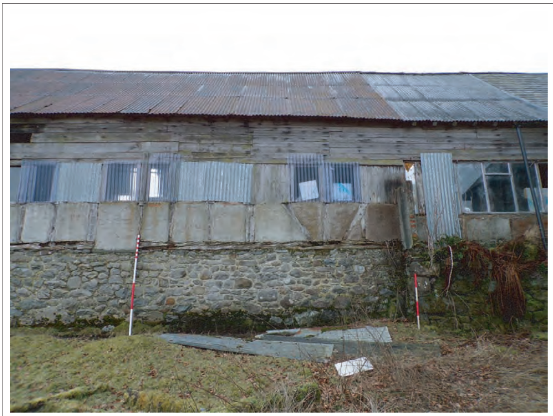
Plate 16: View of 1772 timber frame sat on stone platform (centre) with 1870s stone platform to right. Looking south, Scales 1x1m & 1x2m
