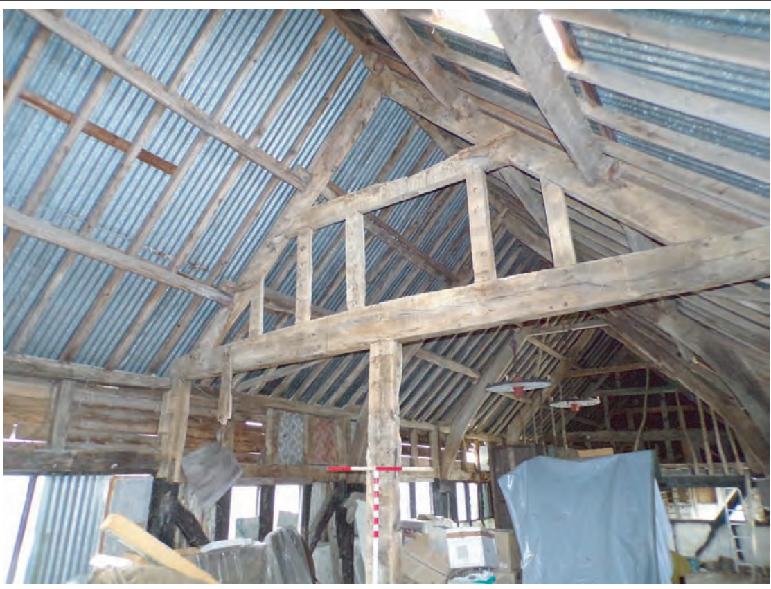
Plate 36: Oblique view north east of surviving timbers of 1772 western gable end Scales 2x1m
