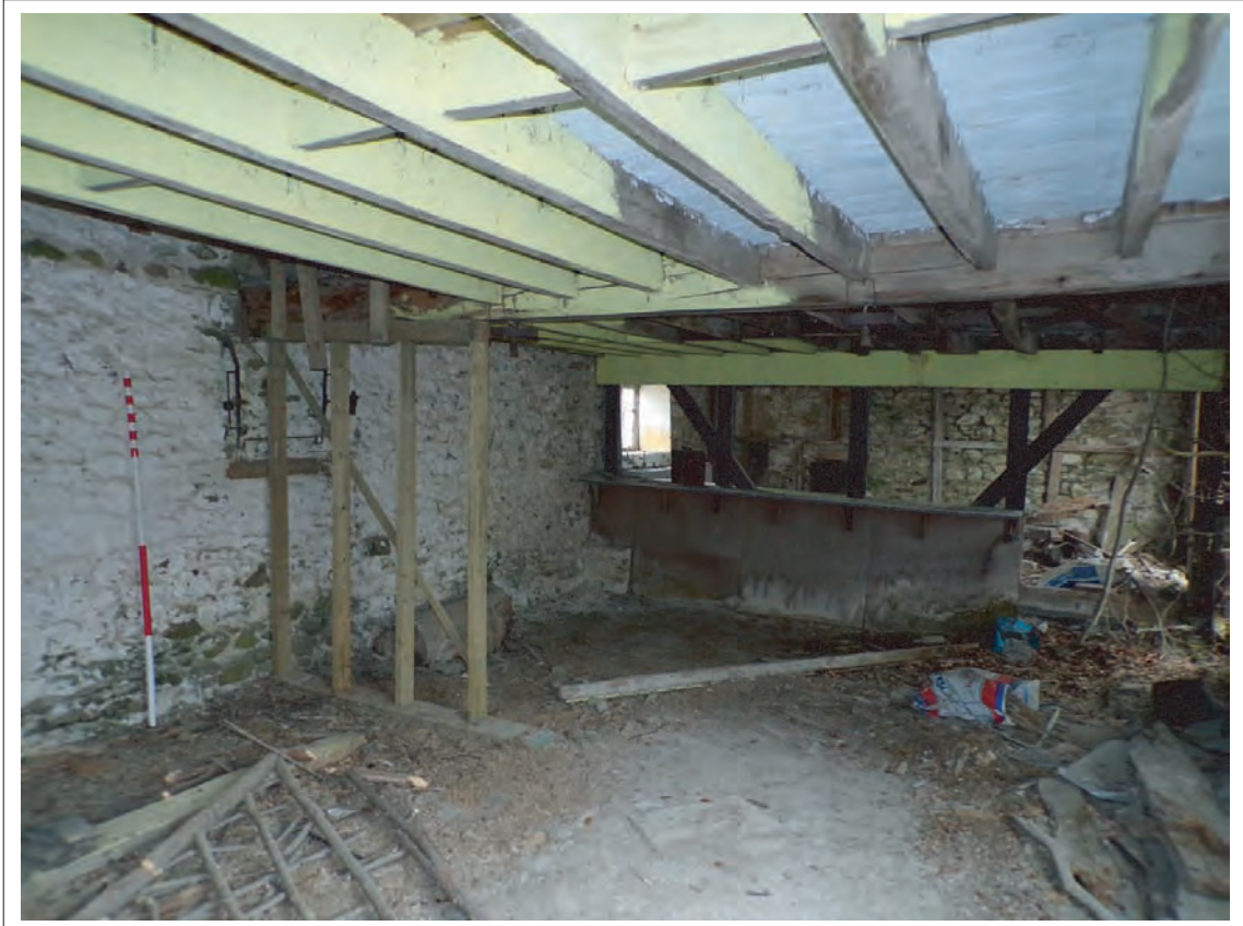
Plate 63: View north east of removed partition within 1870s extension now propped with modern supports. Scale 1x2m
