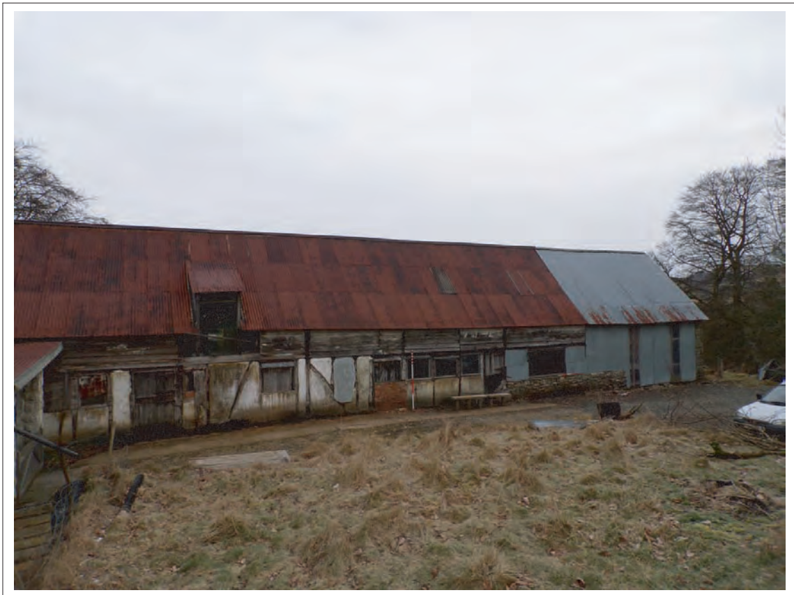
Plate 29: View north east of northern elevation. Scales 1x1m & 1x2m
