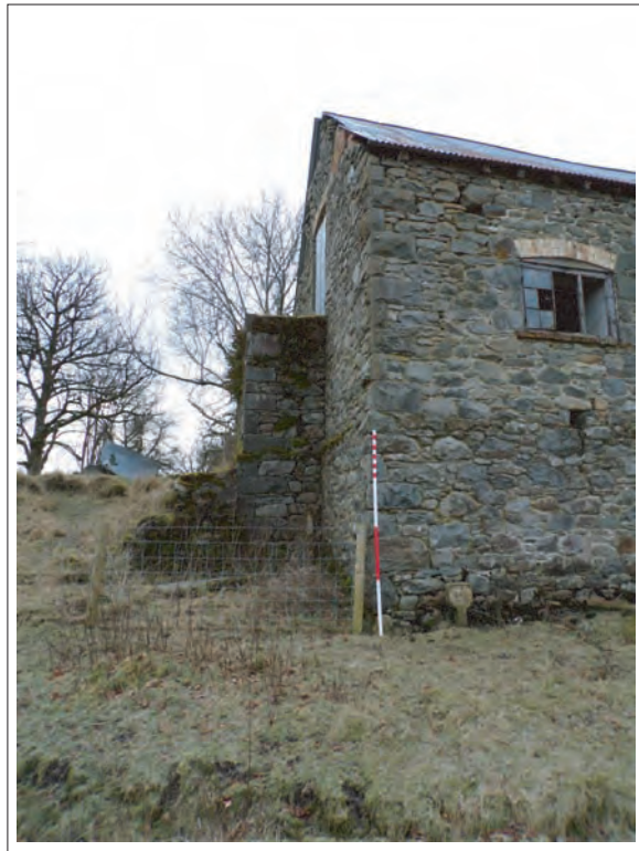
Plate 26: View of upper level access stairs butting eastern elevation of 1870s extension Looking south, Scale 1x2m
