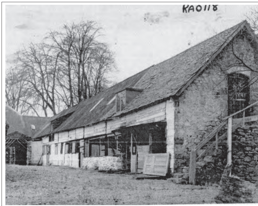
Plate 80: RCAHMW 1973 photo along southern elevation
