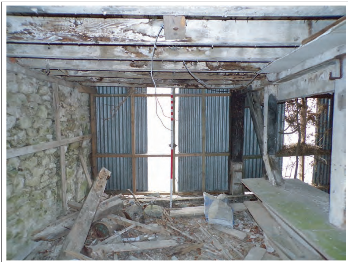
Plate 66: View of modern corrugated sheeting covering former open area within southern elevation of 1870s extension. Looking south, Scale 1x2m
