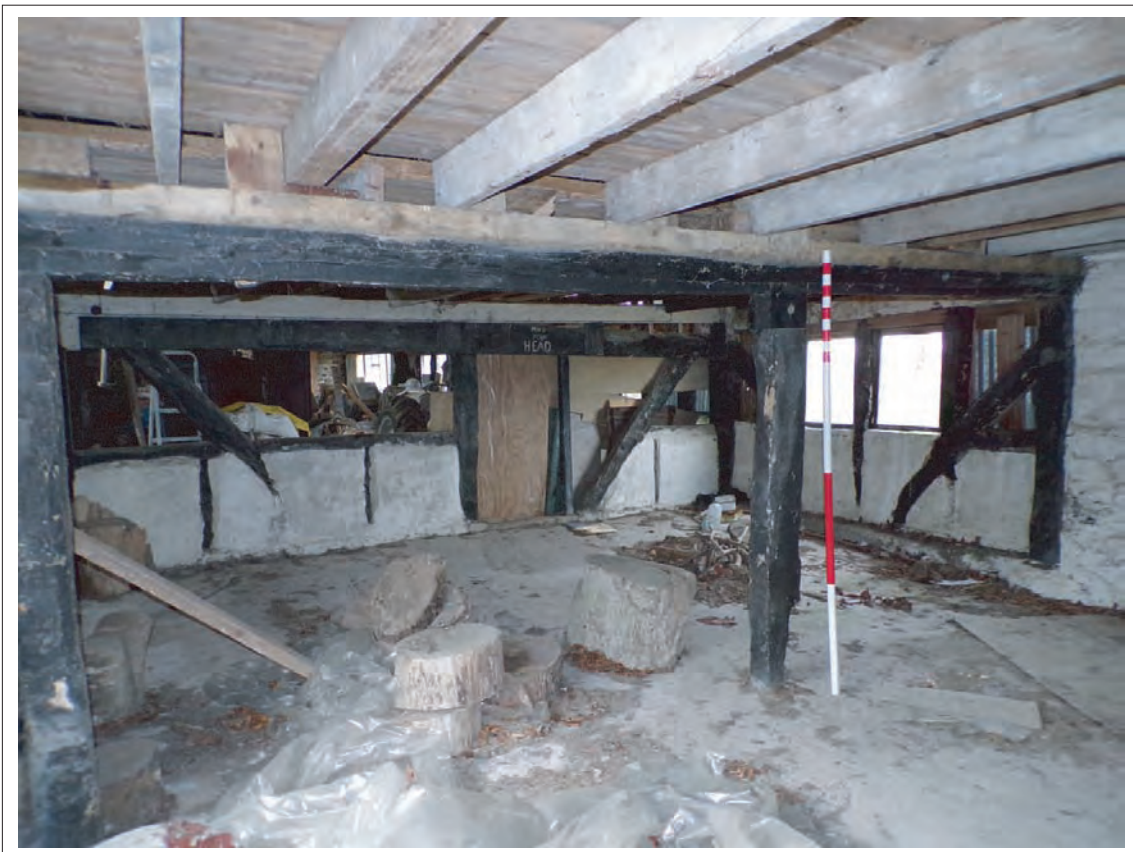
Plate 58: View of lower portion of easternbox framed gable end of 1772 structure against which 1870s extension is butted. Looking north west, Scale 1x2m
