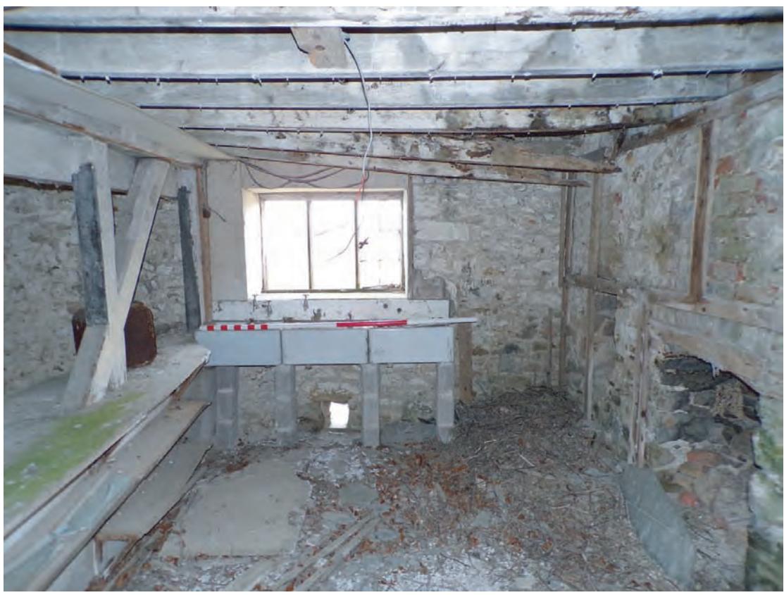
Plate 67: View north within eastern end of 1870s extension, Scale 1x2m
