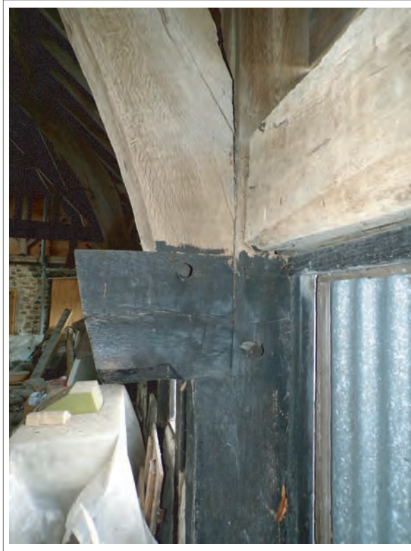
Plate 77: View of upper cruck sat on stub of removed horizontal brace.
