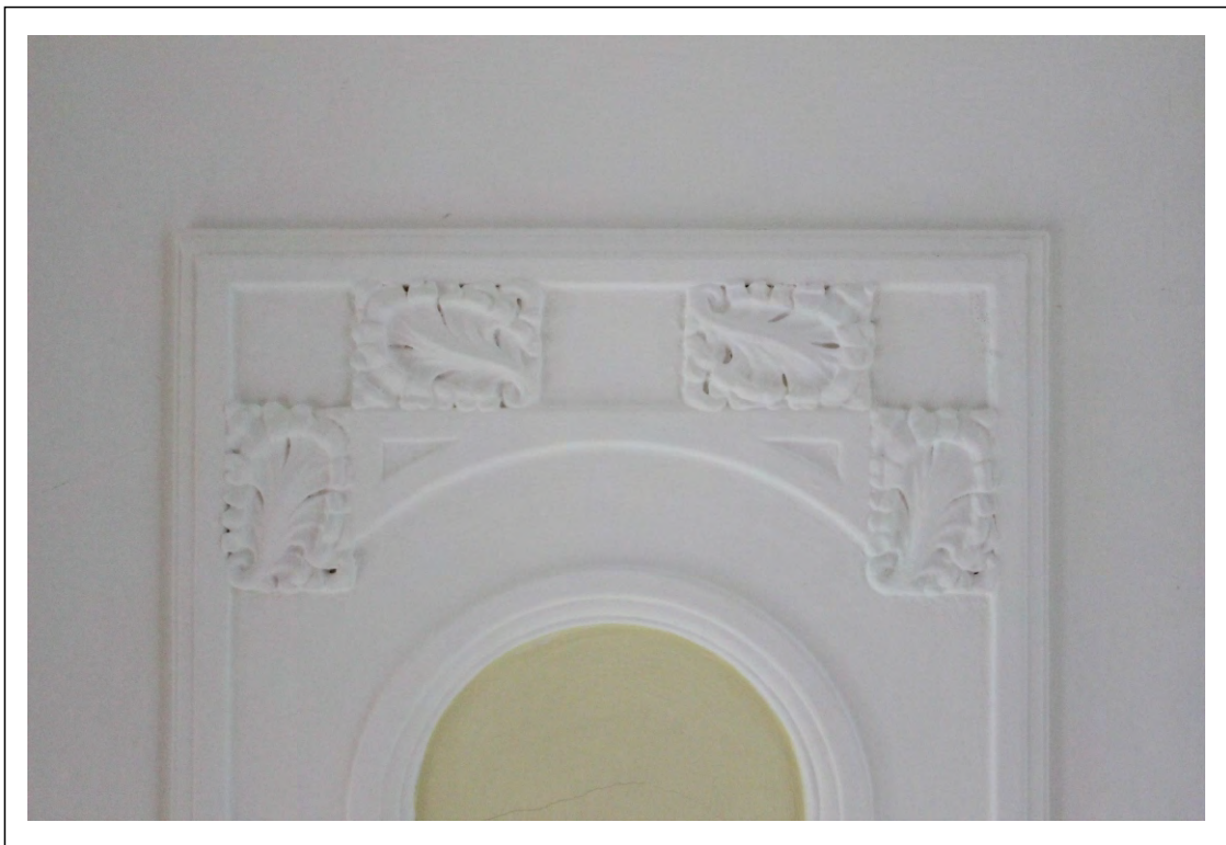
Plate 32: Close-up detail of plaster work ceiling panel borders
