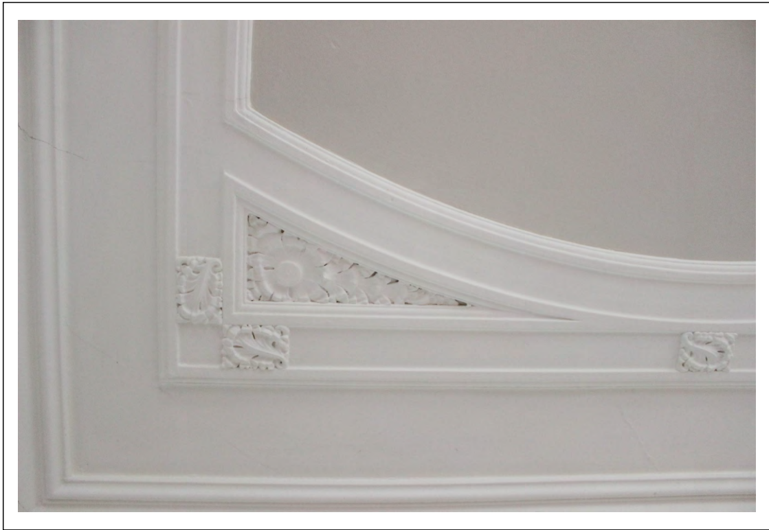
Plate 33: Close-up detail of plaster work ceiling panel borders
