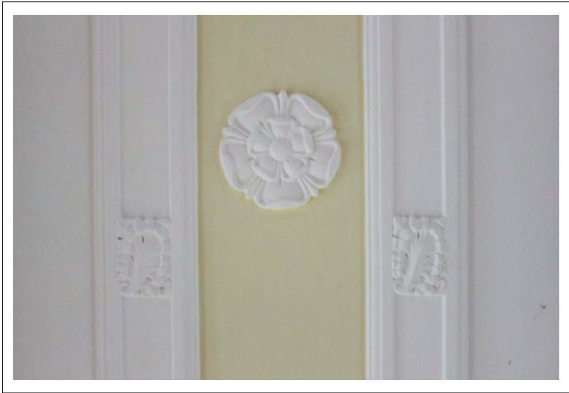
Plate 31: Close-up detail of plaster work ceiling panel Tudor rosettes
