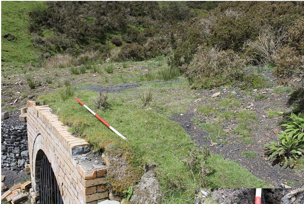
a. Location of the investigation trench
