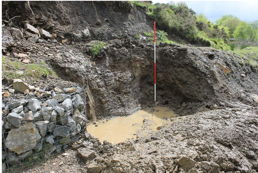
b. Gabion basket trench, post-excitation
