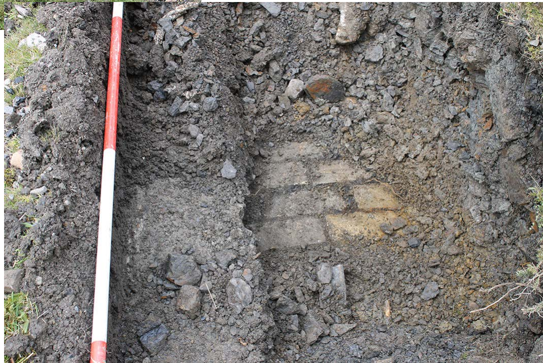
b. Original brickwork (right) and modern concrete (left)
