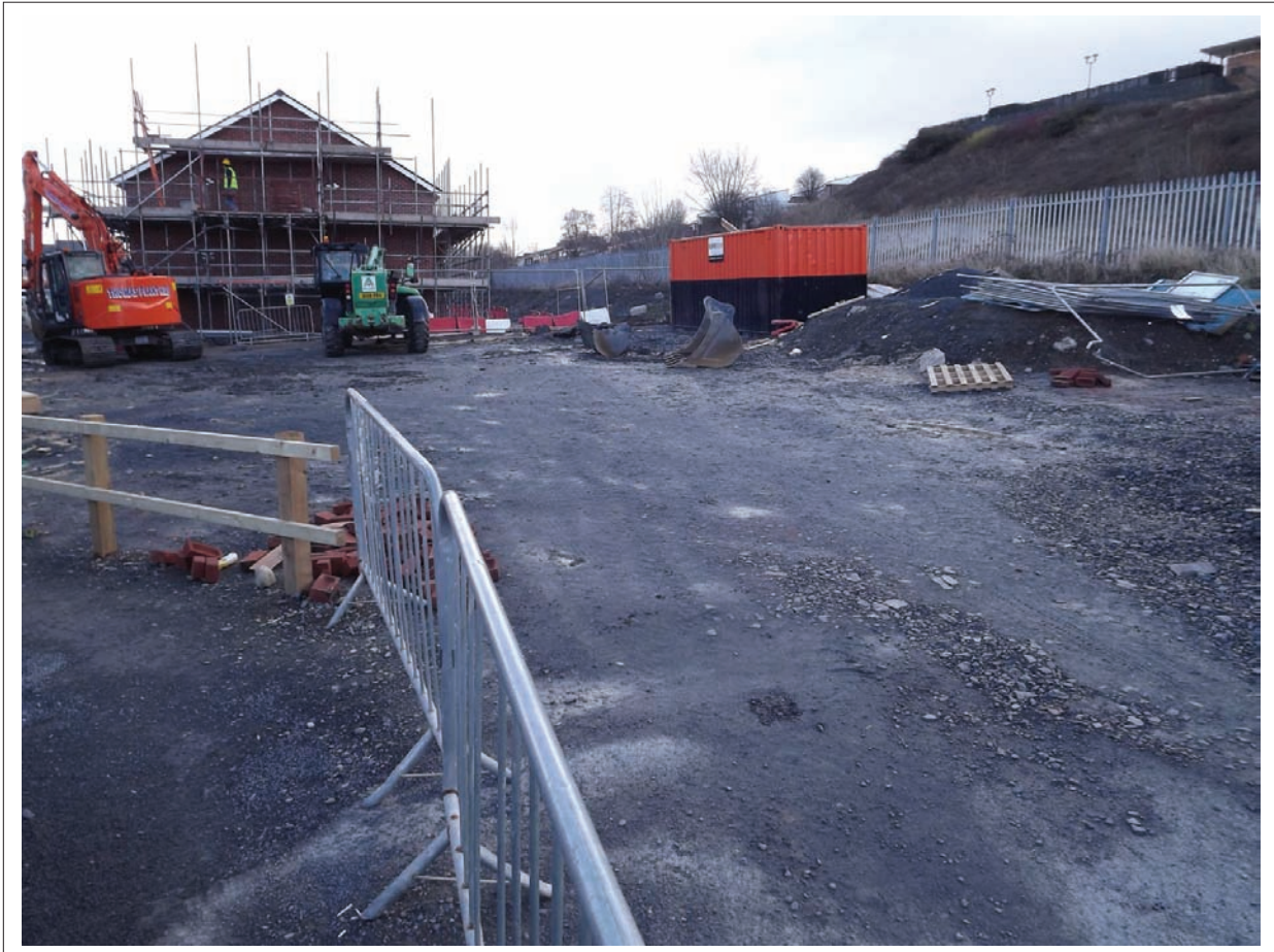
Plate 1:View of assessment area prior to reduction in ground levels looking west
