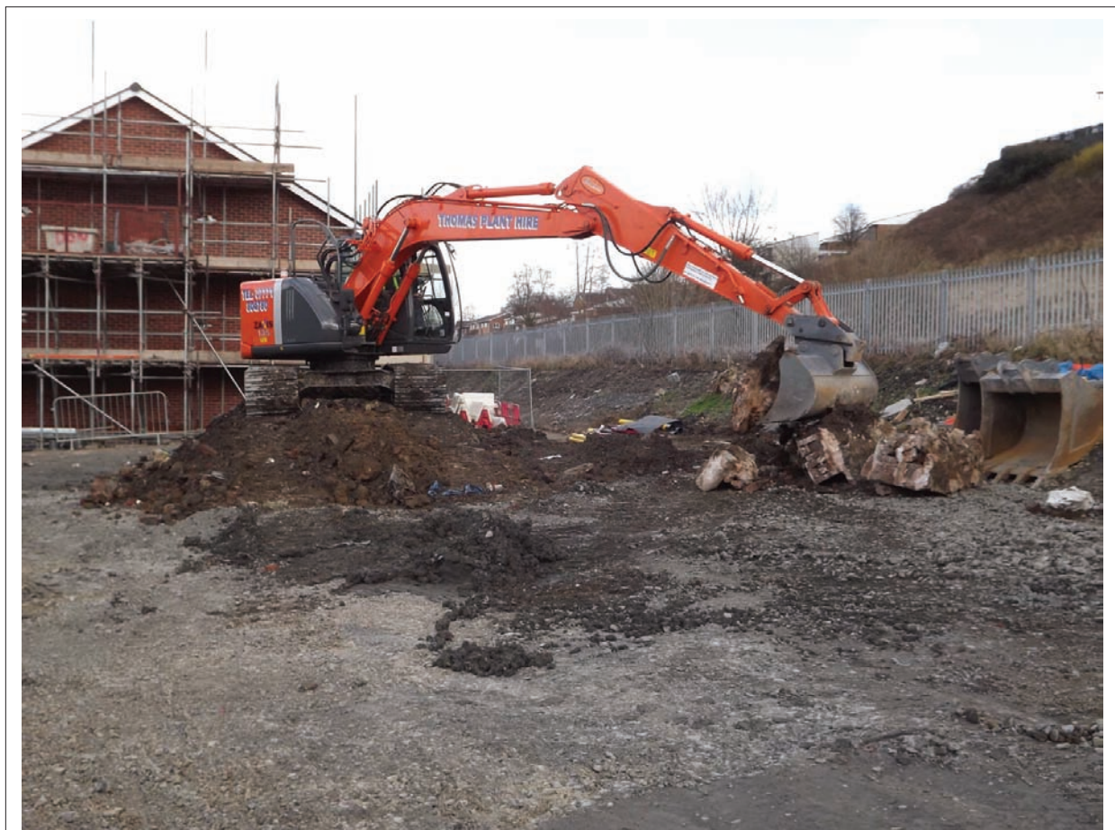
Plate 2:View of ground levelling and overburden removal underway Looking west
