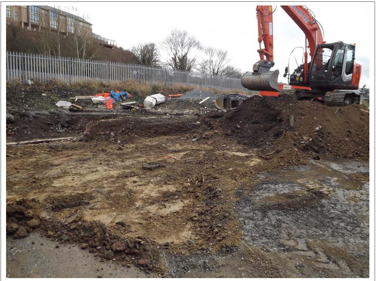
Plate 3: View of modern overburden deposit - Mid orange brown clay Looking north east
