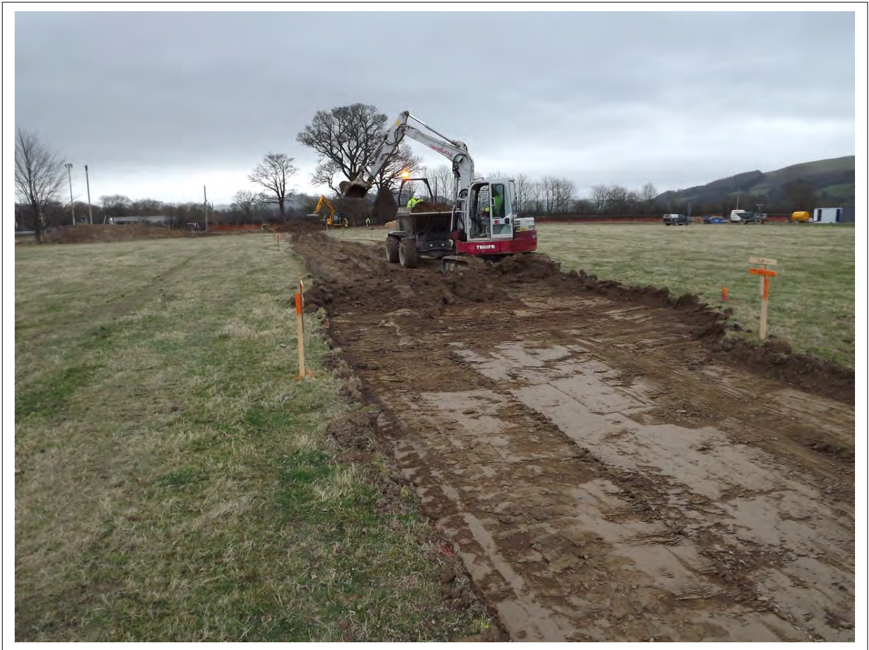
Plate 5: View of road area under excavation, looking east
