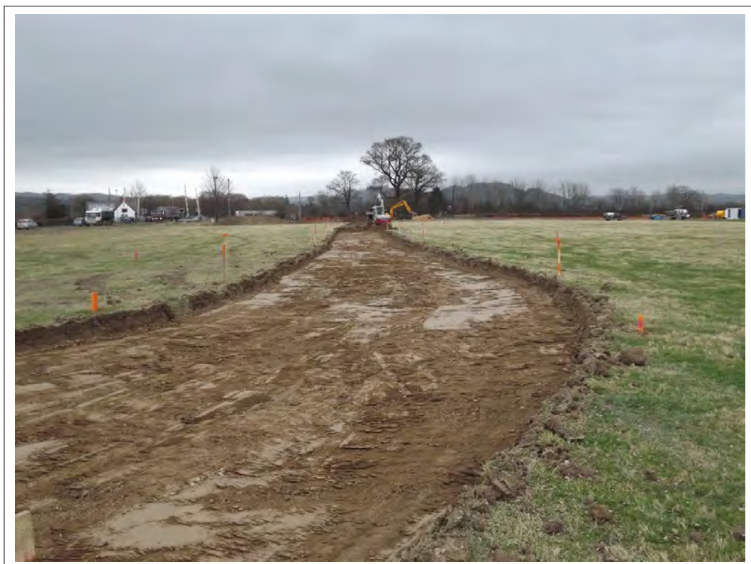
Plate 4: View across road area of watching brief, looking north east
