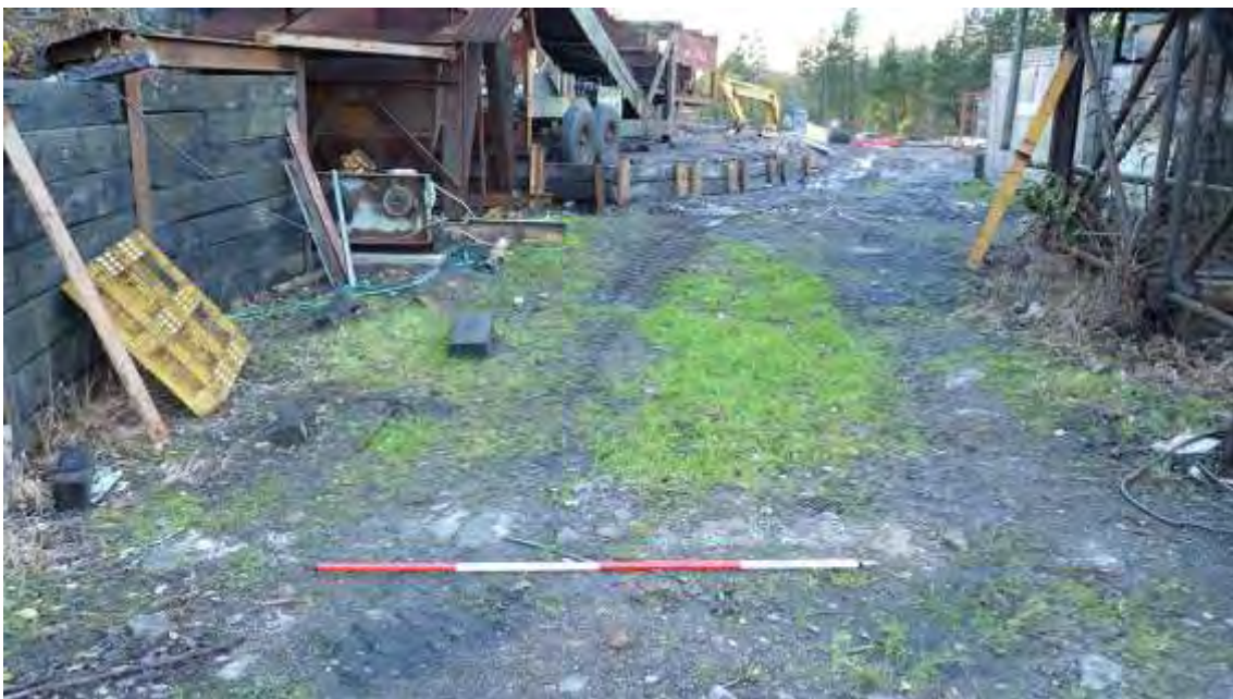
Photo 22: View WSW along the raised area that covers the site of the blast furnaces and main brickworks building. The remains of the earlier stone wall is visible just above the 2m scale.
