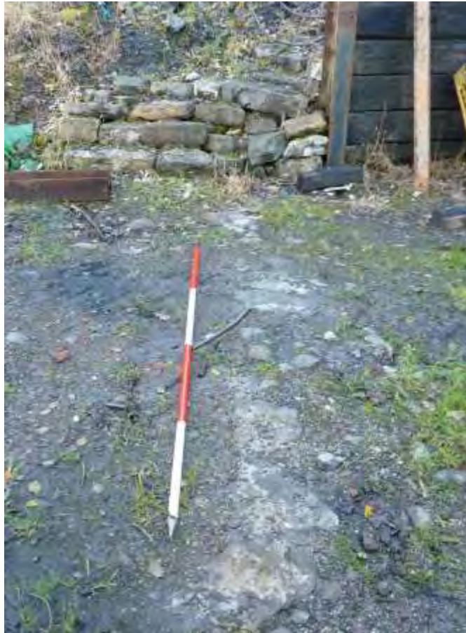
Photo 21: View SSE of the remains of an earlier mortared stone wall visible in the ground surface, to the right of the 2m scale.
