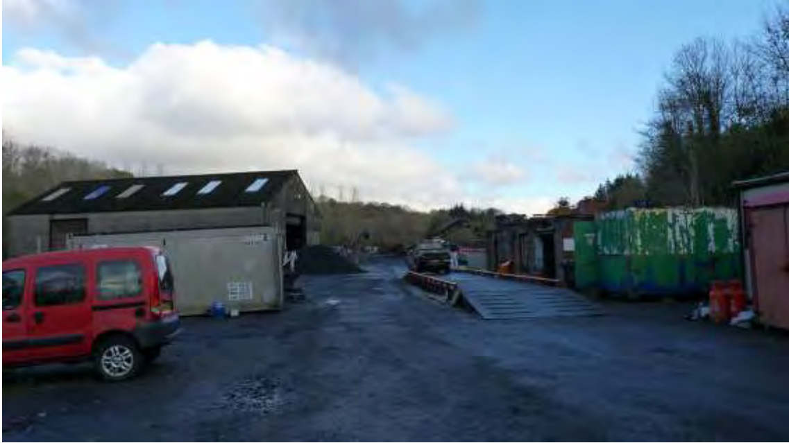
Photo 3: View NE from the main entrance to the site.
