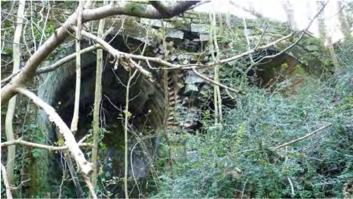
Photo 13: View SSE of the easternmost arched recesses within the wall.
