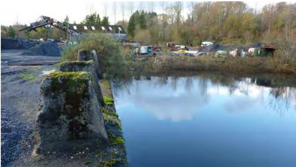
Photo 8: View W of former washery pond.
