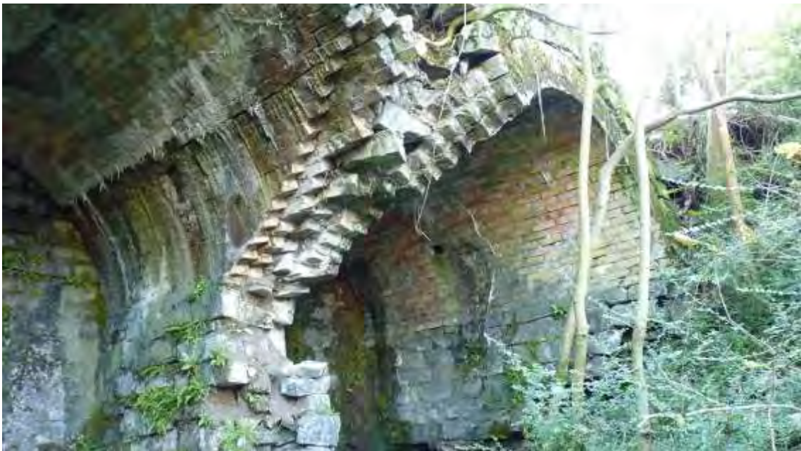
Photo 14: View SE showing more detail on the arched recesses.
