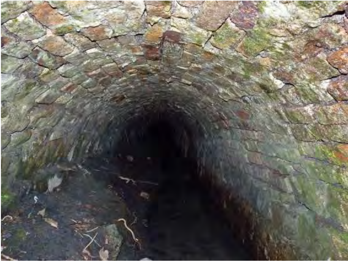
Photo 25: View SE inside the brick-arched culvert.
