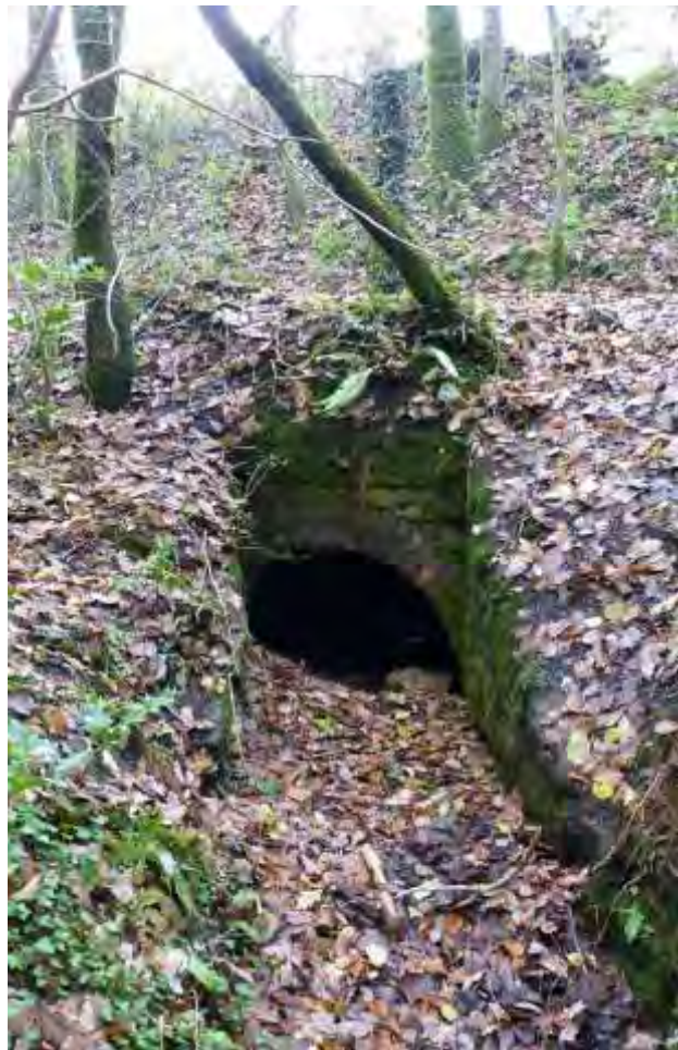
Photo 24: View SE of the brick-arched culvert surviving in the river bank outside the site boundary.
