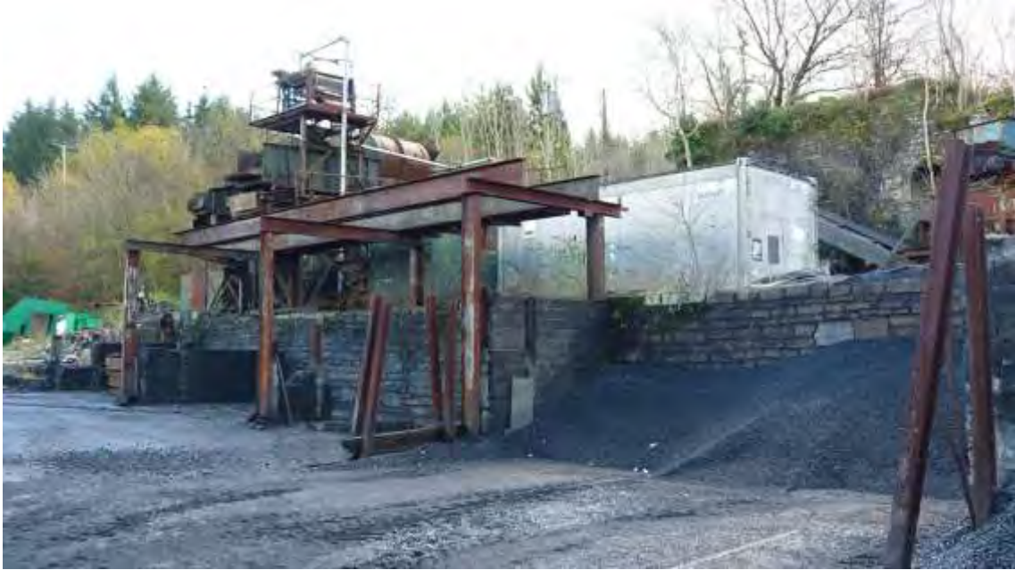
Photo 19: View SE of the mortared stone wall forming the rear of the coal-bays. This wall is thought to represent possible remains of the brickworks building.
