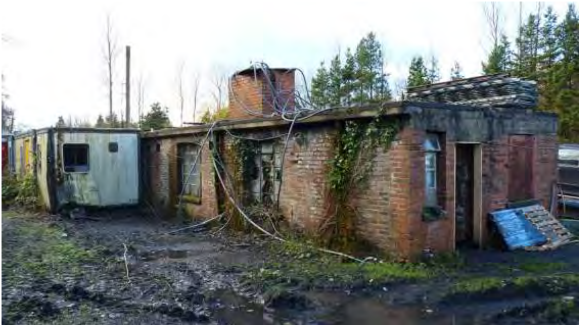
Photo 4: View NW of the brick-built building adjacent to the weighbridge.
