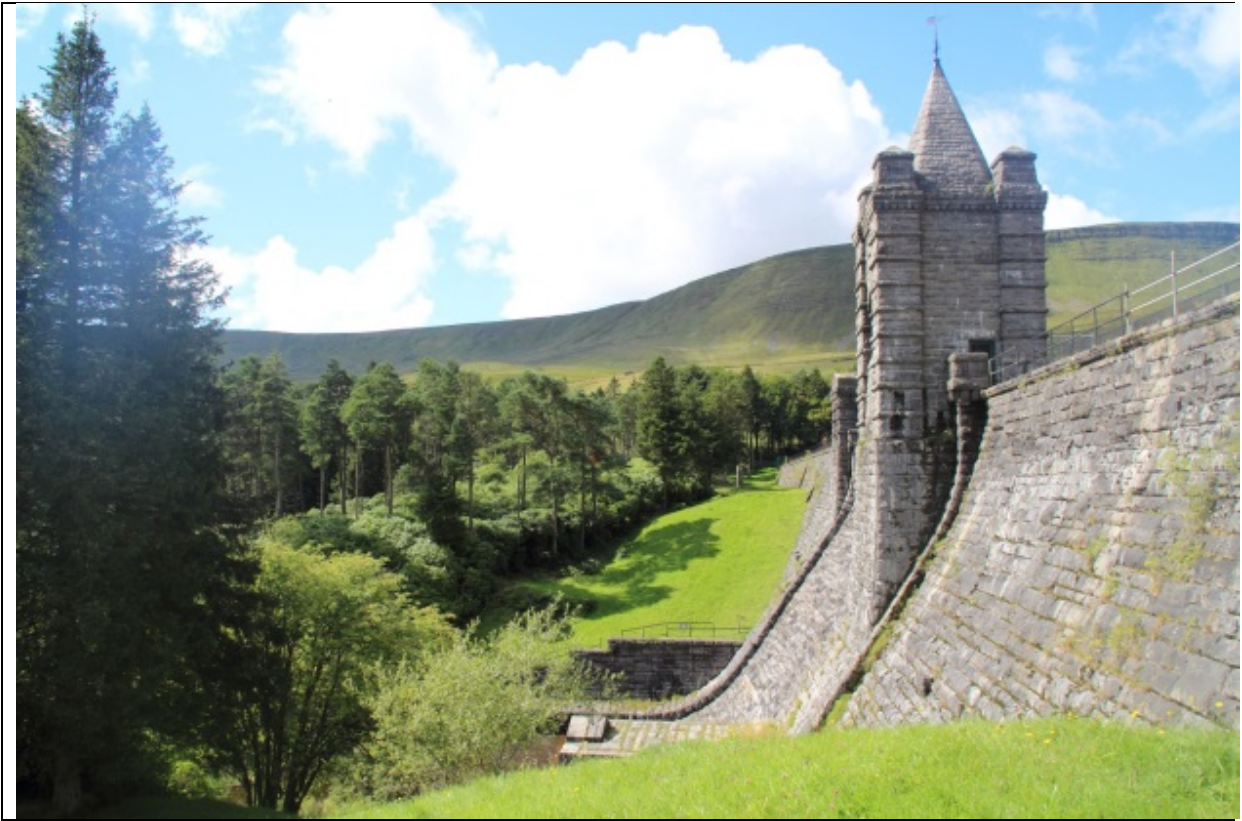
Upper Neuadd dam, looking west
