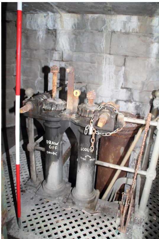
Figure 12 The north end of the tunnel showing the base of the shaft in the tower and the pipework and control gear. The tunnel is to be driven through the brick work at the far end
