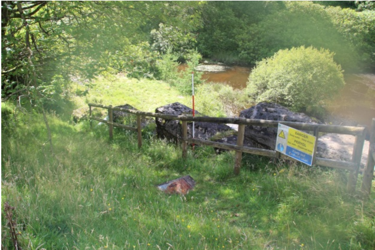
Figure 10 The top of the retaining wall and the grassy area beyond, which will be terraced, looking south-west (scale 2m)
