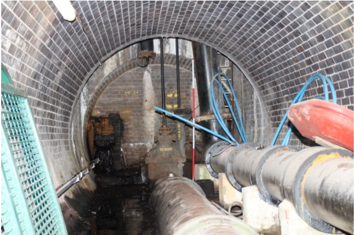
Figure 12 The north end of the tunnel showing the base of the shaft in the tower and the pipework and control gear. The tunnel is to be driven through the brick work at the far end
