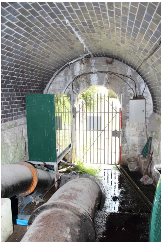
Figure 11 The south end of the tunnel just inside the entrance, looking south (scale 2m)
