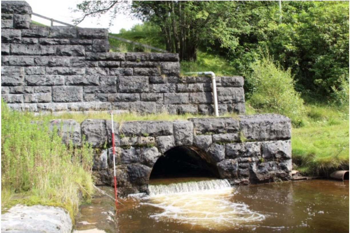
Figure 7. The eastern retaining wall from the spillway base and the lower outfall (scale 2m)
