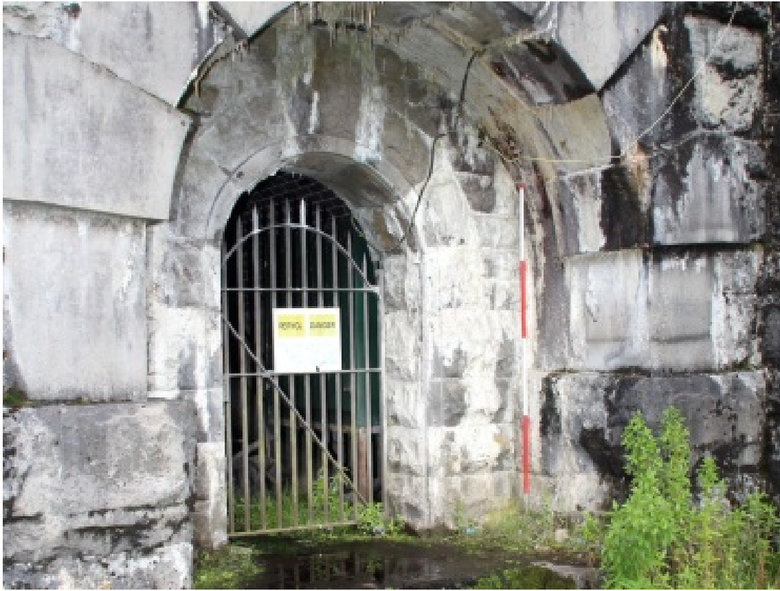
Figure 5. The treatment of the jambs of the inner doorway to the tunnel building (scale 2m)
