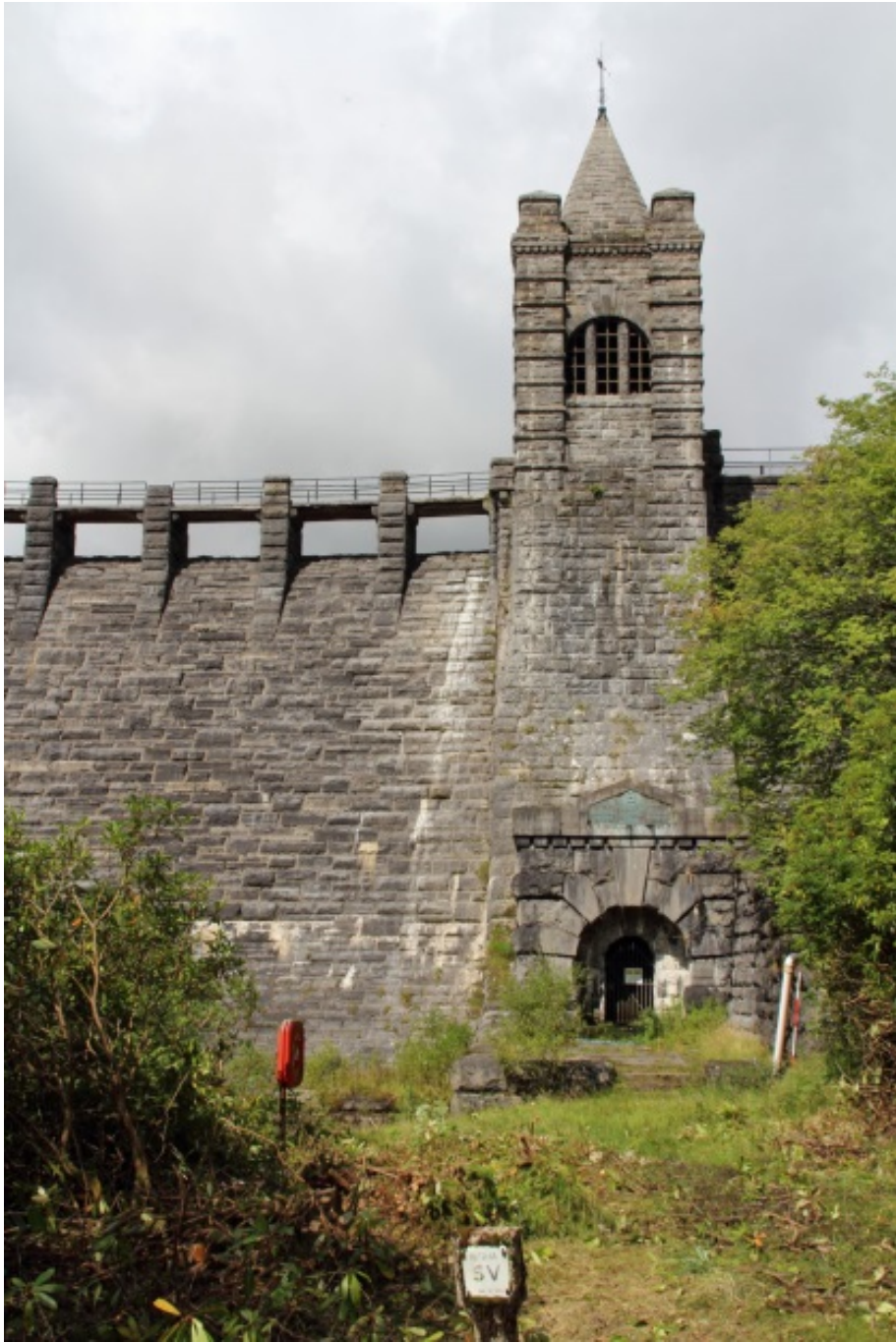
Figure 9. The grassy area to be terraced to stop erosion by the new outflow from the tunnel
