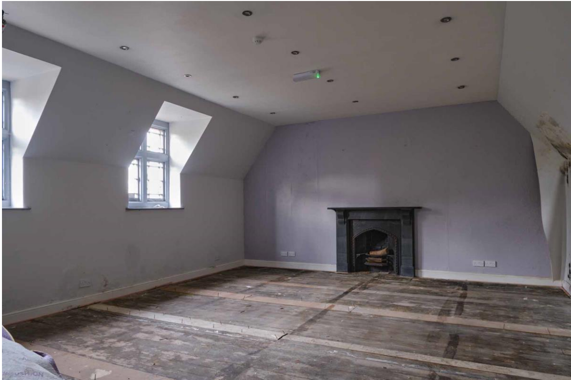
Figure 48. Attic, room 2.1, former billiards room.
