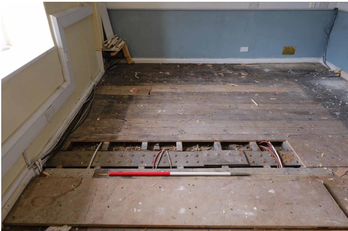
Figure 49. Composite beam in room 2.5.
