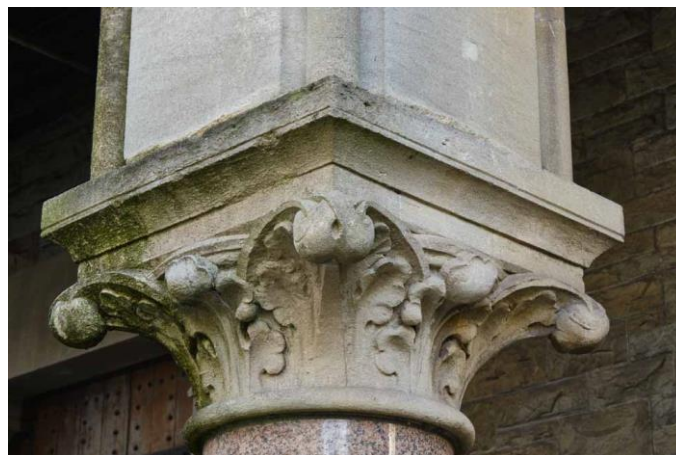
Figure 22. Capital, porch, north front
