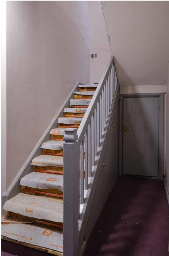
Figure 45. Dog-leg stair on first floor, inserted 1926.
