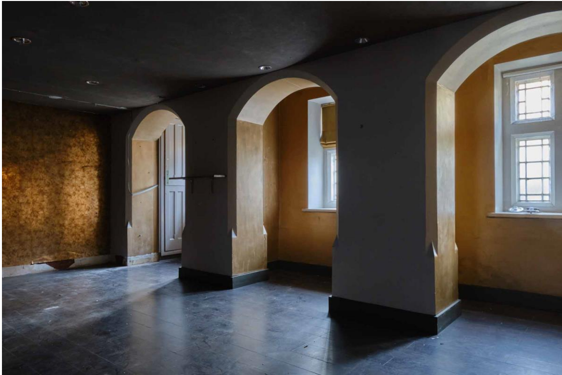
Figure 51. Arcade in basement (B1) supporting the upper floors, added after 1891.
