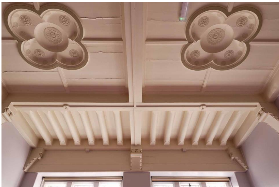
Figure 41. Dining room ceiling.
