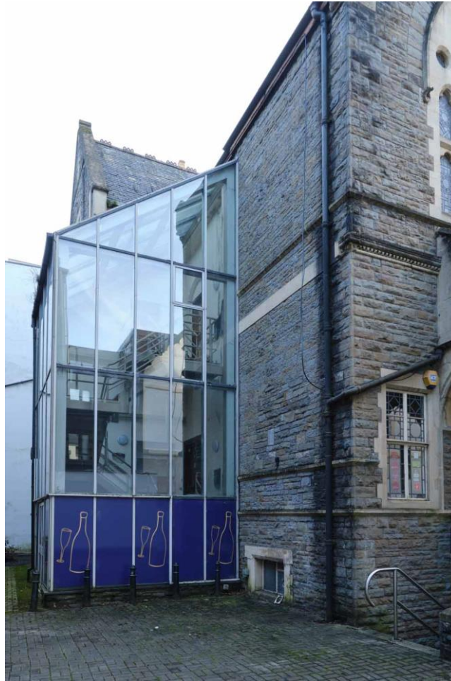
Figure 25. Escape stairs in east front.
