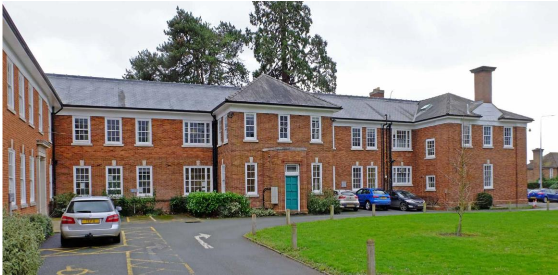
Figure 12. North-west front of entrance range (on the right) and later rear wings
