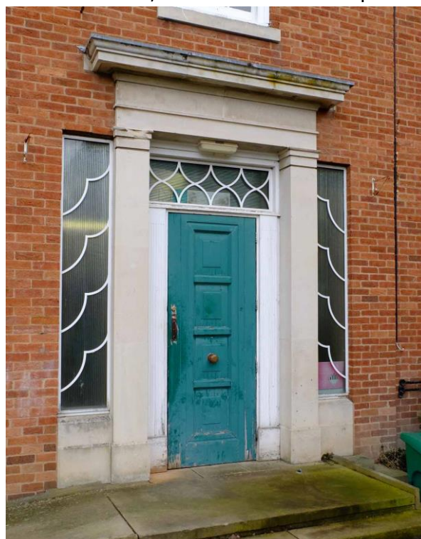
Figure 17. Doorway in the secondary wing.
