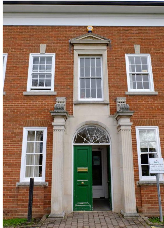
Figure 18. Entrance to the council suite.
