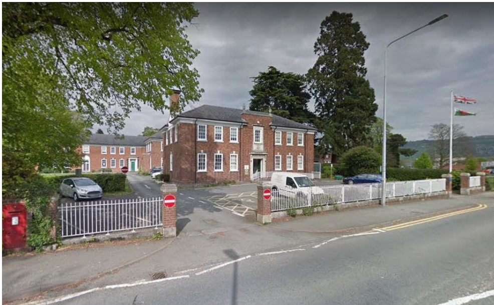
Figure 26. Railings and gate piers fronting Severn Street (© Google Street View).
