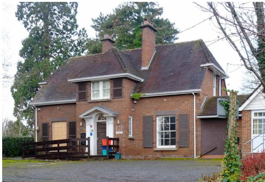
Figure 31. Chalfont, Severn Street.
