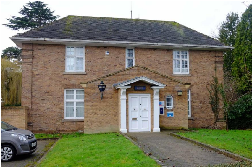
Figure 29. Police Station, Severn Street.
