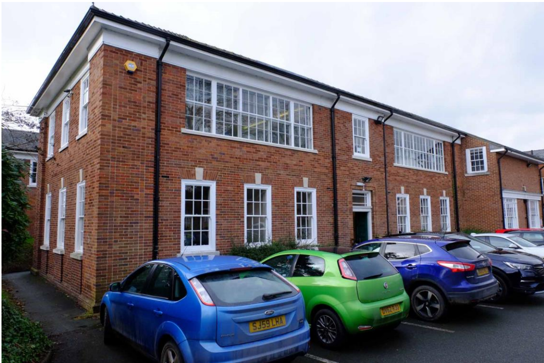
Figure 14. Rear (north-east) wall.
