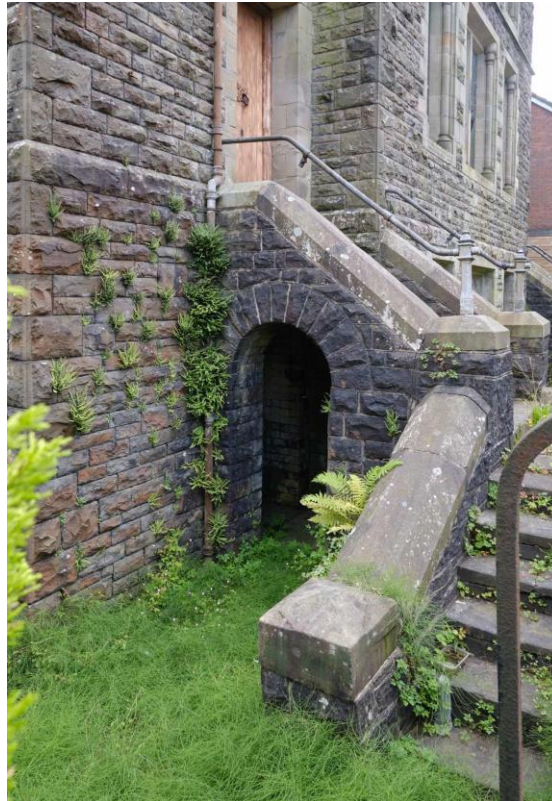
Figure 6. Steps to main entrance and basement doors, Church Road front.
