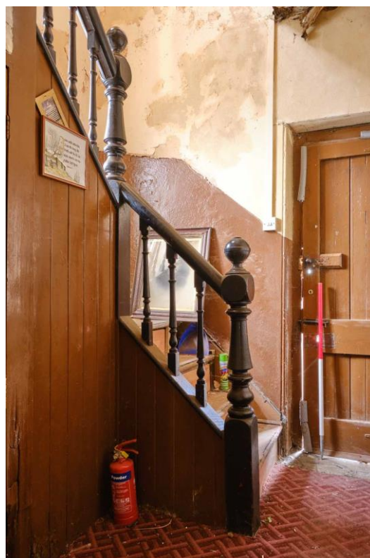
Figure 20. Rear stairs to basement.
