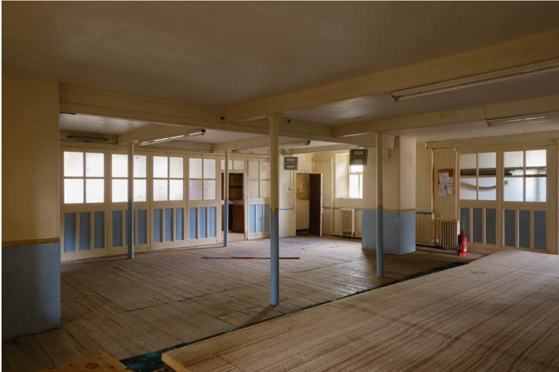
Figure 21. Basement with cast-iron posts supporting the ground floor.
