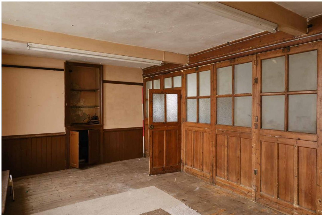
Figure 22. Basement, with partition to inner room.
