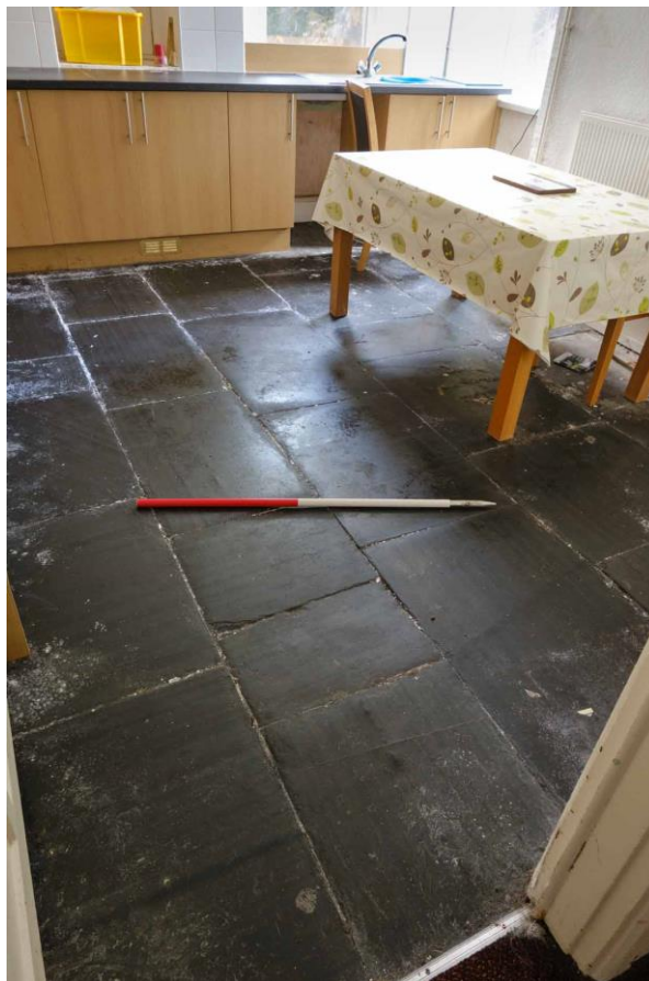
Figure 8. Flagstone kitchen floor.
