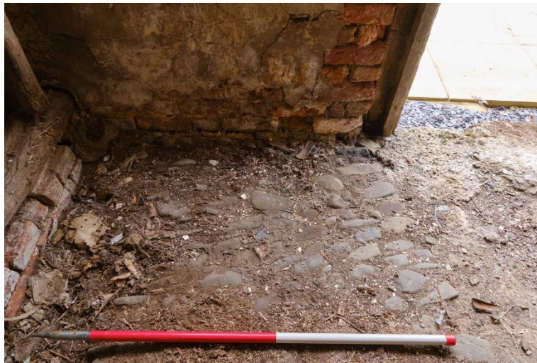
Figure 14. Cobbled floor in Unit 2.
