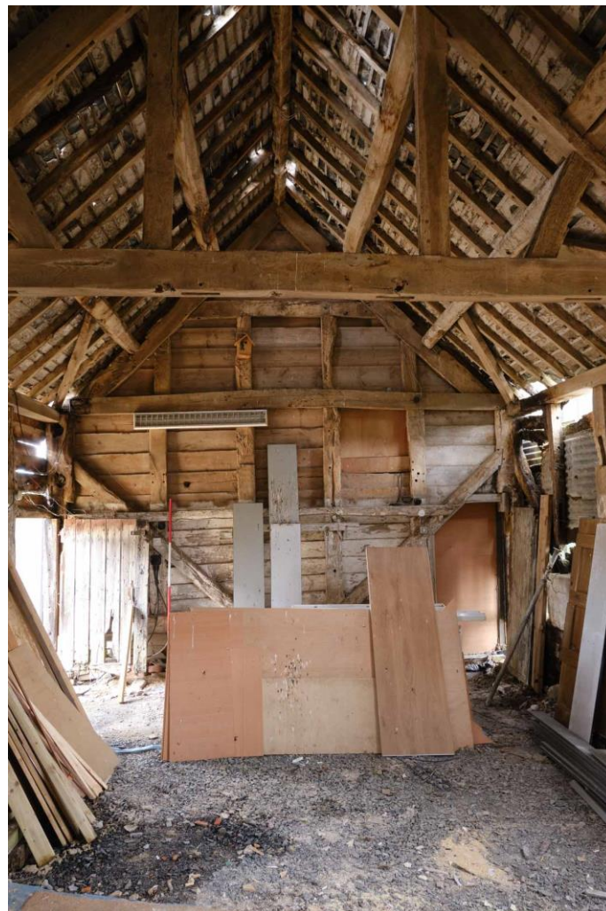
Figure 15. West gable end of the main barn, showing the passing braces.
