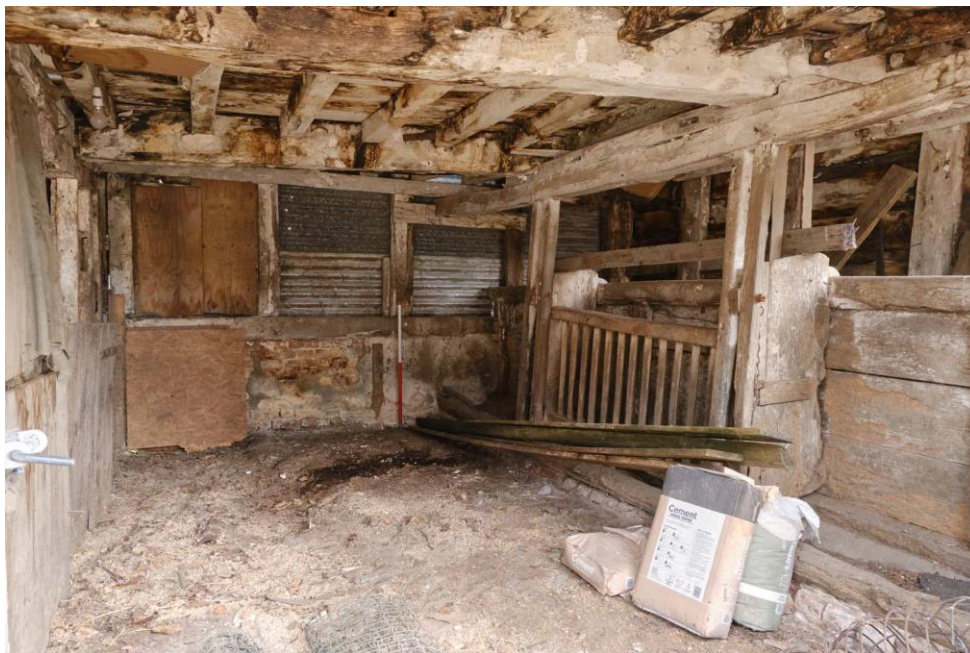
Figure 13. Unit 2, loose box, with feeding trough on the right.
