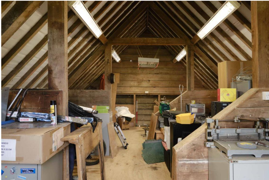
Figure 21. Loft (Unit 6) in the garage.
