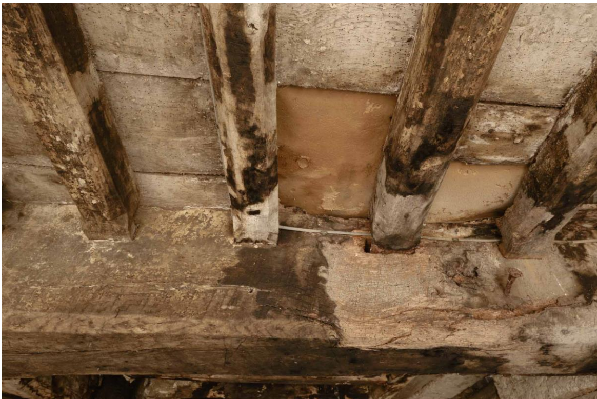
Figure 17. Chamfered joists and spine beam supporting the loft.
