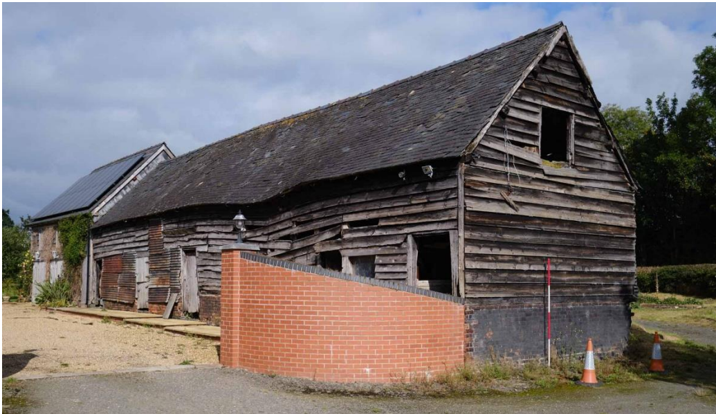
Figure 7. The barn, viewed from the south-east, with modern boundary wall.
