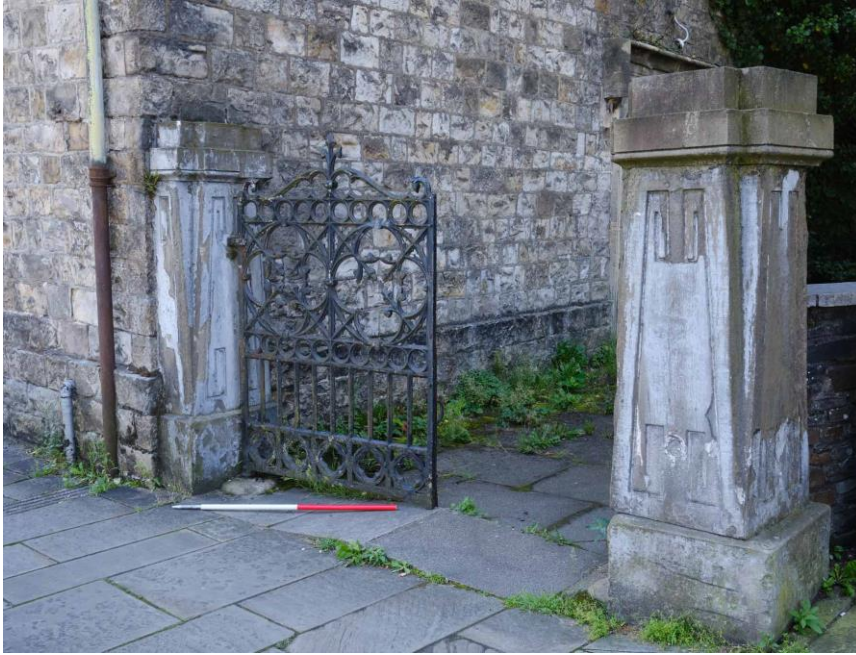
Figure 11. Gate piers and gates facing Hanbury Road.
