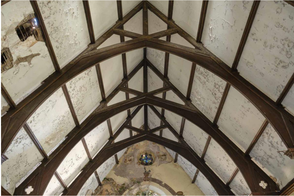
Figure 13. The nave roof.
