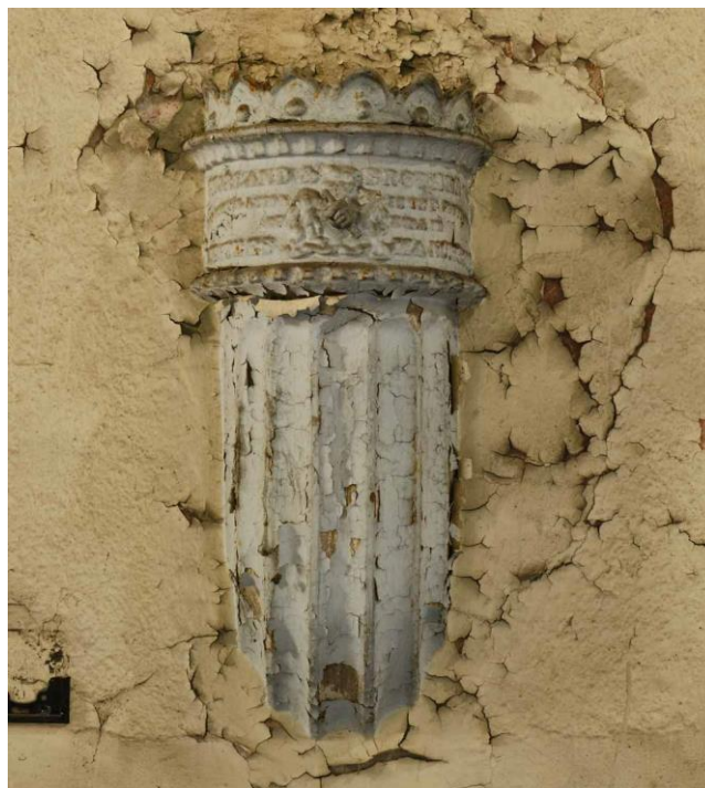
Figure 19. Cast iron ventilator in the nave wall.
