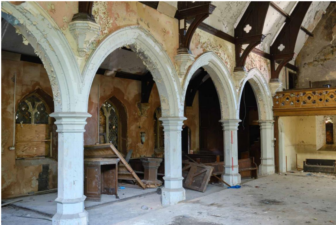
Figure 12. The nave arcade, looking south-west.
