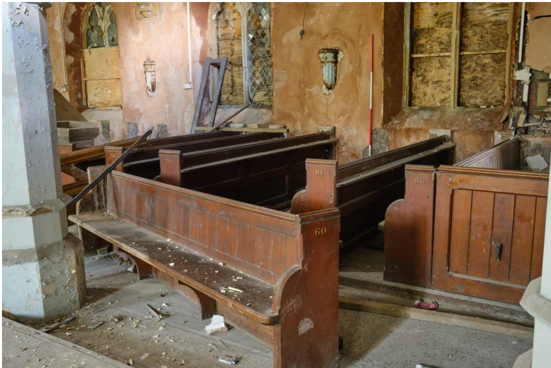
Figure 23. Numbered pews in the south aisle.
