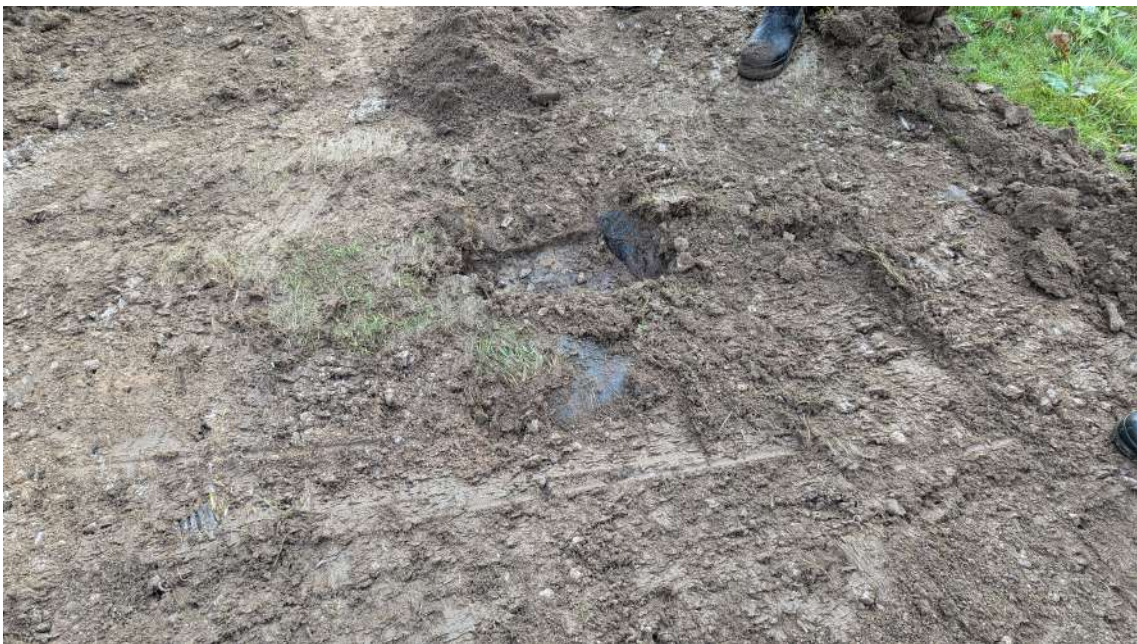
Plate 5: Ribbed plastic land drain directly below topsoil.
