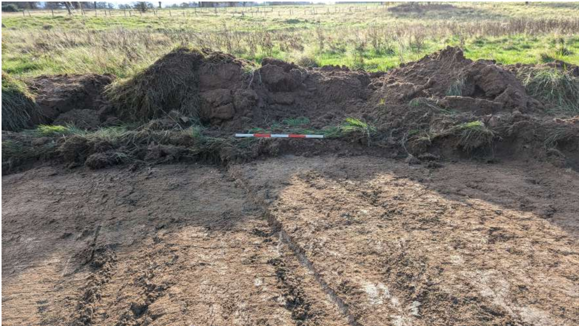
Plate 4: West facing section of path stripping, looking towards practice trenches
