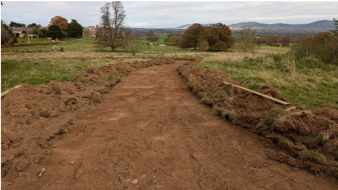
Plate 3: Working shot of excavation area, looking northwest.
