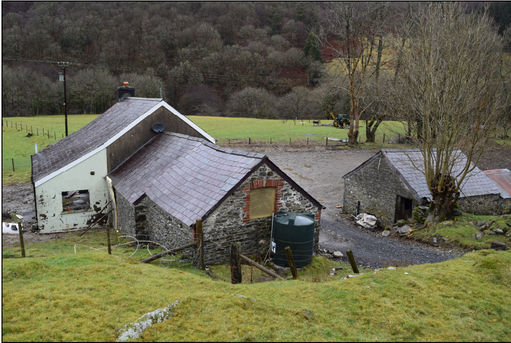
Plate 9: GFN2022_009. A view from the Gelli Burial Chamber, looking at the buildings of Gelli Fechan farm and its yard. Looking north.
