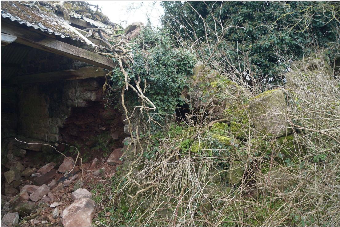
Plate 19: GTB2021_019 - A view of the eastern end of the open-sided storage shed showing the ruinous fragments of the original building and the collapsed southern end of the northern barn. Looking east.
