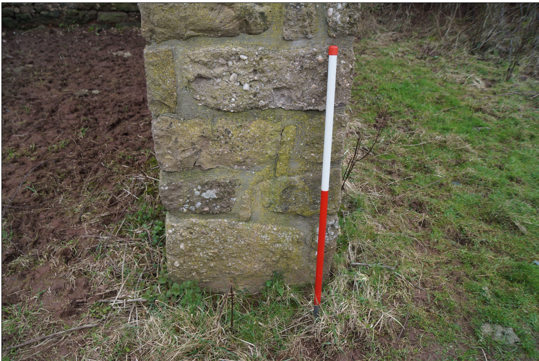
Plate 41: GTB2021_041 - A view of the door reveal at the eastern side of the southern doorway into the threshing barn. This is a modern reconstruction. Looking east-southeast.
