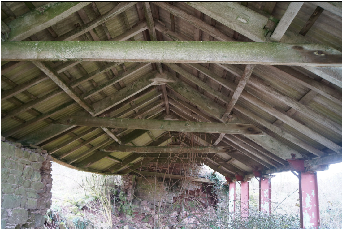
Plate 15: GTB2021_015 - A view inside the open sided storage shed next to the barn showing its combination of old and modern roof timbers. Looking east-southeast.
