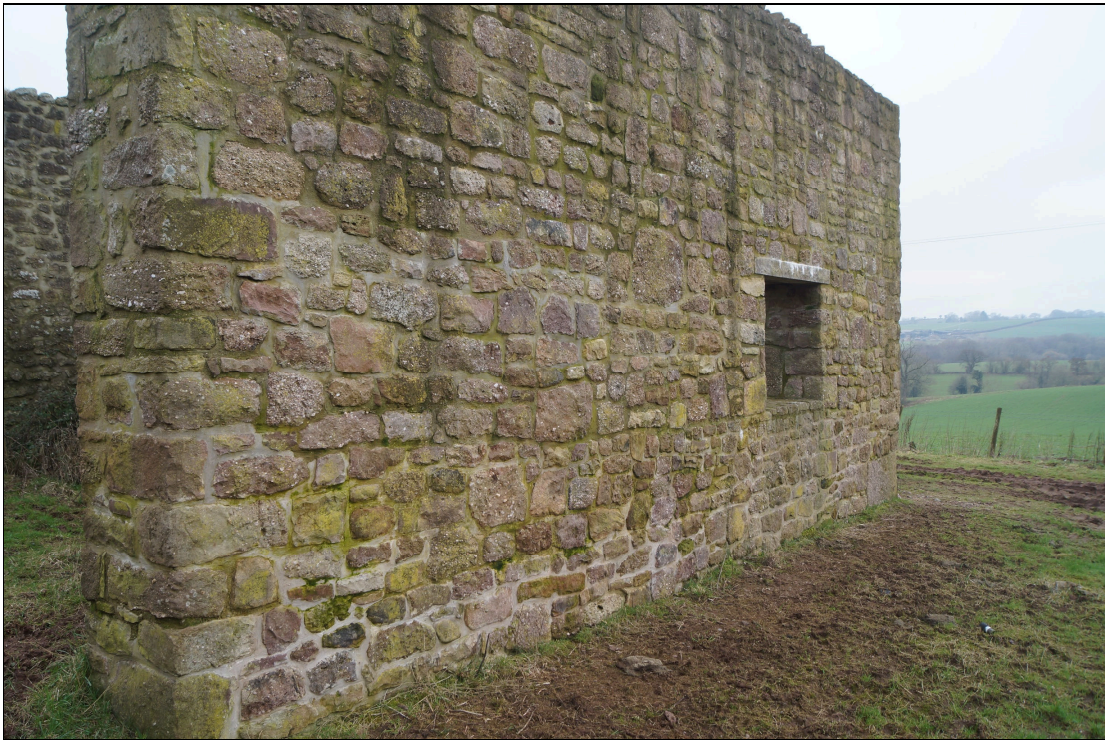
Plate 23: GTB2021_023 - A view of the western end of the external side of the northern lateral wall, which has been completely reconstructed on the original wall line. Looking west.
