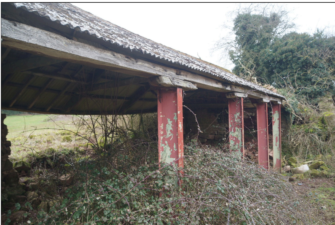
Plate 16: GTB2021_016 - A view of the steel girders holding up the roof of the open-sided storage shed next to the barn. Looking east-southeast.
