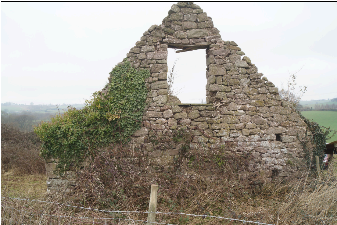
Plate 4: GTB2021_004 - A view of the external face of the eastern gable wall, showing the pitching window and a pair of ventilation holes on the right, the other four are obscured by vegetation. Looking west-northwest.
