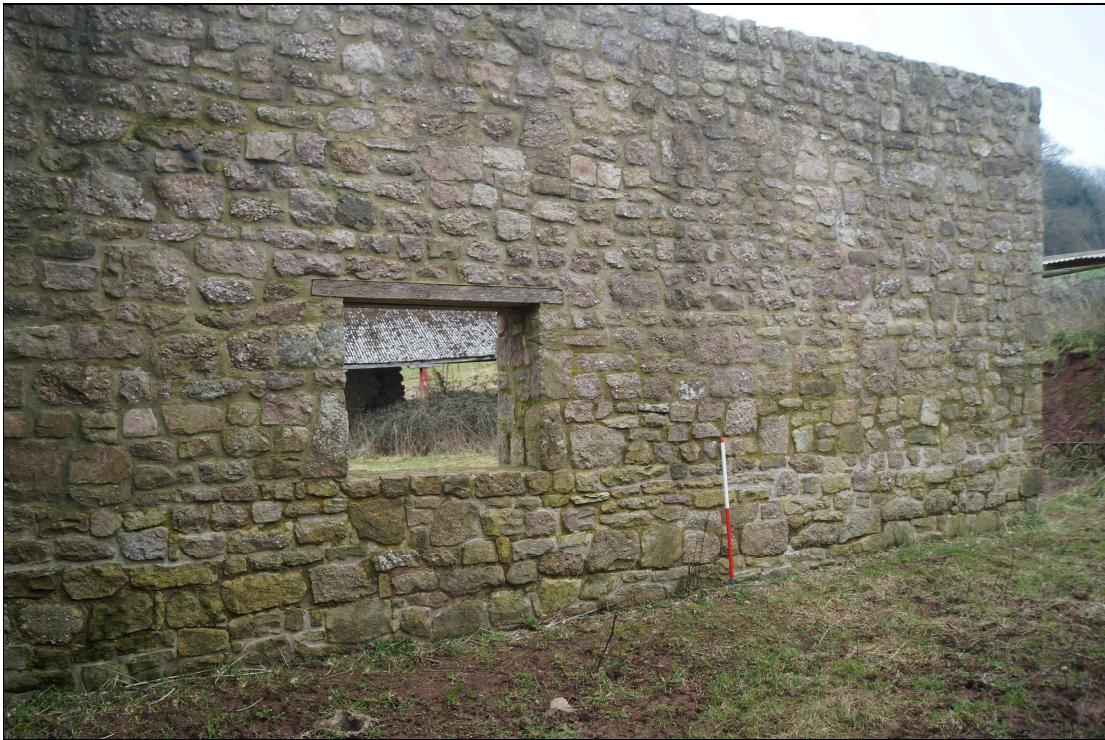
Plate 48: GTB2021_048 - A view outside the western end of the southern lateral wall, which has been reconstructed on the original foundation. Looking northeast.
