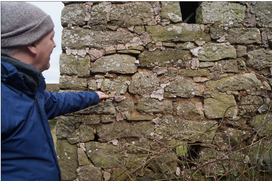
Plate 55: GTB2021_055 - A view showing Martin Locock taking Mortar Sample B from the eastern end of the northern lateral wall of the threshing barn. Looking north-northeast
