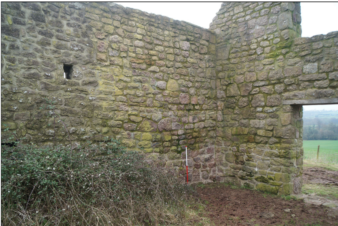
Plate 47: GTB2021_047 - A view inside the western end of the threshing barn, showing the reconstructed wall bonded with the original wall to the left. Looking west-southwest.
