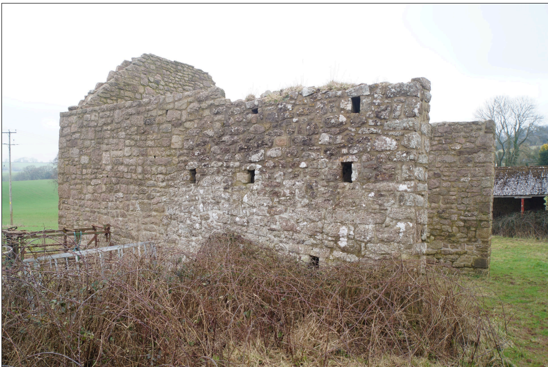
Plate 43: GTB2021_043 - A view of the western end of the threshing barn, showing the rebuilt western end of the southern lateral wall. The section of wall with ventilation holes is original. Looking north.
