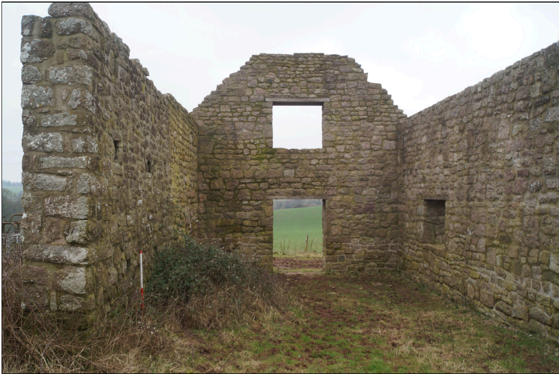
Plate 46: GTB2021_046 - A view inside the western end of the threshing barn, showing largely reconstructed walls. Only the first part of the wall to the left is original. Looking west-northwest.
