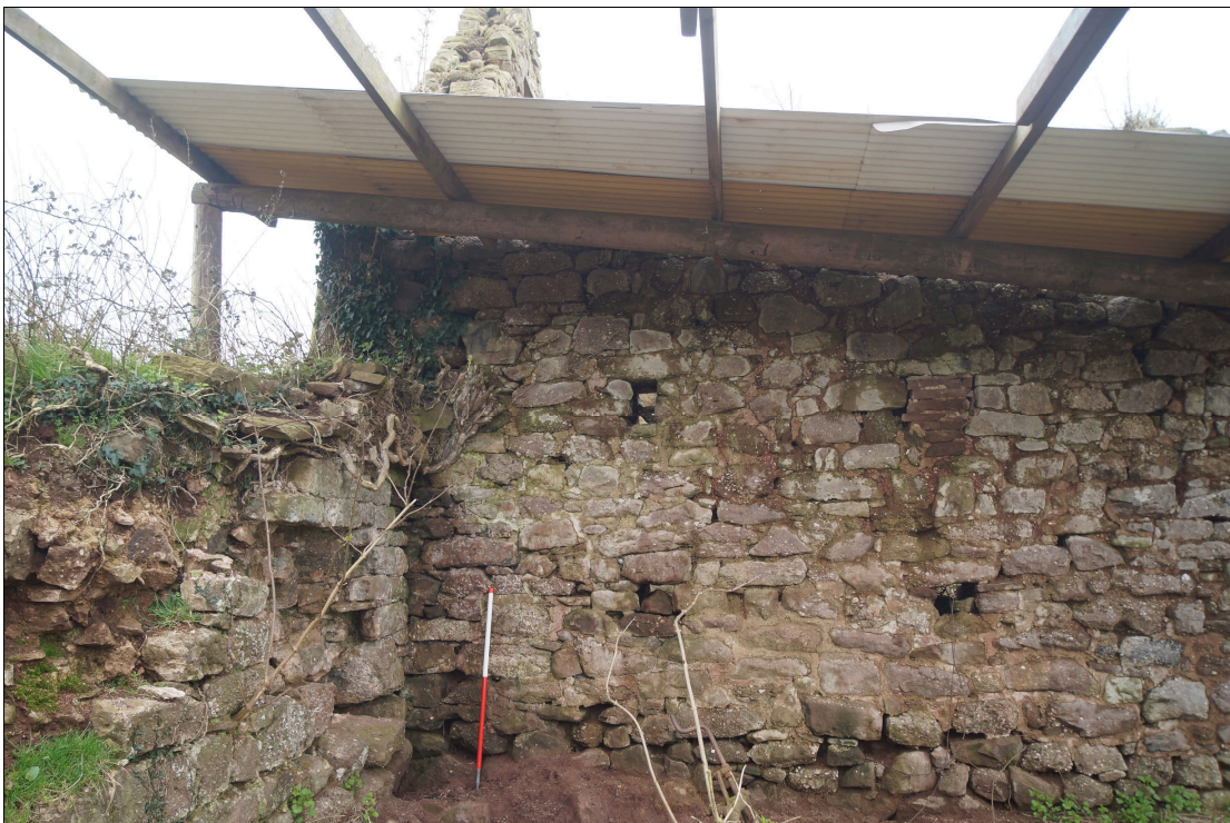
Plate 32: GTB2021_032 - A view of the eastern end of the northern lateral wall. A surviving section of the revetment wall. Note the ventilation holes of the threshing barn. Looking south-southwest.
