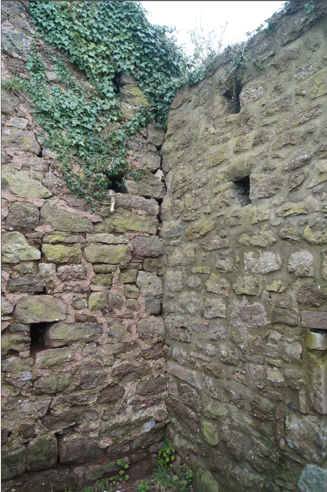
Plate 39: GTB2021_039 - A view of the inside of the southeast corner of the threshing barn showing a straight joint where the lateral wall and gable wall meet. Looking south.
