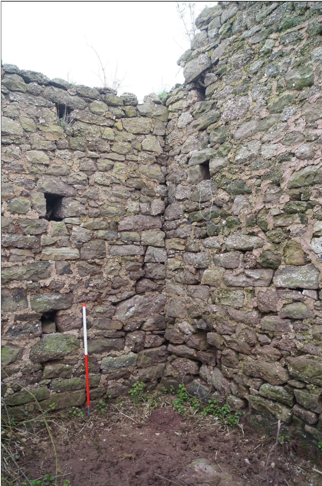
Plate 38: GTB2021_038 - A view of the inside of the northeast corner of the threshing barn showing a straight joint where the lateral wall and gable wall meet. This compares with the threshing barn at Llan y Nant Farm. Looking east-northeast.
