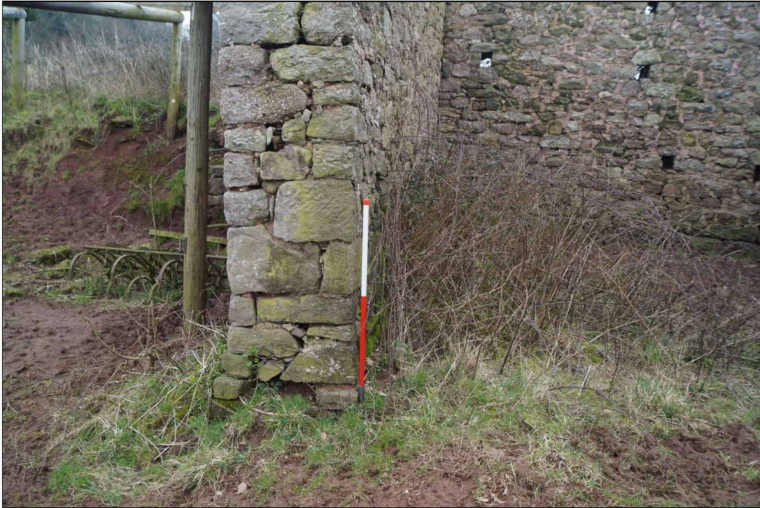
Plate 33: GTB2021_033 - A view of the door reveal at the eastern side of the northern doorway into the tithe barn. This is an original wall. Looking east-southeast.
