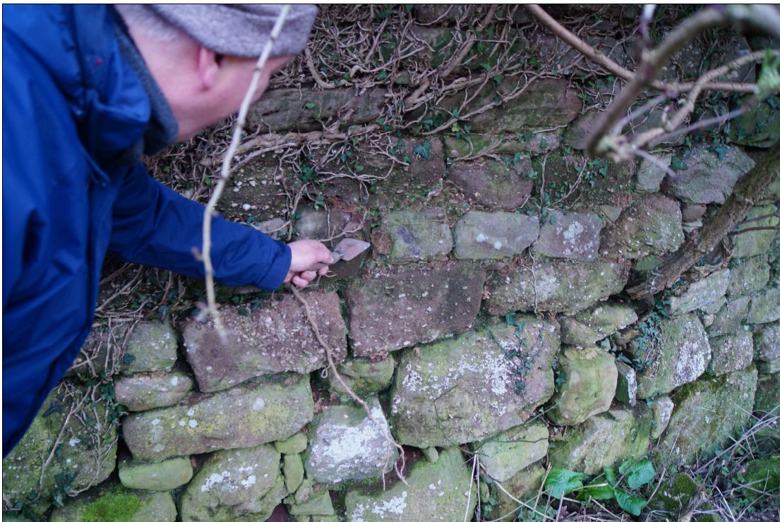
Plate 61: GTB2021_061 - A view showing Martin Locock taking Mortar Sample I from a surviving fragment of walling from the largely lost northern building in the complex at Gethley Barn. Looking southeast.
