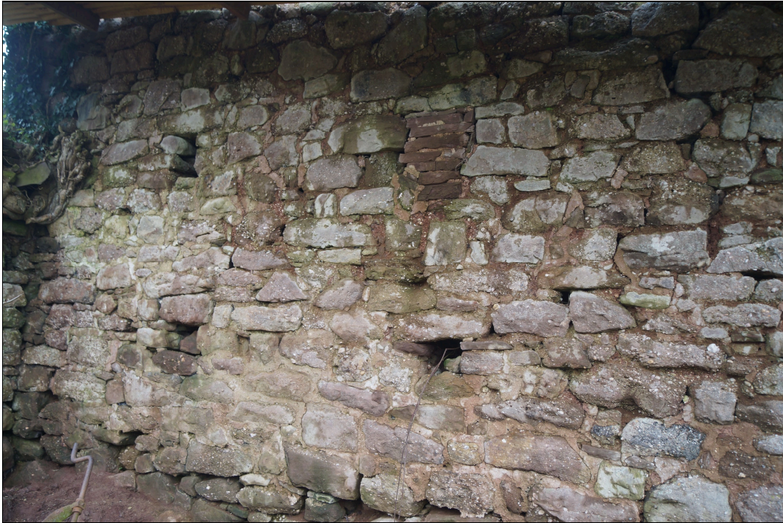
Plate 21: GTB2021_021 - A view of the eastern end of the external side of the northern lateral wall of Gethley Barn showing four ventilation holes, one of which has been blocked up. Looking south-southeast.
