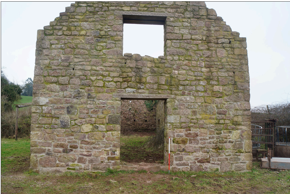
Plate 49: GTB2021_049 - A view of the wholly reconstructed western gable wall. Looking east-southeast.
