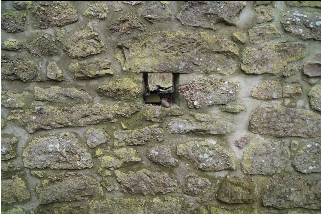
Plate 58: GTB2021_058 - A view of the lowest ventilation hole to the east of the doorway through the southern lateral wall. Looking south-southwest. Mortar sample F was taken from the core of the wall within the ventilation hole
