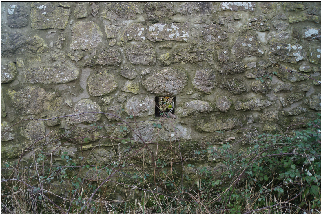
Plate 59: GTB2021_059 - A view of the lowest ventilation hole to the west of the doorway through the southern lateral wall. Looking south-southwest. Mortar sample G was taken from the core of the wall within the ventilation hole.
