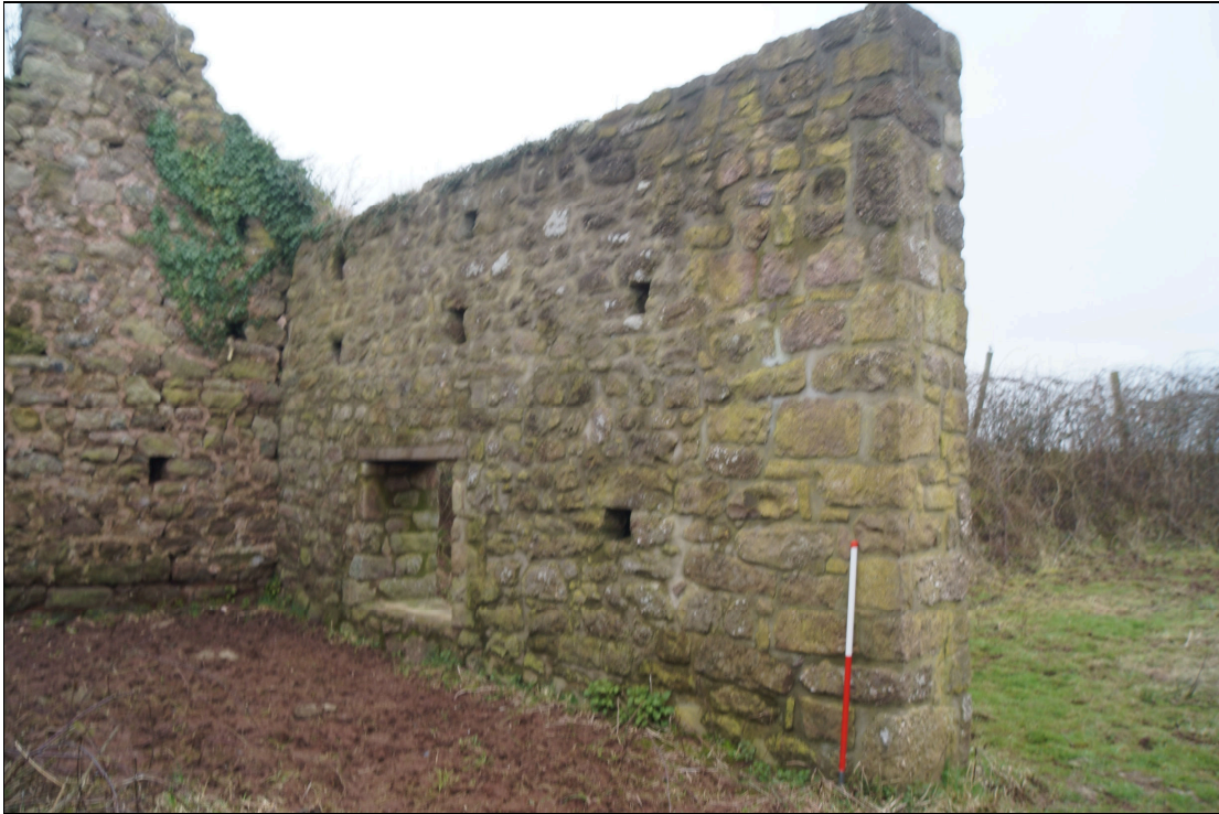
Plate 40: GTB2021_040 - A view inside the eastern end of the threshing barn, showing the original eastern end of the southern lateral wall. The door reveal to the right has been repaired in modern times. Looking south-southeast.
