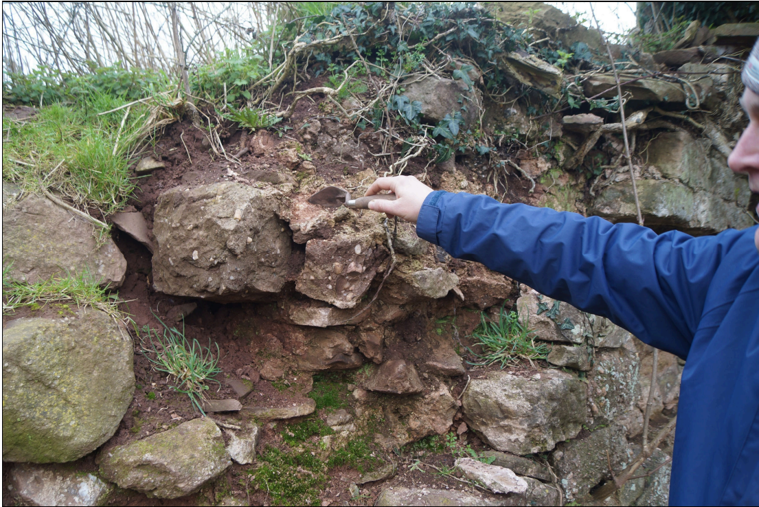
Plate 54: GTB2021_054 - A view showing Martin Locock taking Mortar Sample A from the revetment wall to the north of the threshing barn. Looking south-southeast
