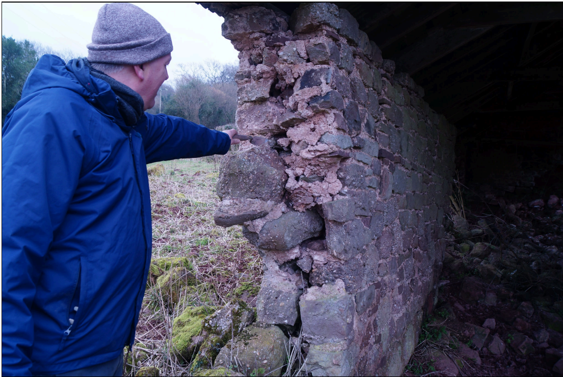
Plate 60: GTB2021_060 - A view showing Martin Locock taking Mortar Sample H from the core of the northern wall of the roofed storage shed to the north of the threshing barn. Looking east-southeast.
