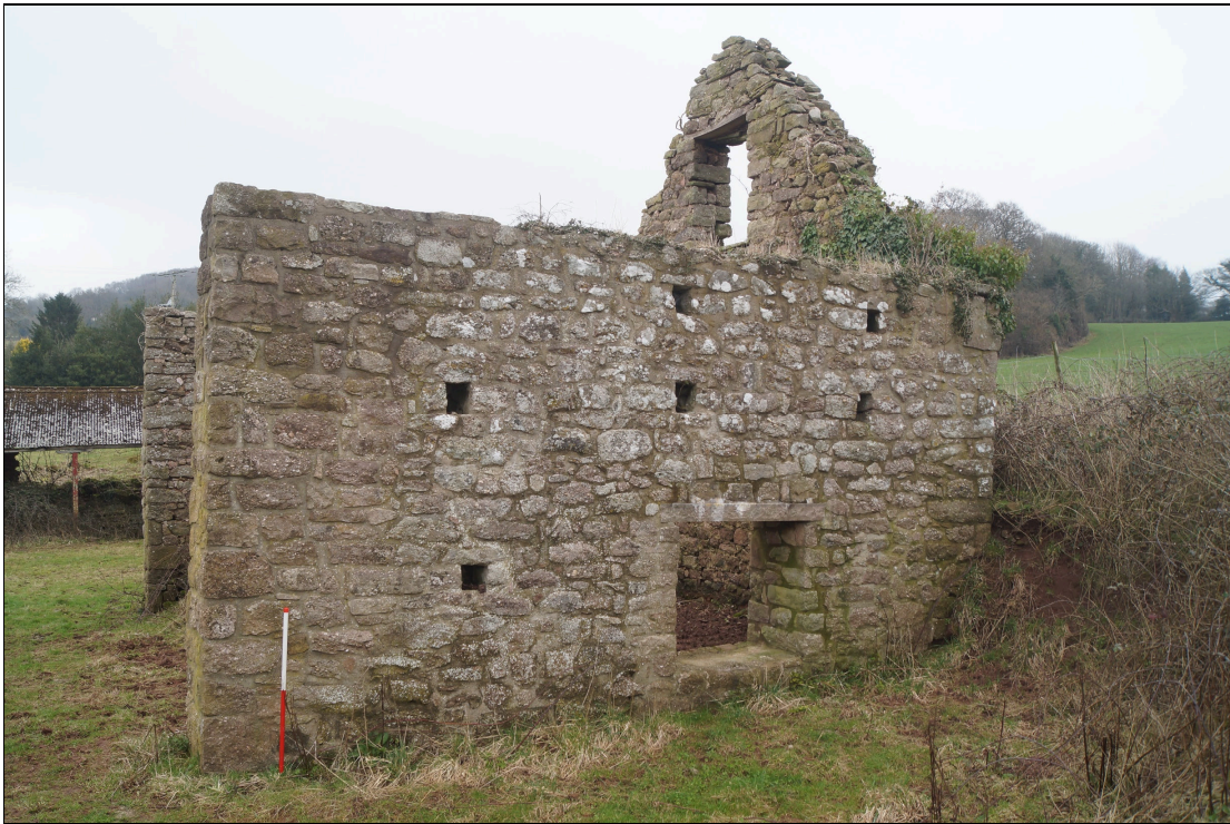
Plate 42: GTB2021_042 - A view of the eastern end of the threshing barn, showing the original eastern end of the southern lateral wall. The door reveal to the right has been repaired in modern times and the window is a modern insert. Looking east-northeast.
