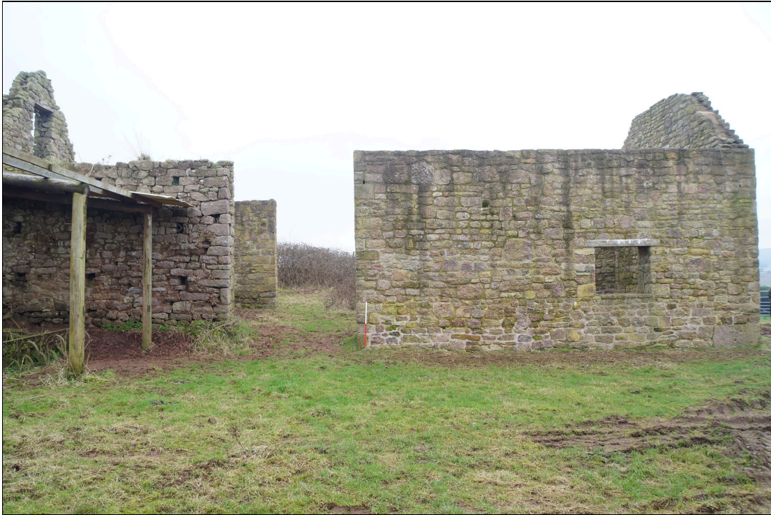
Plate 27: GTB2021_027 - A view of the threshing barn, showing the opposed doors through the lateral walls. Looking south-southwest.
