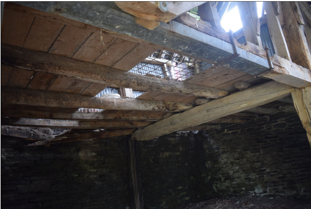
Plate 34: GBB2022_034 – A view of the timbers supporting the floor of the hayloft, looking from the ground floor level below. Looking northeast.
