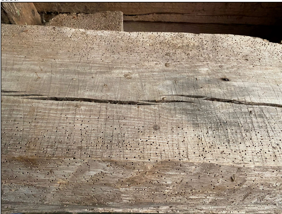
Plate 58: GBB2022_058 – A view of pit-saw kerf marks on the same beam as seen in photograph GBB2022_057 under the hayloft in the East West Barn. These usually might be assigned a pre-19 th century but are on the same beam as band saw kerf marks. Looking east.
