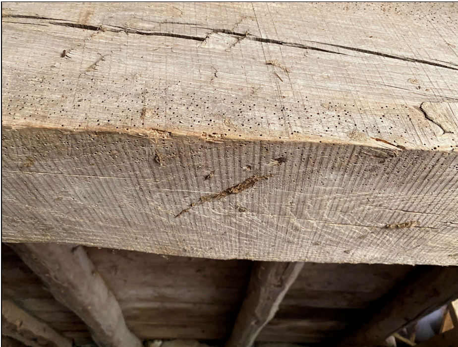
Plate 57: GBB2022_057 – A view of bandsaw kerf marks on a beam under the hayloft in the East West Barn. These would usually be dated to the mid-19 th century. Looking east.
