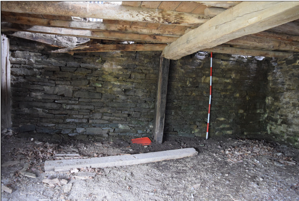
Plate 29: GBB2022_029 – A view inside the area beneath the hayloft at the north end of the East Barn, showing the stone revetment wall forming its northern side. Looking north.
