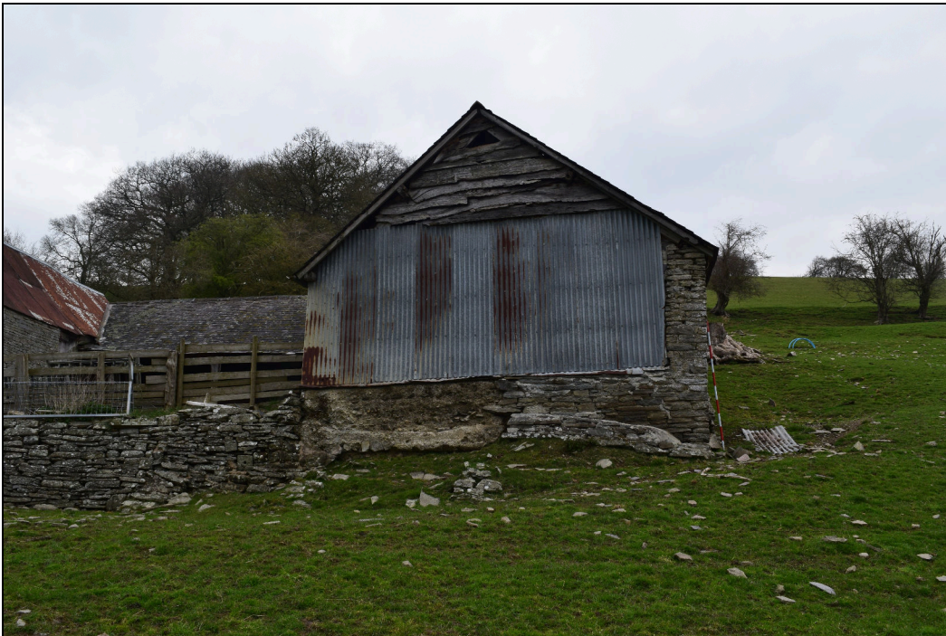
Plate 4: GBB2022_004 – A view of the southern gable of the East Barn, showing the plinth on which the south end of the building stands. Some facing stones have fallen away and been replaced by modern concrete mixed with stone. Looking north.
