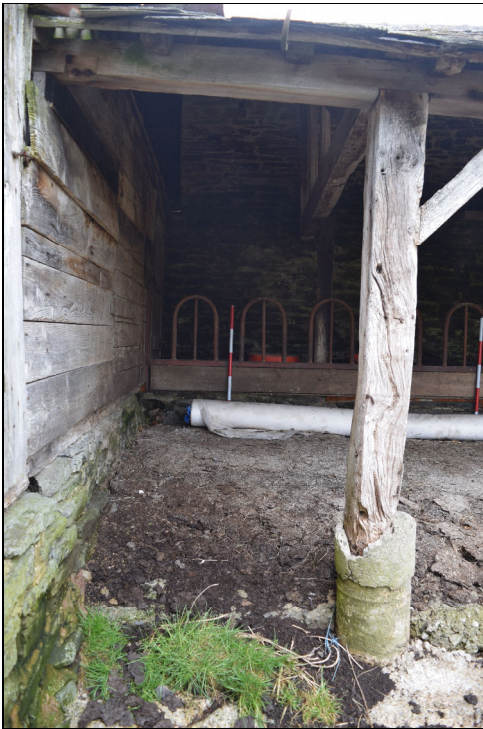
Plate 13: GBB2022_013 – A view of a wooden post supporting the Cowhouse roof along its southern side. The posts have evidently rotted at their base and had concrete poured around them in a mould to extend their use. Looking north.
