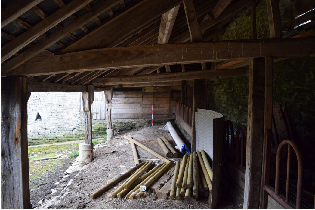
Plate 15: GBB2022_015 – A view inside the Cowhouse, showing the stalls and the raised feeding trough. Note the stone wall to the right, the bottom half of which is a revetment into the hillside. Looking west.
