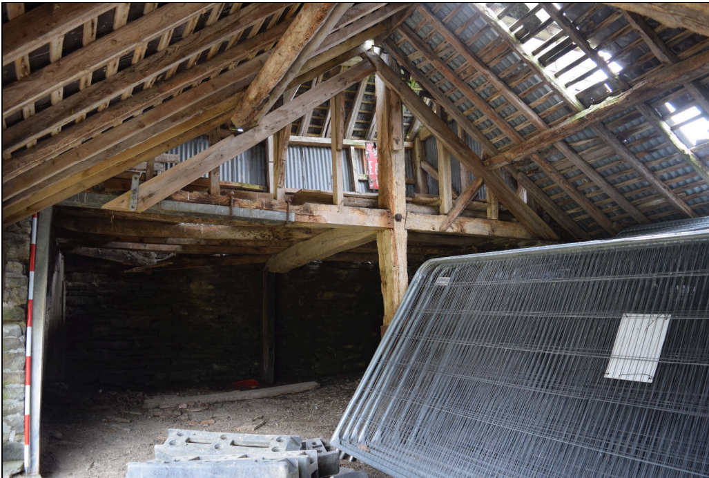
Plate 27: GBB2022_027 – A view inside the East Barn towards the hayloft. The corrugated sheeting visible at first-floor level is the inside of the north wall of the hayloft. Substantial beams support the floor of the hayloft. Looking north-northeast.
