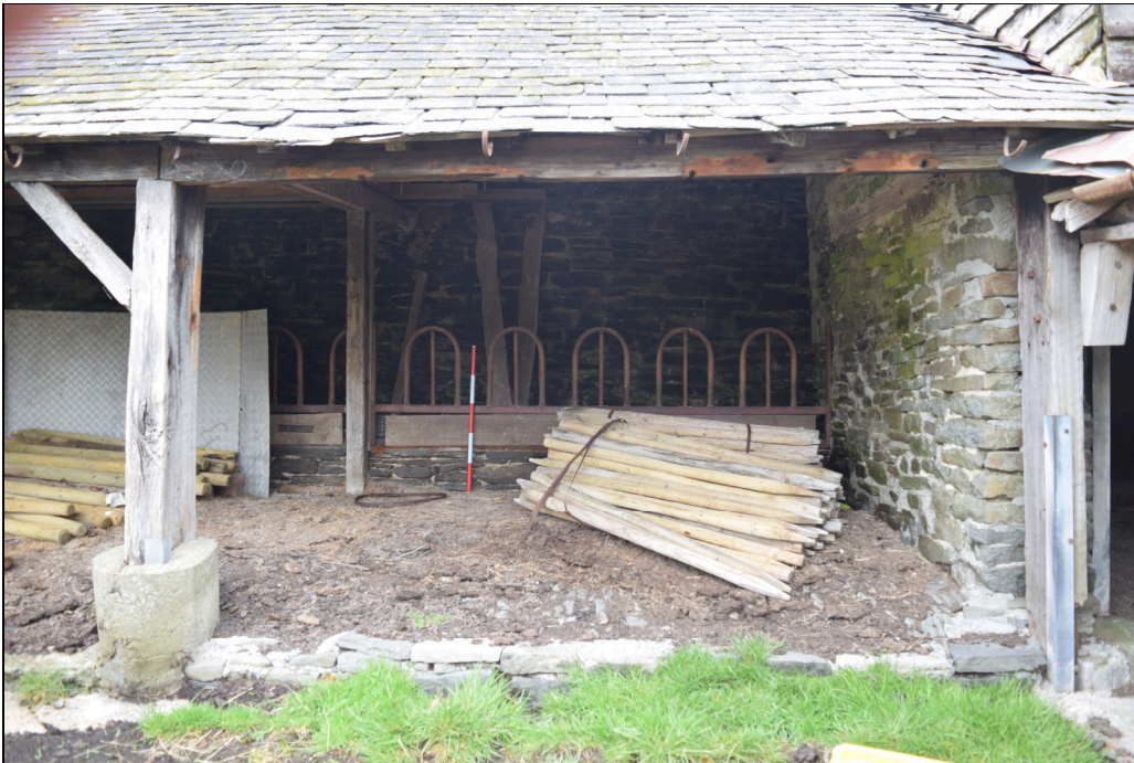
Plate 14: GBB2022_014 – A view of the east side of the Cowhouse. The original roof posts here have been replaced with wooden railway sleepers. Looking north.
