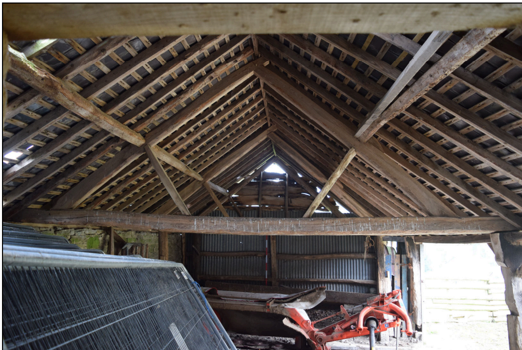
Plate 24: GBB2022_024 – A view inside the East Barn towards the south gable end, the wall of which is crudely built and clad in corrugated sheeting. Looking south.
