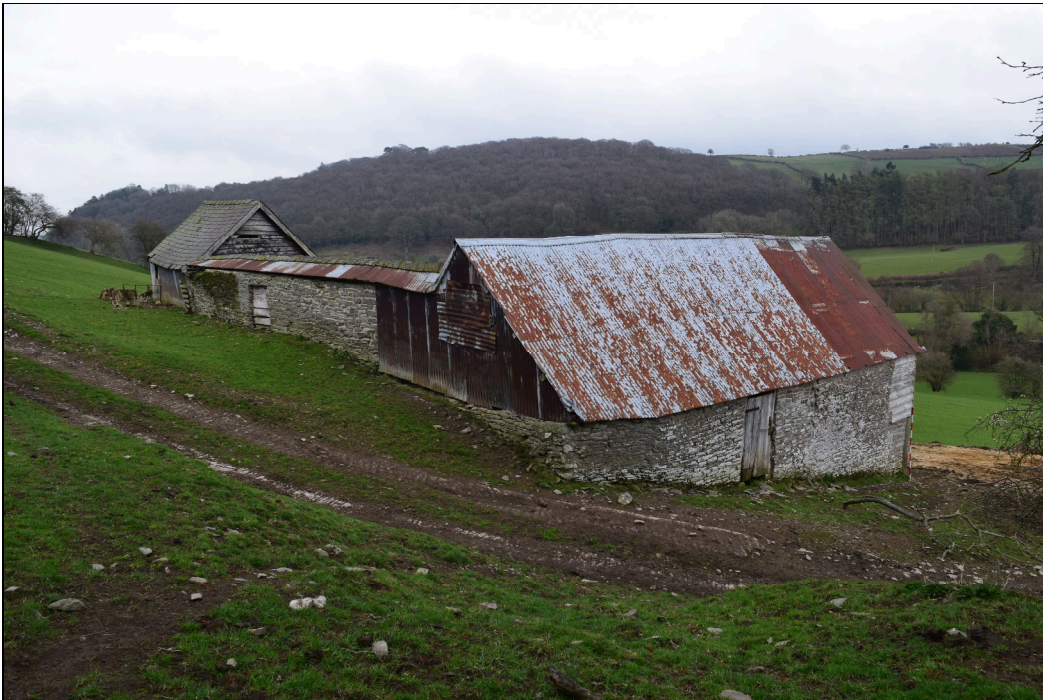
Plate 11: GBB2022_011 – A view of the barn complex, showing the stone western wall of the West Barn, which has a corrugated steel roof over timber. Looking southeast.
