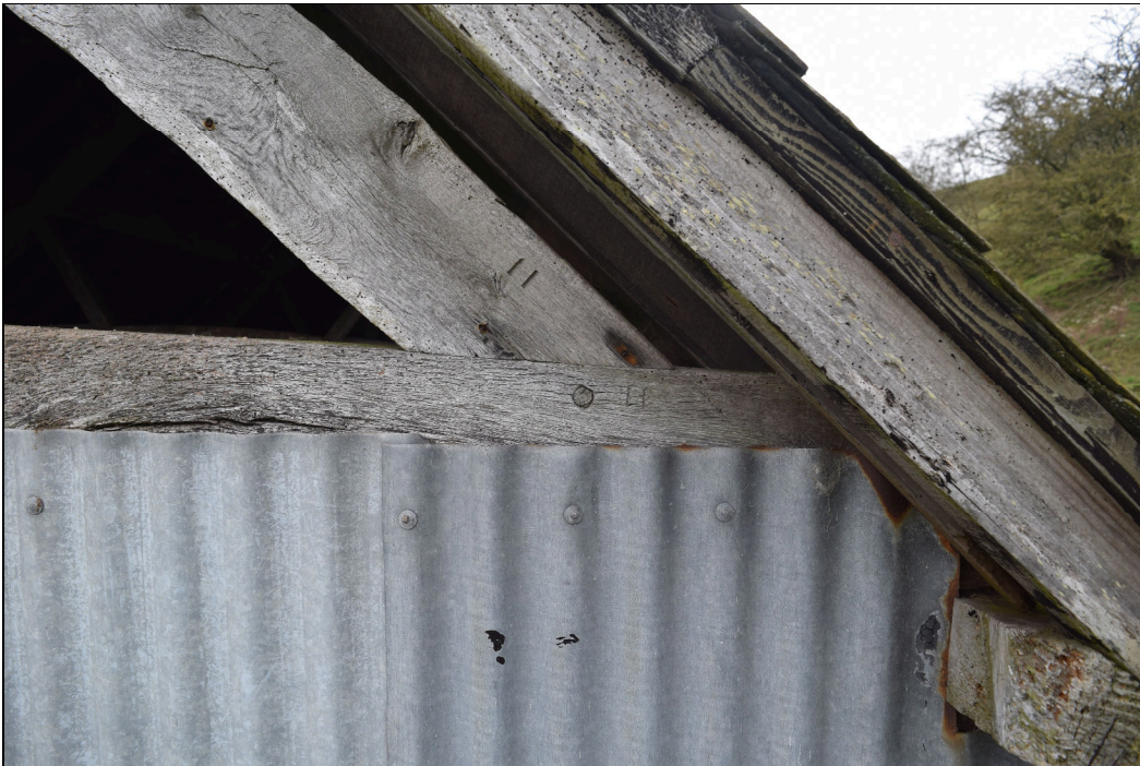
Plate 37: GBB2022_037 – A view of carpenters' marks in the roof truss in the east side of the hayloft. Looking west.
