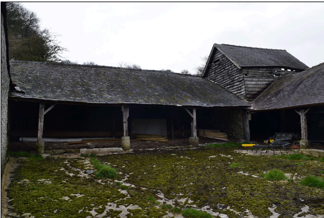
Plate 18: GBB2022_018 – An external view of the Cowhouse, showing its relationship with the hayloft at the north end of the East Barn. The hayloft is weatherboarded at first-storey level and has a stone wall at its west side at ground floor level. Looking northeast.
