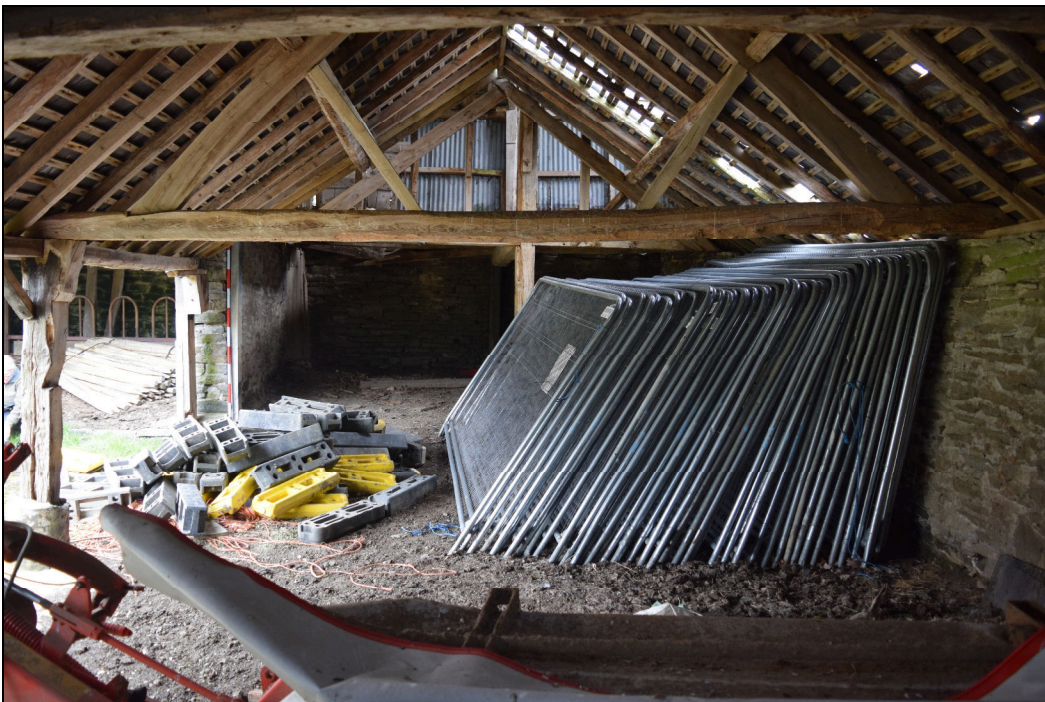
Plate 26: GBB2022_026 – A view inside the East Barn towards the north end, where there are stone walls beneath the hayloft. The corrugated sheeting visible at first-floor level is the inside of the north wall of the hayloft. Looking north.
