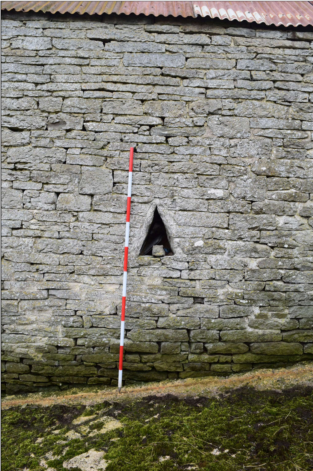
Plate 50: GBB2022_050 – A view of a triangular ventilation hole in the east wall of the West Barn, viewed from outside. Looking west.
