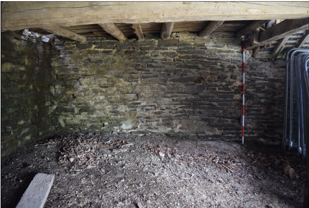
Plate 30: GBB2022_030 – A view inside the area beneath the hayloft at the east side of the East Barn, showing the stone revetment wall forming its eastern side. Looking east.
