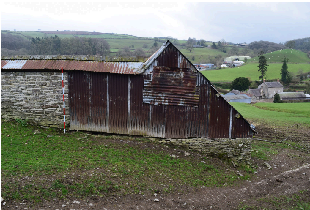
Plate 10: GBB2022_010 – A view of the north side of the West Barn. The timber-framed wall is clad in corrugated sheeting. Looking south.
