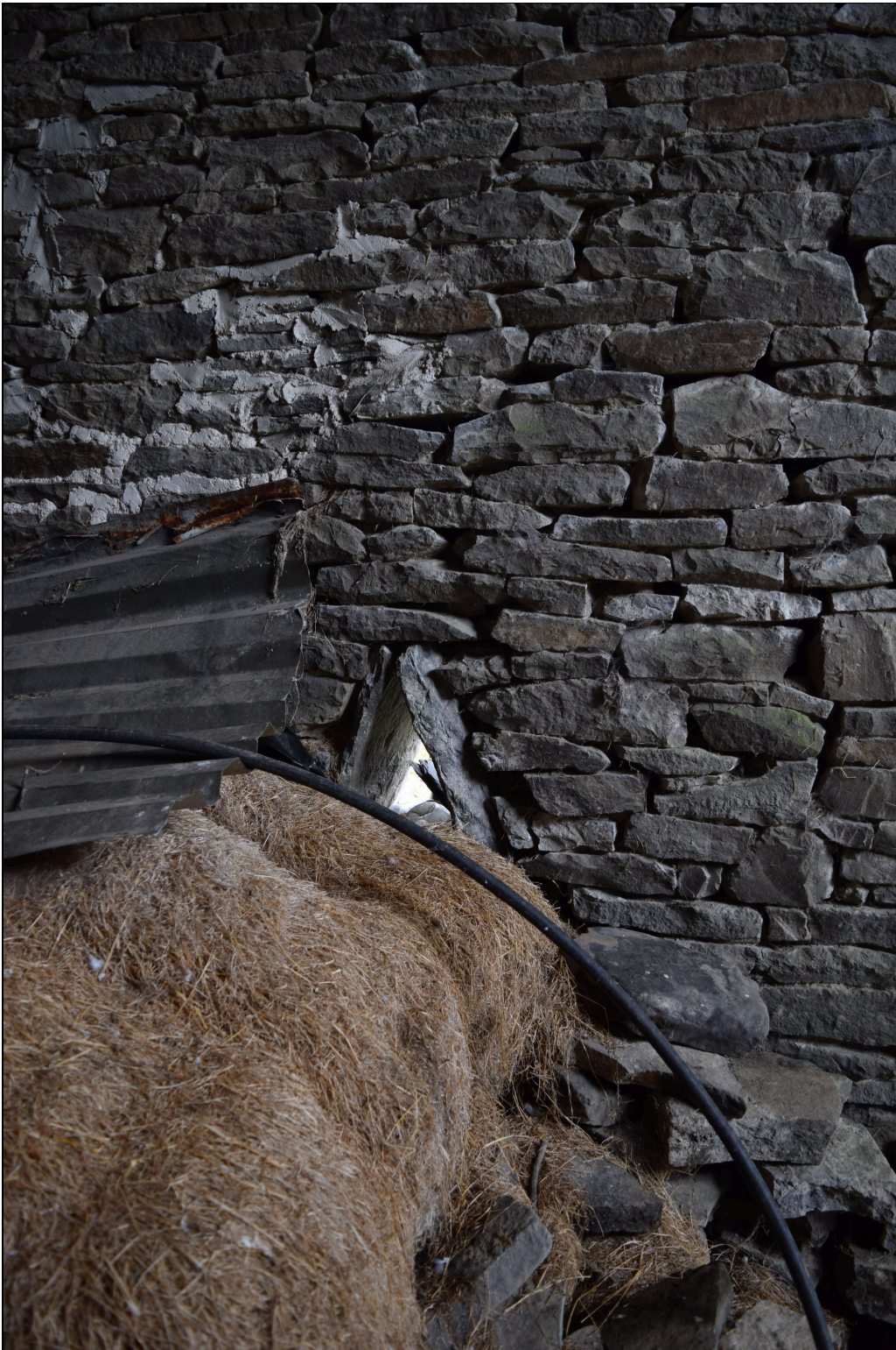
Plate 51: GBB2022_051 – A view of a triangular ventilation hole in the east wall of the West Barn, viewed from inside the barn. Looking east.
