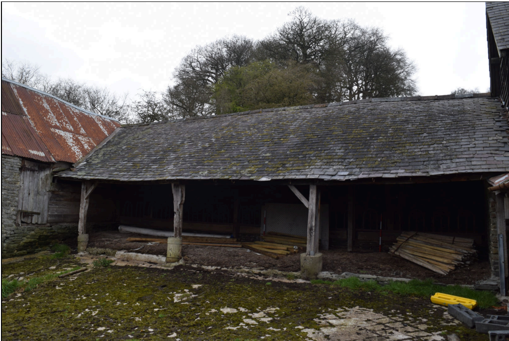
Plate 19: GBB2022_019 – An external view of the Cowhouse, showing its relationship with the north end of the West Barn. It appears that the Cowhouse is a later insertion into the complex. Looking north-northwest.
