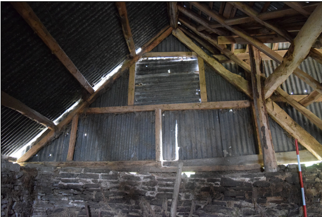
Plate 48: GBB2022_048 – A view inside the West Barn, showing the timber-framed gable wall above the revetment wall at the north end of the barn. Looking north.
