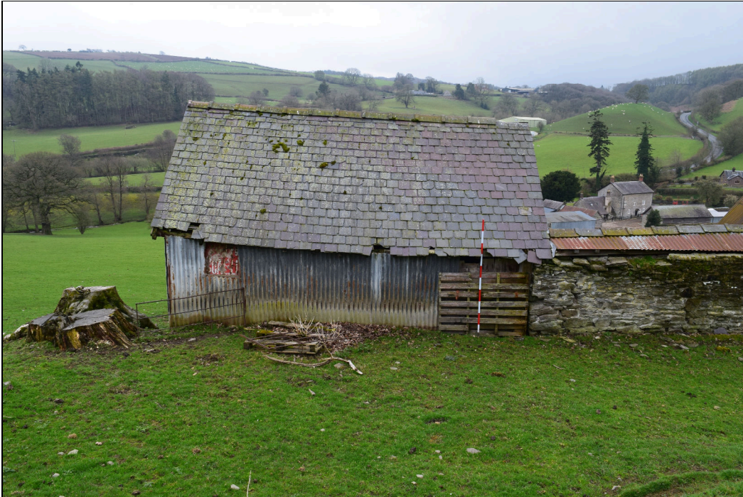
Plate 7: GBB2022_007 – A view of north side of the Hay Loft, showing the slate roof. The timber-framed north wall has been clad with corrugated sheeting. Looking south.
