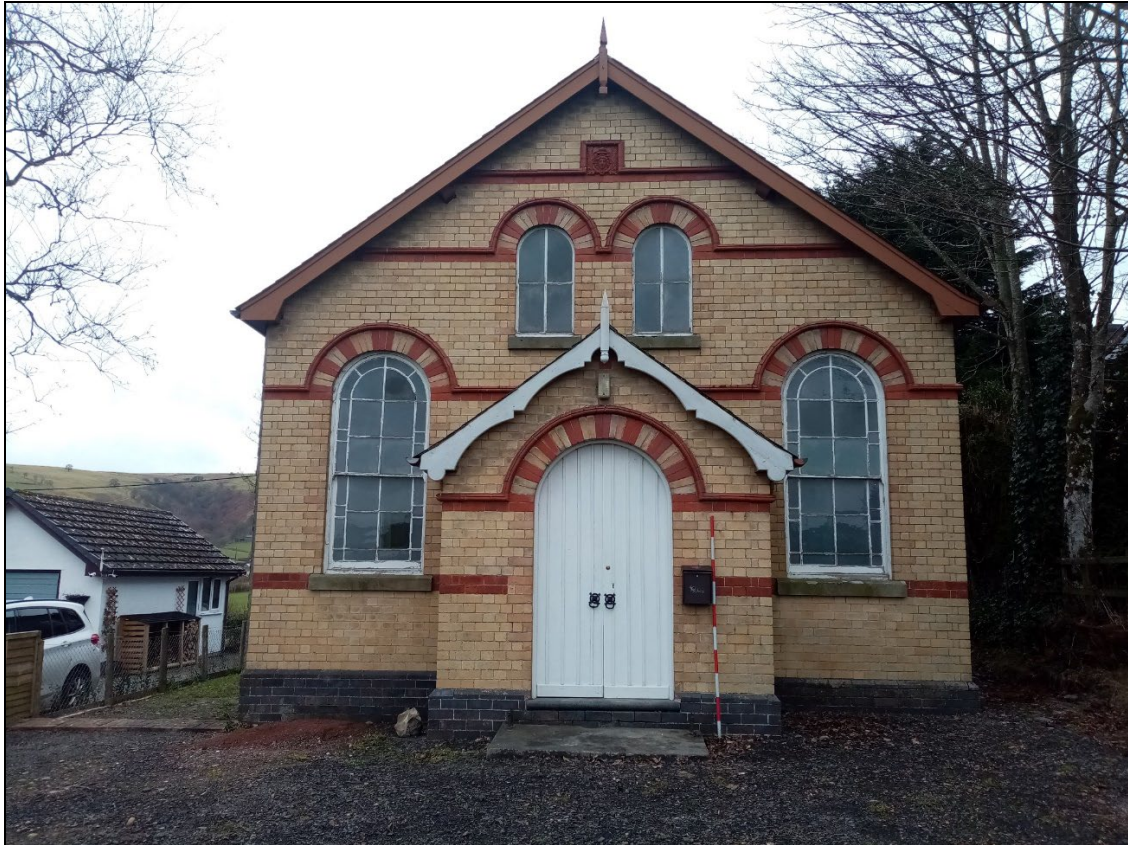
Plate 1: GCP2023_001. A view of the façade of Green Chapel. Looking west-northwest. Two metre scale.
