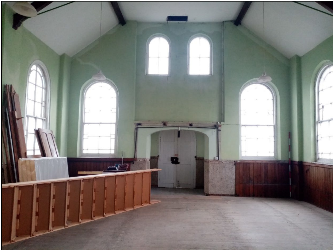
Plate 19: GCP2023_019. A view of the interior of the chapel, looking towards the eastern end of the building, with the main door closed. Looking east-southeast. Two metre scale.
