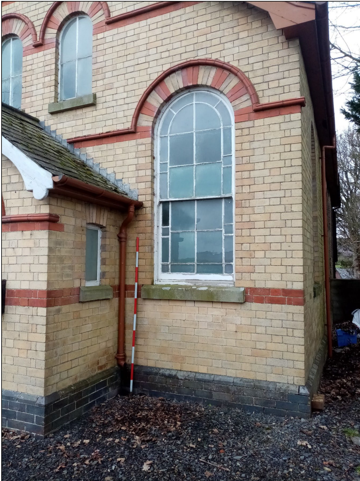
Plate 9: GCP2023_009. A view of a window in the northern side of the façade of the chapel. Looking west. Two metre scale
