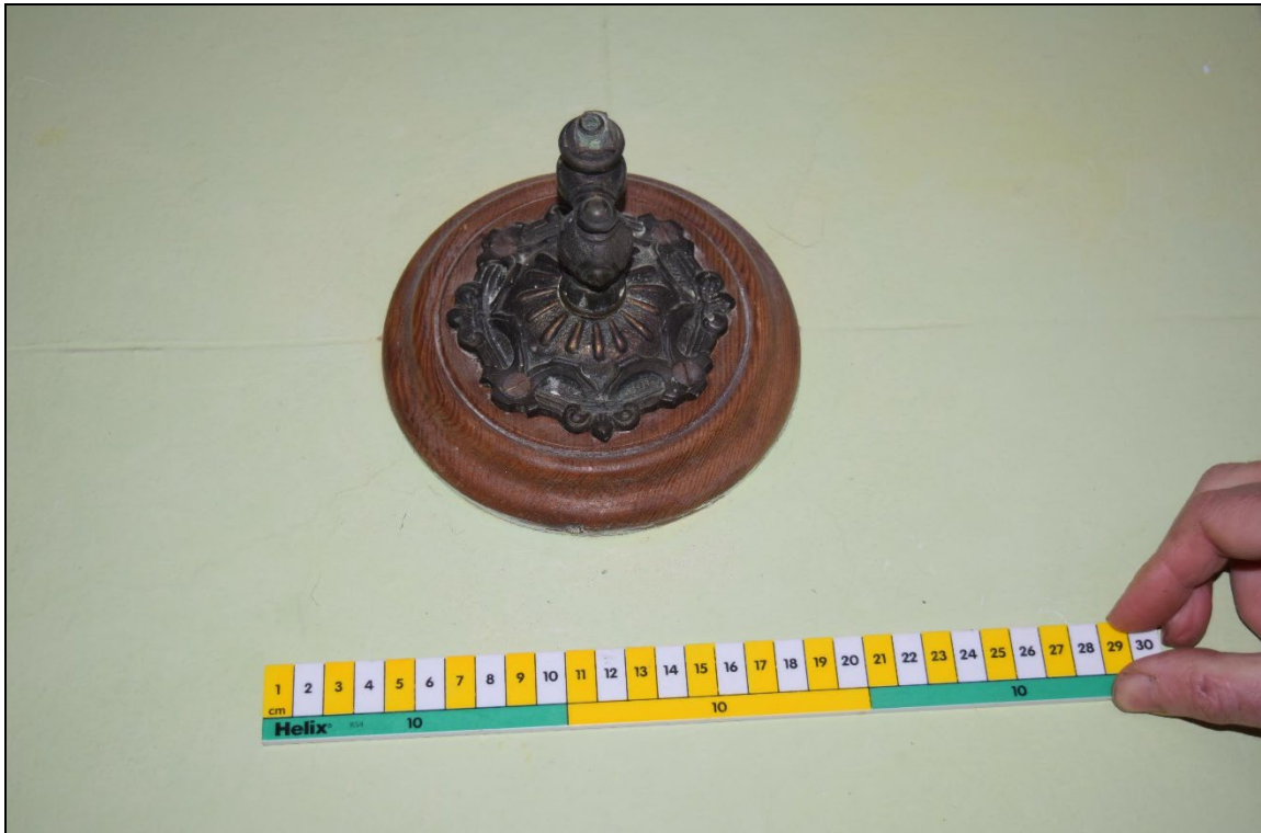
Plate 34: GCP2023_034. A view of a former gas lamp mount on the northern wall of the chapel. Looking north-northeast. Centimetre scale.
