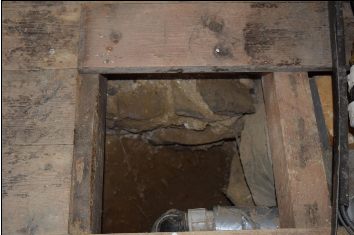
Plate 36: GCP2023_036. A view of stone footings supporting the wooden floor of the chapel, exposed through a gap in the flooring. Looking west-northwest.
