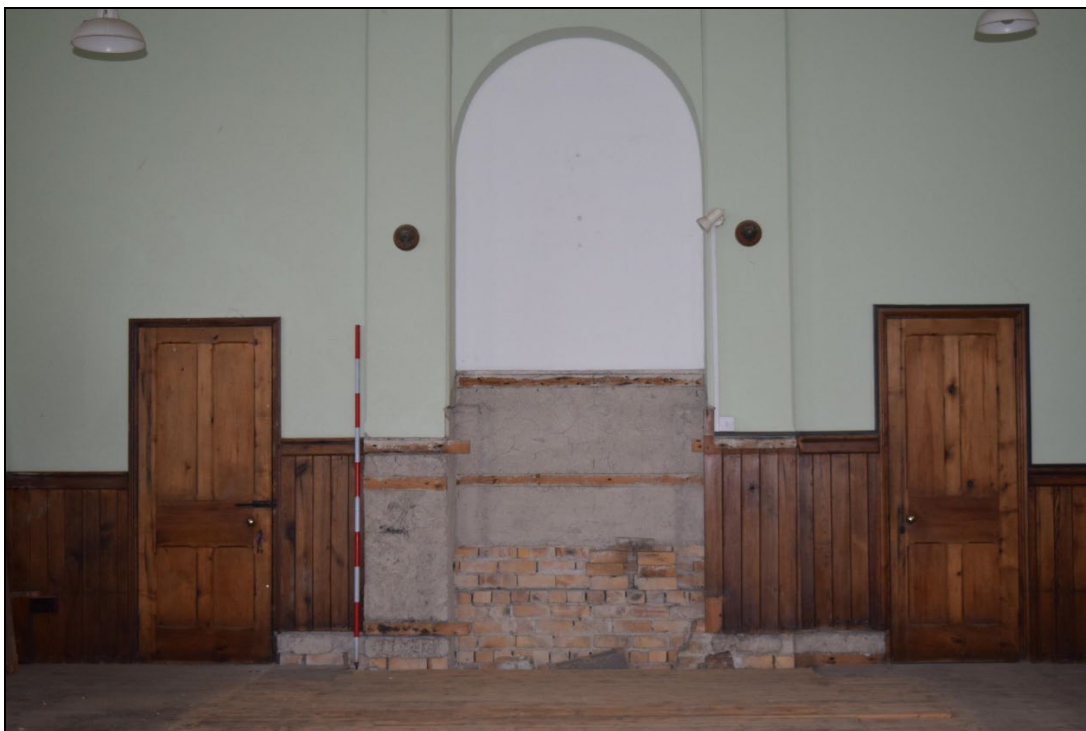
Plate 20: GCP2023_020. A view of the former location of the pulpit showing flanking doorways. Looking west-northwest. Two metre scale.
