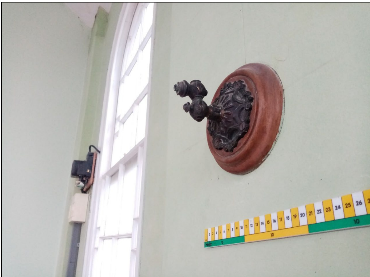
Plate 33: GCP2023_033. A view of a former gas lamp mount on the northern wall of the chapel. Looking north-northwest. Centimetre scale.
