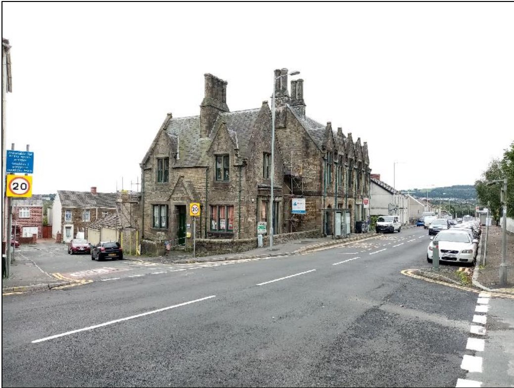
Plate 9: A view towards the former Police Station and house, looking south-southeast. 69, Martin Street is just out of view on the right of the photograph, but would be within peripheral view of an onlooker.
