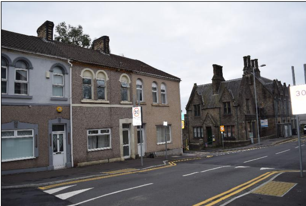
Plate 15: A view of the former Police Station, looking south-southeast.
