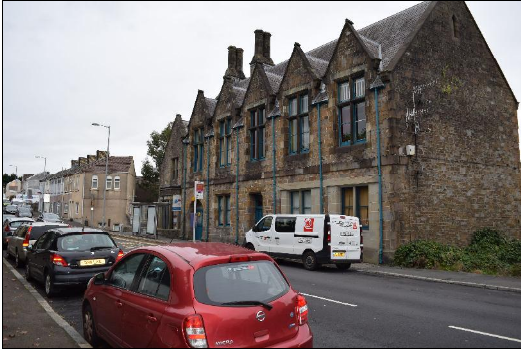
Plate 14: A view of the former Police Station, looking northeast.
