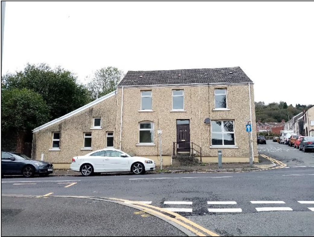
Plate 1: A view towards the front of 69, Martin Street, from the junction of Lower Banwell Street and Martin Street, looking west. The building has been insulated and rendered but note the raised doorway and stone steps.
