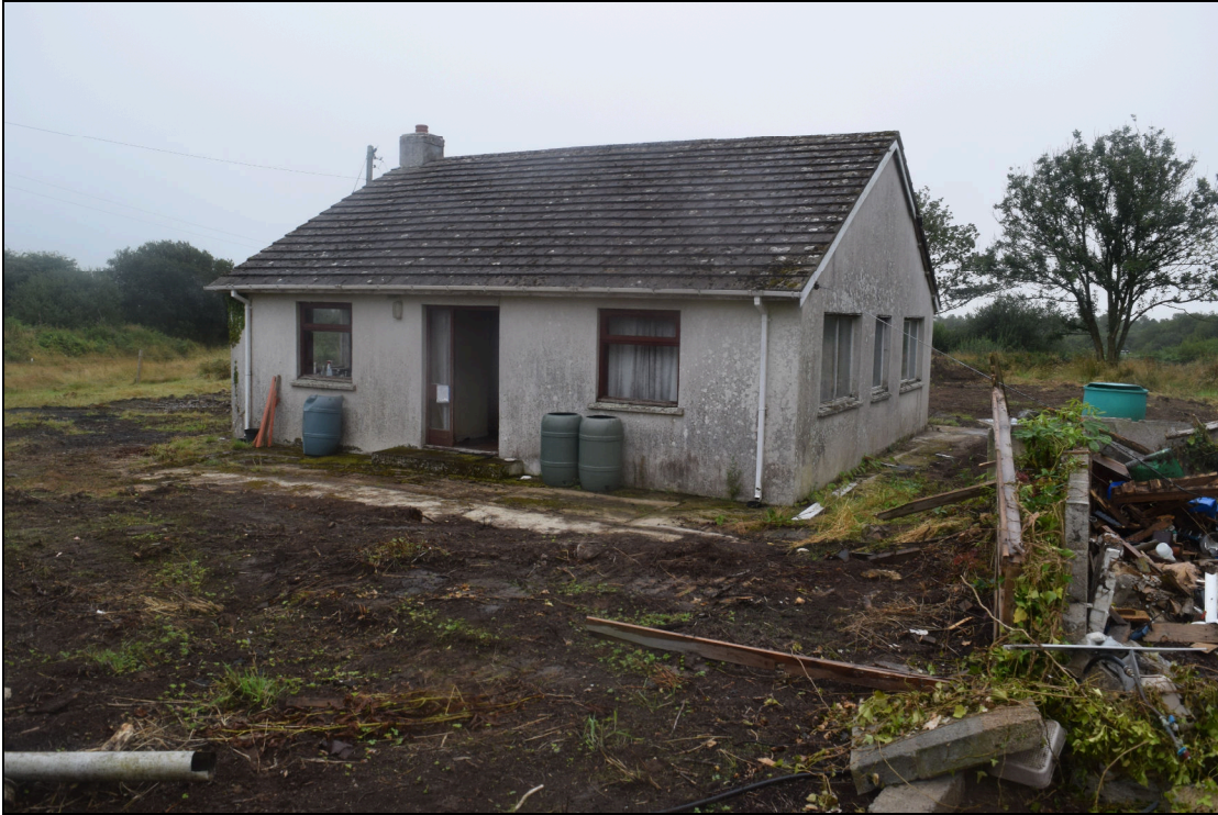
Plate 9: PCG2021_109, General view of the northern side of the plot and the front of the current house after vegetation scraped off but before topsoil (001) was removed, looking south.
