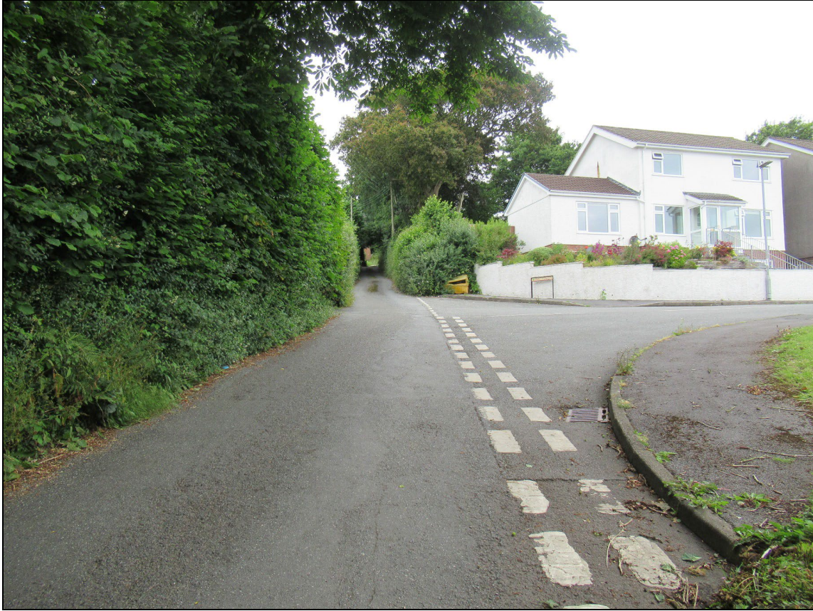
Plate 9 – PYD2024_009: A view up Penlan Road at the junction with Parc y Delyn, showing the narrow roadway leading up the hill. Looking north-northwest.
