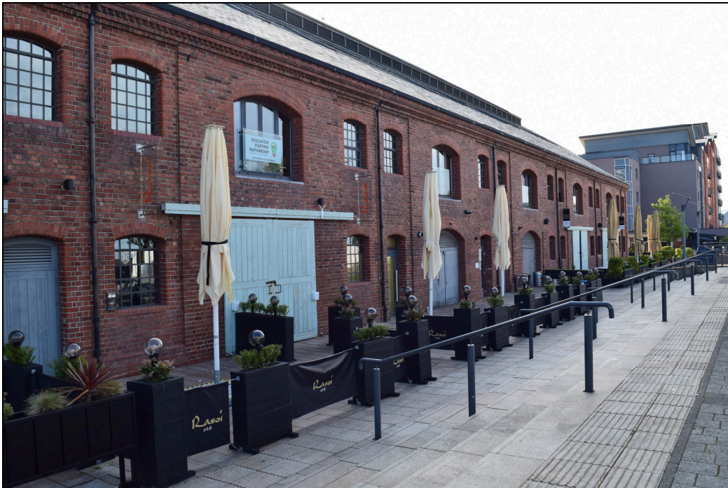
Plate 15: RAS2021_015. A view of the western side of Rasoi, showing the sliding doors of the entrance and the uncovered exterior seating area. Looking southeast.
