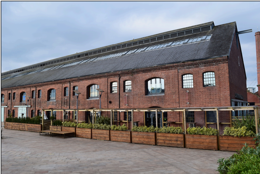
Plate 3: RAS2021_003. A view of the northern end of the J Shed showing an existing external pergola outside Unit 1 of the building. Looking south-southwest.
