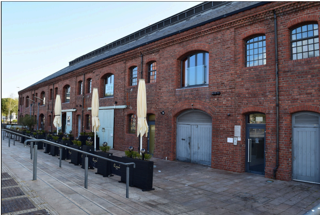
Plate 14: RAS2021_014. A view of the western side of Rasoi, showing a pair of sliding doors and the uncovered exterior seating area. Looking north-northeast.
