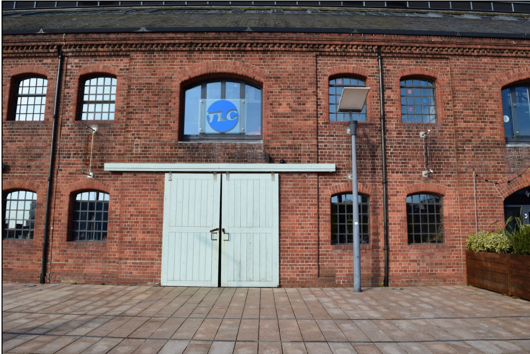
Plate 6: RAS2021_006. A view of the northern set of sliding doors into Rasoi. These doors are defined as "original" by the listing description but they do not match the appearance of the doors seen in historic photographs and are likely to be late 20 th century or early 21 st century additions. Looking southwest.
