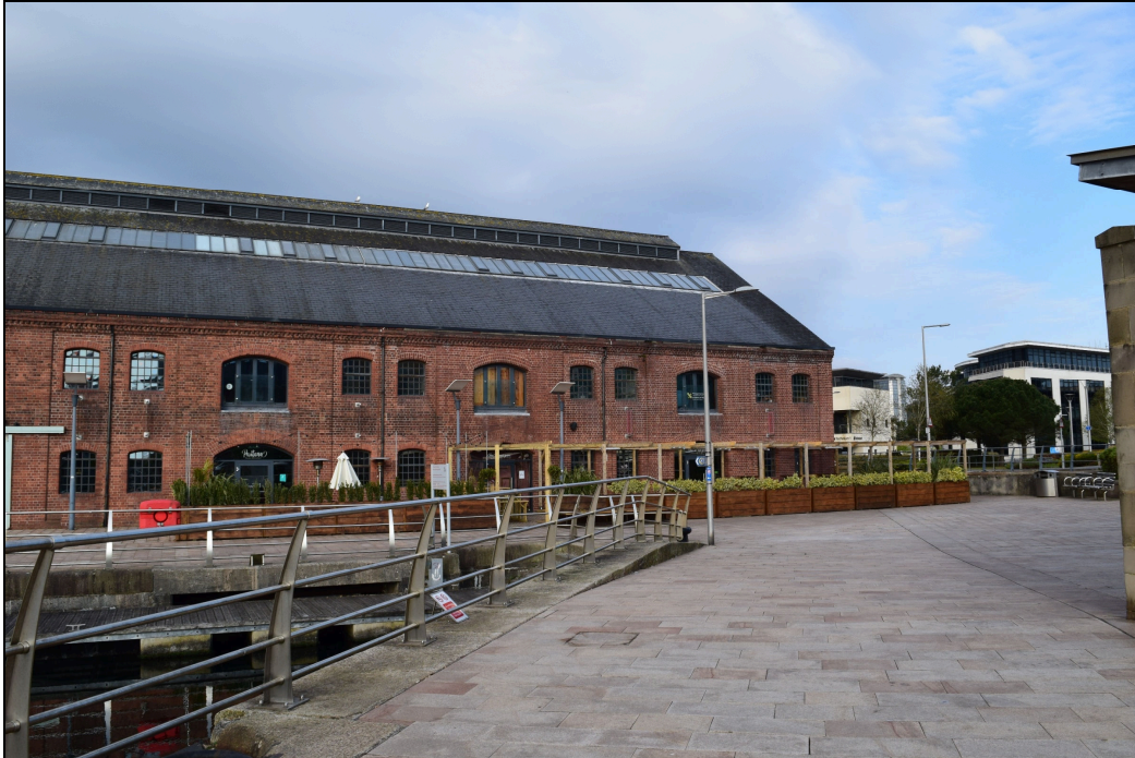
Plate 1: RAS2021_001. A view of the northern end of the J Shed showing an existing external pergola outside Unit 1 of the building. The building was converted in 2005 which included addition of the row of skylights and the ridgeline ventilation. Looking west.
