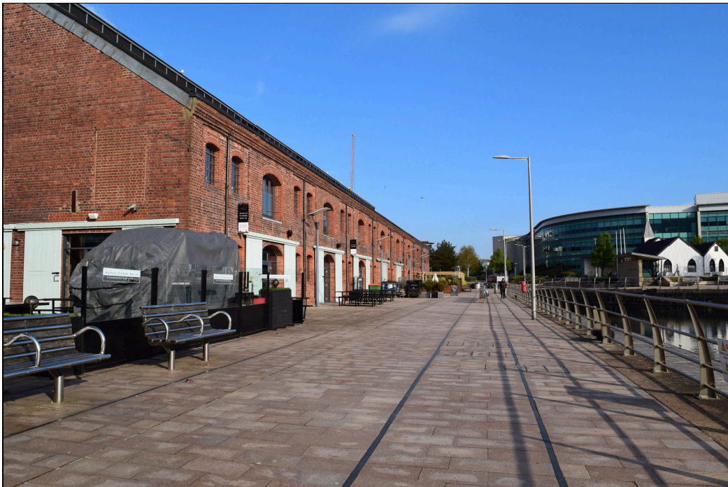
Plate 10: RAS2021_010. A view along the eastern side of the J Shed showing exterior street furniture. The pergola outside Unit 1 is visible at the far end of the building and the closed doors of Rasoi are seen at the centre of the image. Looking northwest.
