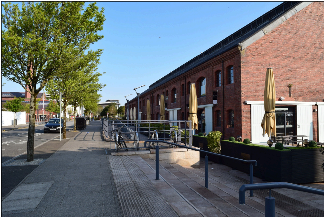
Plate 13: RAS2021_013. A view along the western side of the J Shed. The sliding doors in the gable end must post-date the demolition of a building which stood abutting the J Shed until the later 20 th century, suggesting all the sliding doors are relatively recent additions and not original. Looking northwest.
