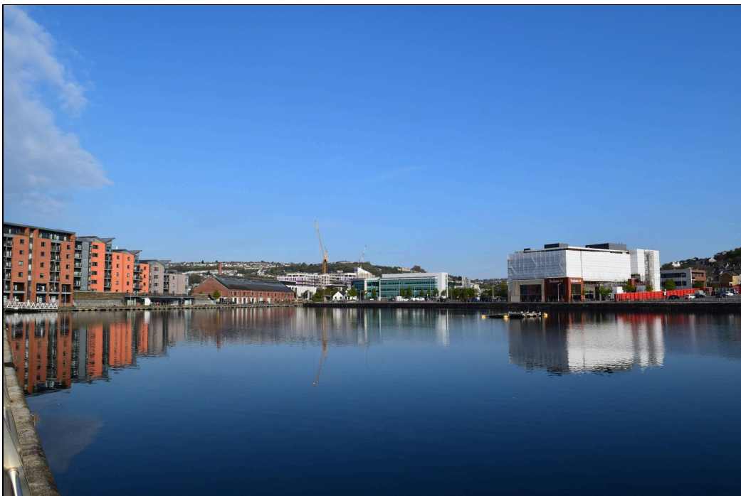
Plate 12: RAS2021_012. A view across the Prince of Wales Dock towards the J Shed which is seen to the left of centre in the image. Modern development dominates the view. Looking west-northwest.
