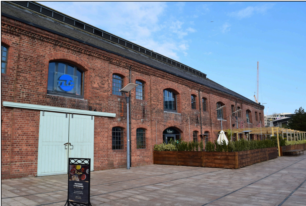
Plate 5: RAS2021_005. A view along the eastern side of the J Shed. A closed pair of sliding doors at Rasoi are to the left. With the exterior planting boxes of Unit 2 beyond and the pergola outside Unit 1 to the right. The exterior seating area of Rasoi would continue the line of external additions to the building. Looking west-northwest.
