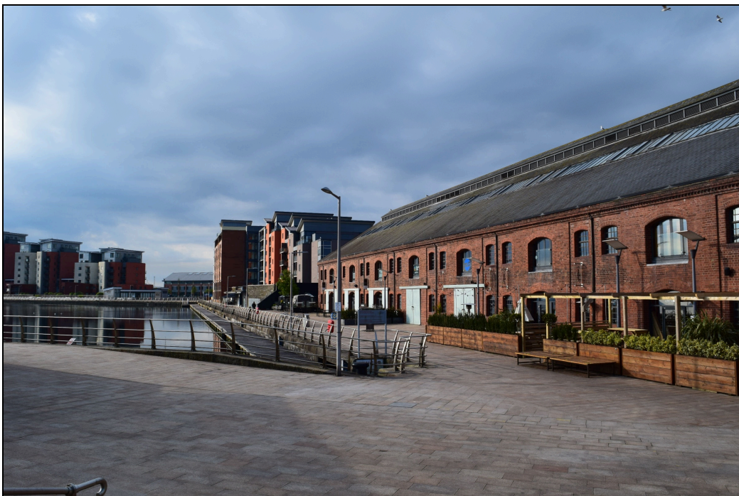
Plate 4: RAS2021_004. A view along the eastern side of the J Shed with the Prince of Wales Dock to the left. The closed sliding doors of Rasoi are right of centre. Note the pergola outside Unit 1 to the right and exterior planting boxes of Unit 2 beyond the pergola. The exterior seating area of Rasoi would continue the line of external additions to the building. Looking south-southeast.
