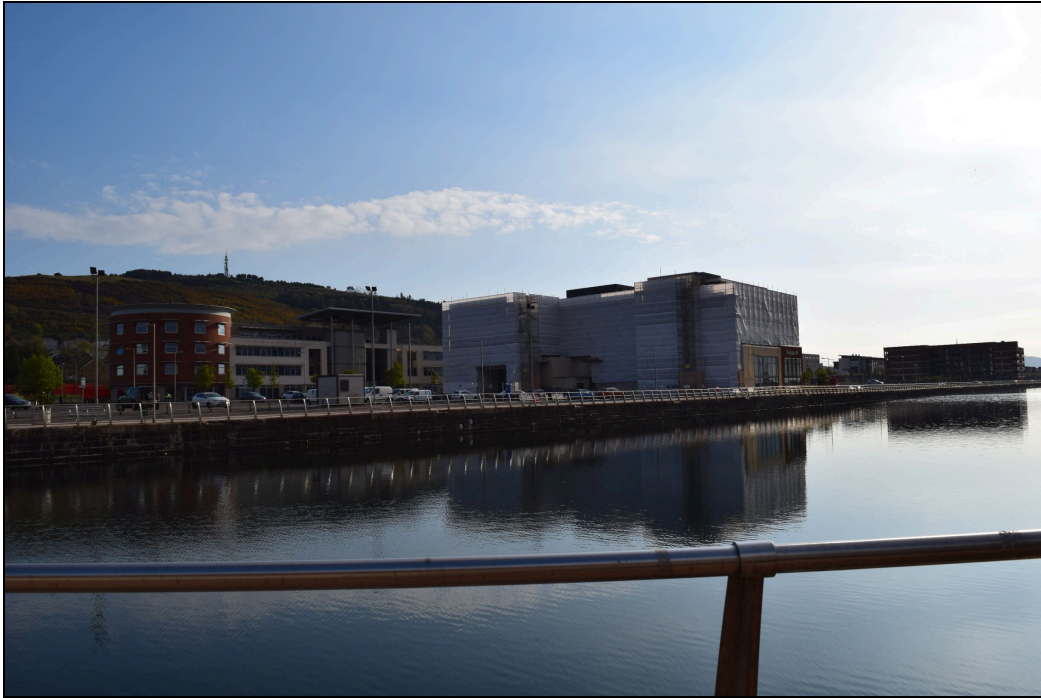
Plate 9: RAS2021_009. A view across the northern side of the Prince of Wales Dock from the promenade outside Rasoi, showing new developments at the dock side. Looking east-northeast.
