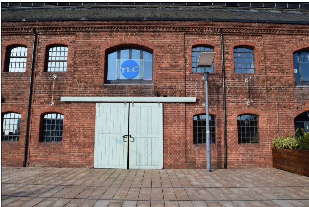
Plate 6: RAS2021_006. A view of the northern set of sliding doors into Rasoi. These doors are defined as "original" by the listing description but they do not
