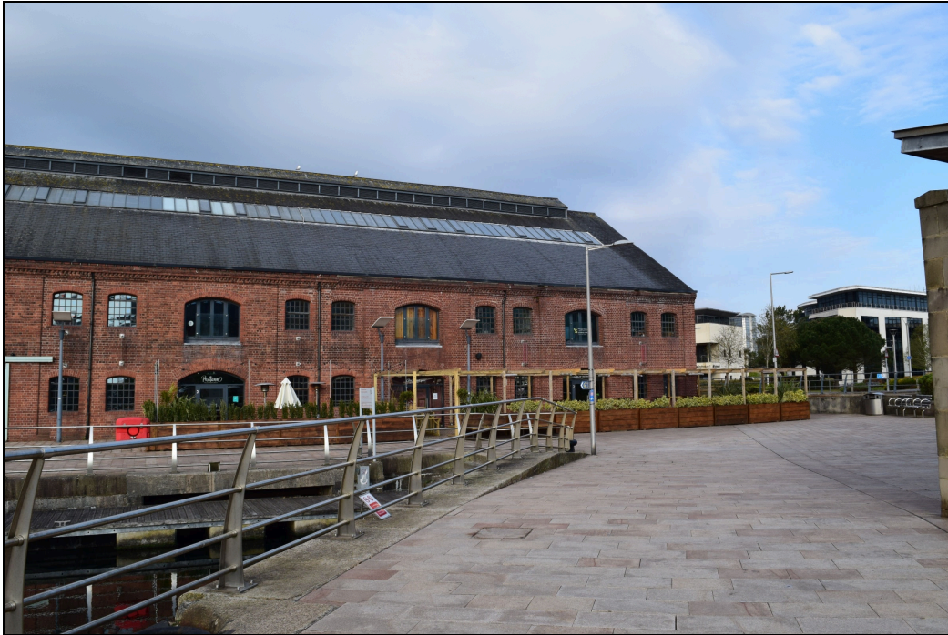
Plate 1: RAS2021_001. A view of the northern end of the J Shed showing an existing external pergola outside Unit 1 of the building. The building was converted in 2005 which included addition of the row of skylights and the ridgeline ventilation. Looking west.
