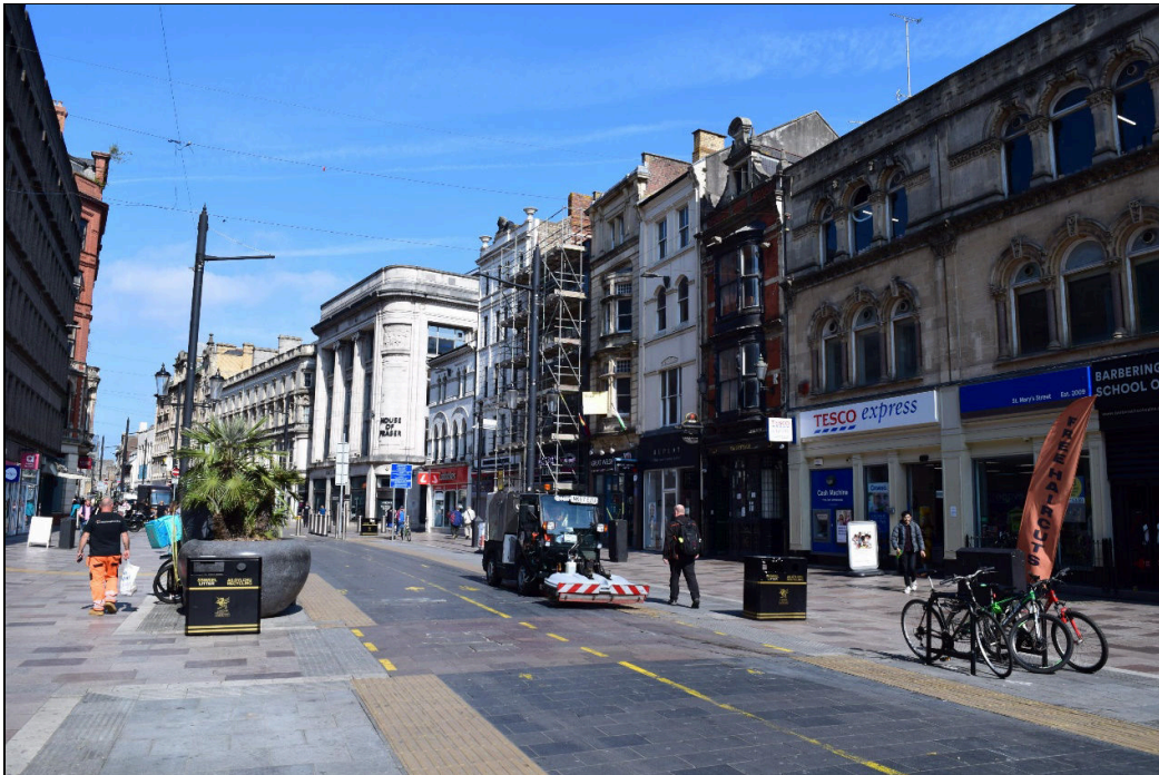
Plate 2: A view northwards along St. Mary Street. The scaffolding in front of No.22 is seen at the centre of the image. The large grey building left of centre is the Grade II* listed Howells Department Store (Listed Building Number 14109), which is built in Portland Stone. The proposed new façade on No.22 will include a render matched to the colour of Portland Stone.
