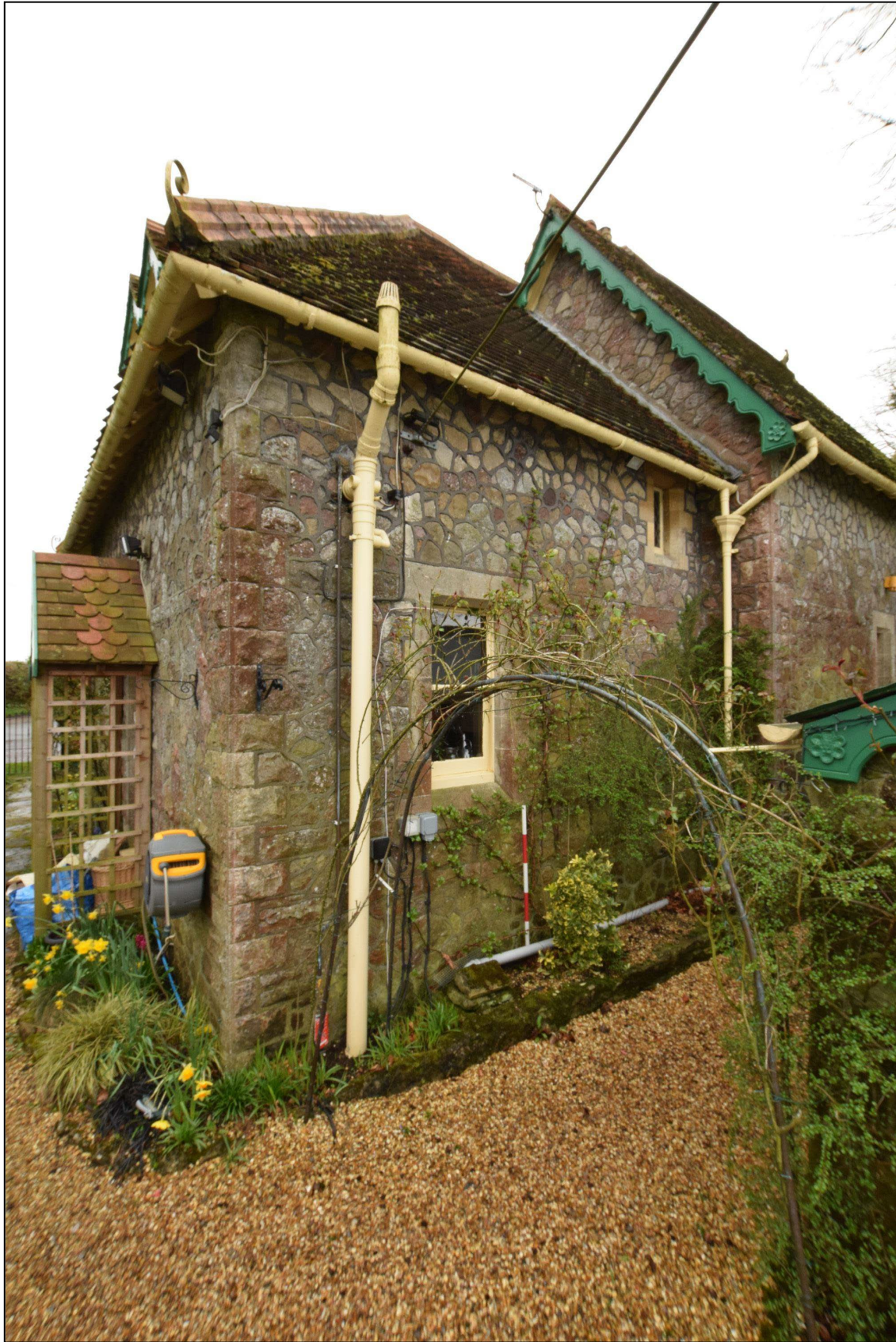
Plate 6: TFR2023_032. A view of the eastern end of the north-facing or rear elevation. Looking southwest. This is the area which will be physically impact by the glass linking walkway between the lodge and the new extension. The larger window will become a door way and the wall above it removed with an insert into the roof.
