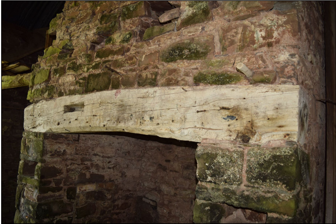
Plate 19: YTB2022_019. A view of the oak beam above the fireplace. The timber has clearly been reused from another building or an earlier iteration of the building. Looking southeast.
