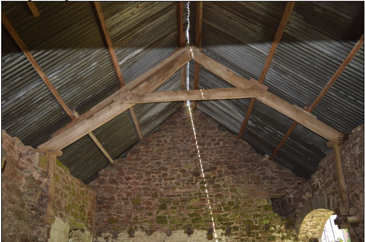
Plate 22: YTB2022_022. A view of the internal wall which divides the parts of the inside the building, showing a simple A-frame oak roof truss which is wooden pegged and rests on wooden pads at wallplate level at either side. Looking north-northwest.
