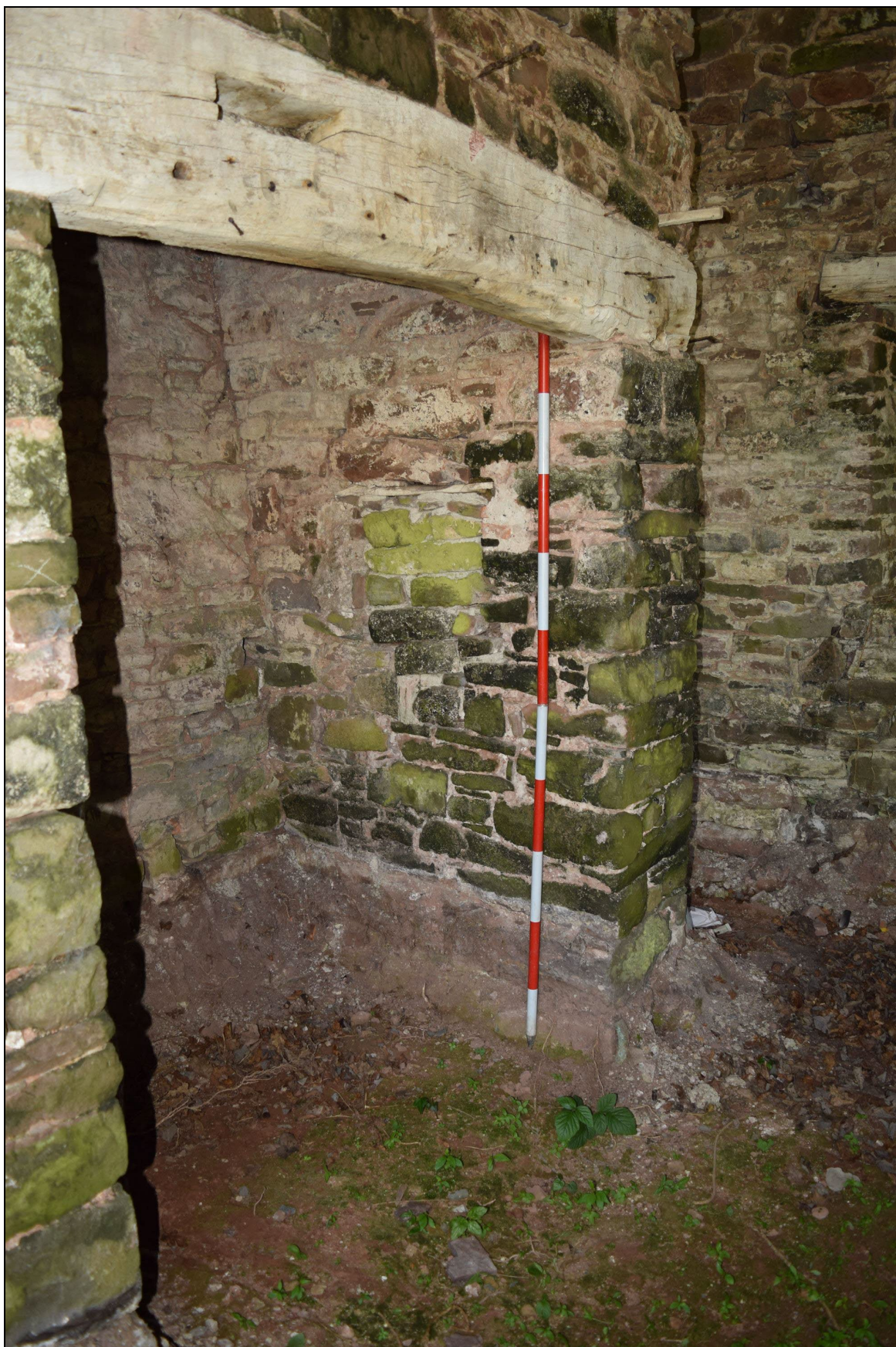
Plate 14: YTB2022_014. A view inside the southern fireplace showing a now blocked-up niche inside the fireplace, left of centre. Note the recycled timber used for the beam above the hearth. Looking southwest.
