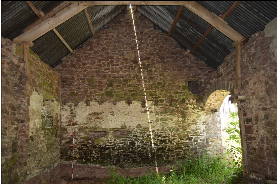
Plate 21: YTB2022_021. A view of the internal wall which divides the two parts of the building. Note the line of joist holes across the wall which is evidence there was formerly a loft inside the building. Sawn-off beams can be seen either side of the building. Looking north-northwest.
