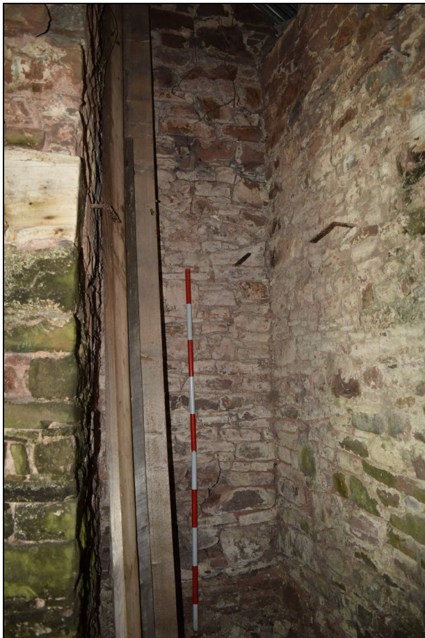
Plate 19: YTB2022_019. A view of the oak beam above the fireplace. The timber has clearly been reused from another building or an earlier iteration of the building. Looking southeast.
