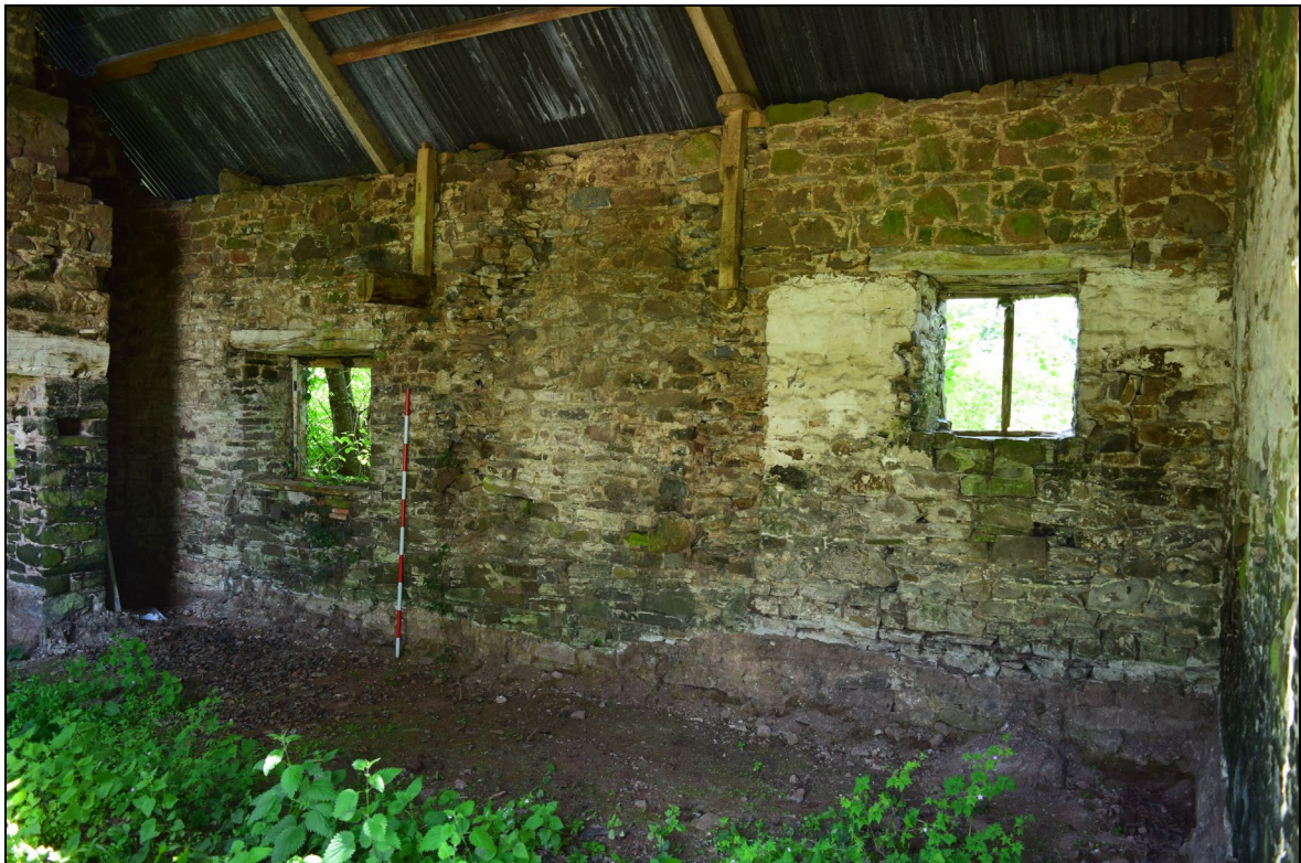
Plate 24: YTB2022_024. A view of the western lateral wall inside the southern end of the building, showing two splayed windows. At the centre is the scar of a former chimney which originally located against this wall. Note the floor has been removed in the past. Looking southwest.
