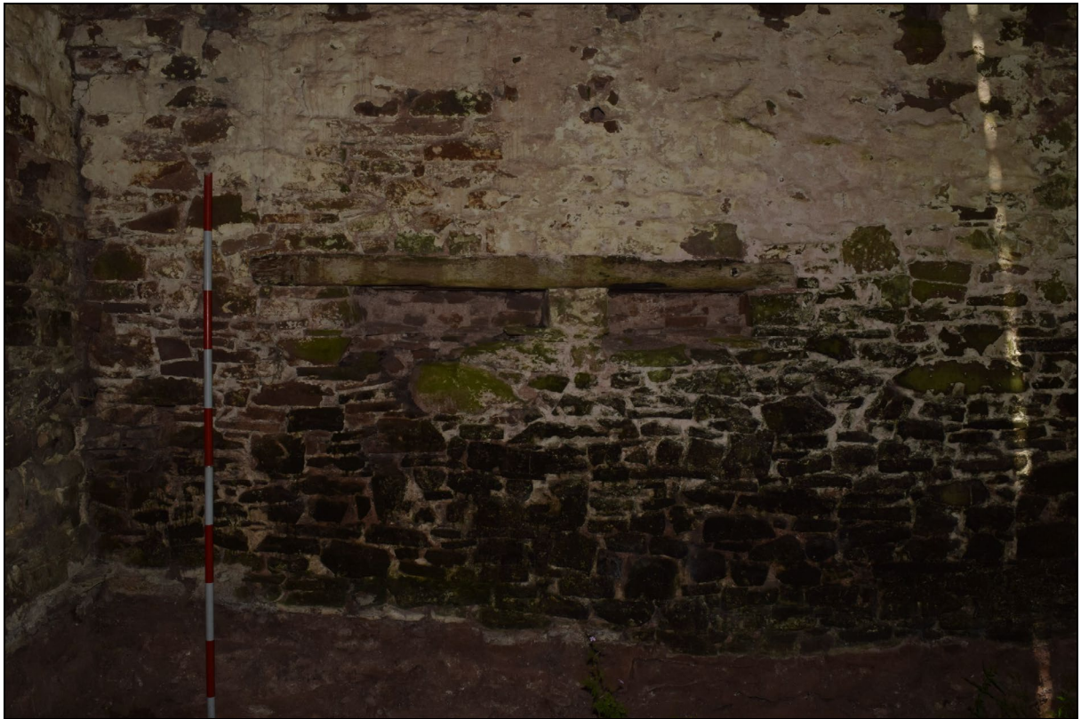
Plate 23: YTB2022_023. A view of niches built into the internal wall inside the southern part of the building, beneath a wooden lintel. Looking north-northwest.
