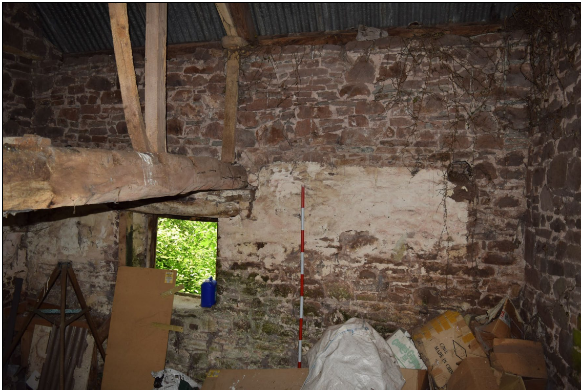
Plate 38: YTB2022_038. A view of the western lateral wall at the northern end of the building showing the heavy beam supporting the loft floor resting on the wooden lintel of the window. Note a sawn-off beam to the right, evidence of a beam which formerly supported the loft floor. Looking southwest.
