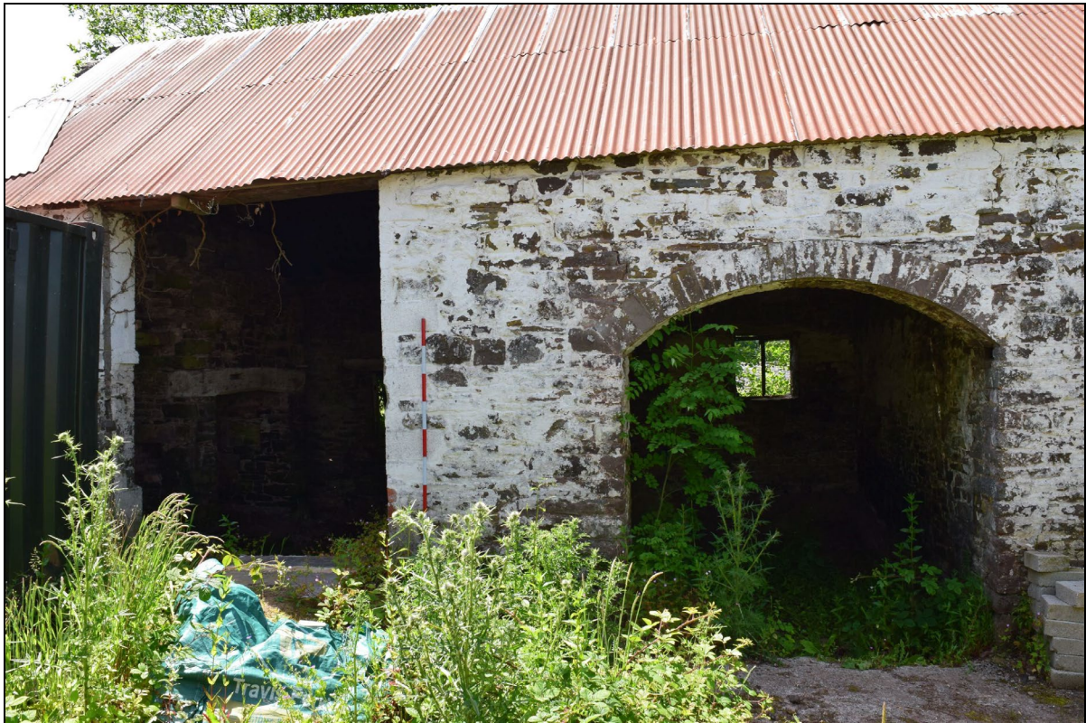
Plate 3: YTB2022_003. A view of the southern end of the east-facing façade of the building showing the two entrances. The arch to the right is original the larger opening to the left appears to have been enlarged in modern times. Looking west-southwest.
