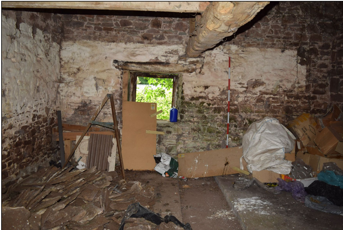
Plate 37: YTB2022_037. A view inside the northern section of the building, showing the window through the western lateral wall. The beam and a joist of the loft can be seen at the top of the image. Note the 20 th century concrete floor with a sunken walkway through its centre. Looking west-southwest.
