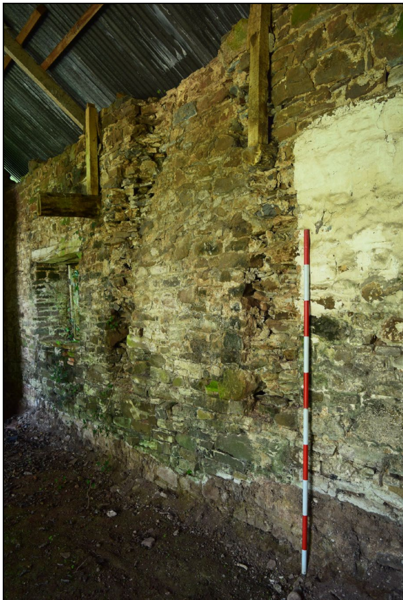
Plate 26: YTB2022_026. A view of the chimney scar against the western lateral wall. Looking south. Note that the scar starts c. 1.10 metre above the current surface. Looking south.
