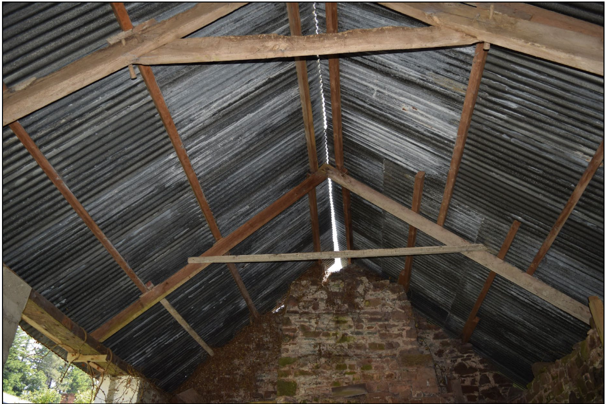
Plate 33: YTB2022_033. A view of the roof inside the southern part of the building, showing a modern A-frame truss. Looking south-southeast.
