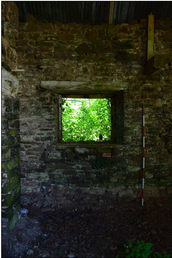
Plate 25: YTB2022_025. A view of the southern window through the western lateral wall. Note the wooden lintel and the sawn-off beam to the right. Looking west-southwest.
