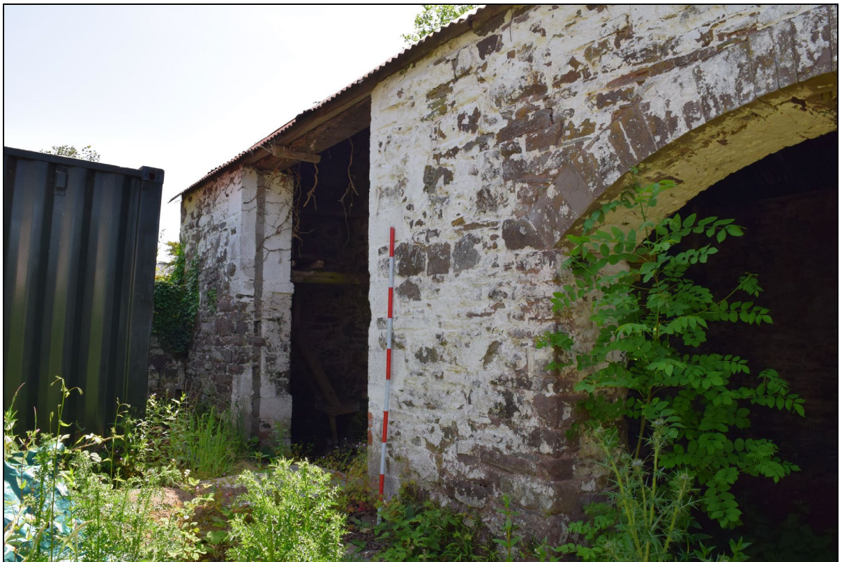
Plate 2: YTB2022_002. A view of the southern end of the eastern-facing façade of the building. The large opening seen left of centre shows evidence of having been enlarged in modern times as concrete blockwork is seen either side of the opening. Looking south.
