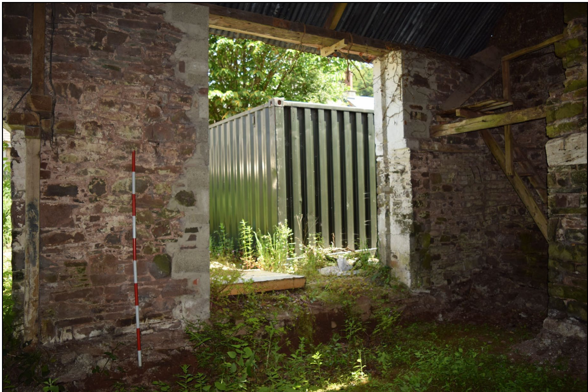
Plate 32: YTB2022_032. A view looking outwards through the large entrance doorway in the east-facing façade at the southern end of the building. Modern blockwork either side of the opening suggests there was an earlier entrance here, which has possibly been widened and heightened. Looking east.
