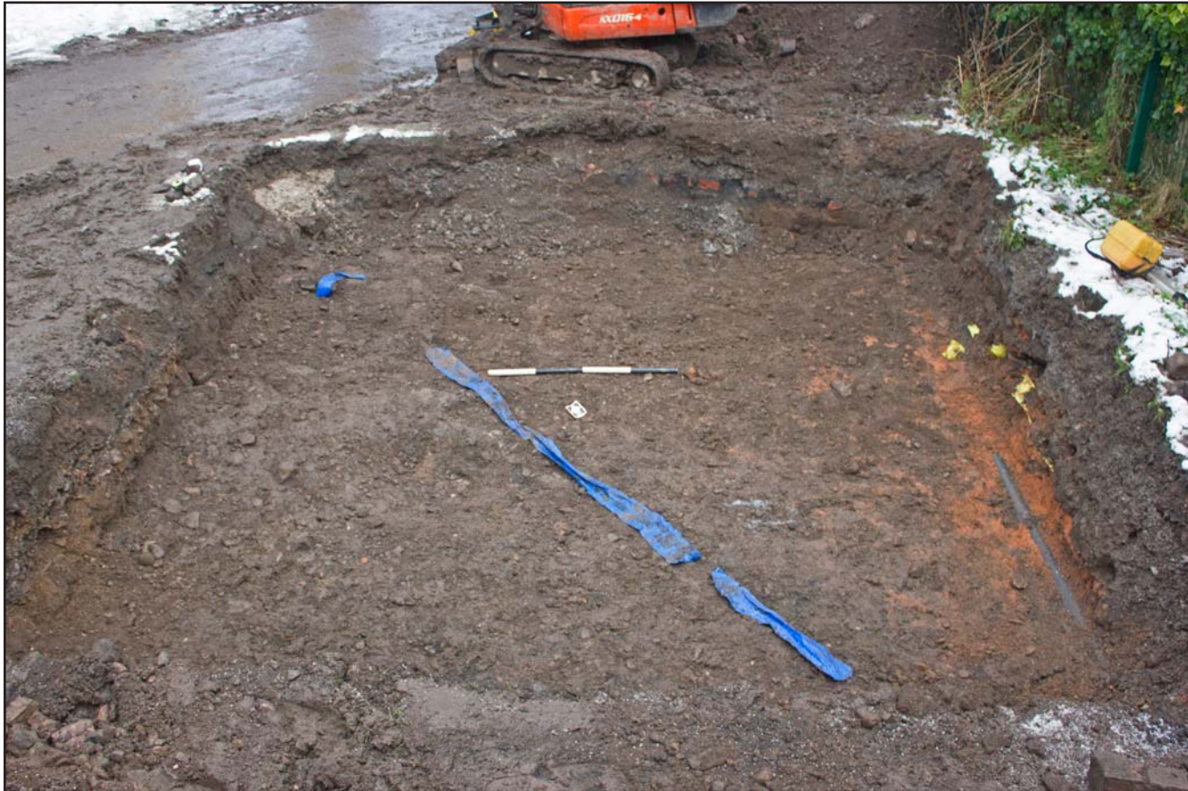
Plate 13: Post excavation shot of trench, Greenfield Valley Heritage Park, Greenfield, Holywell, Flintshire - from the southwest - 1.00m scale
