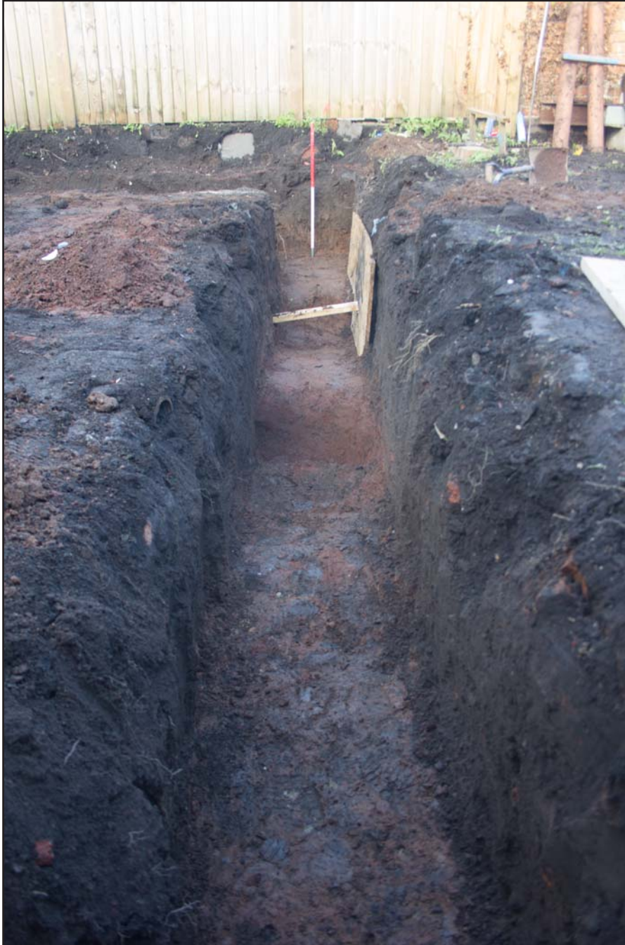
Plate 07: Plan shot - Trench B, at Bridgewater, Church Street, Holt, Wrexham - from the north - 1.00m
