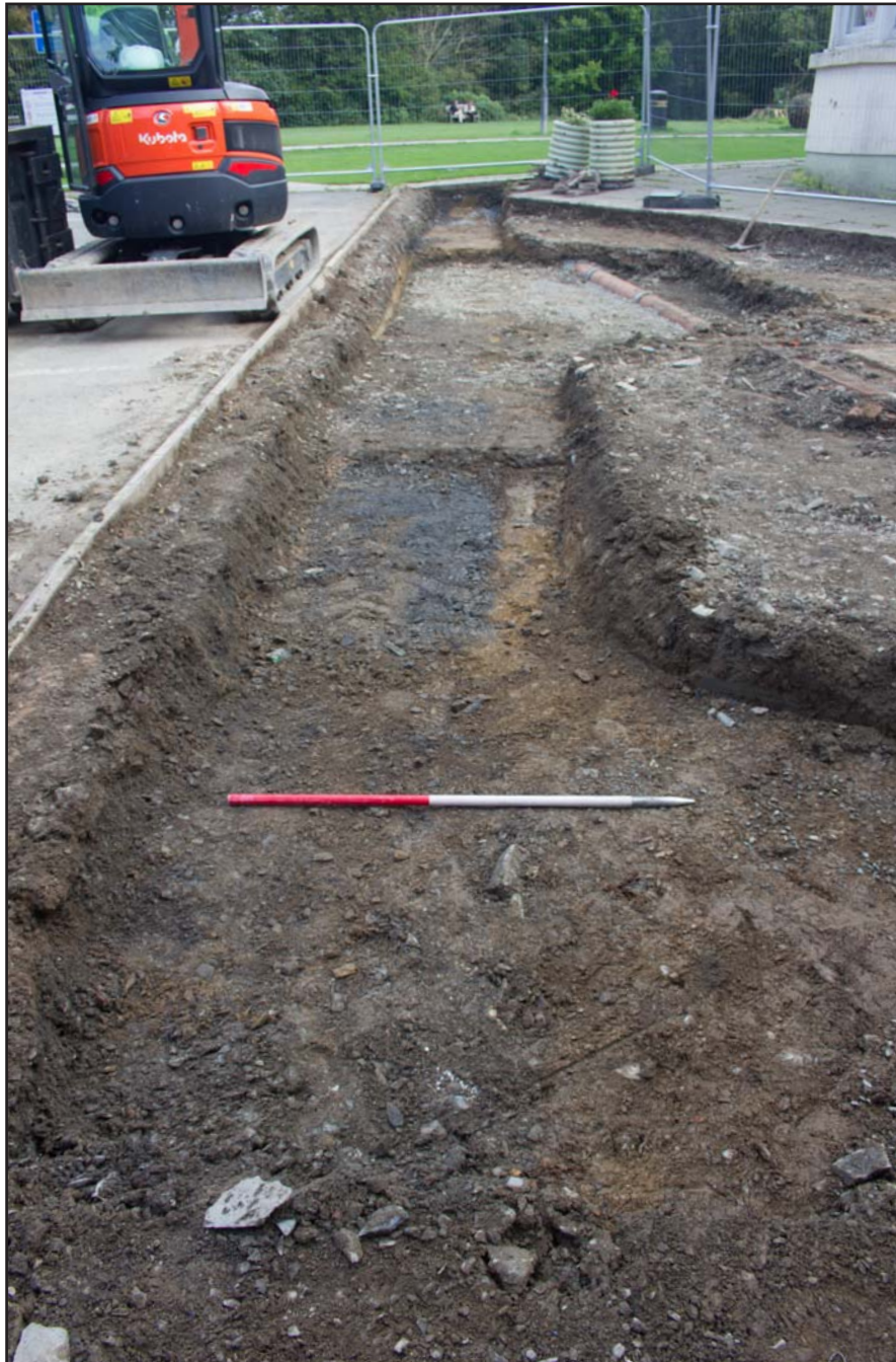
Plate 08: Wall foundation within development area, Y Plâs, Community Centre, Machynlleth, Powys - from the northwest - 1.00m
