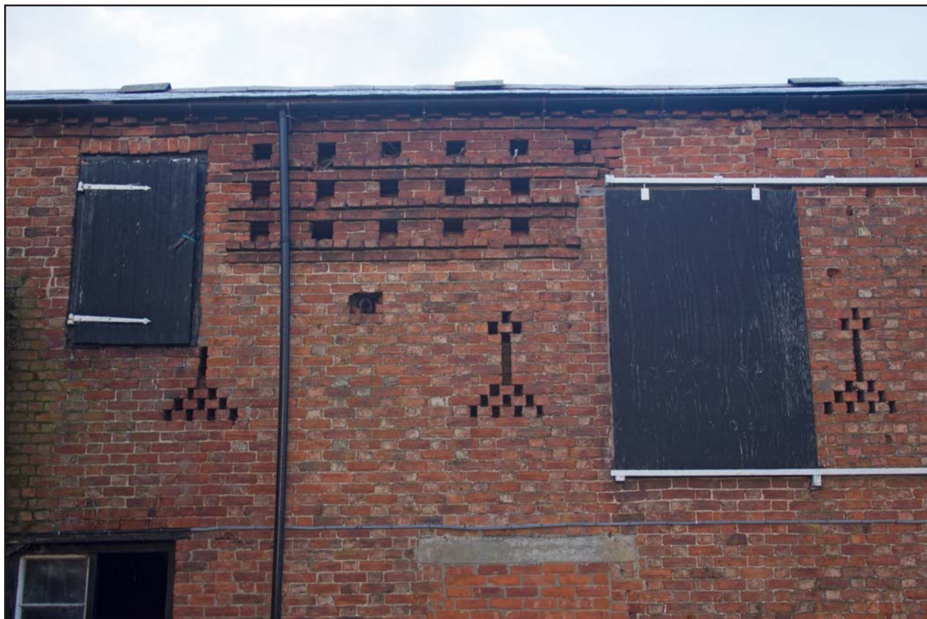
Plate 10: Dovecote and embrasures in SE of northern barn, at Lower Farm, Lower Farm Road, Bowling Bank, Wrexham - from the southeast - 2.00m scale
