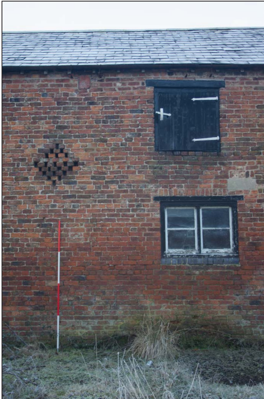
Plate 05: Example of embrasure, window and loft hatch in NE elevation, at Lower Farm, Lower Farm Road, Bowling Bank, Wrexham - from the northeast - 2.00m scale
