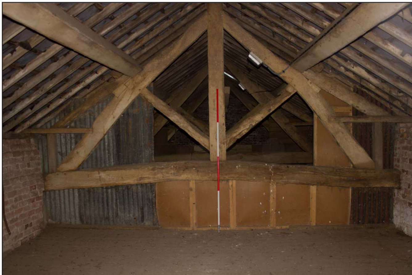
Plate 33: Stall/partition incorporated into (south barn) roof truss, at Lower Farm, Lower Farm Road, Bowling Bank, Wrexham - from the northwest - 2.00m scale
