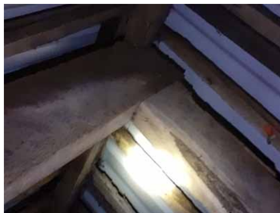
Photo 2: Truss 4: upper cruck with type E apex
