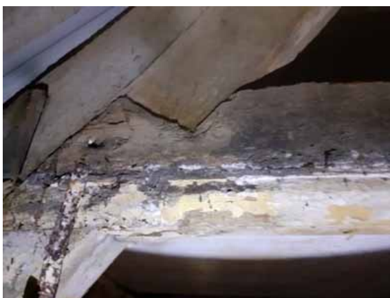
Photo 3: A notched-lap halved joint with simple entry
